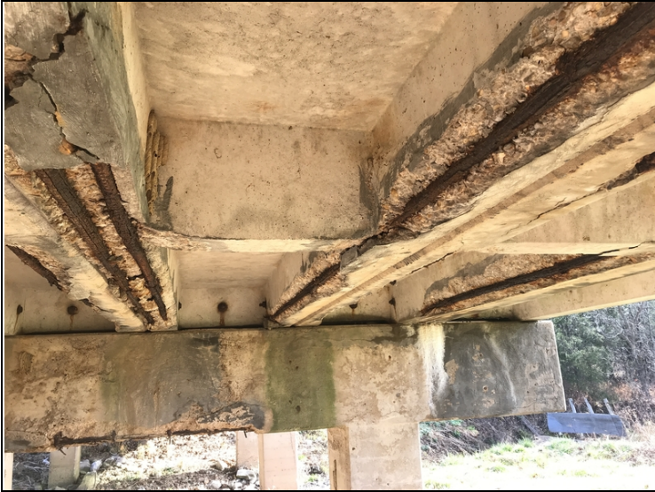
Large spalls with rebar exposed to girders: Span 2 - Units 3 ,4, 5, 6.
