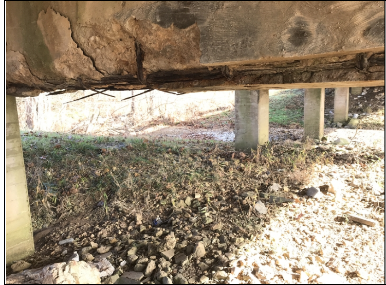
Areas of delamination, large deep spalls with rebar exposed & heavy cracking to concrete caps at Bent 1, 2, 3, & 4. Bent 1.
