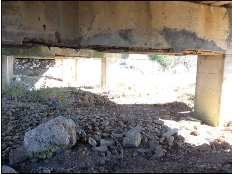
Typical of Delaminating areas with large deep spalls with rebar exposed to bottom of cap between columns at Bents 1, 2, & 3.
