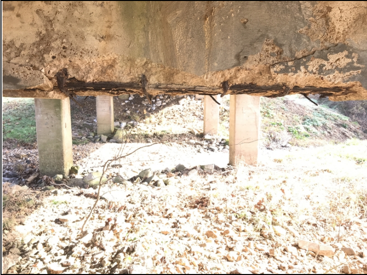
Areas of delamination, large deep spalls with rebar exposed & heavy cracking to concrete caps at Bent 1, 2, 3, & 4. Bent 2.
