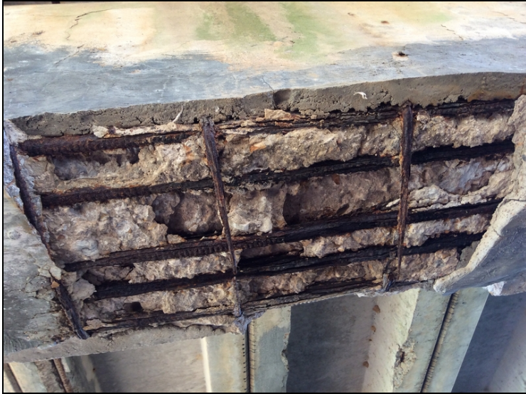
Delaminating areas with large deep spalls with rebar exposed to bottom of cap between columns at Bents 1, 2, & 3.(Bottom of cap Bent 1)
