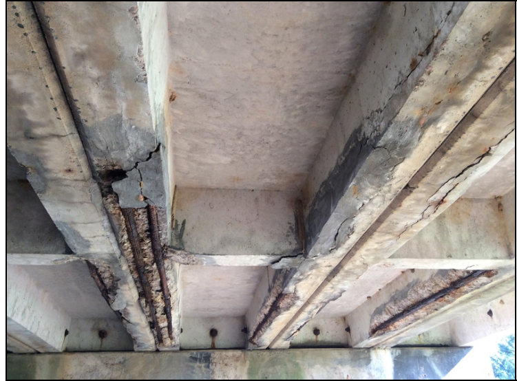
Typical of Spalls with rebar exposed to: Units 2, 4, 5, & 6 at Span 1. Units 3, 4, 5, & 6 at Span 2. Units 1 thru 7 at Span 3. Units 3, 4, 5, & 6 at Span 4. (Unit 5 Span 2)
