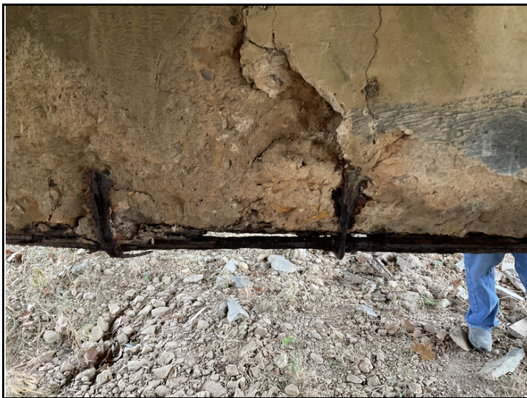
Spalls with rebar exposed with s/l & areas that are not adhered to concrete @ bottom of cap @ Bent 1.(#4)
