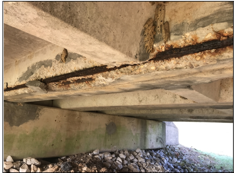
Large spalls with rebar exposed to girders: Span 1 - Units 2, 3, 4, 5, 6, 7.
