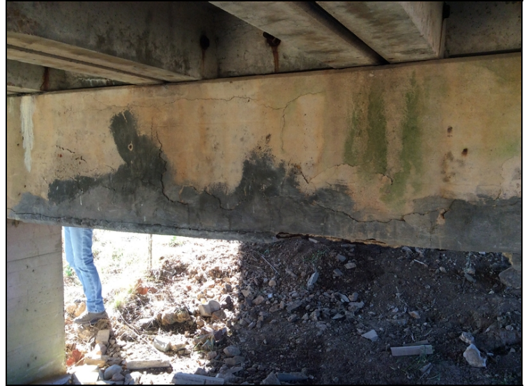
Typical of Caps at Bents 1, 2, & 3 have delaminated areas, cracks & heavy spalls with rebar exposed. (Ahead side Bent 1)
