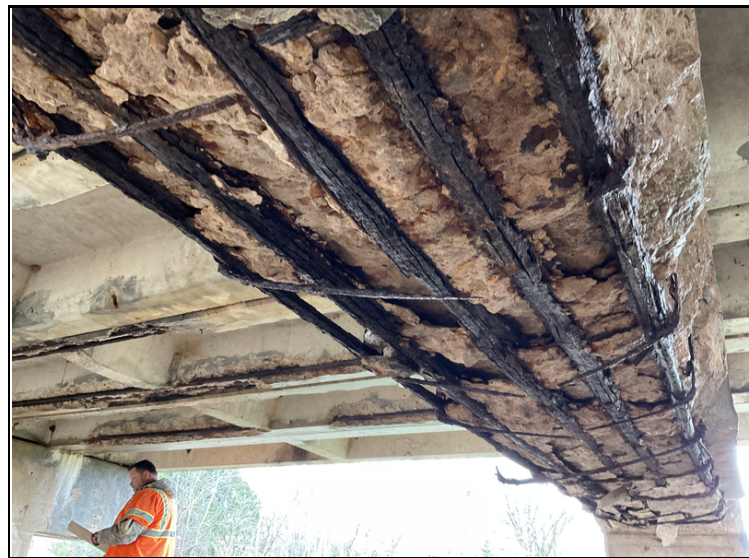
Spalls with rebar exposed with 100% s/l to bottom of cap @ Bent 1.(#4)
