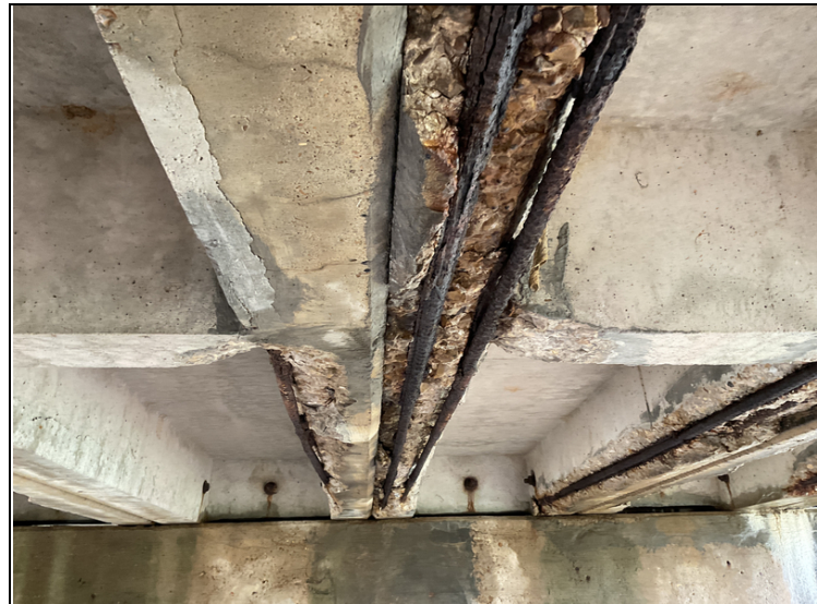
Spalls with rebar exposed with s/l @ areas not adhered to concrete @ Units 4 & 5 @ Span 2.
