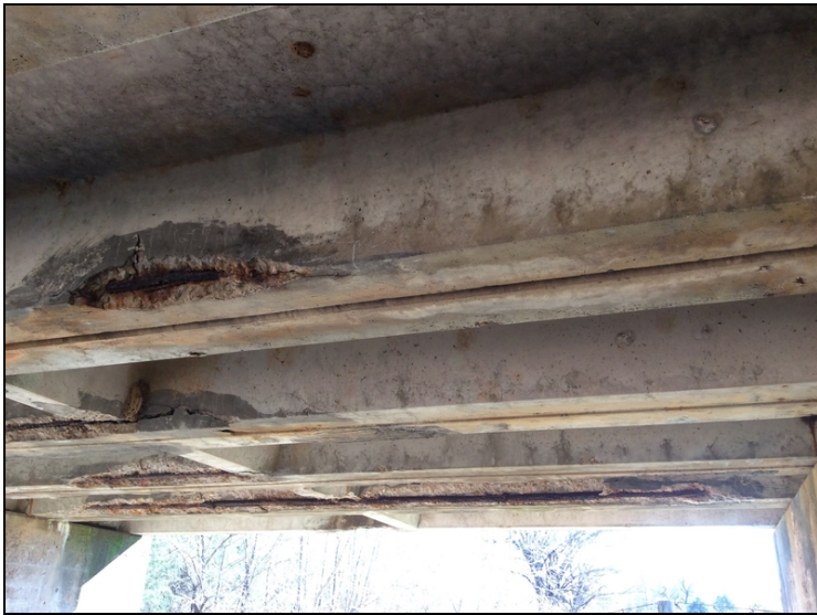
Typical of Spalls with rebar exposed to: Units 2, 4, 5, & 6 at Span 1. Units 3, 4, 5, & 6 at Span 2. Units 1 thru 7 at Span 3. Units 3, 4, 5, & 6 at Span 4. (Span 3)
