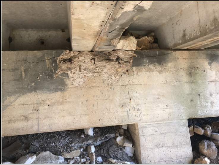
Spalls & cracking to Abutment 2.
