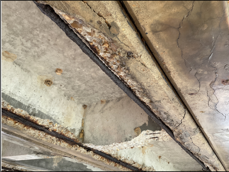
Spalls with rebar exposed with s/l @ areas not adhered to concrete @ Unit 6 @ Span 3.
