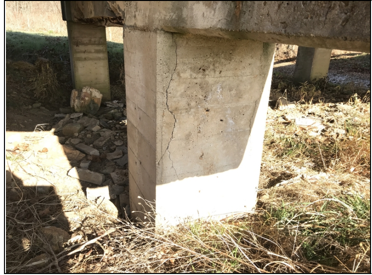
Vertical cracks to all columns at Bents 1 thru 4.
