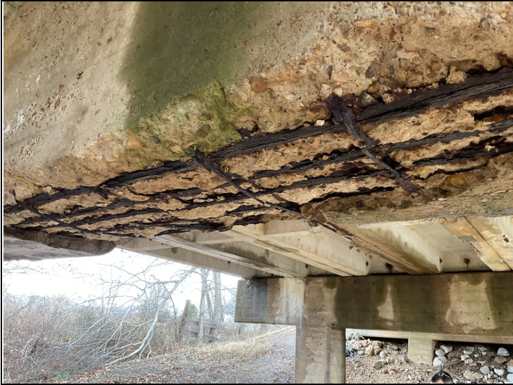
Spalls with rebar exposed with 100% s/l to bottom of cap @ Bent 3.(#4)
