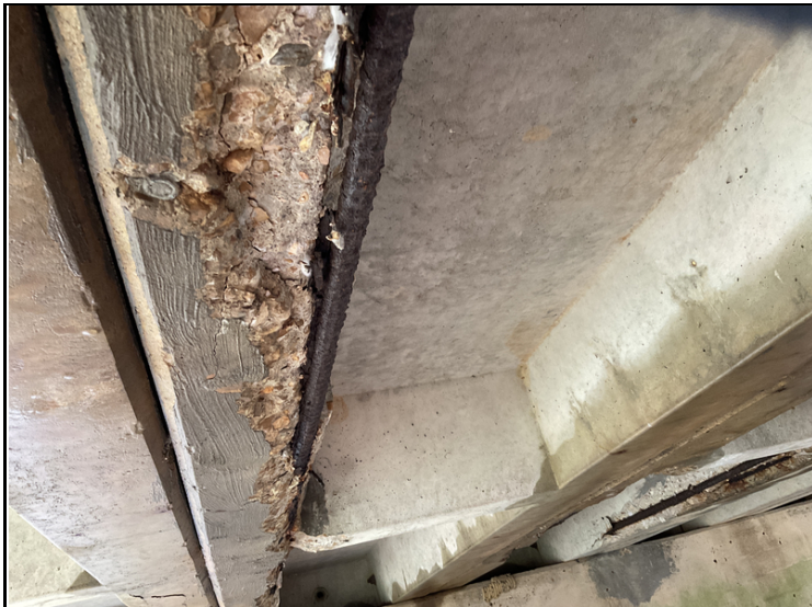
Spalls with rebar exposed with s/l @ areas not adhered to concrete @ Unit 6 @ Span 1.
