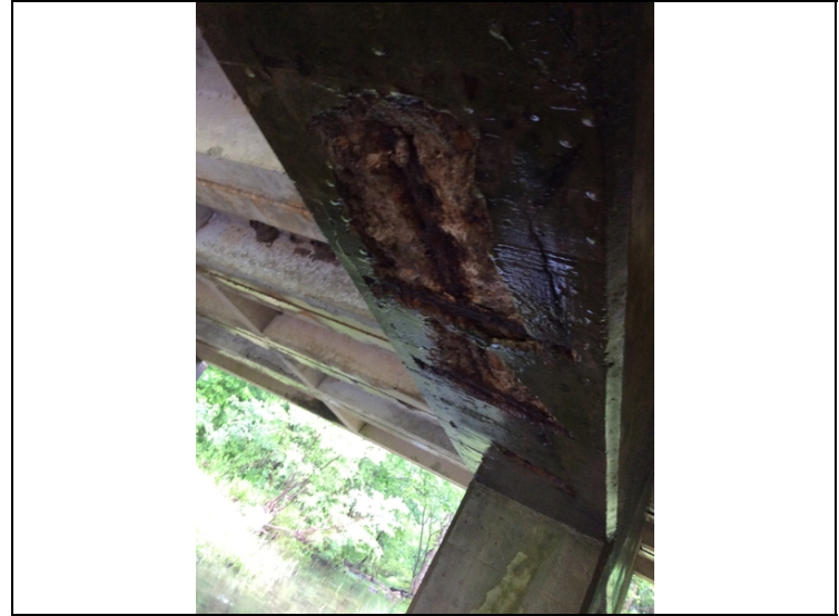
Spalling with rebar exposed & areas of delamination to Caps @ Bents 1 & 2.
