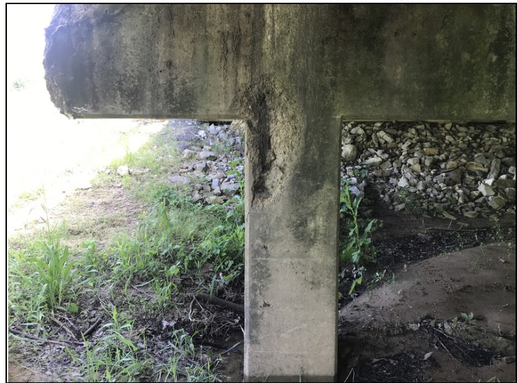
Cracking & spalls (some with reb. exposed) to Column 1-3 @ Bent 1 & 2.
