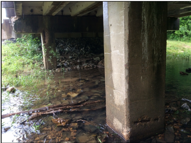
Cracking & spalls (some with rebar exposed) to Columns 1-3 @ Bents 1 & 2.
