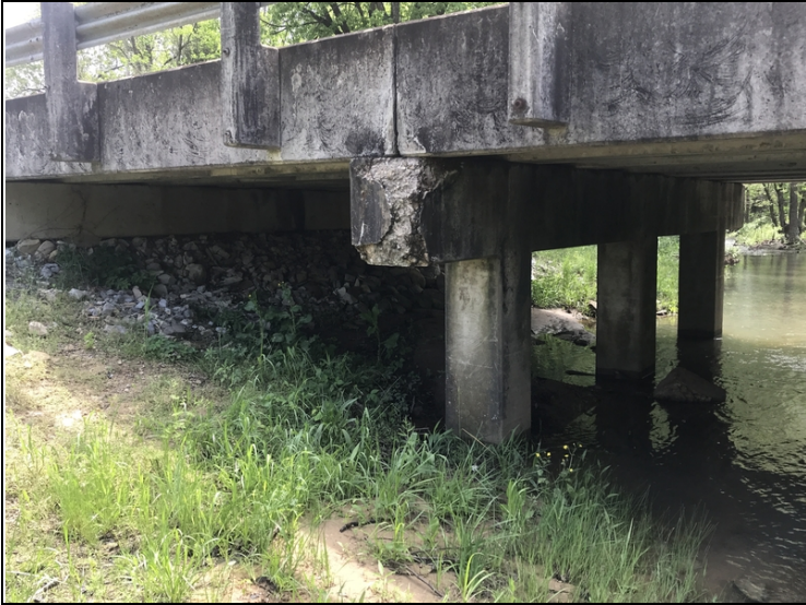
Heavy deterioration to left end of cap @ Bent 2
