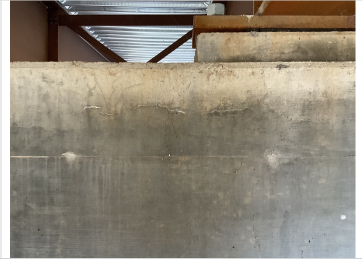
Horizontal efflorescent cracking to ahead side of cap @ Bent 1.(#2)
