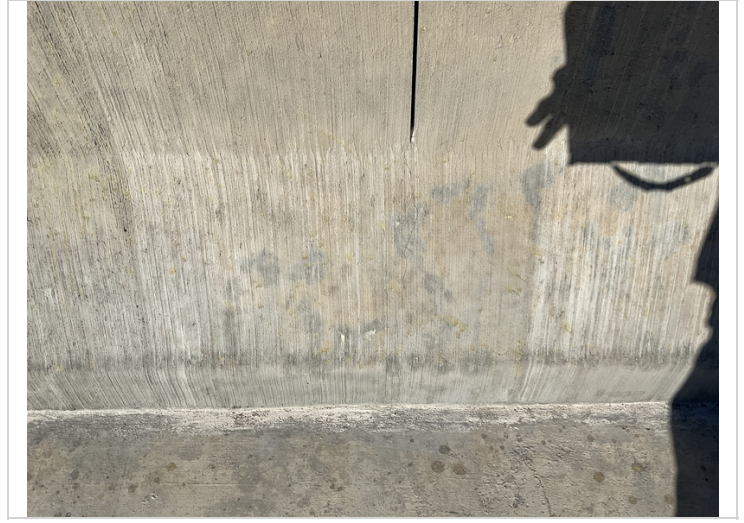
Vertical cracking to parapets.(#2 typical)
