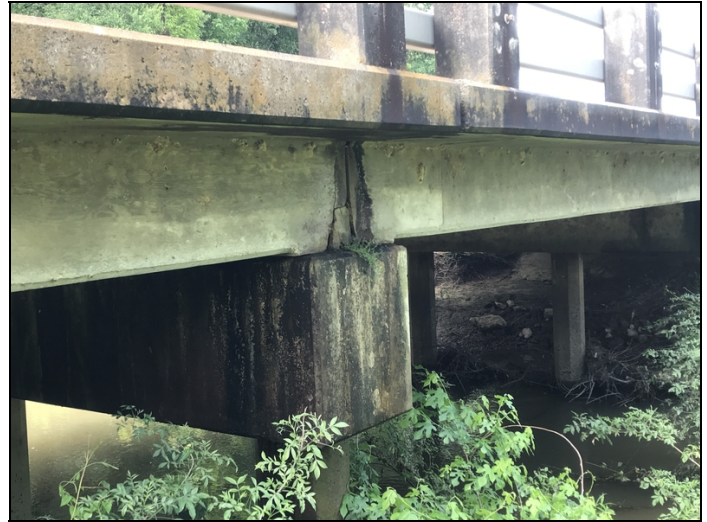
Cracks to Left & Right outside edge of Deck at Bent 1.
