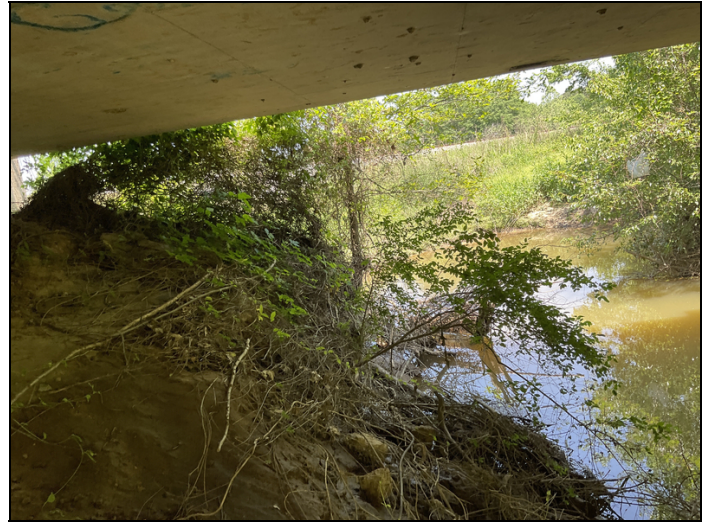
Erosion to embankment on Right side of Abutment 2.
