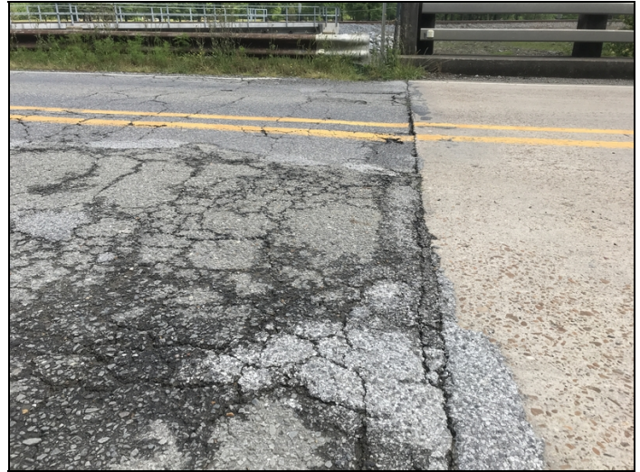
Visible settlement to Roadway at Abutment 2.
