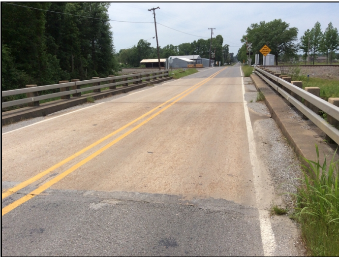
Debris in gutters at all spans.
