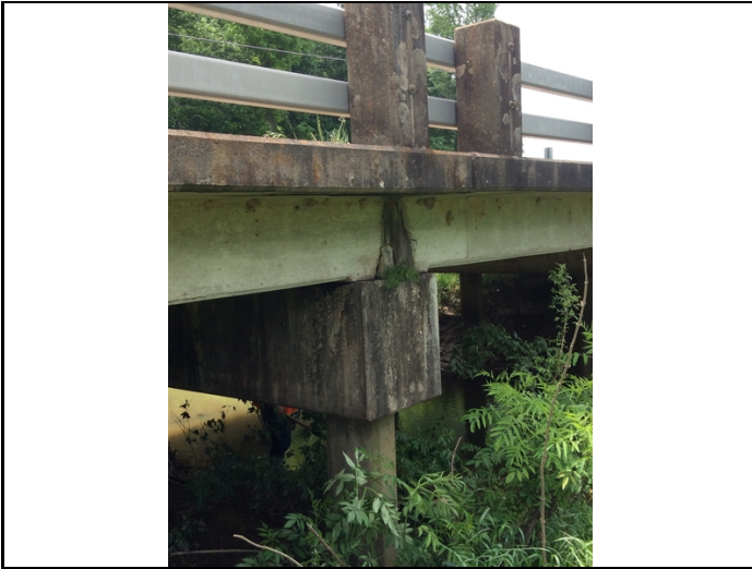
Cracking/spalls to Left & Right outside edge of Deck at Bent 1.
