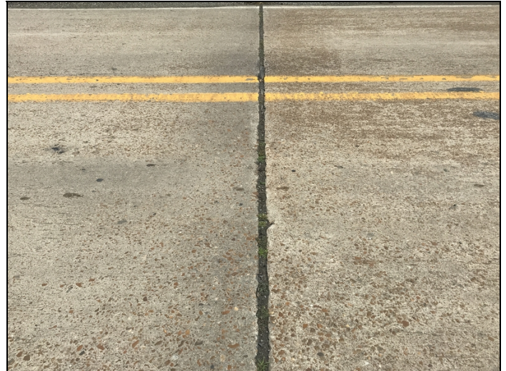
All poured joint seals are deteriorated & leak.
