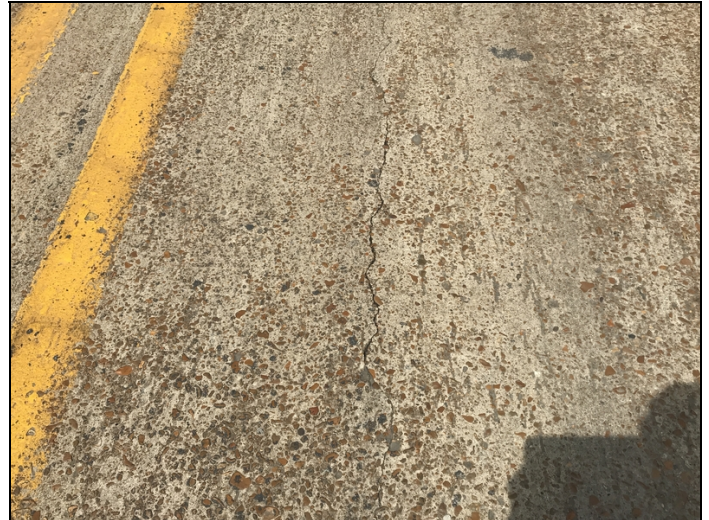
Unsealed cracks to Deck at Span 1, 2, & 3.
