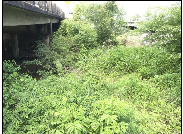
Sediment buildup on Right side of Span 2 restricting flow and realigning channel.
