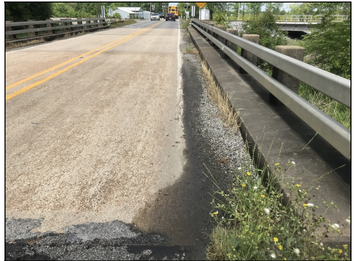
Debris in gutters at all spans.
