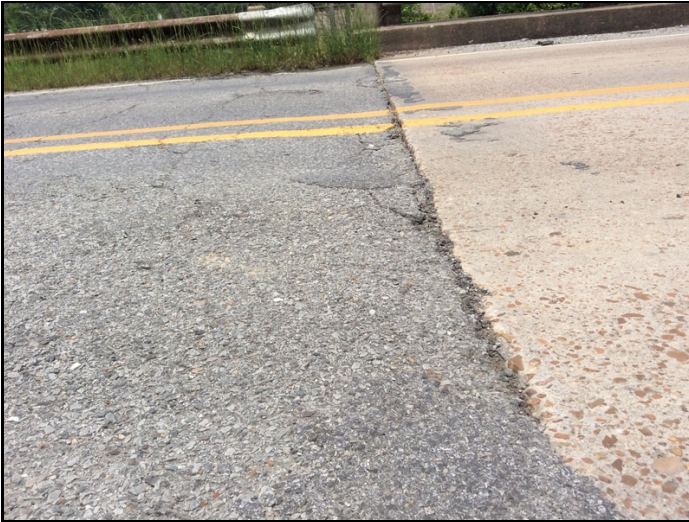
Visible settlement to Roadway at Abutment 2.
