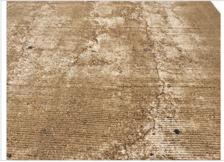
Span 5, longitudinal cracks.
