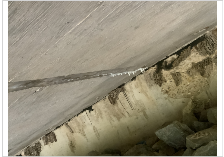
Span 1 soffit has cracks with efflorescence.
