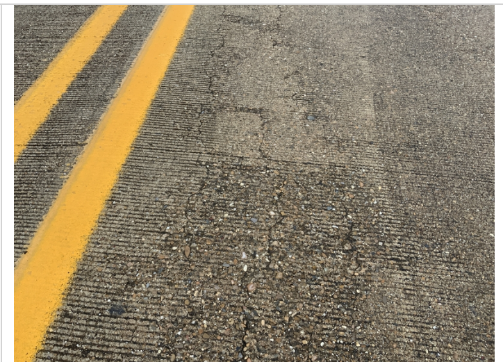
Deck span 1 has longitudinal cracks.
