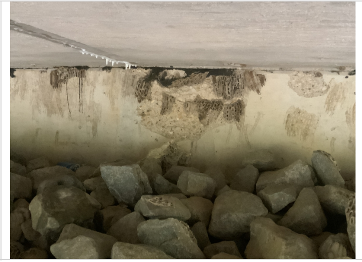
Bent 1 abutment has spall.
