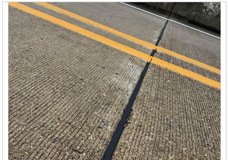
Bent 5 joint seal loss of bond, common all joints.
