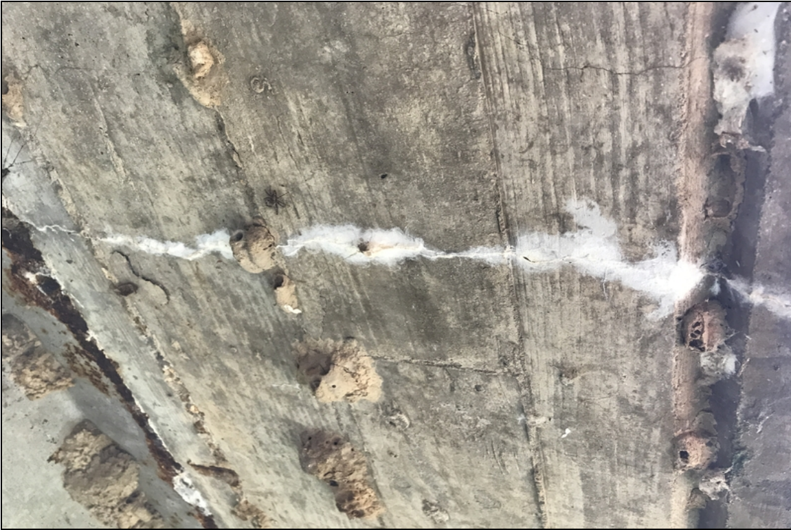
Typical cracks to Lt & Rt overhangs.
