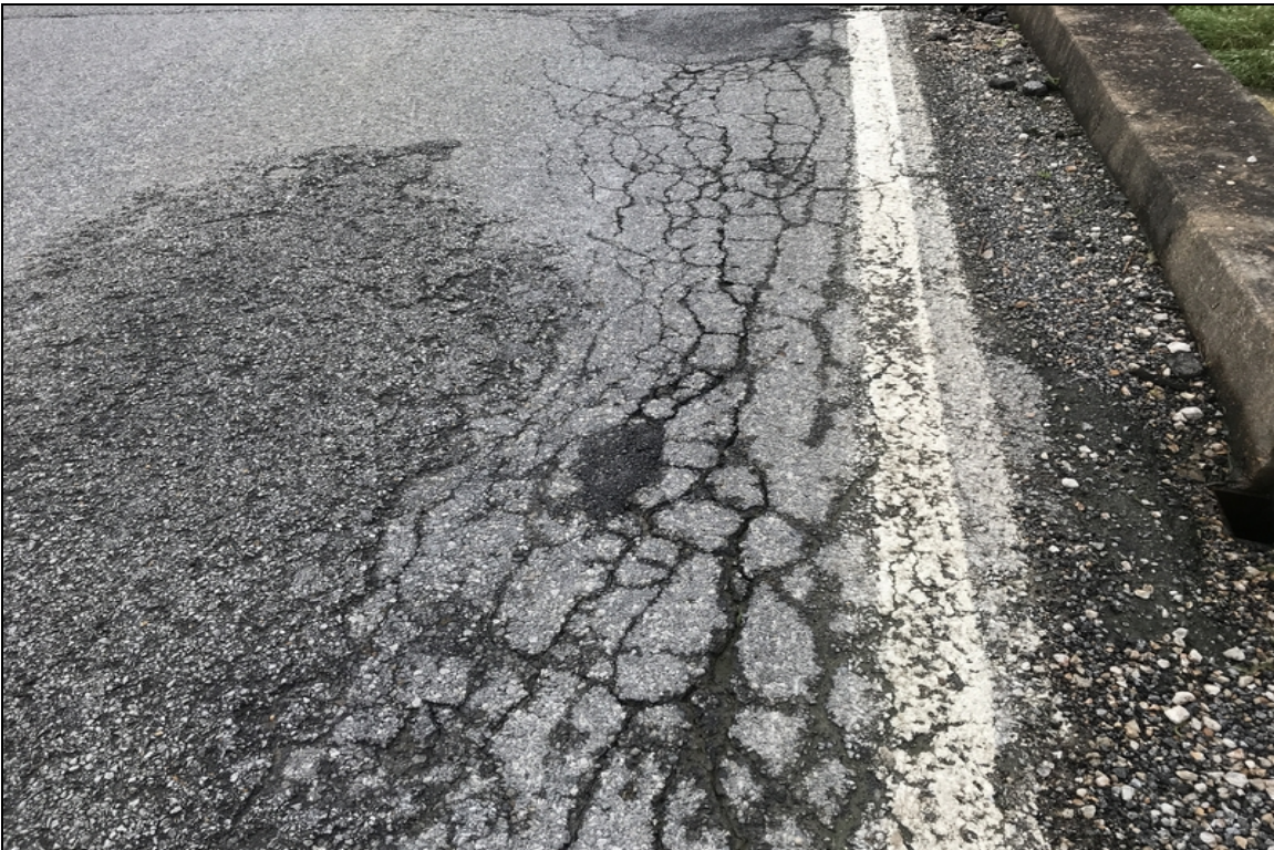
Typical cracks to a/c overlay @ all spans.
