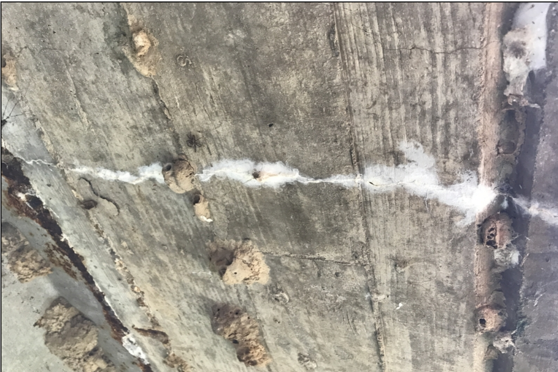
Typical cracks to Lt & Rt overhangs.
