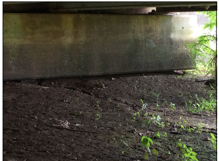
Undermining @ Abutment 1 with 2 piles exposed.
