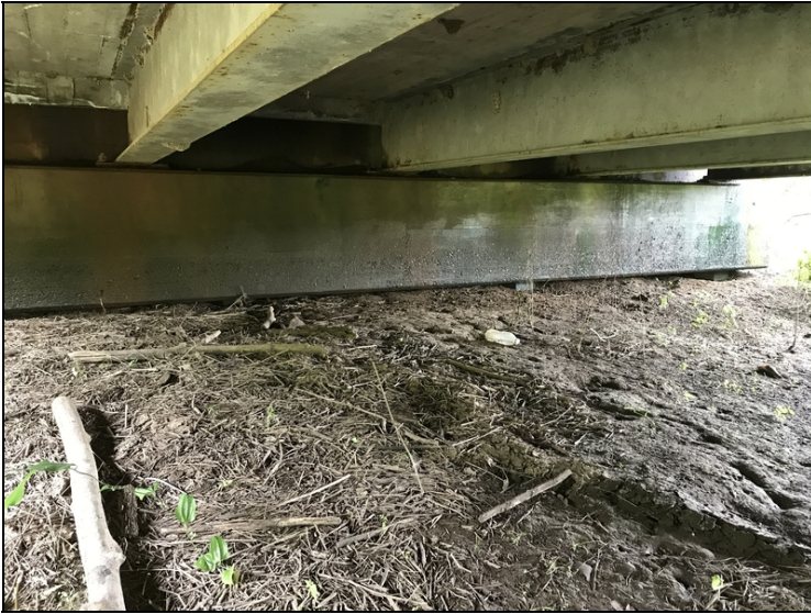
Undermining @ Abutment 1 with 3 piles exposed.
