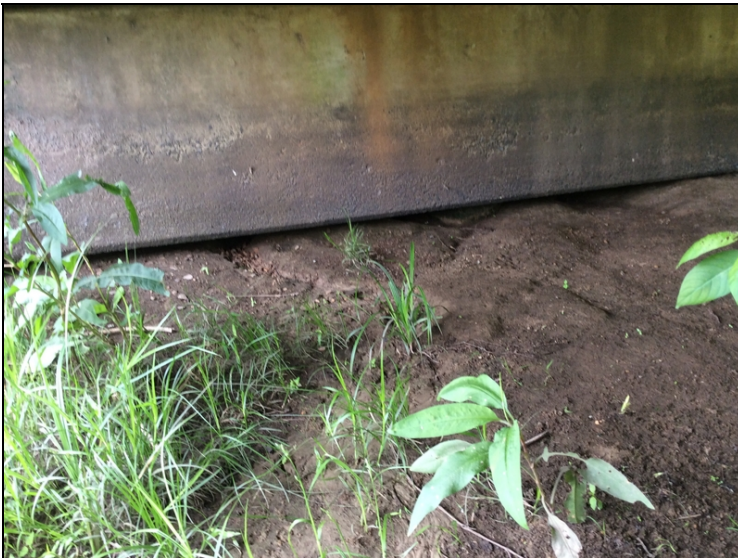
Undermining @ Abutment 2 with 1 pile exposed.
