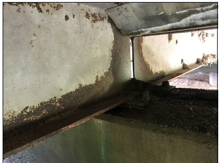
Rust to ends of all girders & bearing assemblies @ all spans.
