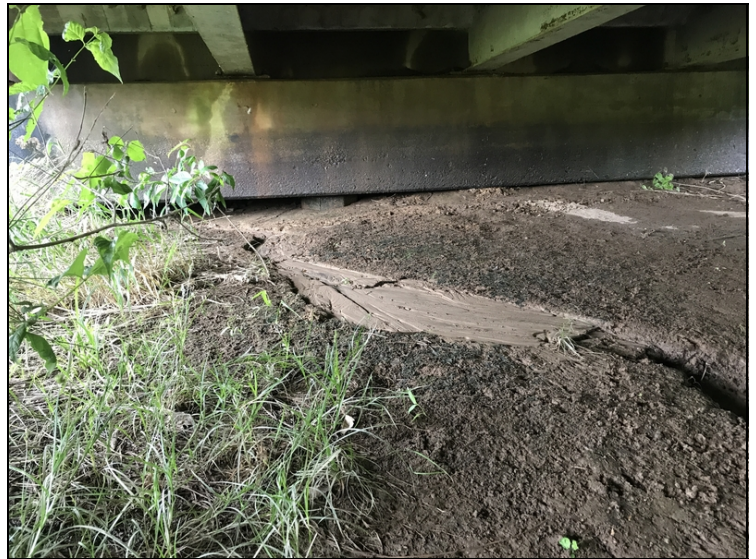
Undermining @ Abutment 2 with 1 pile exposed.
