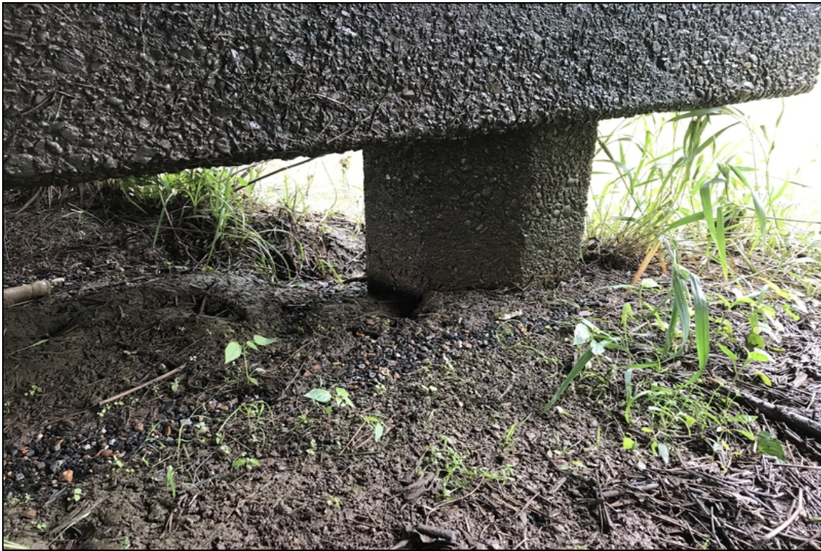
Typical abrasion to all piles.
