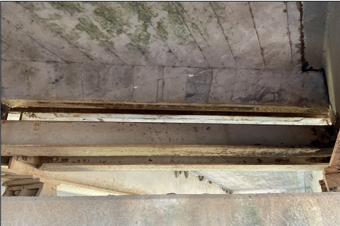
Efflorescent cracks to Left & Right overhangs and to Concrete haunch between ends of girders.
