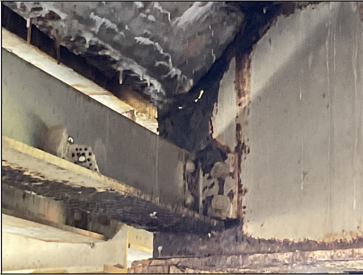
Span 3 - Girders 2 & 4 have large holes in web below haunch @ beginning of span. Girder 2.
