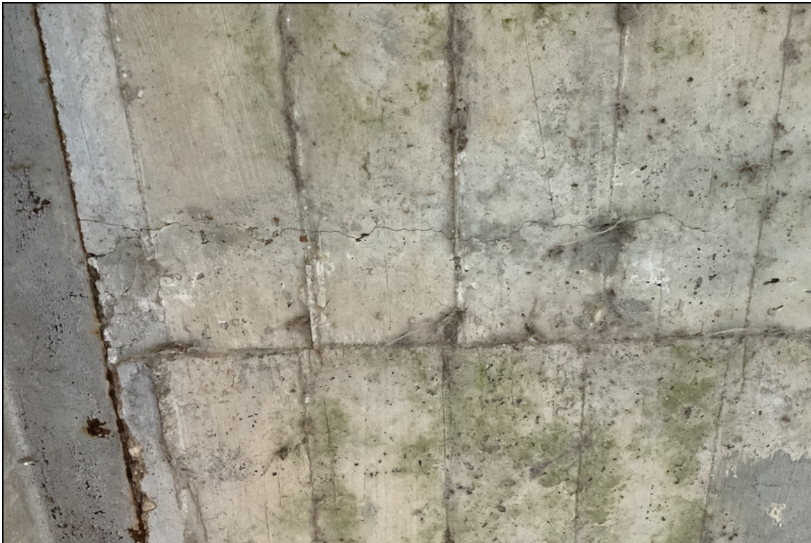
Typical cracks to soffit.
