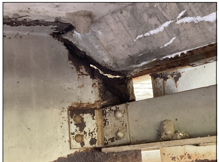
Span 3 - Girders 2 & 4 have large holes in web below haunch @ beginning of span. Girders 4
