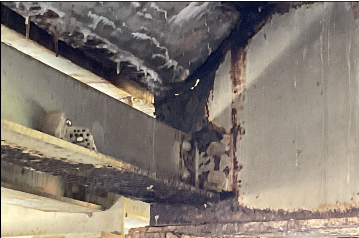
Span 3 - Girders 2 & 4 have large holes in web below haunch @ beginning of span. Girder 2.
