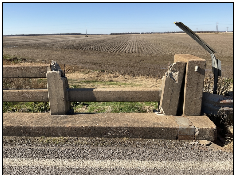
Span 3 - Top concrete guard rail is missing & Post 5 & 6 on Left side at Abutment 2 are broke due to collision damage.
