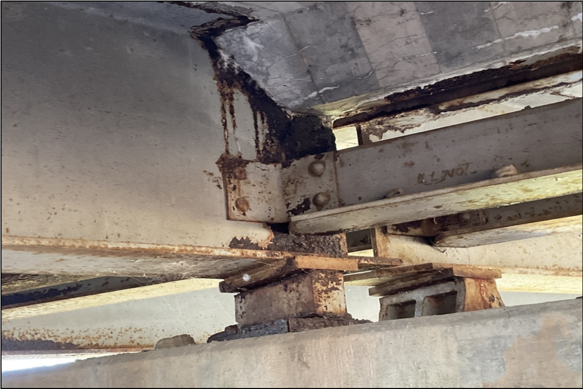
Typical corrosion to girders @ all spans.
