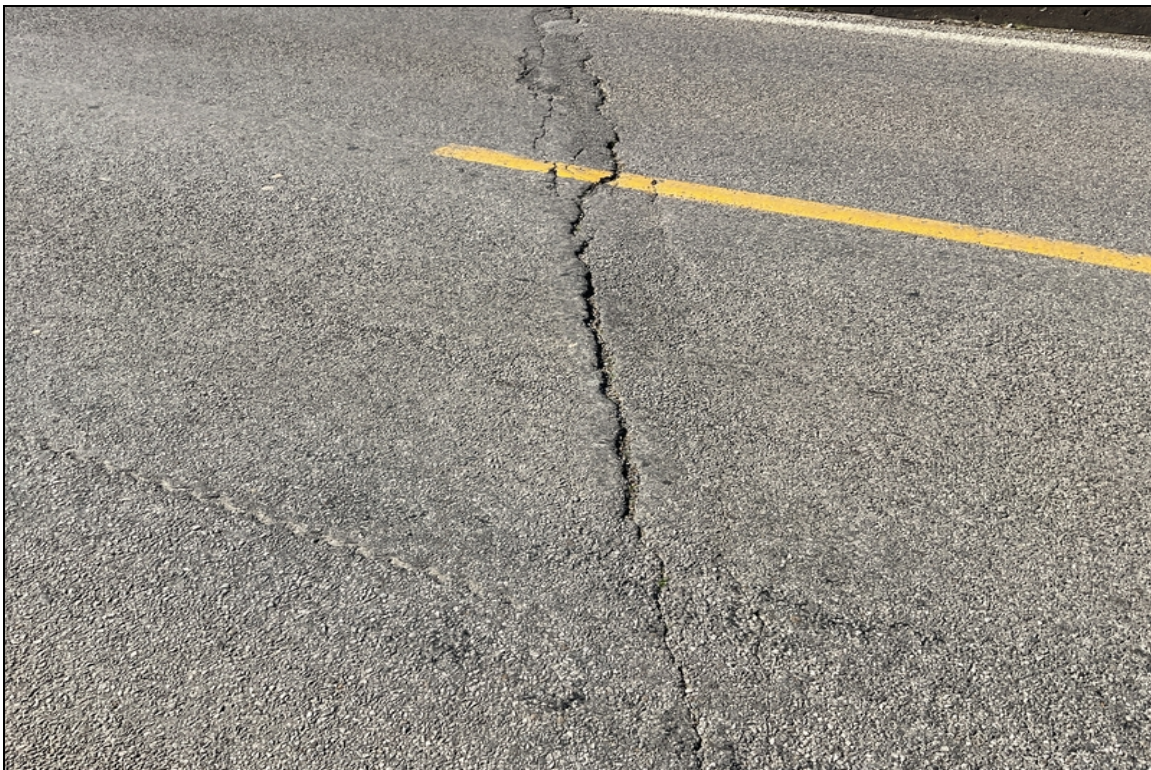
Typical cracks to wearing surface @ all joints.
