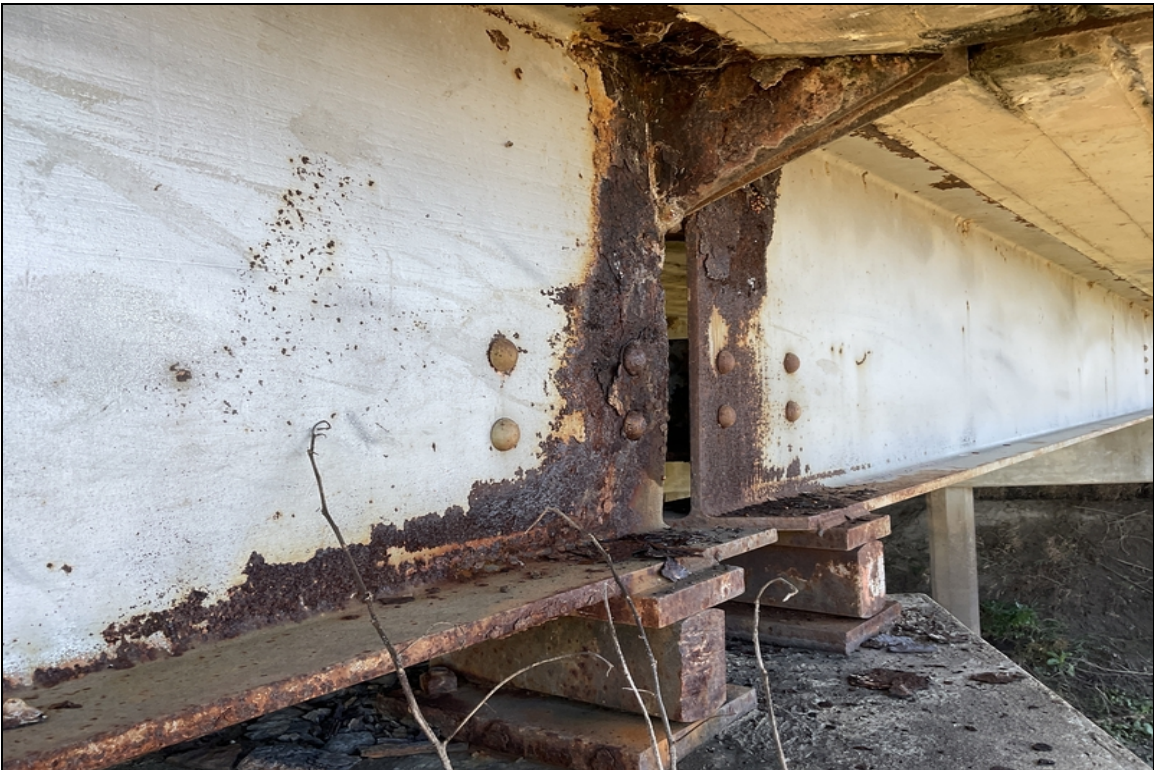
Girder 1 @ beginning of span 3 has out of plane bending & severe sections loss.
