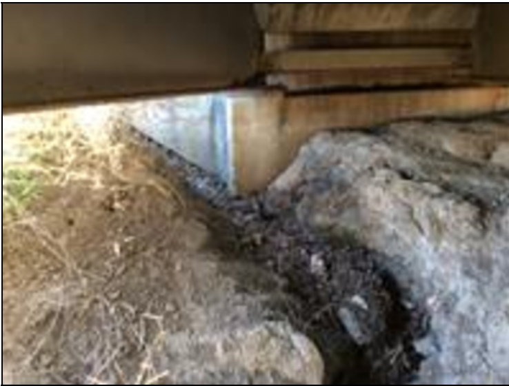
Erosion to slope at Span 1.
