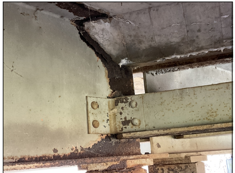
Girders over Bent 2 near paving haunch have Rust with moderate to severe section loss.
