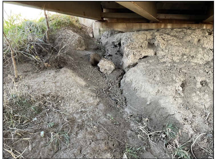
Erosion to slope at Spans 1 & 3. Span 3.
