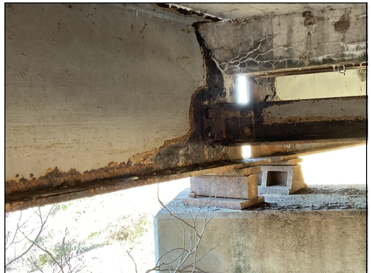
Girder Ends over Bent 1 Rust with minor to moderate section loss.
