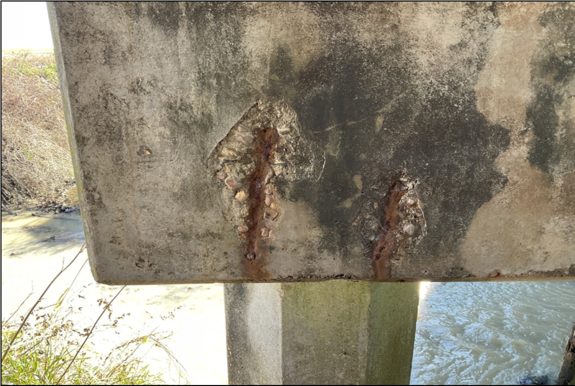
Spalls with rebar exposed to Lt & Rt ends of bent 2.
