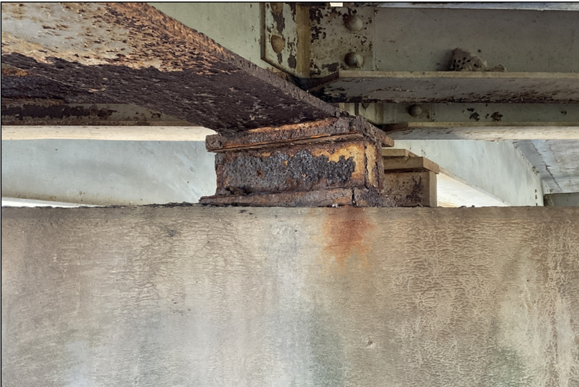
Typical corrosion to bearings @ all bents.
