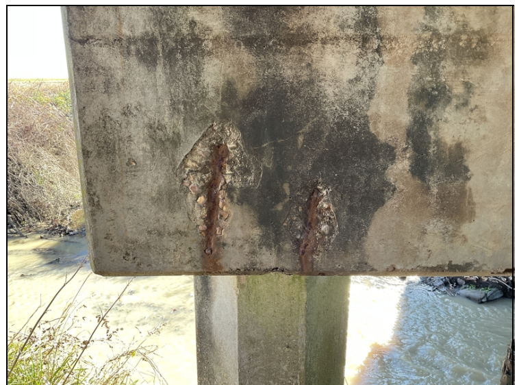
Bent 2 Cap Spall with 2' of exposed rebar to Right end & 6" to Left end.
