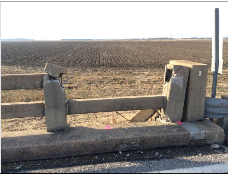
Span 3 - Top concrete guard rail & Post 5 & 6 on Left side at Abutment 2 are broke or missing from collision damage.
