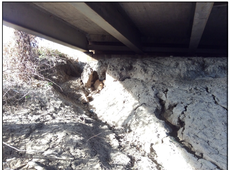
Erosion at Abutment 2 Left side.
