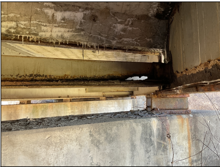
Hole in diaphragm between Girders 1 & 2 @ beginning of Span 3.
