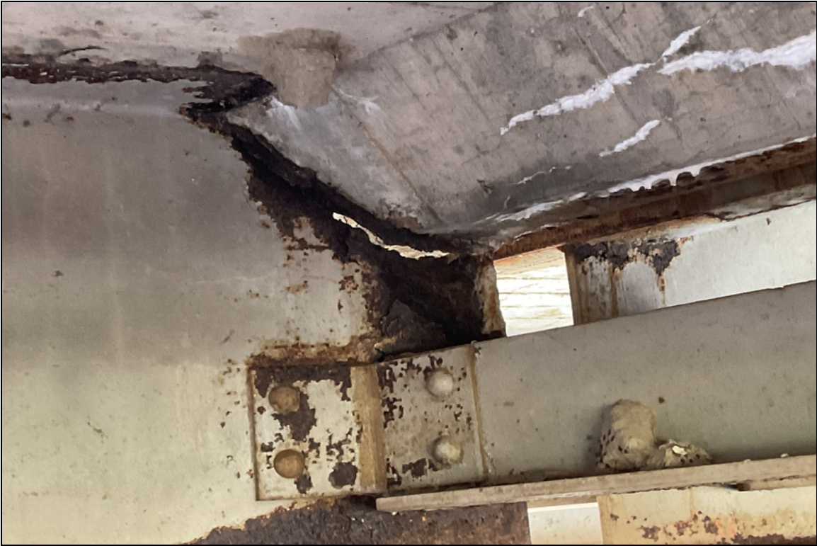
Span 3 - Girders 2 & 4 have large holes in web below haunch @ beginning of span. Girders 4
