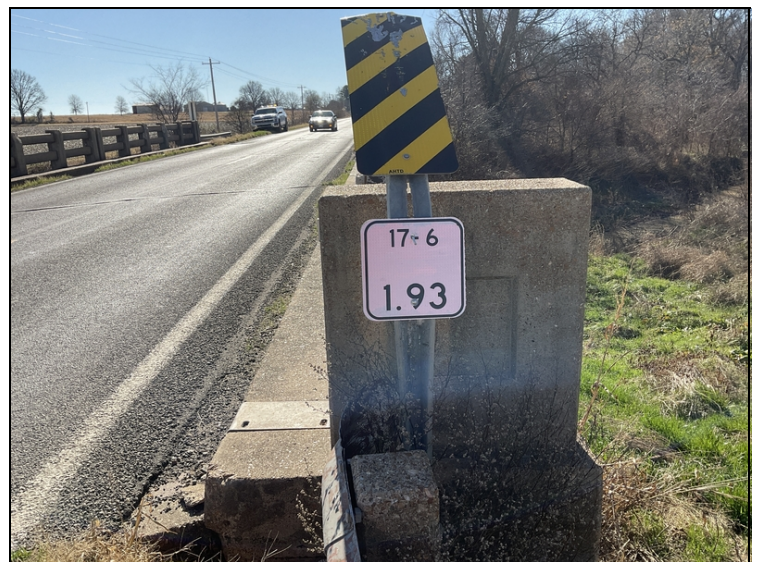
Log Mile sign is missing @ Abutment 2. Should read 1.93. Repaired.
