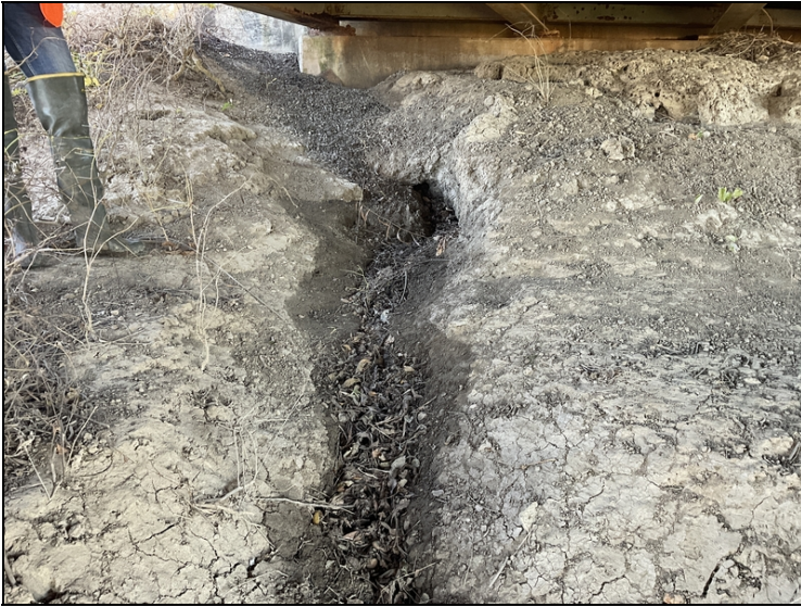
Erosion to slope at Spans 1 & 3. Span 1.
