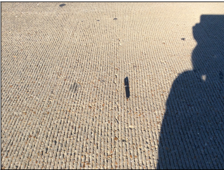
Typical unsealed cracks to deck @ all spans.
