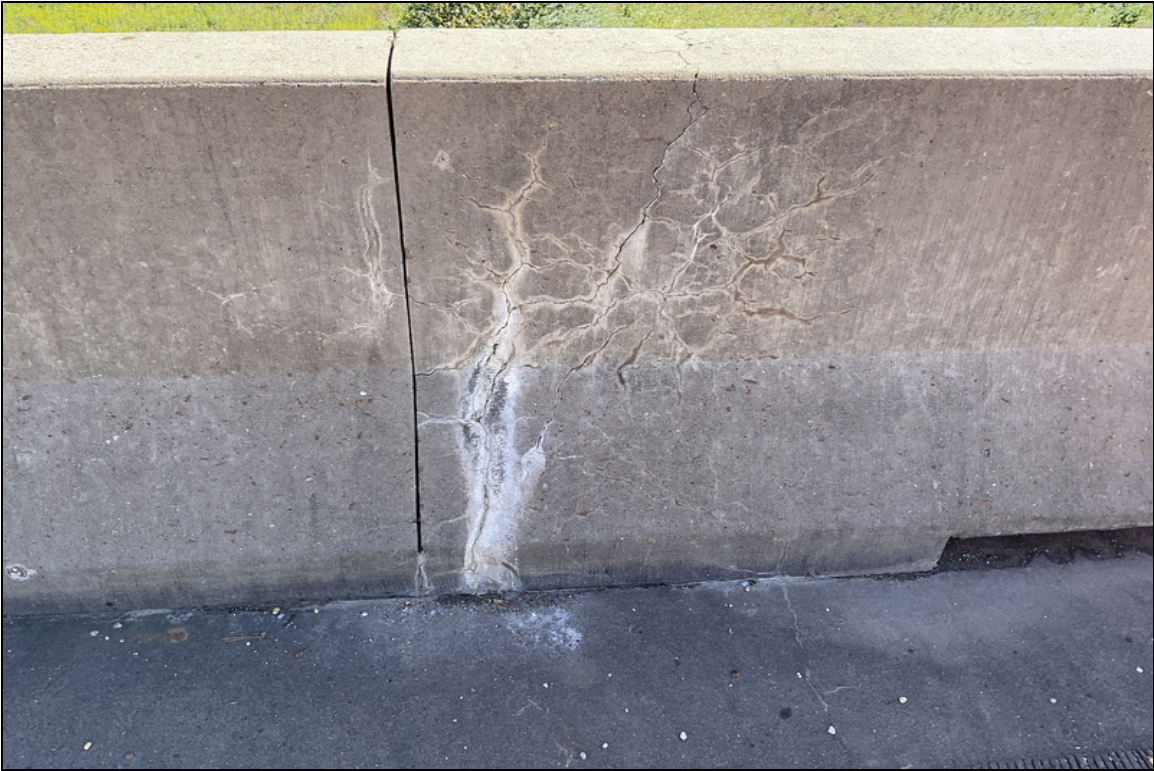
Efflorescence map cracking to Lt parapet wall @ spans 2 & 3.
