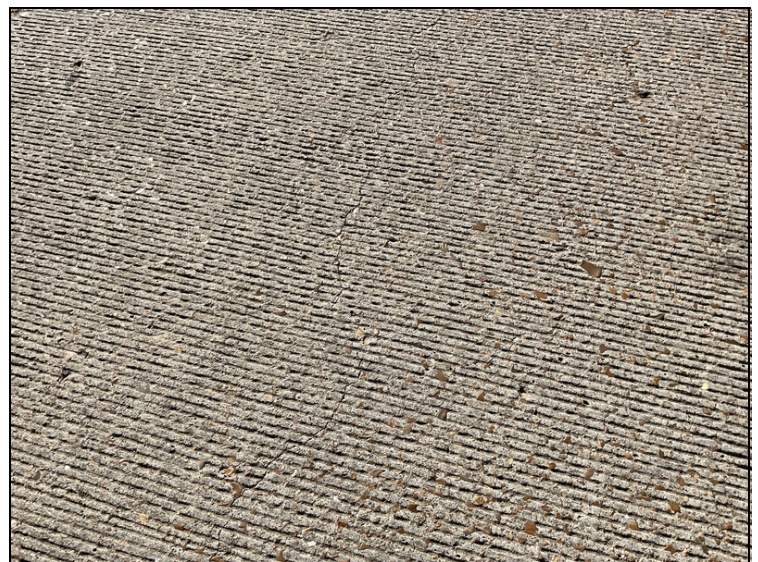
Unsealed cracks to deck @ all Spans.
