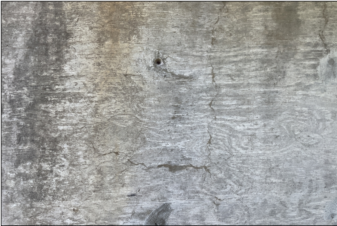
Minor cracks to rt side of cap @ bent 8.
