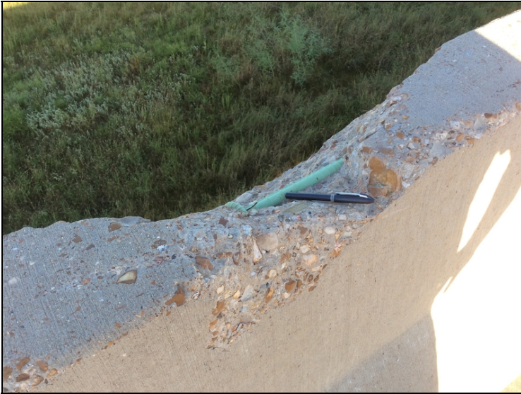
Large spall with 1' rebar exposed to Right parapet wall @ Span 11.
