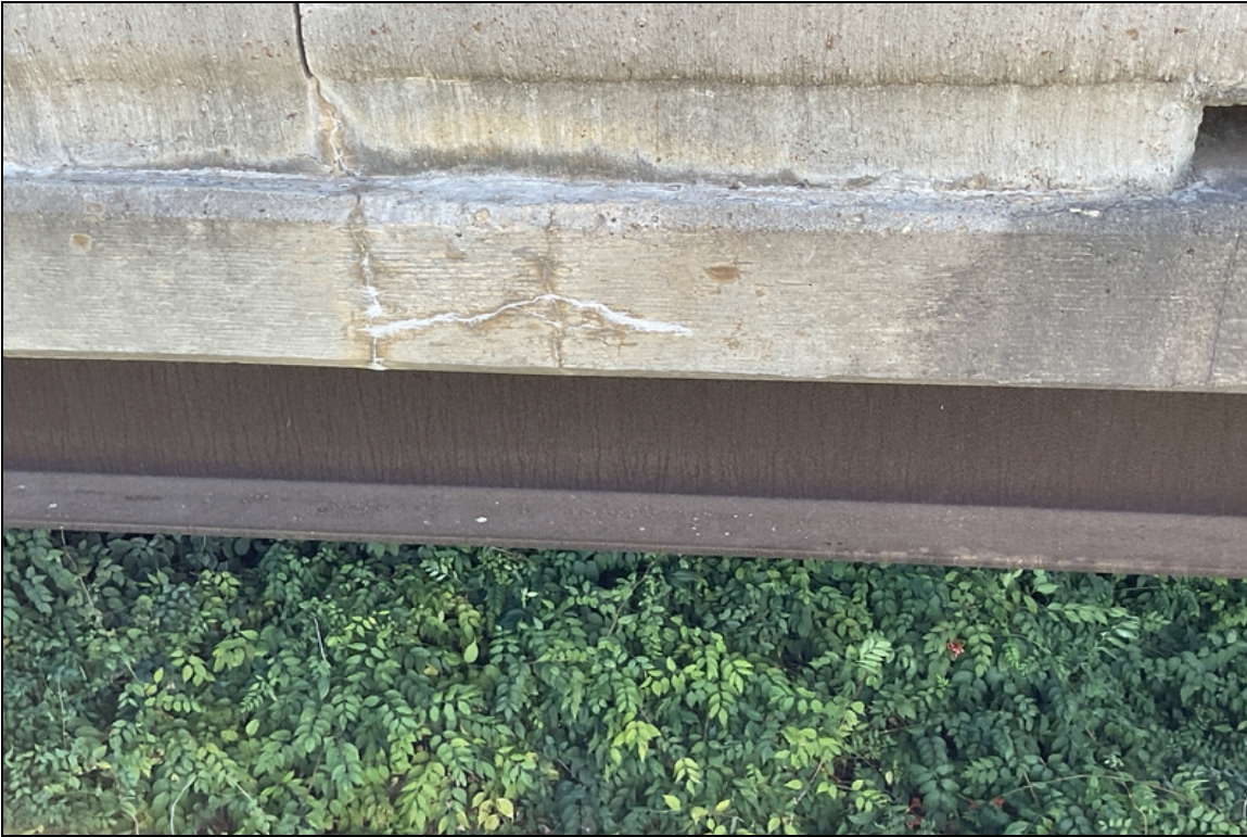
Typical efflor cracks to Lt & Rt overhangs.
