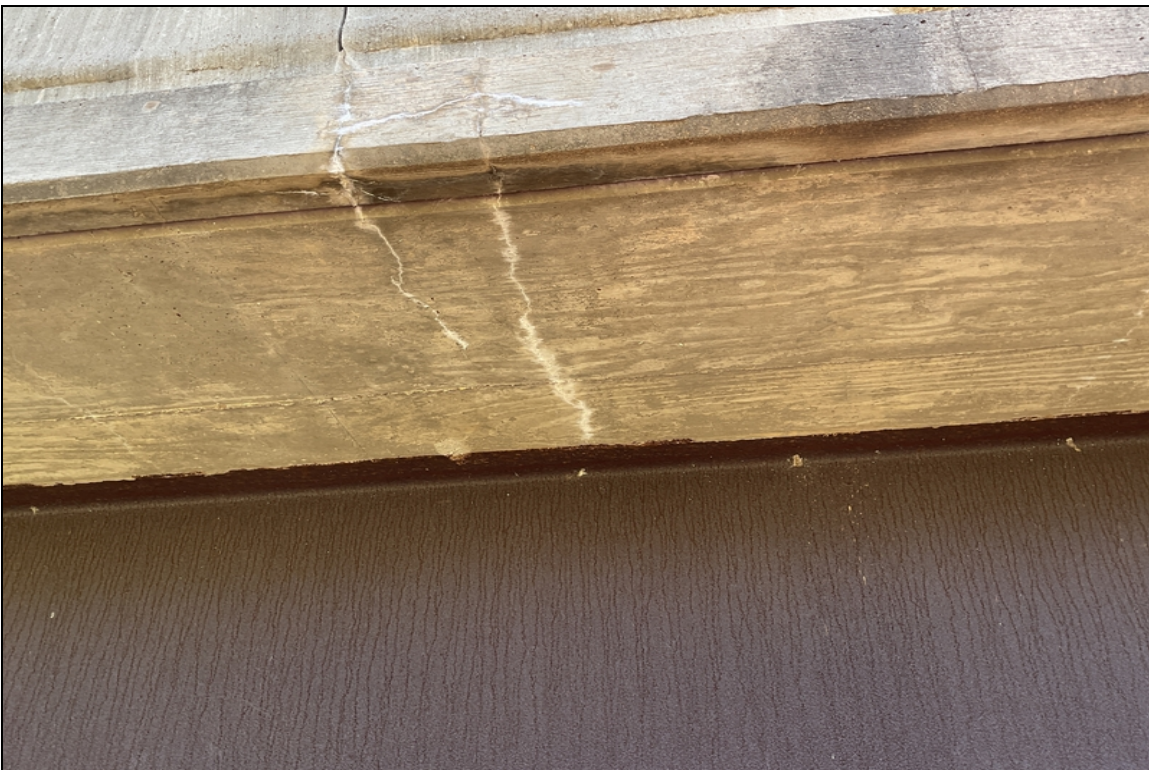
Typical efflor cracks to Lt & Rt overhangs.
