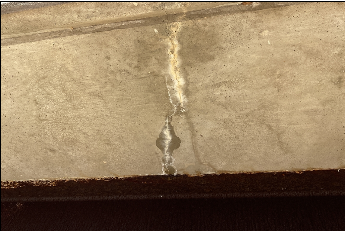
Typical efflor cracks to Lt & Rt overhangs.
