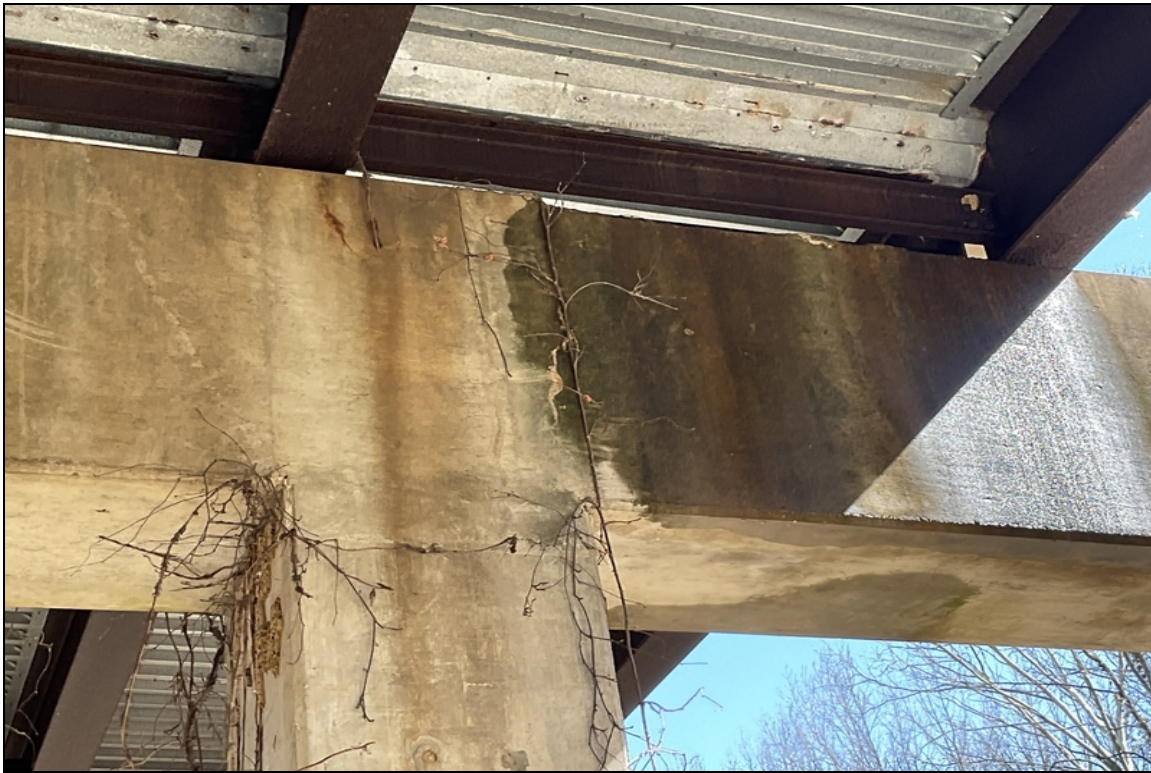
Efflor crack to cap, rt side @ backside of bent 1.
