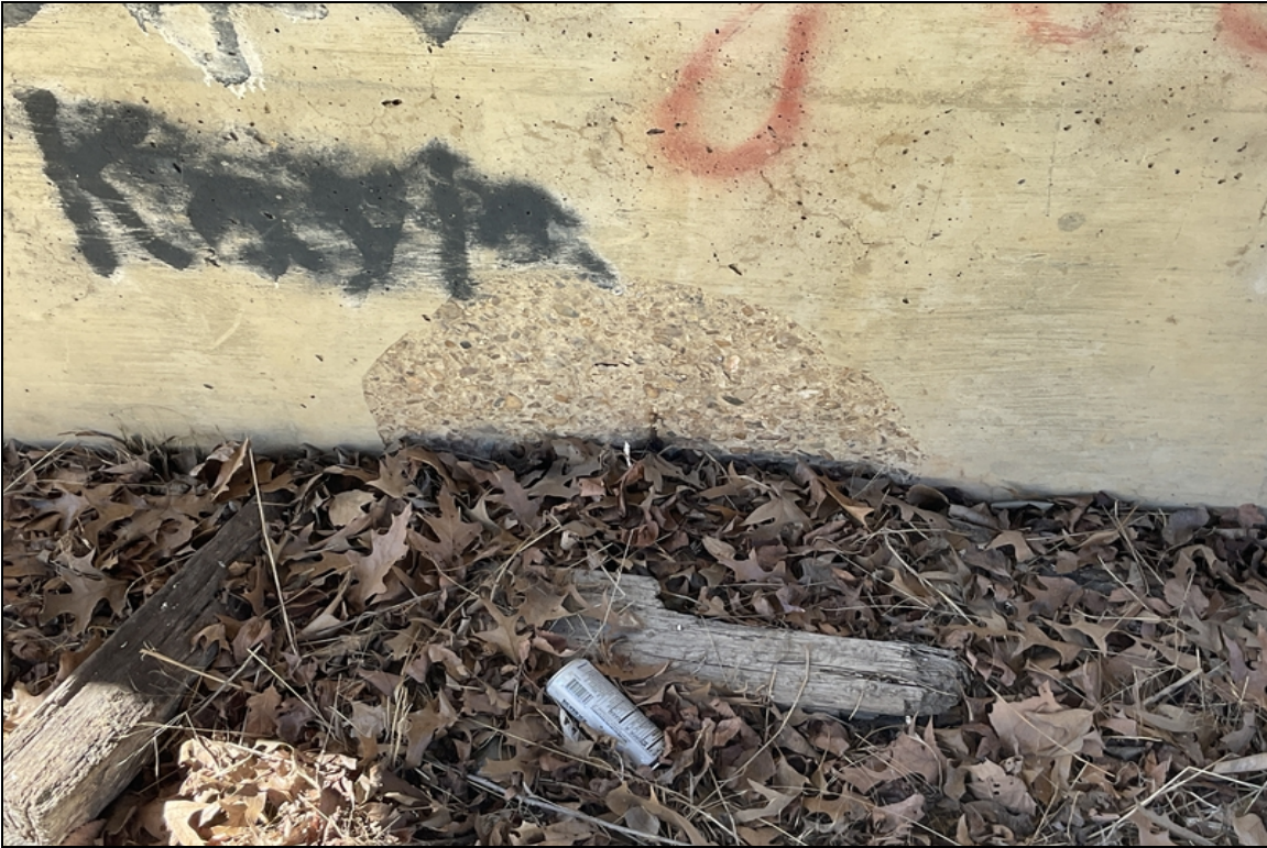
Spall to pier wall @ ahead side of bent 2.
