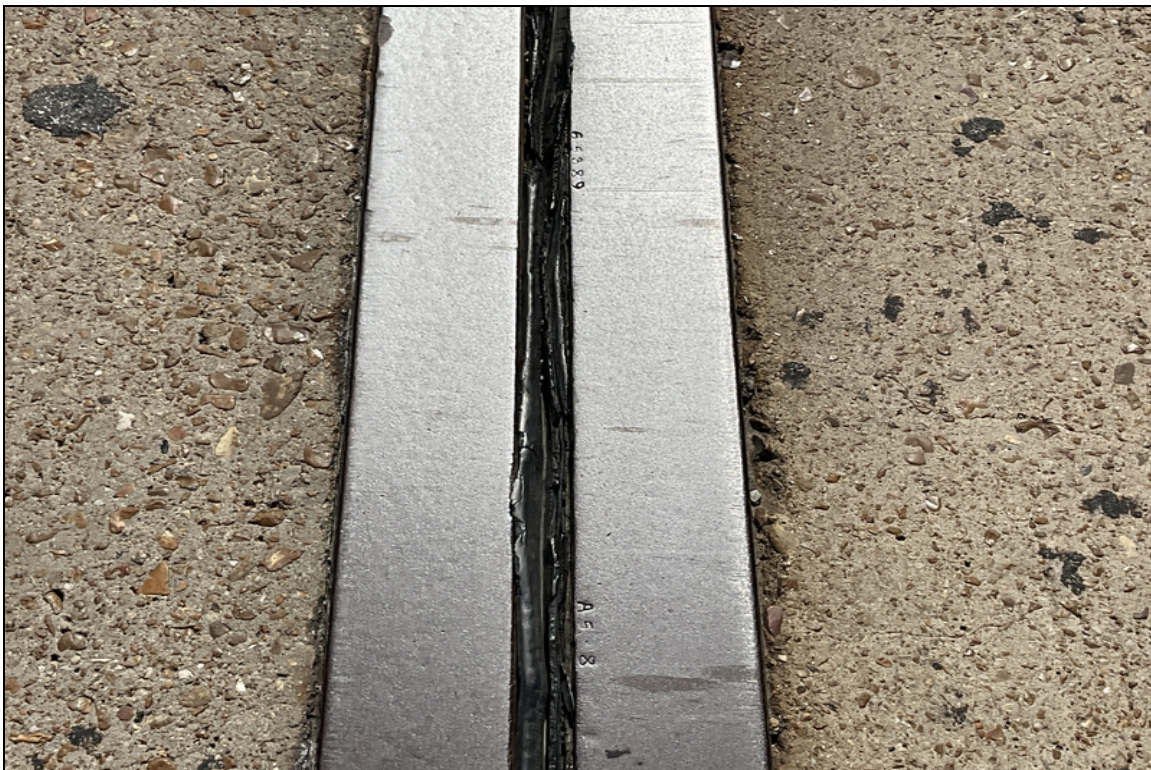
Cracking to joint seals @ all bents.
