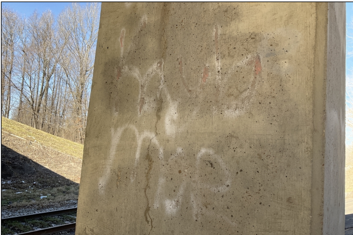
Vertical crack to column 1 @ bent 2.
