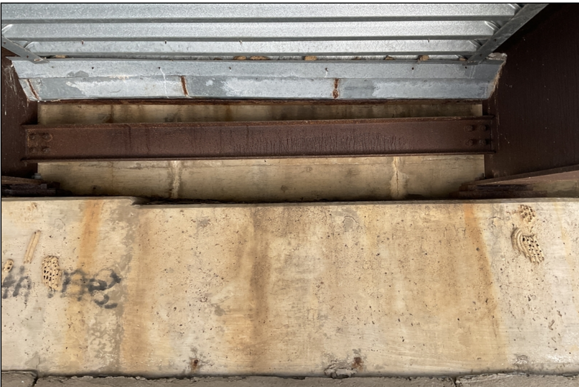
Vertical efflor cracks to back wall @ abutments 1 & 2.
