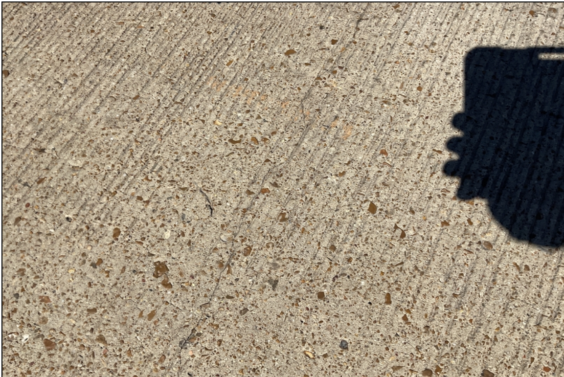
Typical cracks to deck @ all spans.
