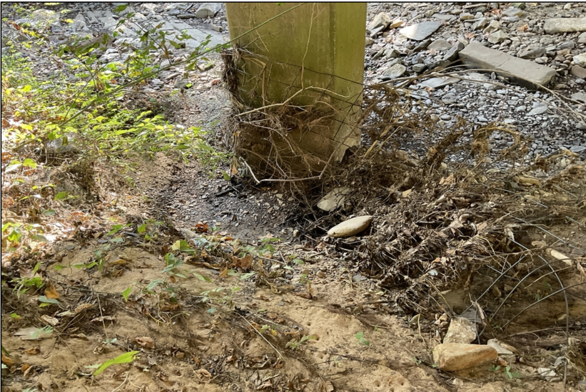
Scour to columns @ bent 1.
