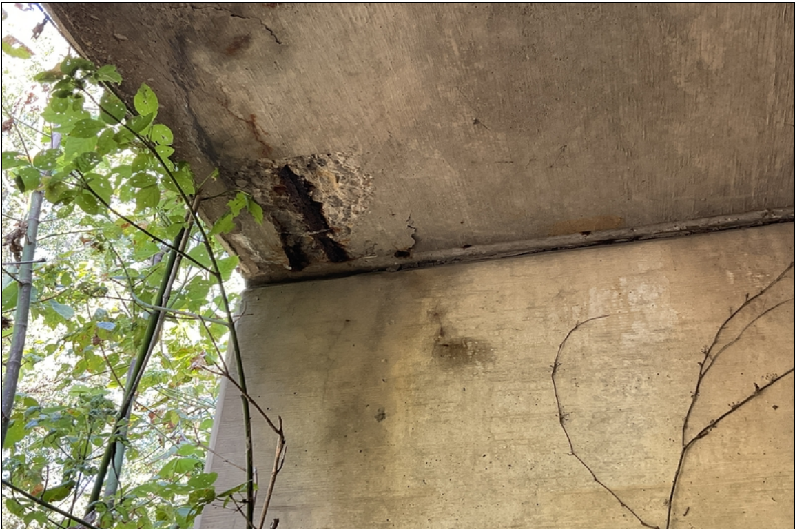
Spall with rebar exposed to rt edge of deck @ beginning of span 3.
