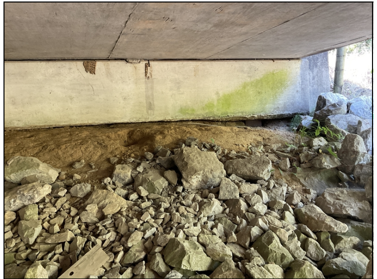
Erosion & embankment has settled @ Abutment 2 with 2 piles exposed.
