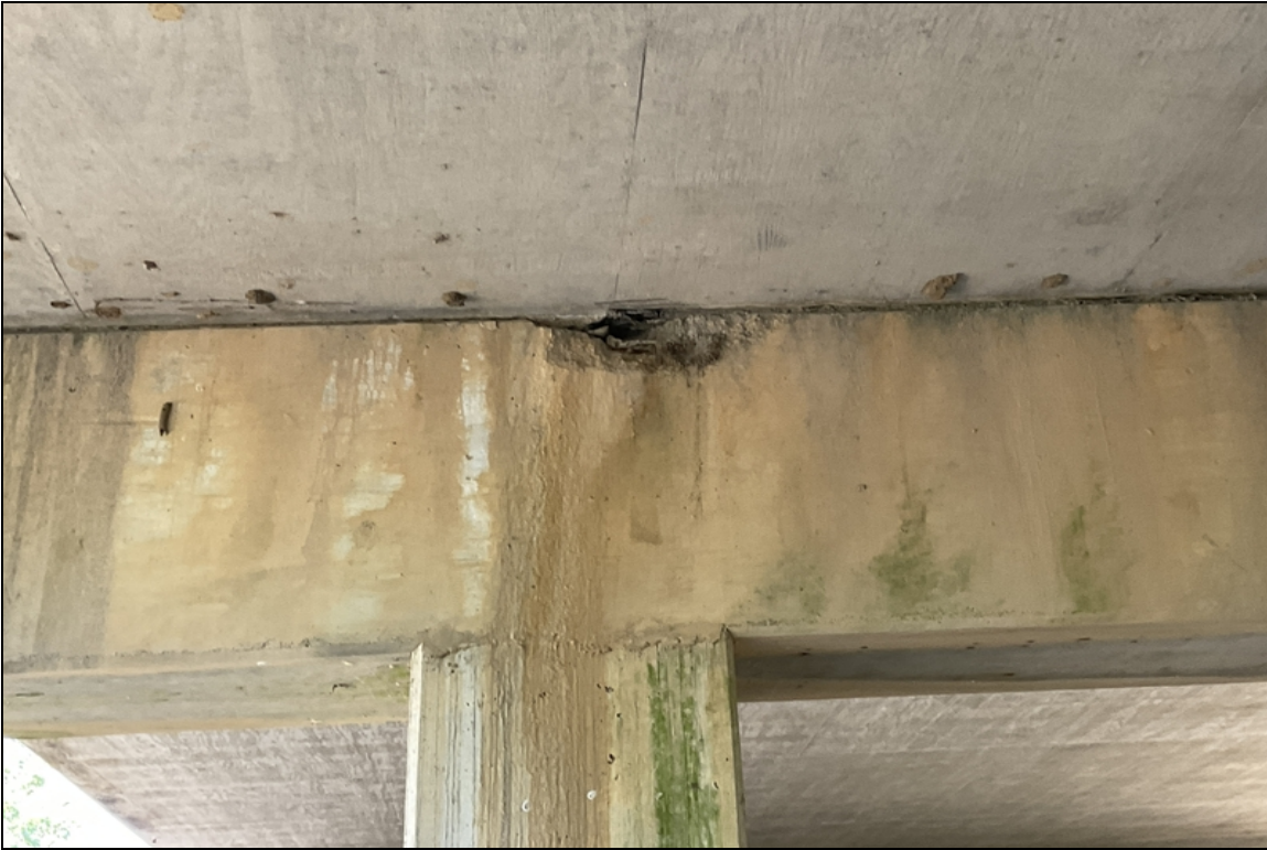
Spall with rebar exposed to ahead side of cap @ bent 1.
