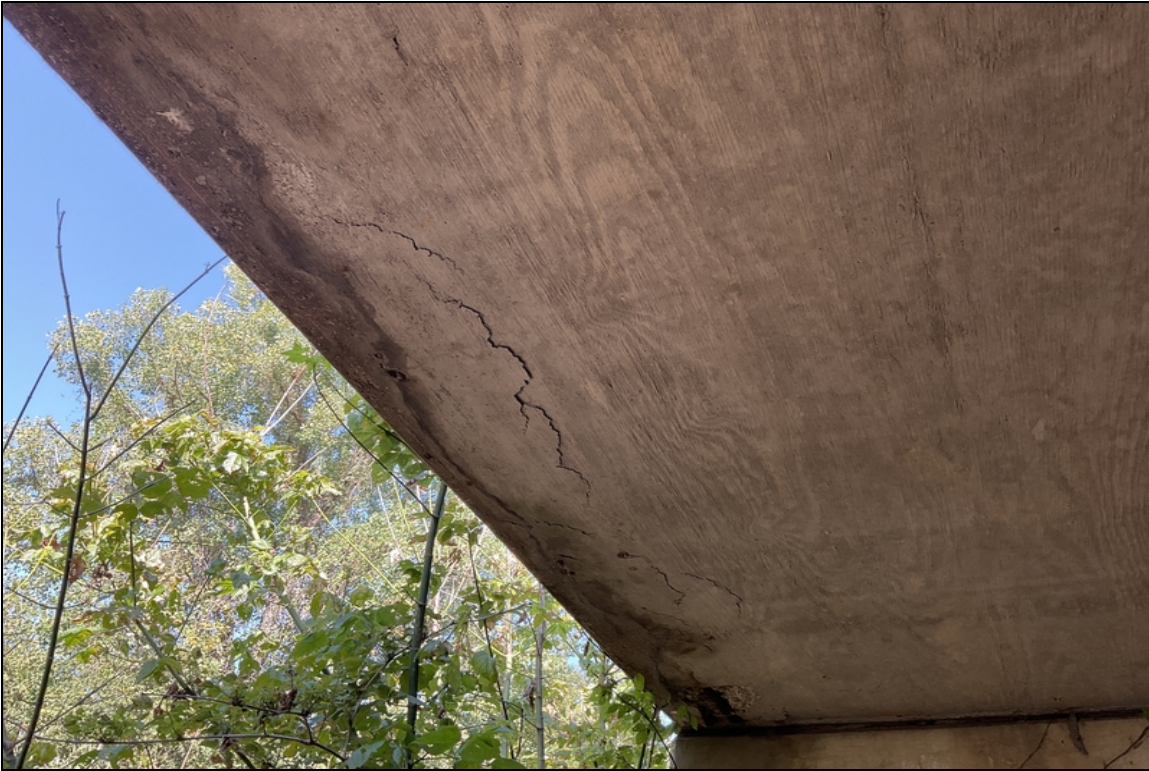
Delam to rt edge of deck @ beginning of span 3.
