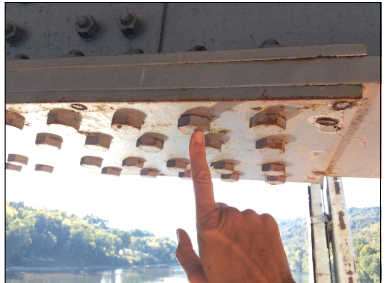
Loose bolt @ bottom splice plate @ Girder 4 Span 4.
