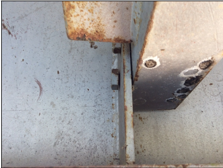
1st diaphragm ahead of Bent 3 has loose bolt @ Girder 3.
