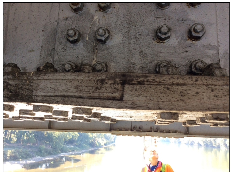
Bottom splice plate @ Girder 3
