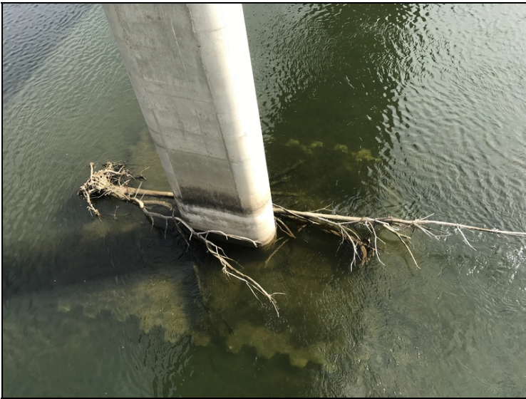
Bent 3 has Drift.
