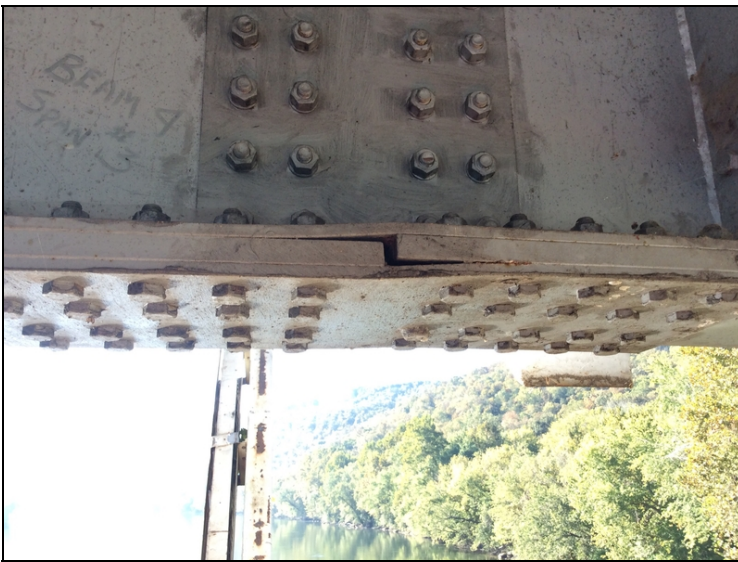
Bottom splice plate is bent 1/4"@ Span 3 Girder 4.
