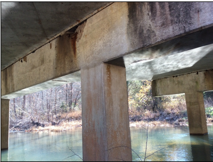
Spalls with rebar exposed to cap @ Bent 4.
