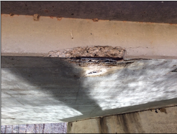
Spall with rebar exposed to Left edge of deck @ Span 5.
