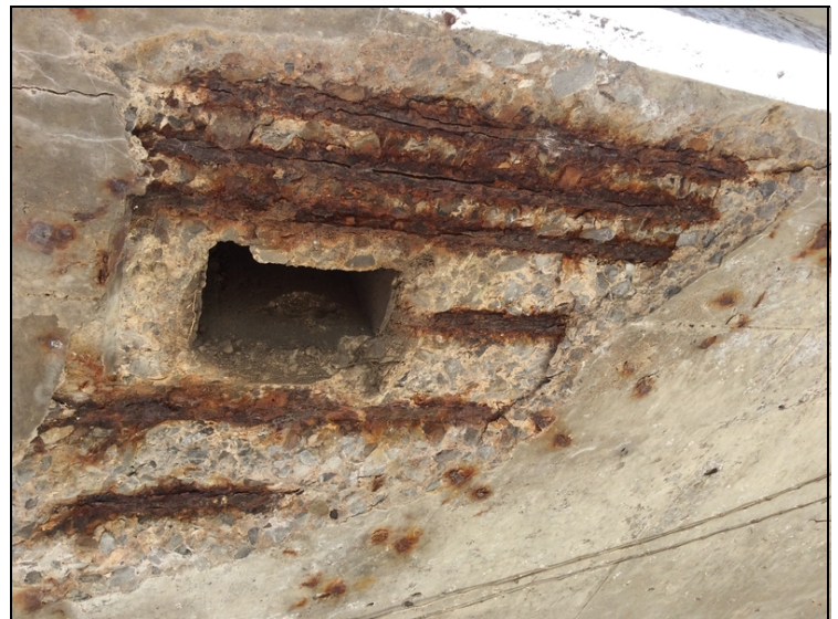
Spalls with rebar exposed to soffit @ Right drain opening @ Span 6.
