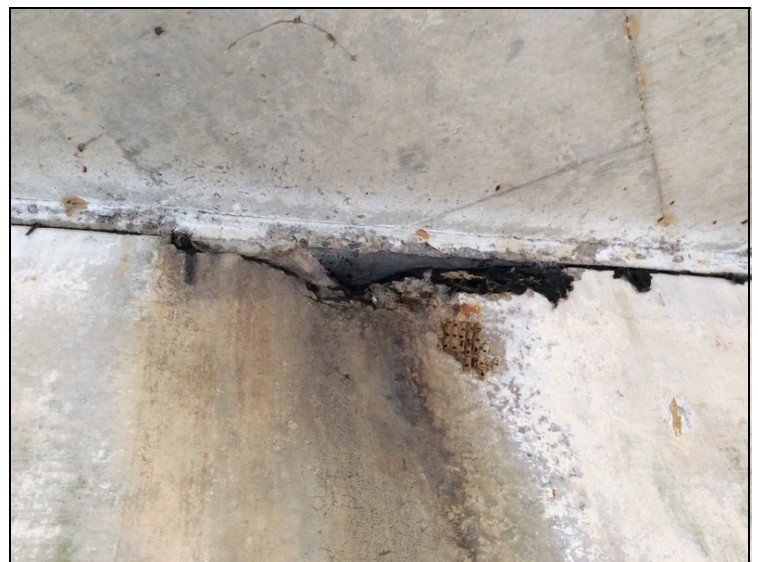
Spalls with rebar exposed to ahead side of cap @ Bent 1.
