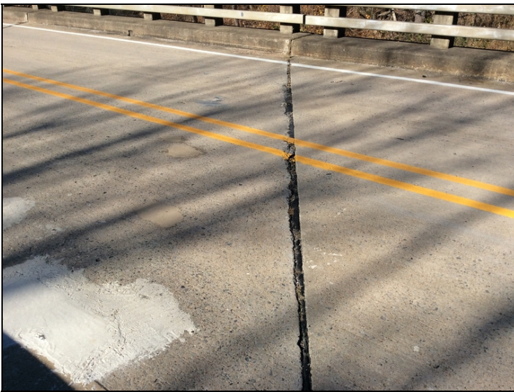
Joint seal @ Bent 3.
