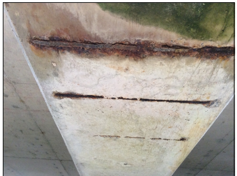
Spalls with rebar exposed to bottom of cap @ Bent 1 Left.
