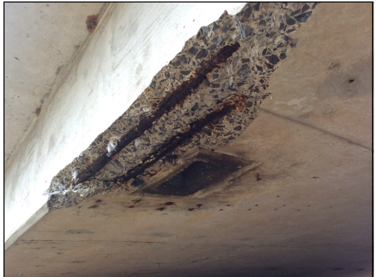
Spalls with rebar exposed to Right drain opening @ Span 1.
