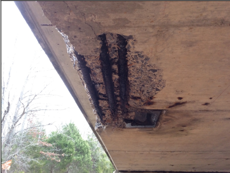
Spalls with rebar exposed to Left drain opening @ Span 2.
