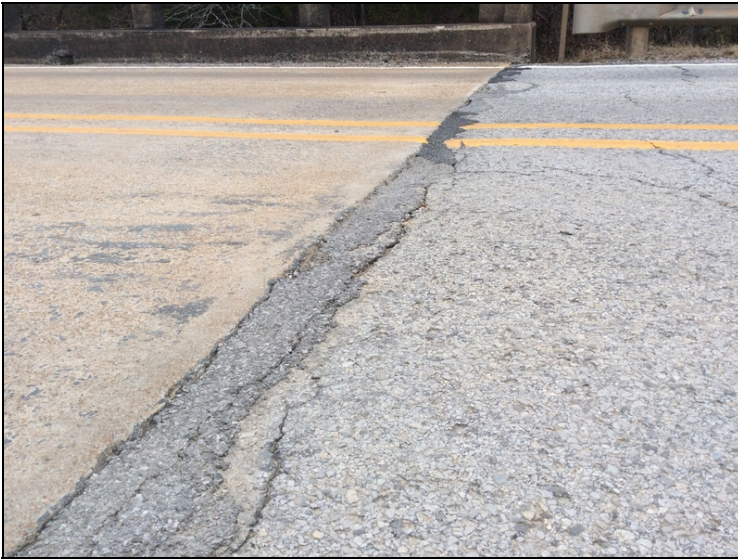
Roadway settlement @ Abutment 2.
