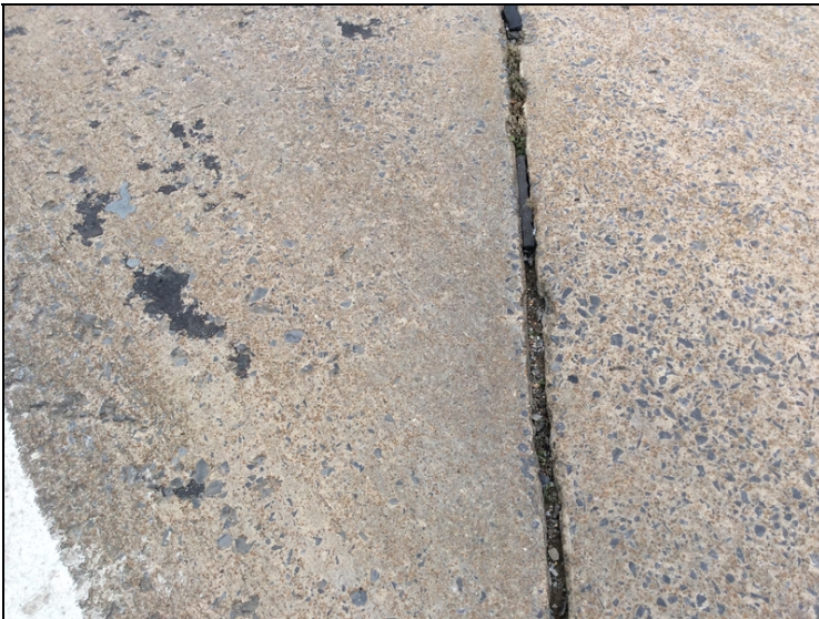
Pourable joint @ Bent 2 has portions missing.
