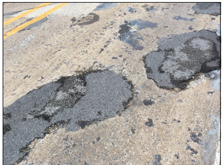
Asphalt patched area to deck @ Span 1.
