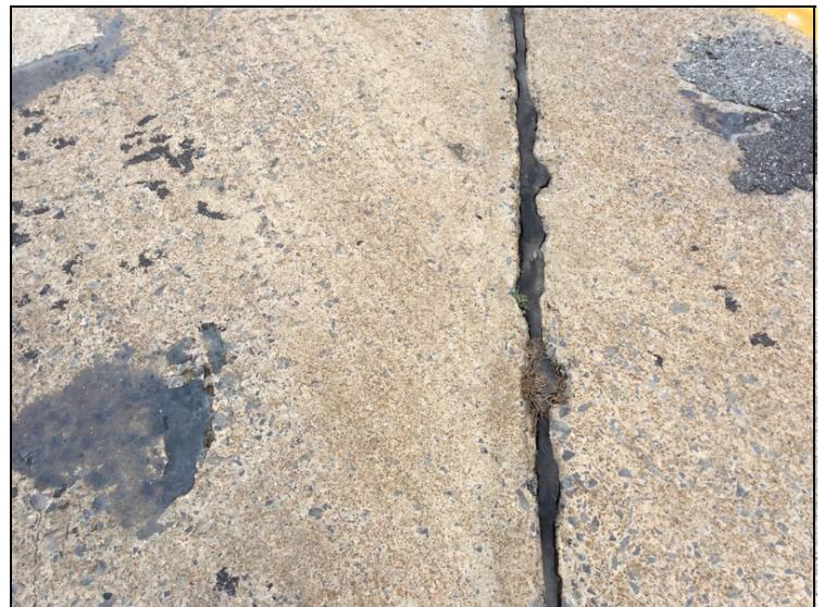
Pourable joint seal is losing adhesion @ Bent 2. (typical)
