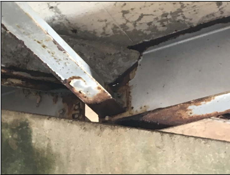
Hole in web below haunch @ Girder 4 @ end of Span 2.
