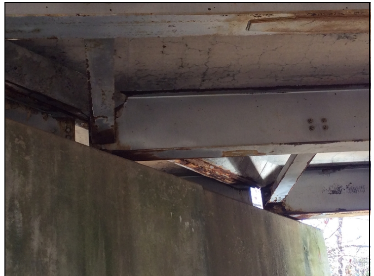
2' of end of all Girders have rust with some minor section loss.
