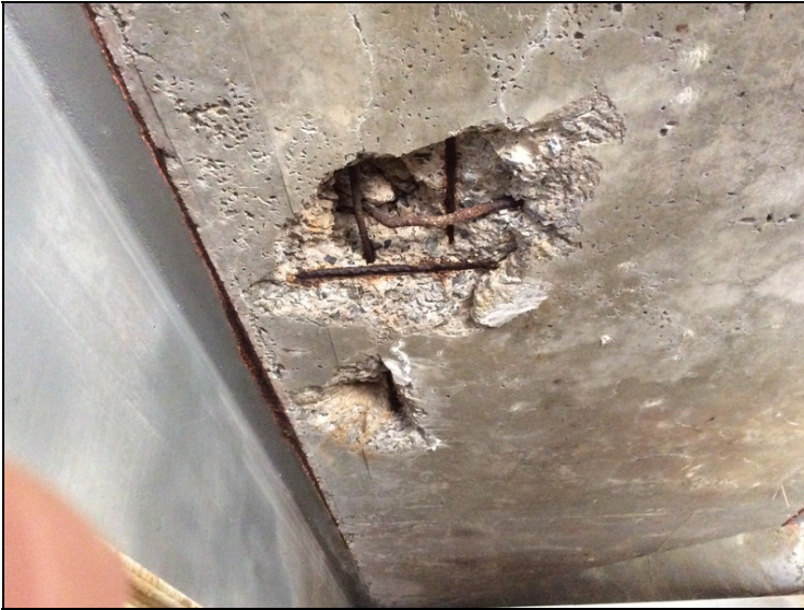
Spalls between Girders 3 & 4 at Span 3.
