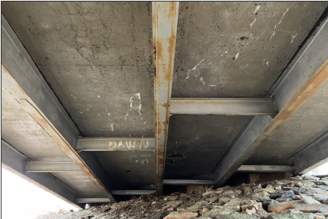
Typical efflor cracks to soffit @ all spans.
