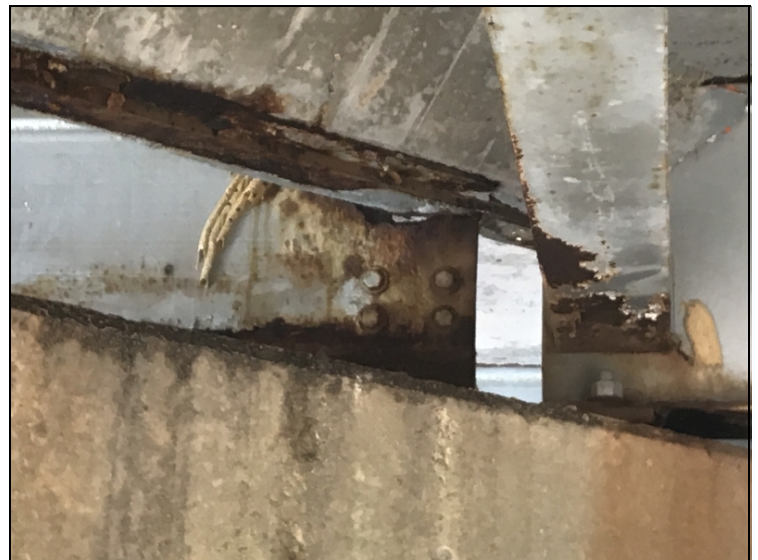
Hole in web below haunch @ Girder 2 @ end of Span 2.
