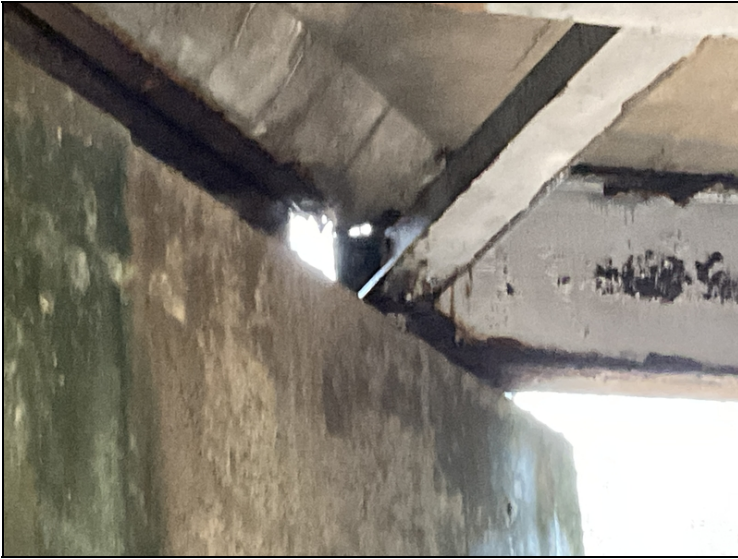
Rust and section loss to girder 5 at Spans 1 & 2. Hole to web, below paving haunch @ girder 5, end of span 2.
