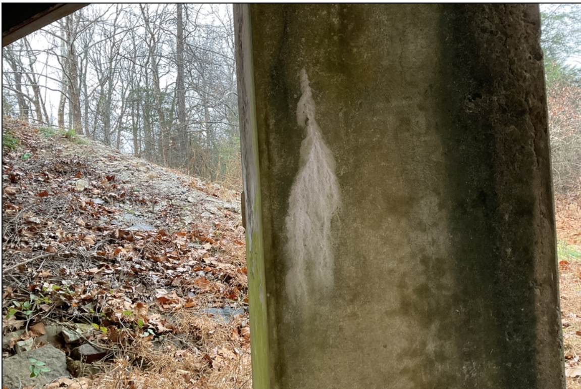
Efflor crack to backside of column 2 @ bent 2.
