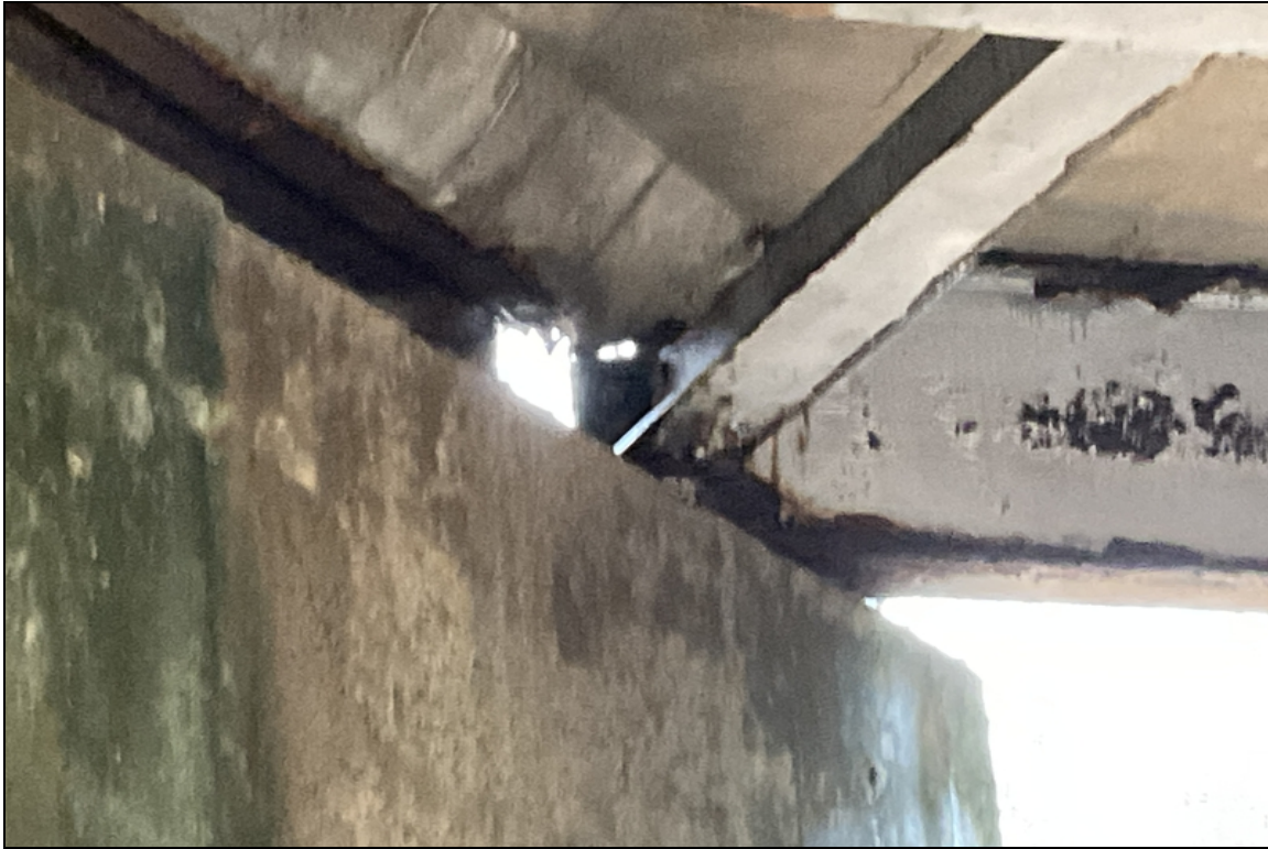
Rust and section loss to girder 5 at Spans 1 & 2. Hole to web, below paving haunch @ girder 5, end of span 2.
