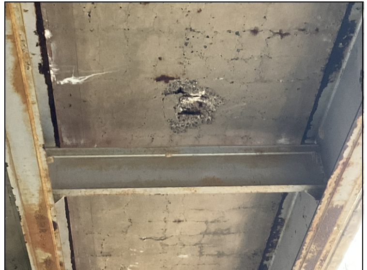
Deep spalls with rebar exposed to deck below at All Spans. Span 2.
