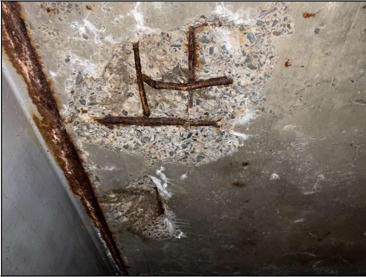
Deep spalls with rebar exposed to deck below at All Spans. Span 3, between girders 2 & 3.
