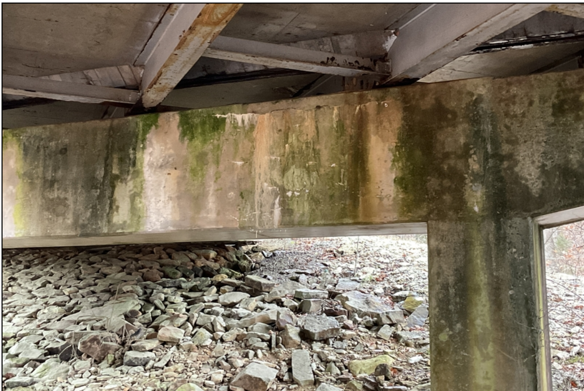
Typical efflor to caps @ bents 1 & 2. Backside of bent 1.
