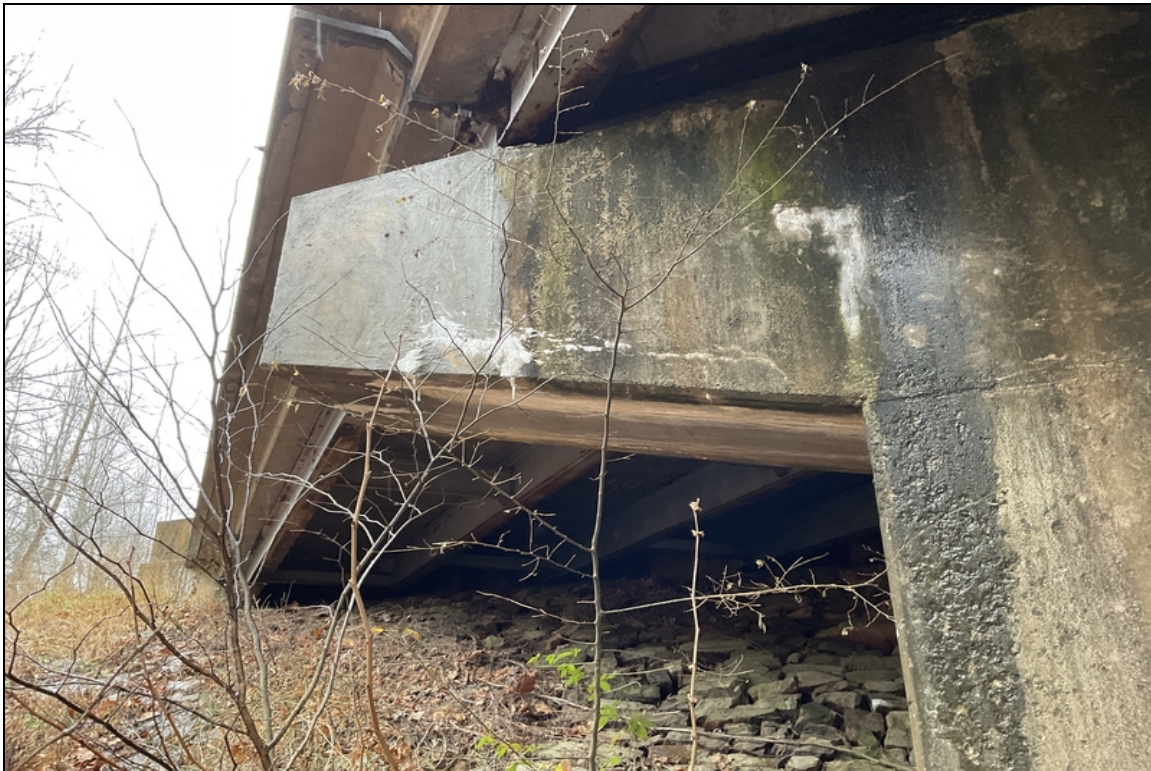
Typical efflor to caps @ bents 1 & 2. Backside of bent 2.
