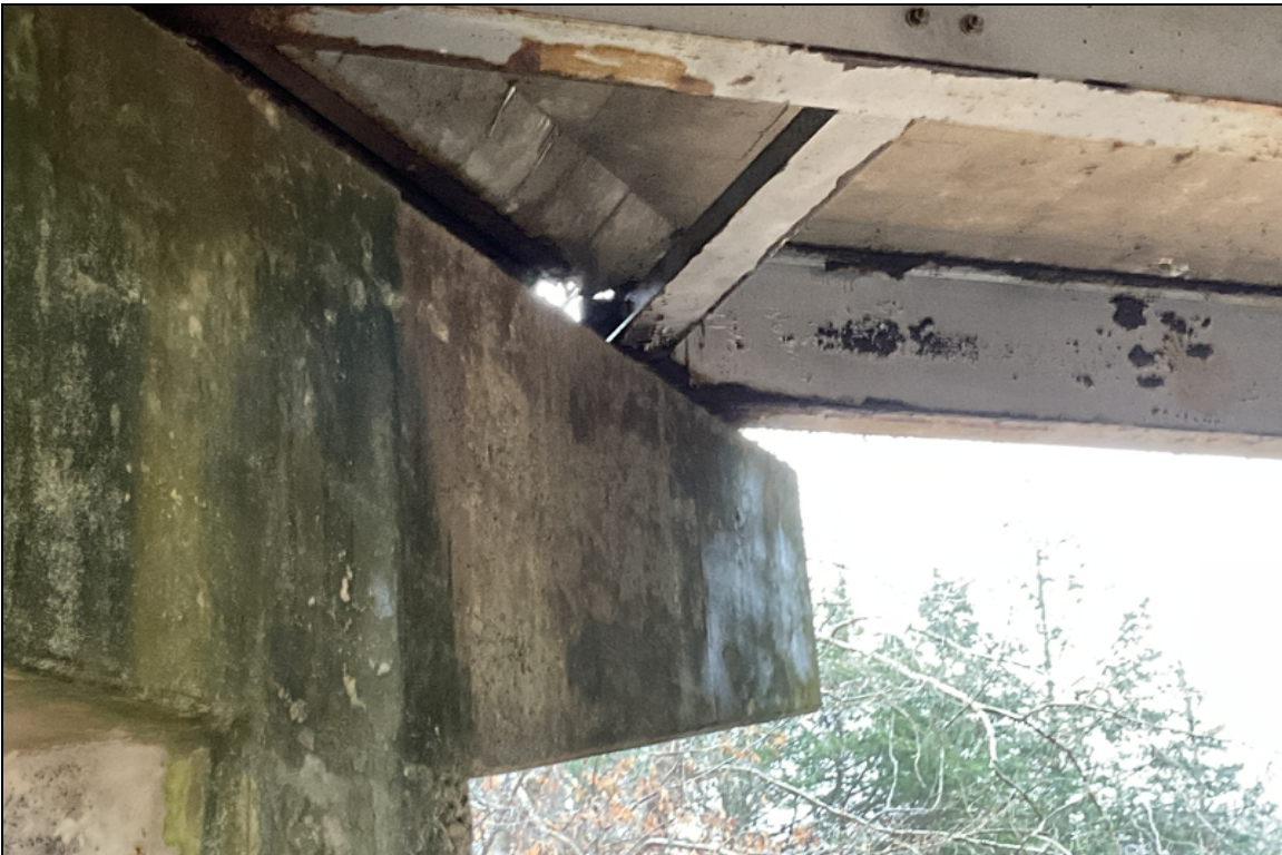
Hole to web @ girder 5, end of span 2.
