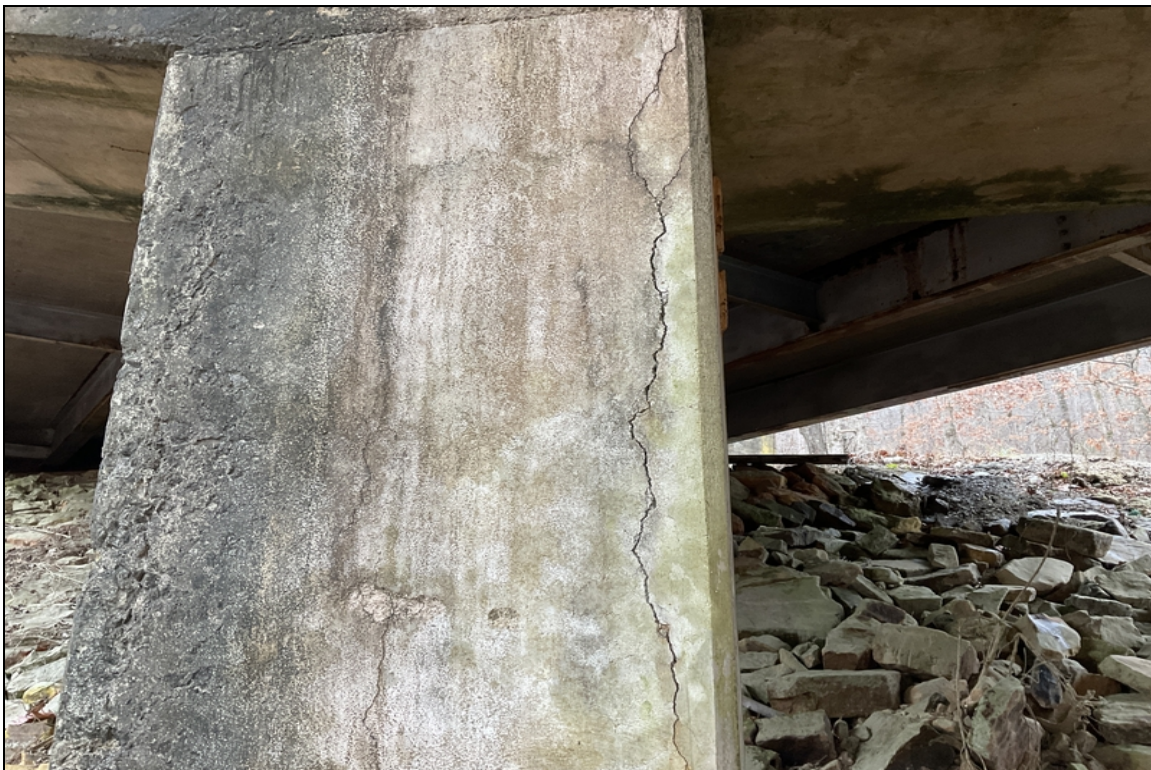
Large crack to ahead side of column 2 @ bent 1.
