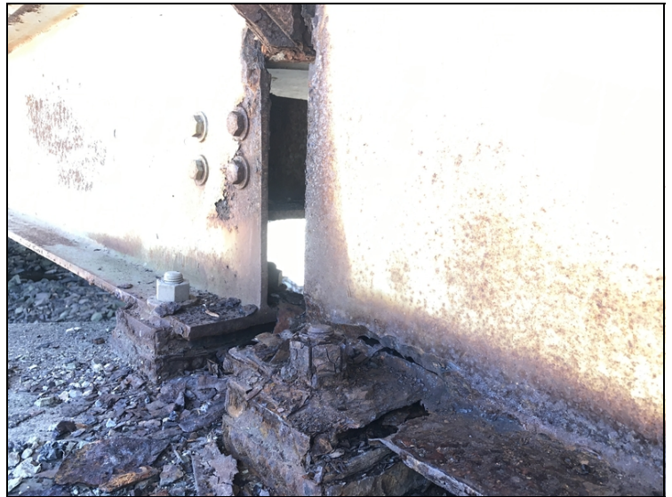
Girder 1 @ end of Span 1 has heavy s/l with holes, cracks & is beginning to crush.
