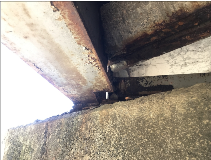
Section loss with large hole to bottom flange @ Girder 5 @ beginning of Span 3.(#4)
