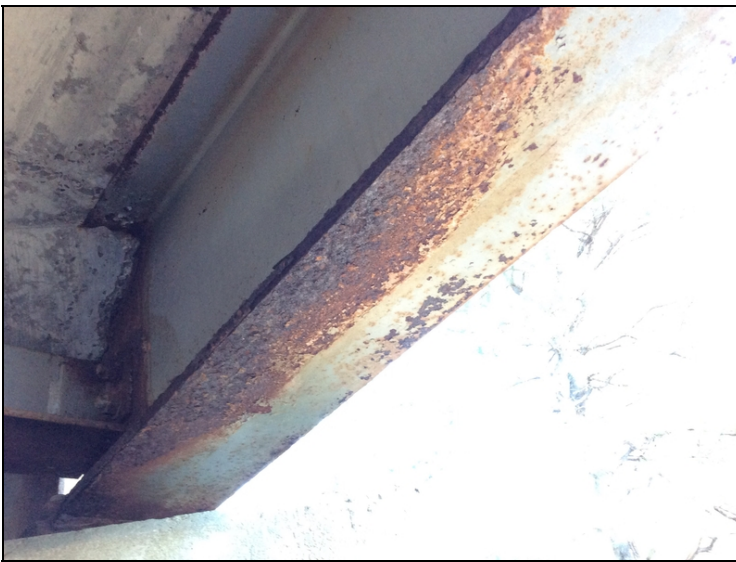
Rust to bottom flange of Girder 5 @ end of Span 2.
