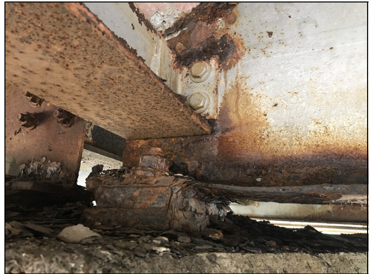
Girder 2 @ end of Span 2 has heavy s/l with holes & is beginning to crush.
