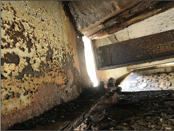
Section loss to bottom flange with hole in web & Crushing to Girder 1 @ end of Span 2.(#4)
