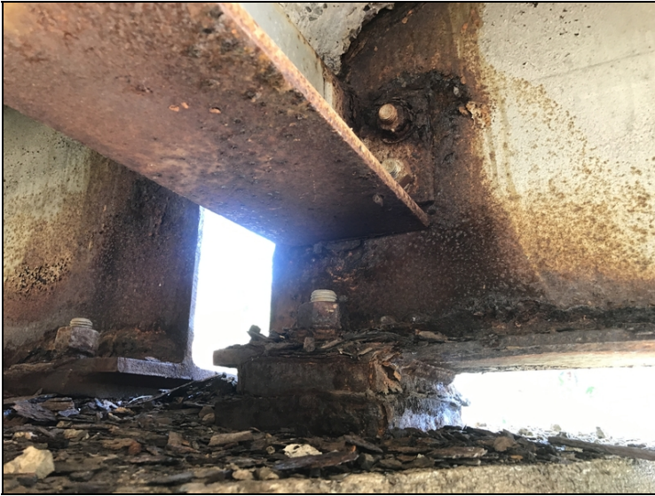
Girder 5 @ end of Span 2 has heavy s/l with knife edge.
