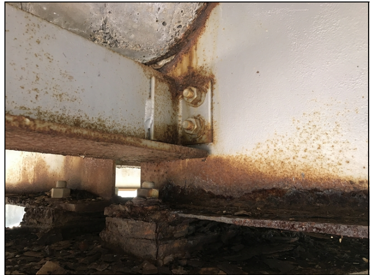
Girder 2 @ end of Span 1 has heavy s/l to bottom flange with holes in web below haunch.(typical to Girders 3 & 4)
