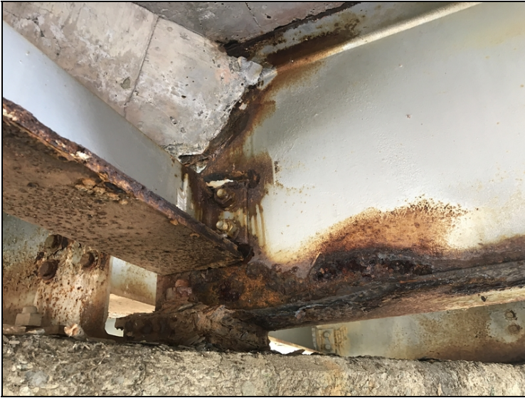
Girder 3 @ end of Span 2 has heavy s/l with holes & is beginning to crush.
