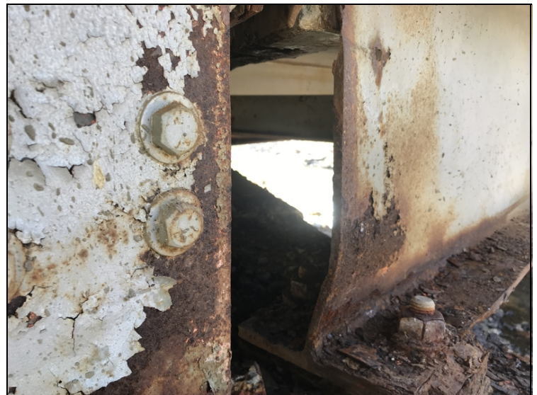
Crushing to Girder 1 @ end of Span 2.(#4)
