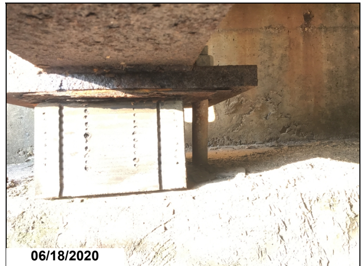
The shim plates between the sole plates and elastomeric bearing pads have active corrosion and are deteriorated. The shim plate for Girder # 1 at the South abutment has rusted into flaking pieces.
