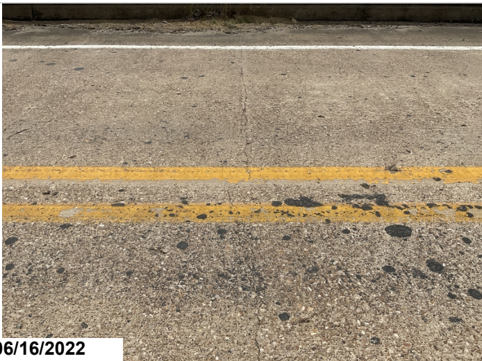
Sealable deck cracking.
