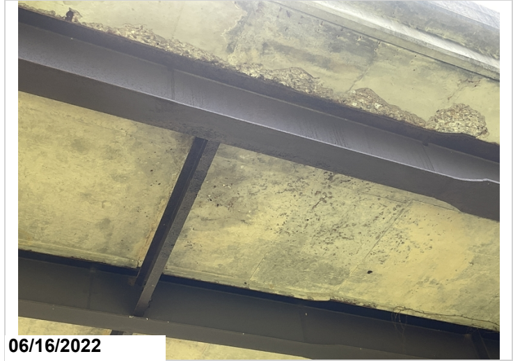
Span #3 beam #1 active corrosion with pack rust.
