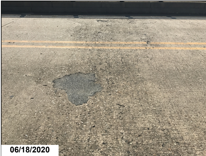
The driving surface of the deck over bent # 3 has scaling with several delaminated areas.
