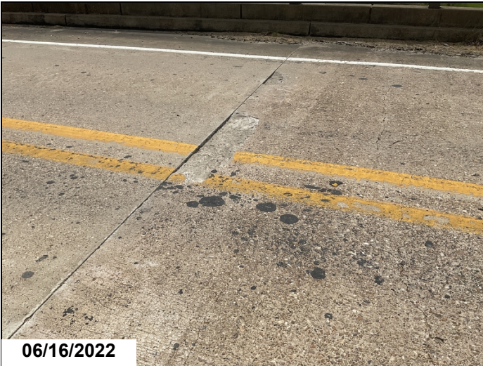
Span #3, spalling on the driving surface of the deck.
