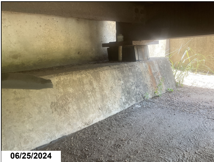
Abutment 2, Bearing 5, Active corrosion with pack rust between loading plate and bearing pad.
