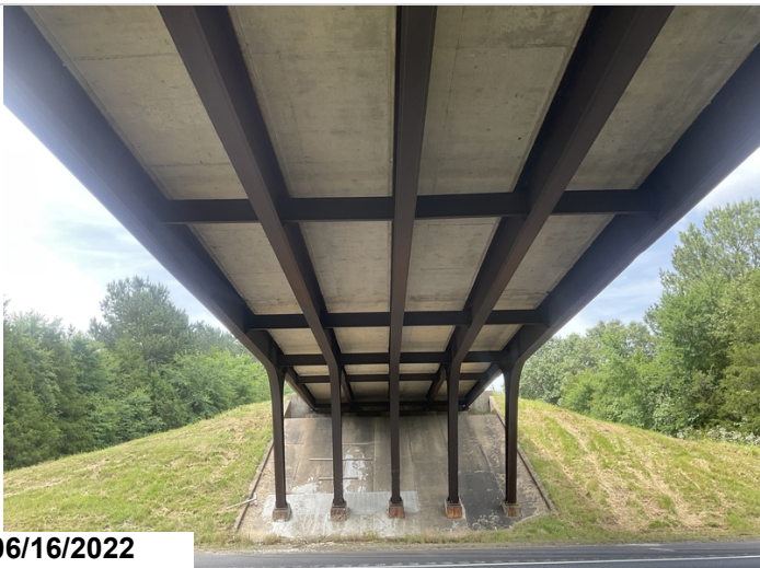
Span #2 no visible delamination over the traveling roadway.
