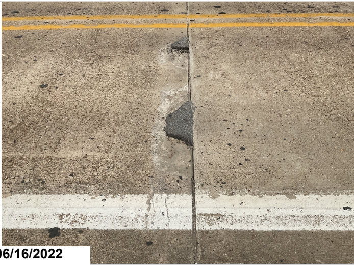
Span #4 spalling with exposed reinforcing steel.
