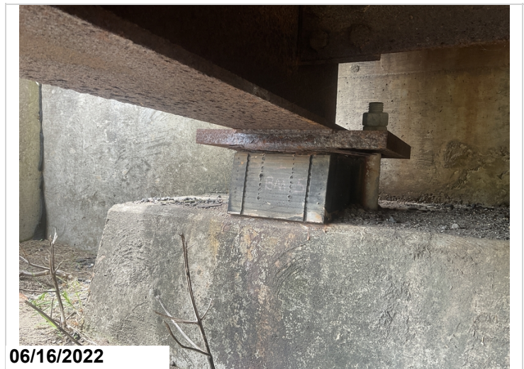
Abutment #1 bearing #5 active corrosion with pack rust.
