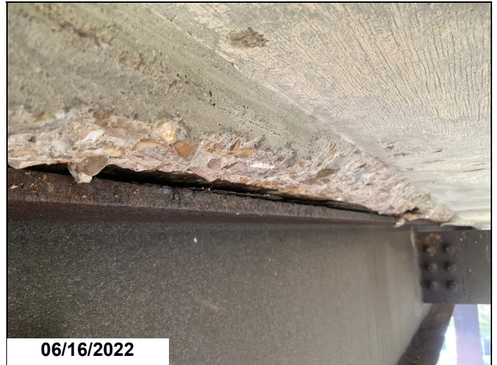
Span #3, Girder #1 deck separation between the deck and girders.
