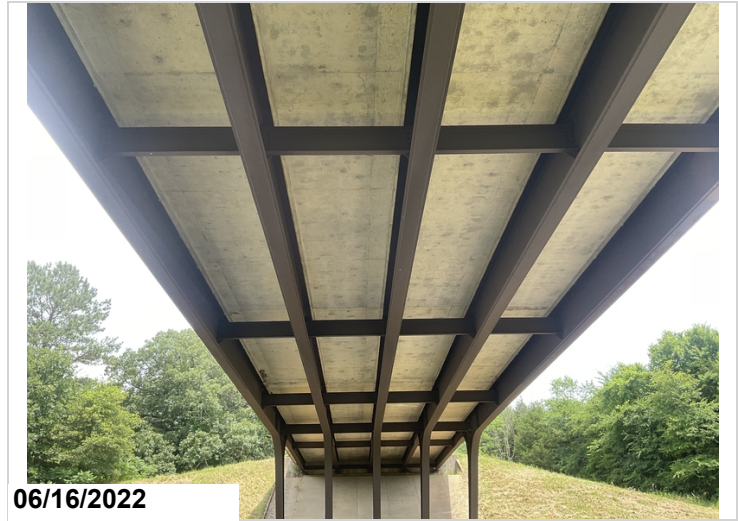
Span #4 no visible delamination over the travel lanes.
