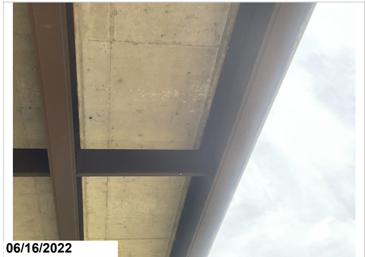
Span #2 beam #5 collision damage with no visible cracks.
