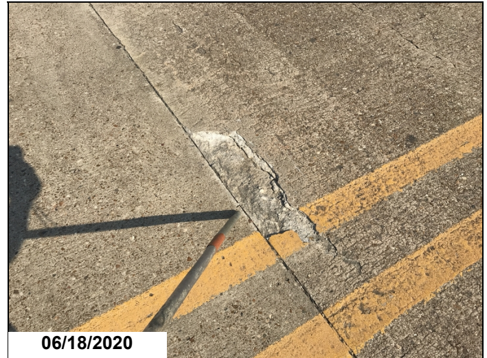
Span 3-Spall near centerline.
