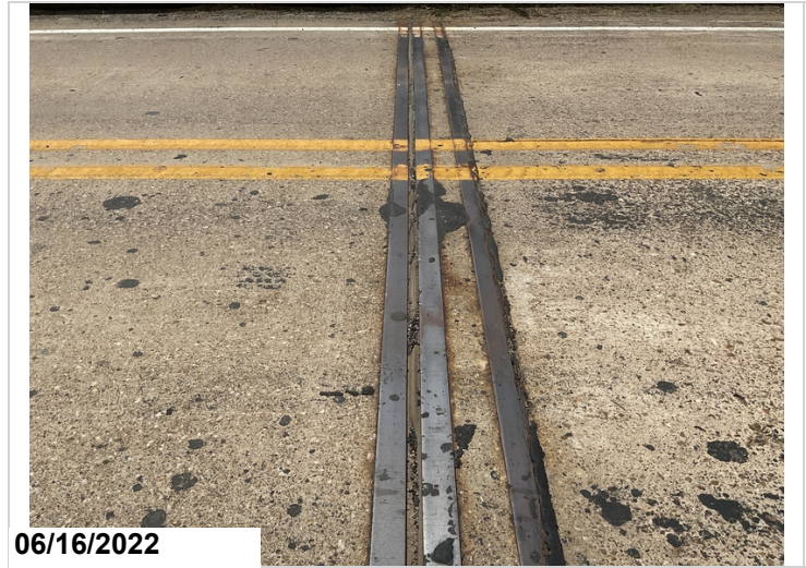
Abutment #2 poured joint seal.
