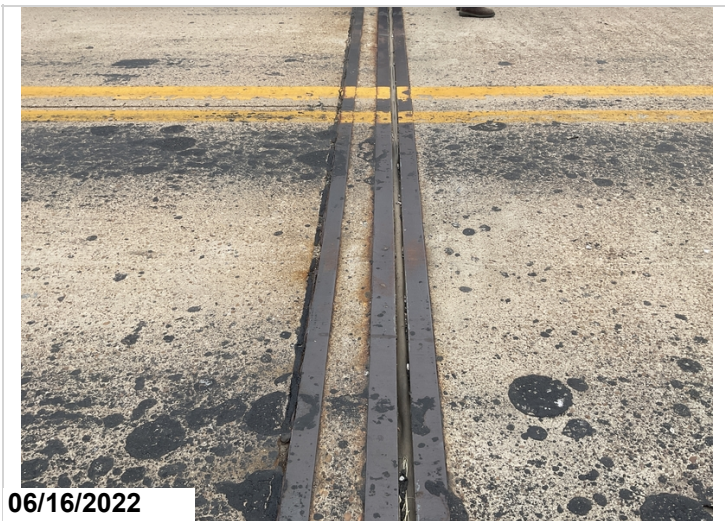
Abutment #1 poured joint seal with adhesion failure in areas.
