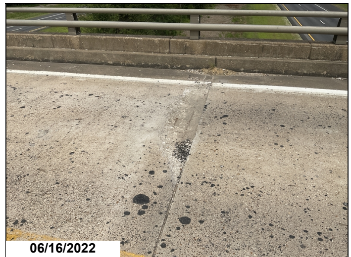
Span #2 spalling with exposed reinforcing steel.
