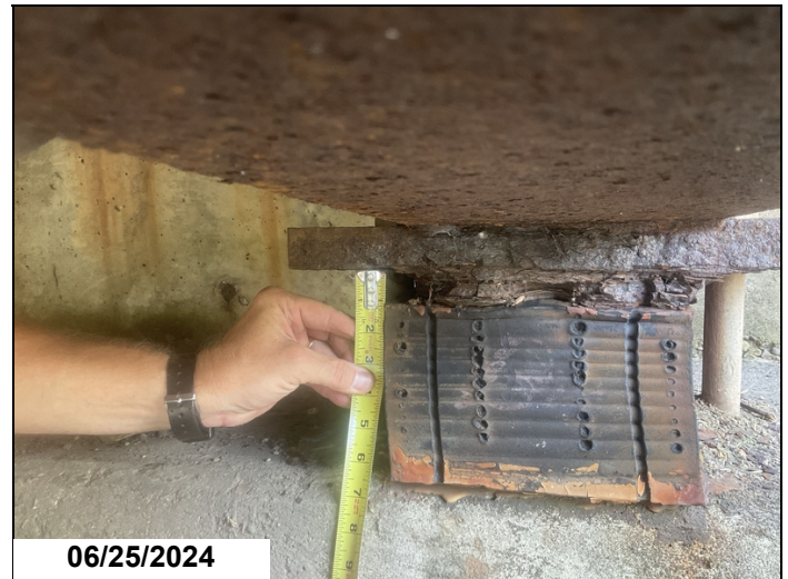
Abutment 1, Bearing 1, has 1" of pack rust between the external loading plate and bearing pad.
