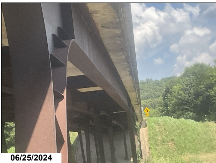
Span 2, Girder 5, out of plane bending due to traffic impact.
