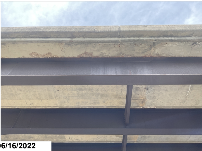
Span #2 beam #5 active corrosion with pack rust along the top flange.
