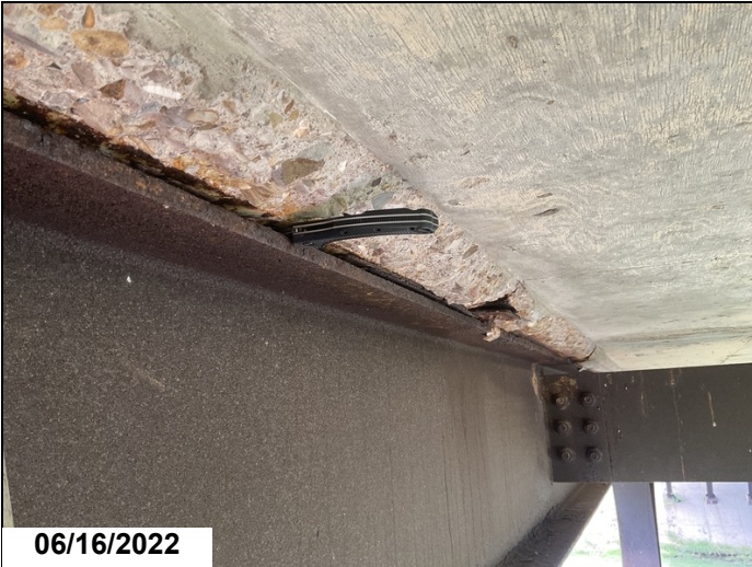
Span # 3, Girder # 1 separation between the deck and the girders.
