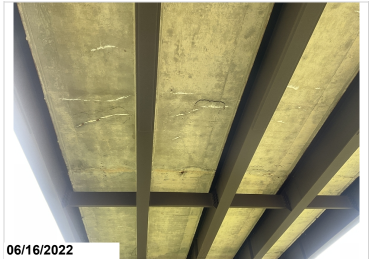
Span #2 transverse cracking with efflorescence buildup and large concrete delaminations.
