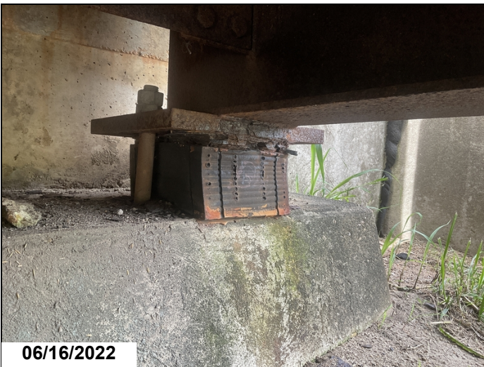
Abutment #1 bearing #1 active corrosion with pack rust.
