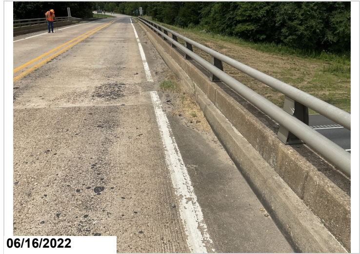
Debris accumulation in the gutters.
