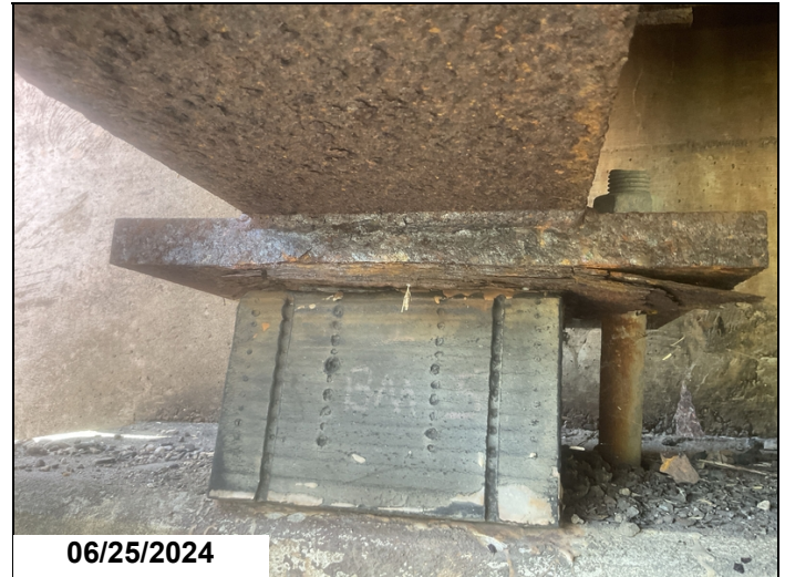
Abutment 1, Girder 5 elastomeric bearing pad has layers of flaking rust in the undersurface of the external loading pad.
