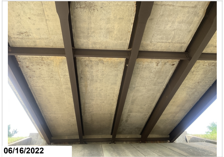
Span #1 typical undersurface of the deck.
