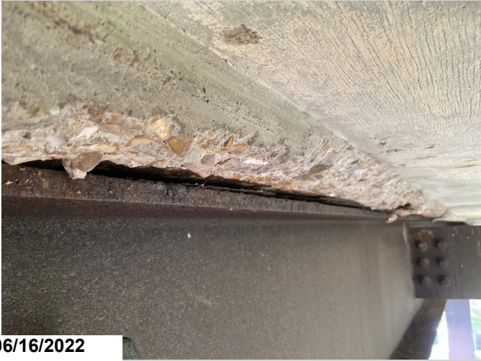
Span #3 beam #1 deck separation between the deck and beams.
