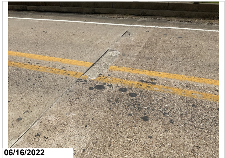
Span #3 spalling on the driving surface of the deck.
