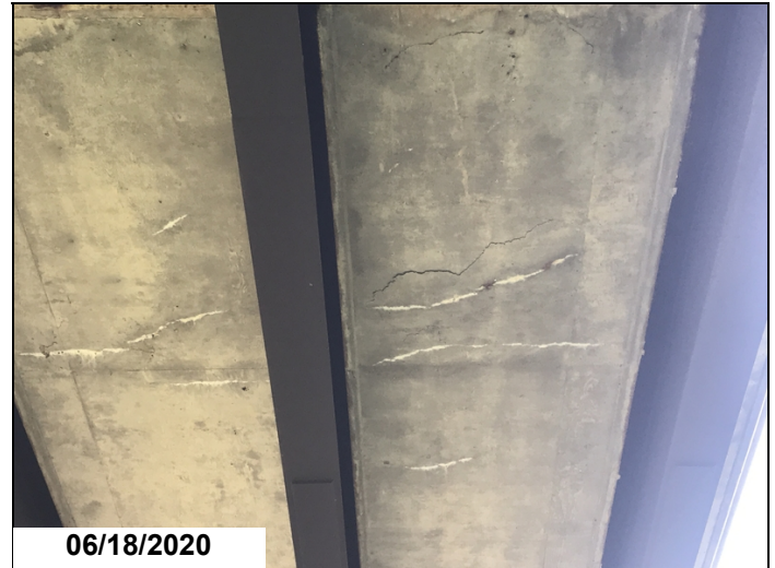
Span 2, bay 1-Delaminated area with transverse cracking with efflorescence.
