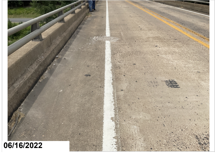
Span #2 Lt spalling in the deck.
