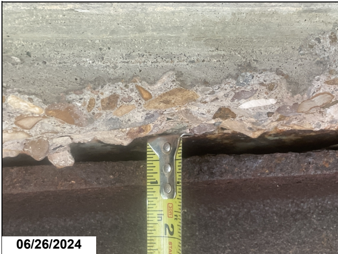
Span 3, Girder 1, Actual field measurement indicates 1/2" air space between the top flange and the undersurface of the deck.
