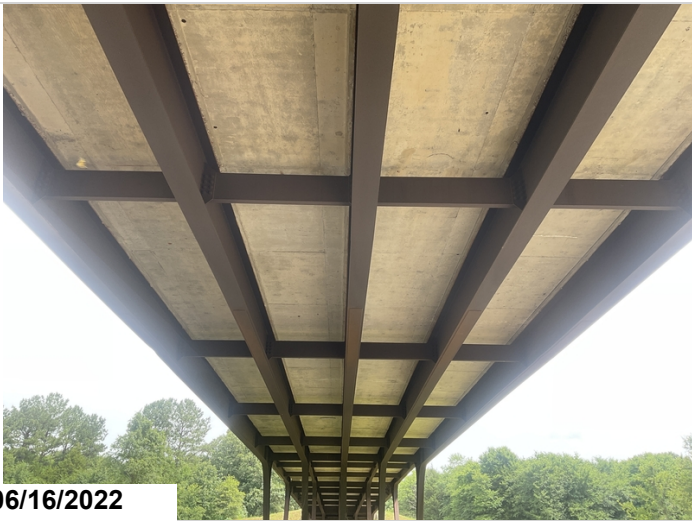
Span #2 typical undersurface of the deck.
