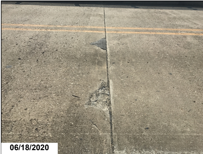
Span 5, left lane-Spalling.
