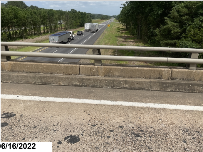
Span #1 Rt rail post with collision damage.
