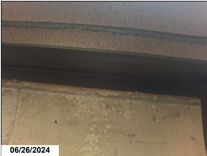
Girder 5, Span 2, Bridge Strike
