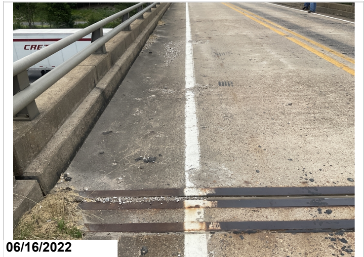
Span #1 Lt spalling in the deck.
