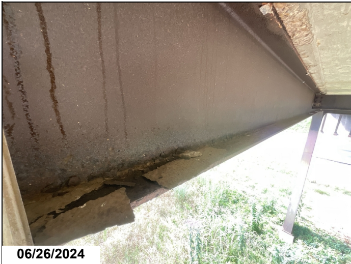
Span 3, Girder 5, Active corrosion and flaking rust on the bottom flange.
