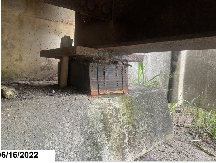
Abutment #1 bearing #1 active corrosion with pack rust.
