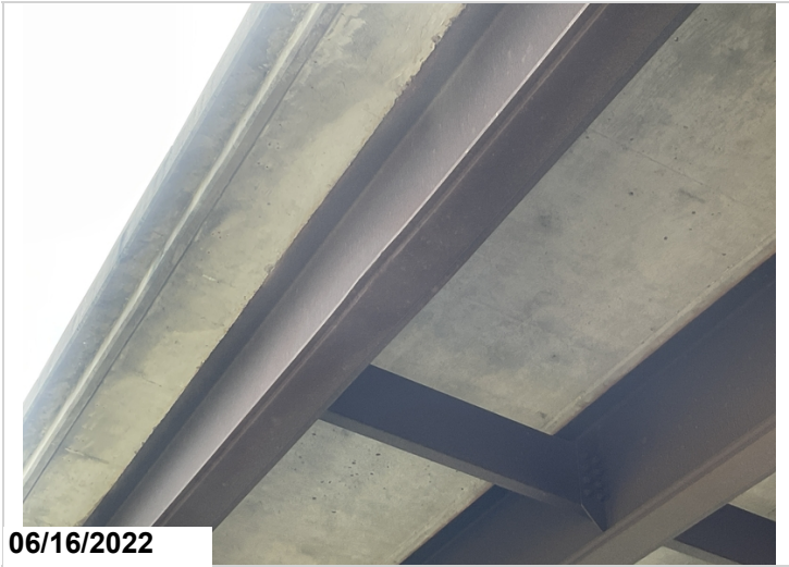
Span #2 beam #1 collision damage with no visible cracks. 06/16/2022
