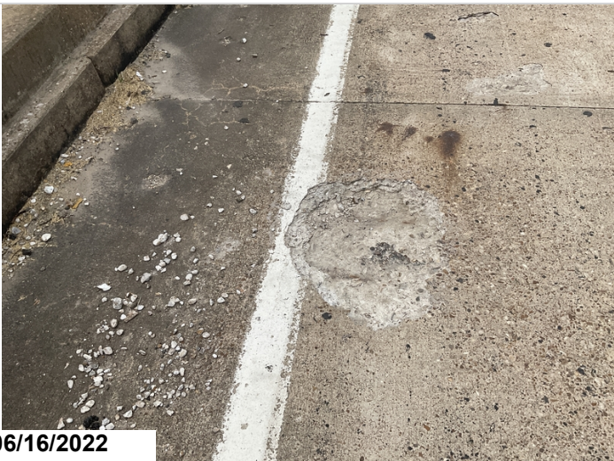
Span #1 Lt spalling with exposed reinforcing steel.
