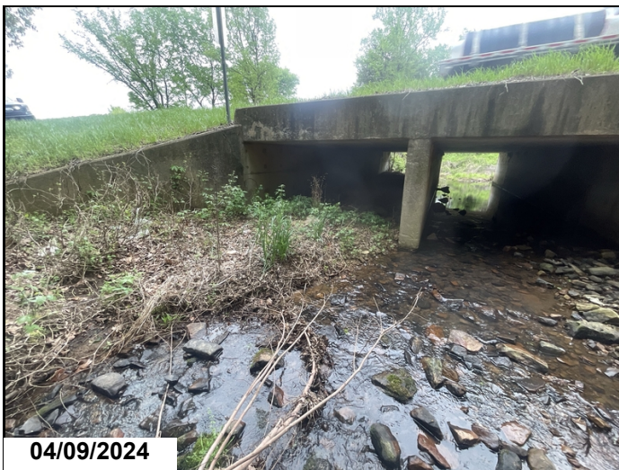
RC Box Culvert - There is approximately 20" of rock accumulation in Barrel # 1.
