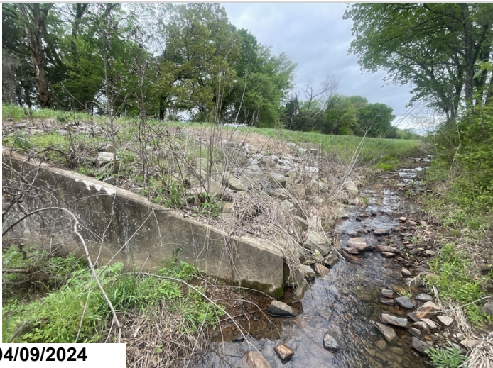
Maintenance forces have placed rip rap in the eroded area behind the Northwest wing wall in the past, repair is still holding.
