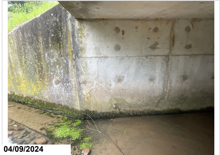
Barrel # 2 Exterior wall, left end has a diagonal crack with efflorescence adjacent to the wing wall juncture. 3LF CS2
