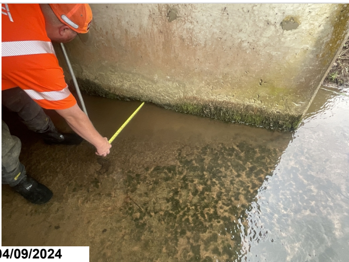
The base of Wall # 2 Ahead face, Right side has minor concrete deterioration up to 2" deep. 1' long x 3 1/2" tall x 3" deep concrete section loss. 1LF CS3
