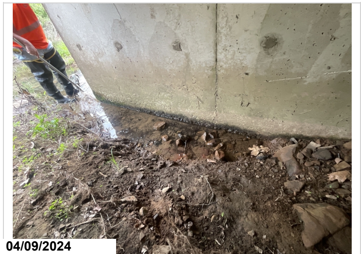
Wall # 2. Abrasion. 7LF CS3
