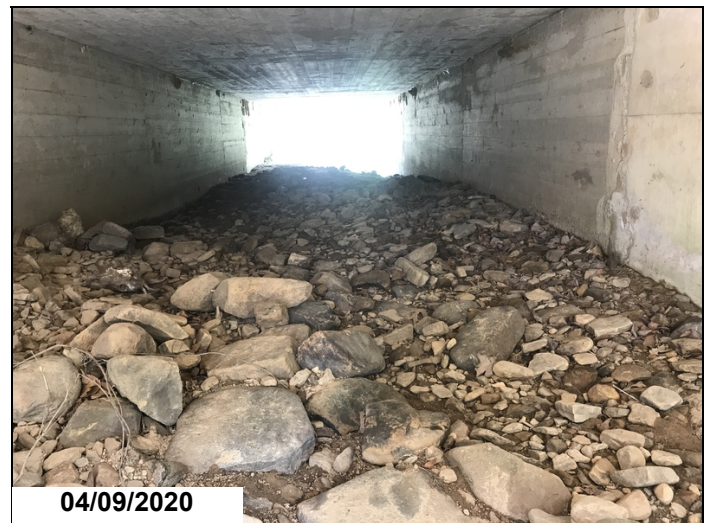
Barrel # 1-Streambed material accumulation.
