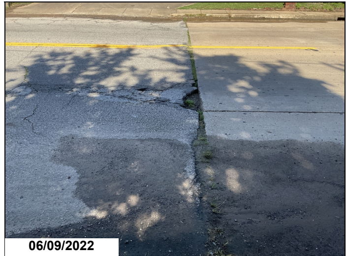
South approach roadway potholes at the end of the approach slab.
