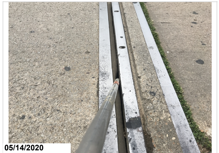
The pourable type expansion joint sealant at abutment # 2 (North abutment) has adhesion failure in the driving lane allowing water, dirt and debris to leak onto the substructure.
