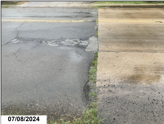
South approach Pot hole. Maintenance Forces have filled the pot hole with an asphalt patch.
