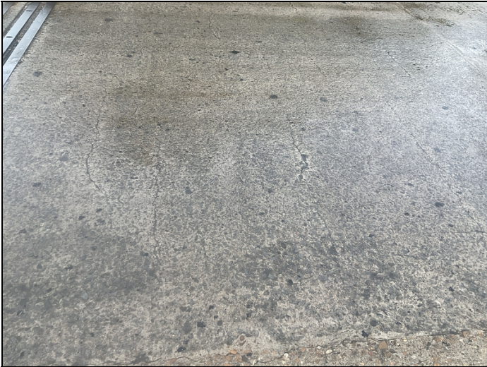
Sealable map cracking in the deck.
