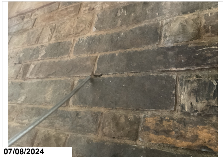
Abutment 2 has one small area of mortar deterioration between the stone. 1 LF CS2
