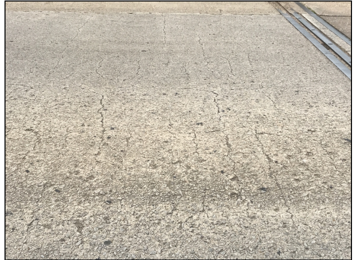
Right lane at abutment 2-Mapcracking.
