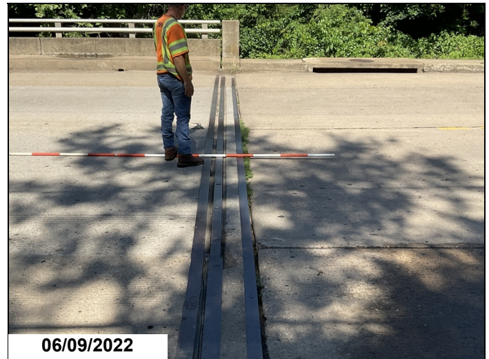
North approach slab settlement.
