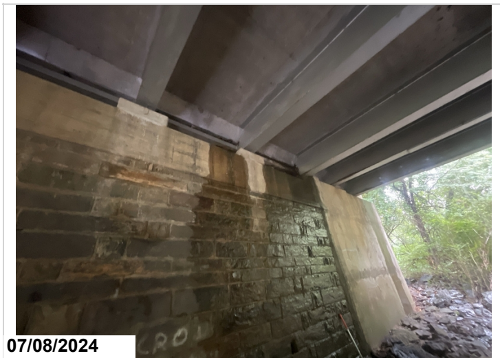
Abutment 2. Expansion joint seal leaking.
