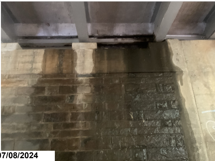
Abutment 2, Joint leakage.
