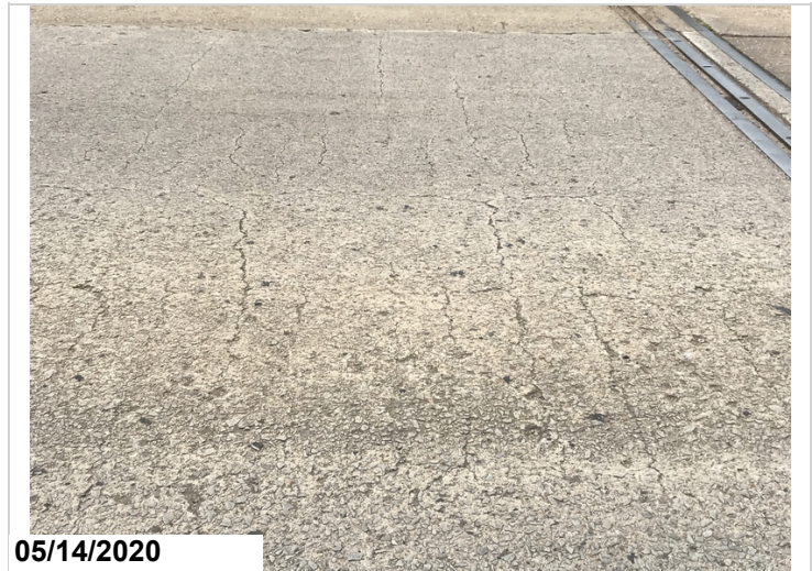
Right lane at abutment 2-Mapcracking.
