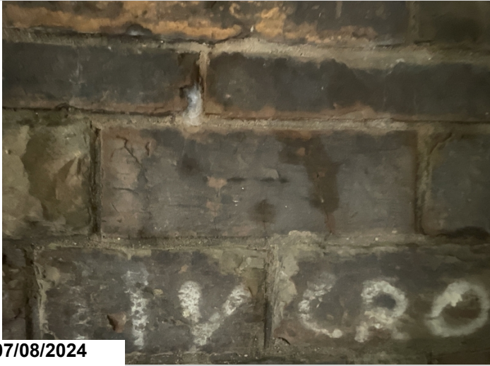
Abutment 2. Vertical crack in a stone.
