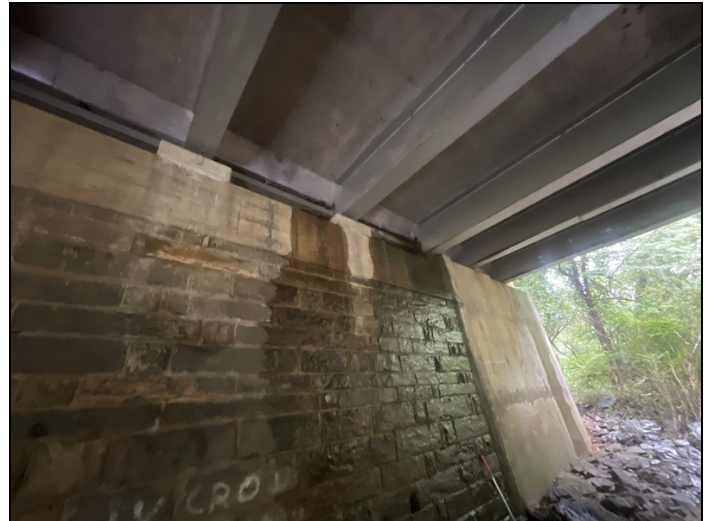
Abutment 2. Expansion joint seal leaking.
