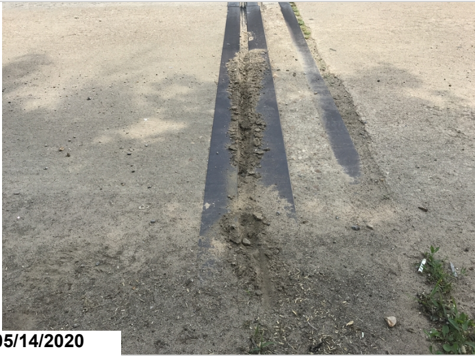
The pre-formed compression joint seal at abutment # 1 has dirt and debris causing adhesion failure.
