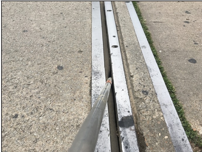
The pourable type expansion joint sealant at abutment # 2 (North abutment) has adhesion failure in the driving lane allowing water, dirt and debris to leak onto the substructure.
