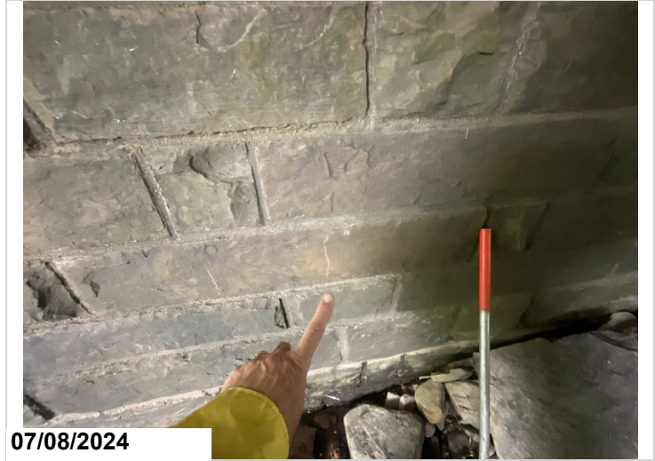
Abutment 2. Vertical crack in a stone.
