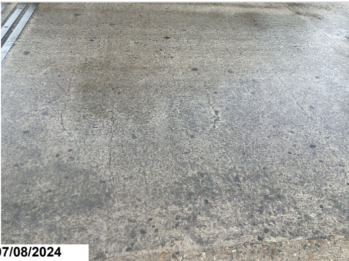
Sealable map cracking in the deck.
