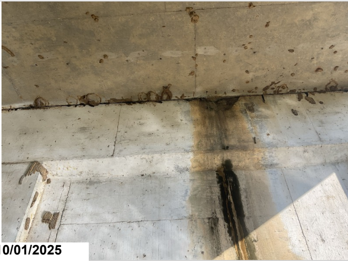
Bent 3, Back face, Right: 1'-6" spall.
