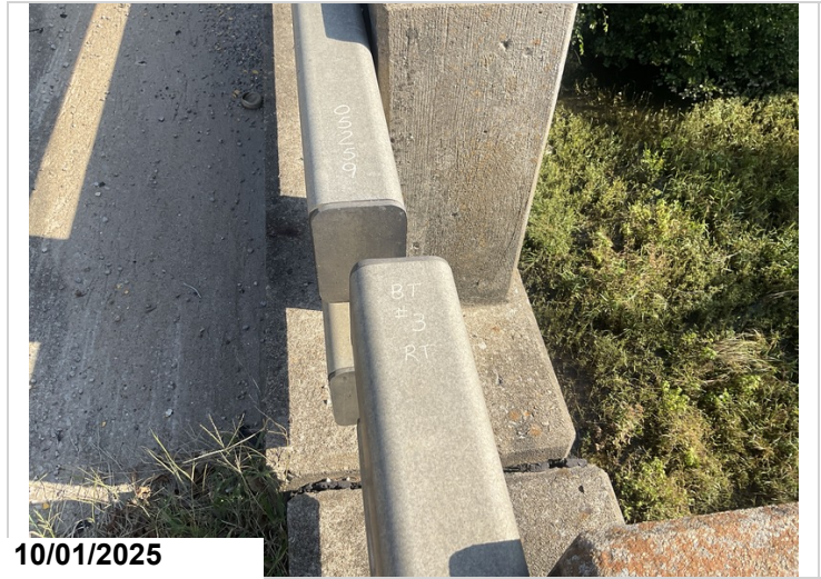
Minor offset in edge of slab over the intermediate bents: Typical for slab span structures on a skew.
