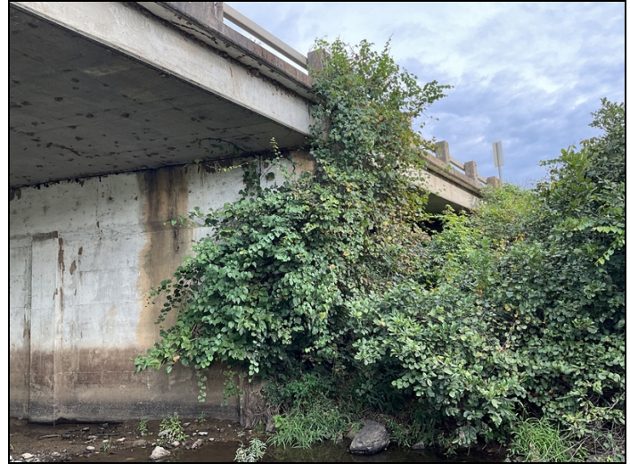
Bent 4 right side has vegetation growth.
