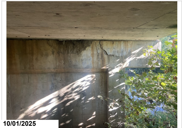
Bent 2 cap, Back face, Right: Spalls with exposed reinforcing steel and delaminated areas.
