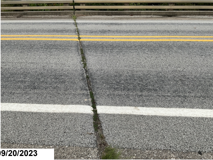
Bent 1, 2, and 3 has debris impaction with vegetation growth in joints.
