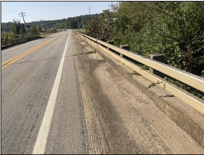
Deck shoulders have minor debris and gravel.
