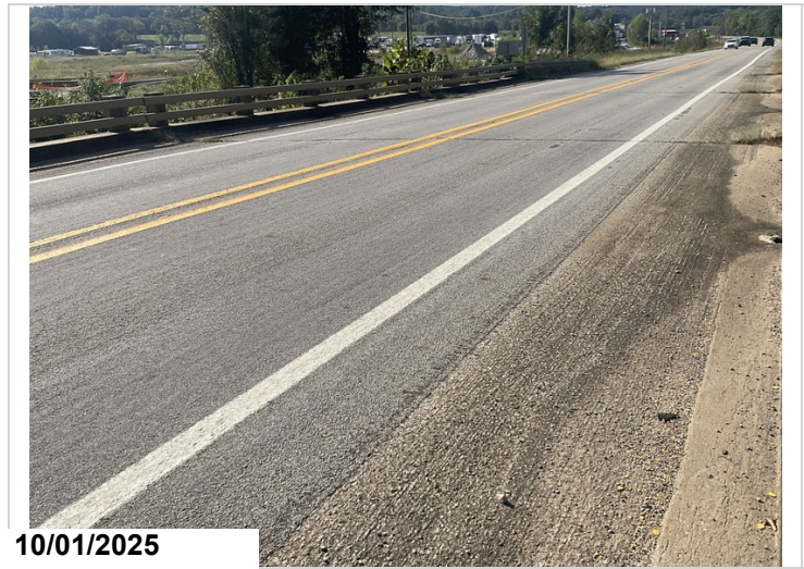
Chip and seal wearing surface, Typical.
