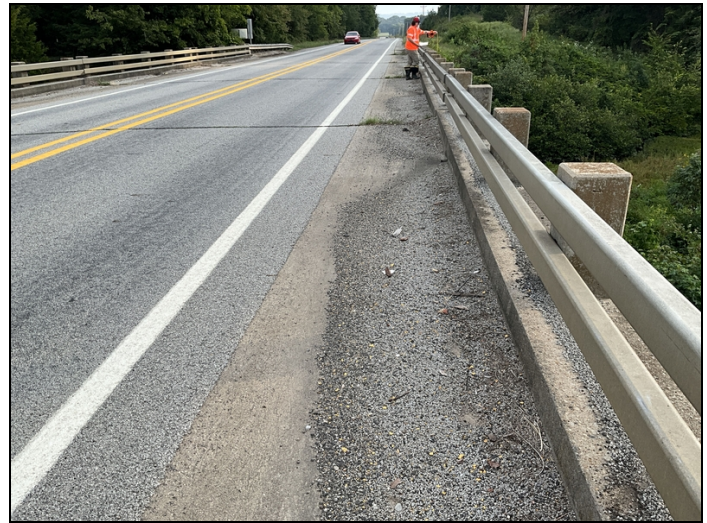
Deck shoulders have debris and gravel.
