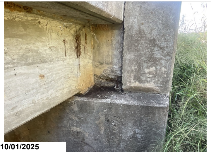
Abutment 1, Left: One 4" spall with exposed reinforcing steel. 1LF CS3
