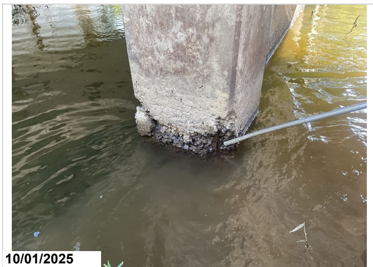
Bent 3, Column 1, Base at water elevation: Concrete deterioration up to 5" deep with exposed reinforcing steel. 1EA CS3
