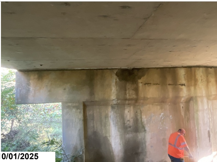
Bent 2 cap, Back face, Left: Spalls with exposed reinforcing steel and delaminated areas.
