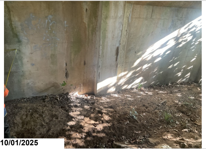
Bent 2, Backface, Adjacent to column 2: Two 10" spalls with exposed reinforcing steel. 2LF CS3
