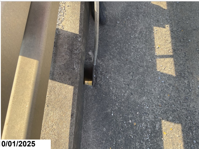
Deck drain, Span 2, Right: Exposed reinforcing steel. 1SF CS2
