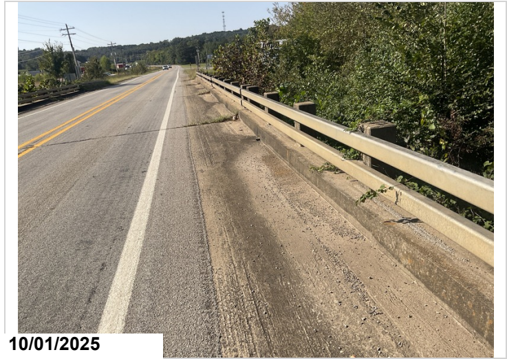
Deck shoulders have minor debris and gravel.
