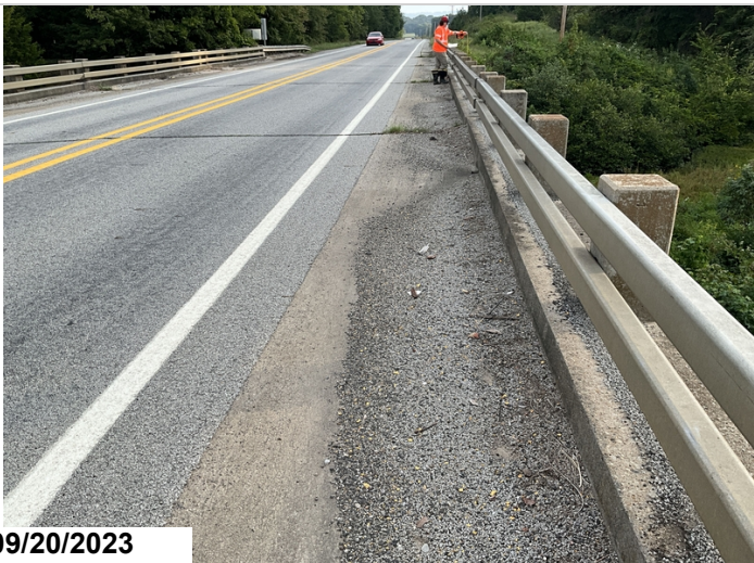
Deck shoulders have debris and gravel.
