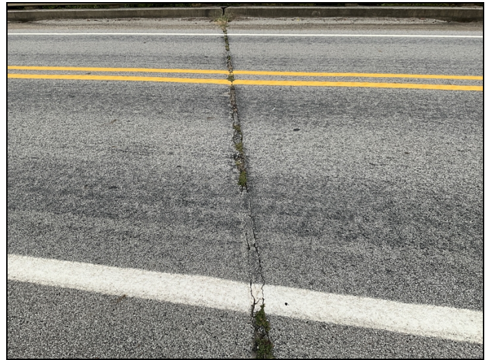
All joints have asphalt in joint that needs to be removed.
