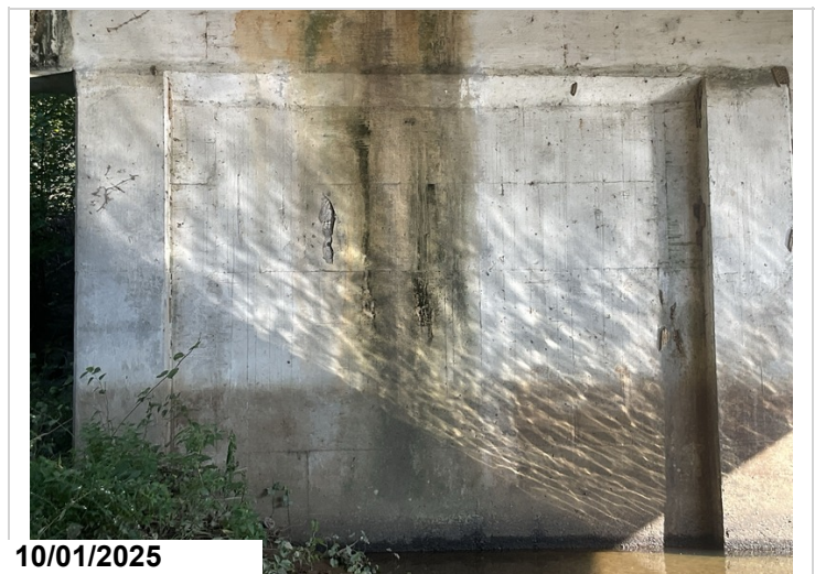
Bent 4, Back face, Left: 1'-8" vertical spall with no exposed reinforcing steel. 1LF CS3
