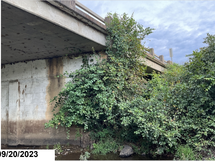
Bent 4 right side has vegetation growth.
