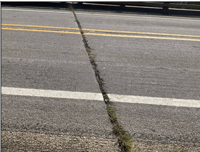
Expansion joint over Bent 4, Debris accumulation
