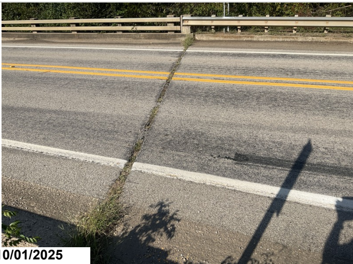
Abutment 2, Expansion joint: Debris accumulation.
