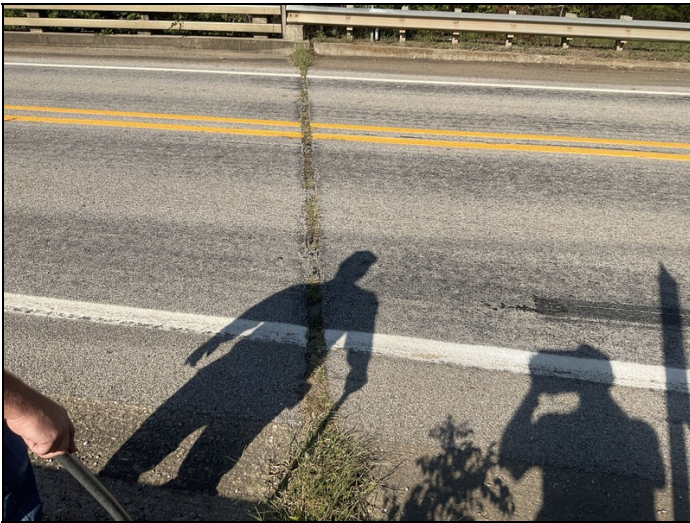
Abutment 2: expansion joint: debris accumulation.
