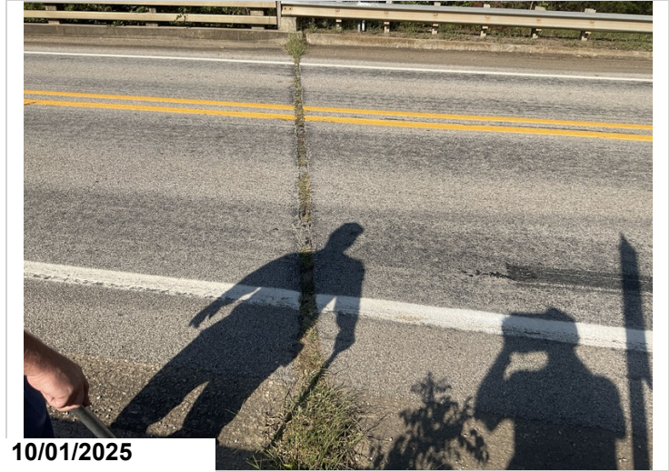
Abutment 2: expansion joint: debris accumulation.
