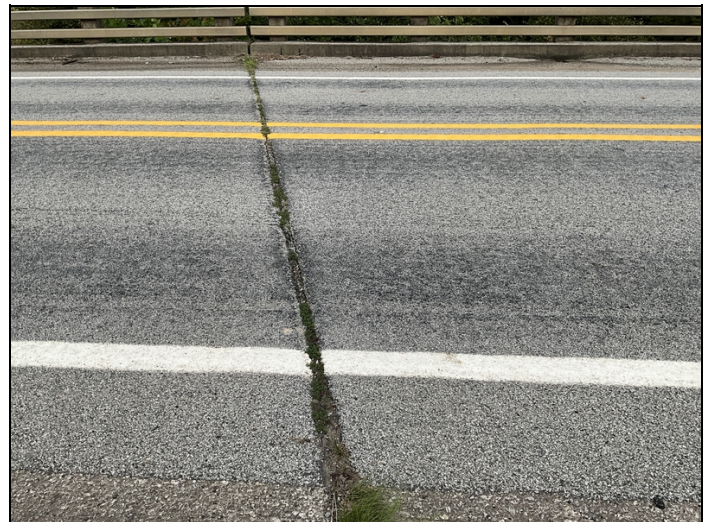
Bent 1, 2, and 3 has debris impactation with vegetation growth in joints.
