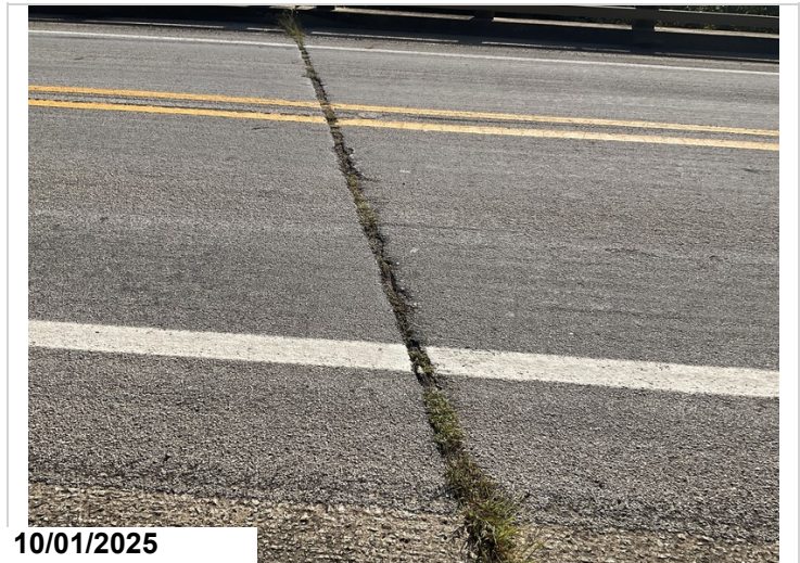
Expansion joint over Bent 4, Debris accumulation
