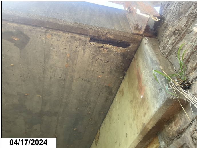
Span # 2, Right edge, Undersurface of slab has one 12" spall with exposed reinforcing steel with approximately 1/8" section loss located adjacent to Abutment # 2.
