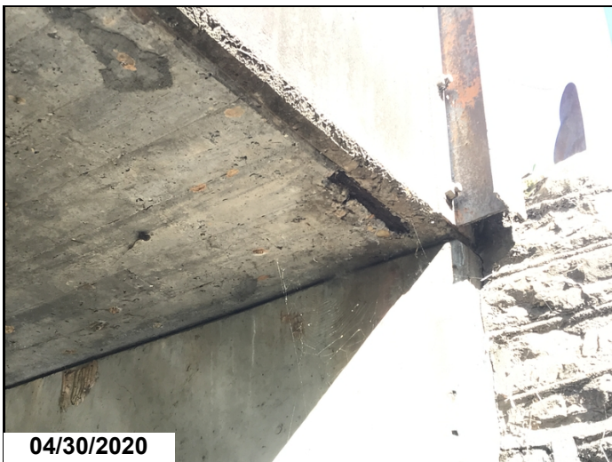
Span # 2, right side-Spall with exposed reinforcing steel adjacent to abutment # 2.
