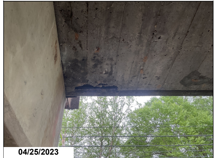
Span # 2 Rt spalling with exposed reinforcing steel.
