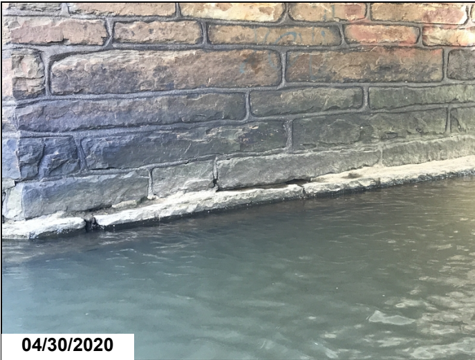
Abutment # 2-Minor grout deterioration.
