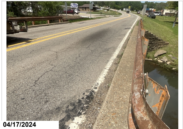
Minor debris and vegetation in the gutters.
