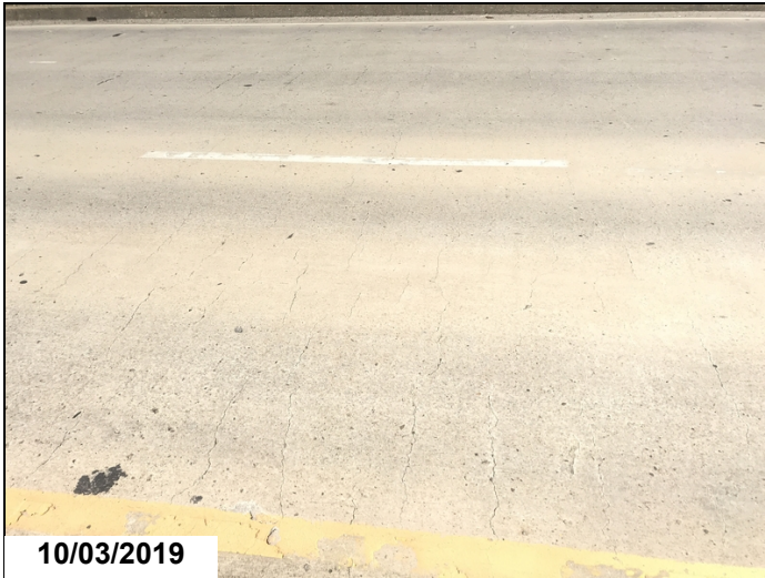
Span # 3 transverse cracking.
