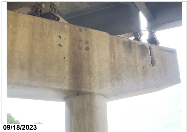
Bent # 3 Span # 3 has an 18" spall with exposed reinforcing steel in the Left side of cap and several smaller vertical delaminated areas in Bay # 2.
