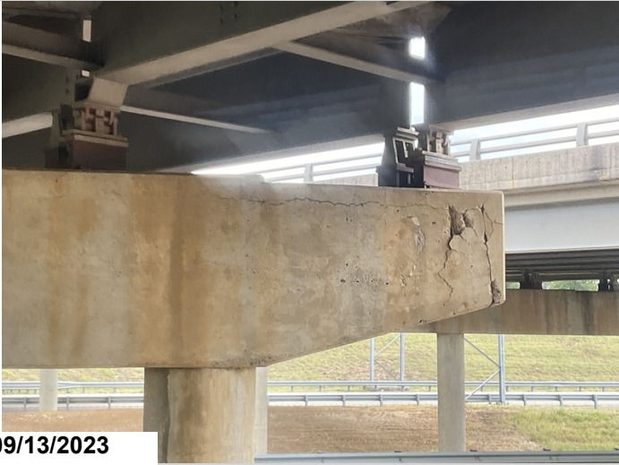
Bent # 2, Right side of cap has a 2' area with delaminated areas, map cracking, and spalls with exposed reinforcing steel with initial section loss.
