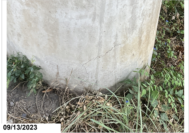
Bent # 3 column # 2 has random cracking at the base.
