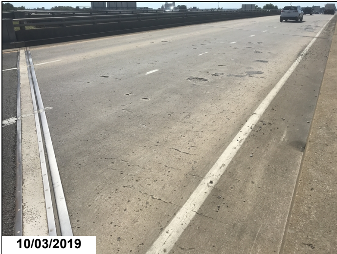
The driving surface of the deck has sealable cracking, large delaminated areas and numerous spalls with exposed reinforcing steel. The temporary asphalt patches have failed in several locations.
