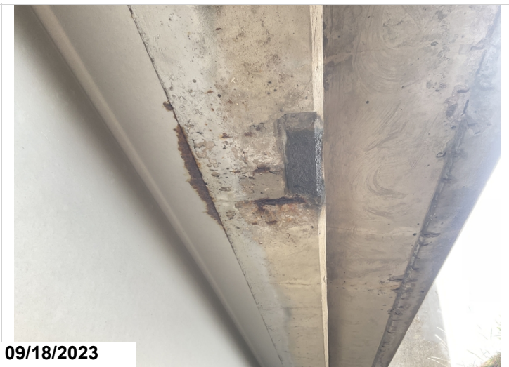
Spalling with exposed reinforcing steel around deck drain.
