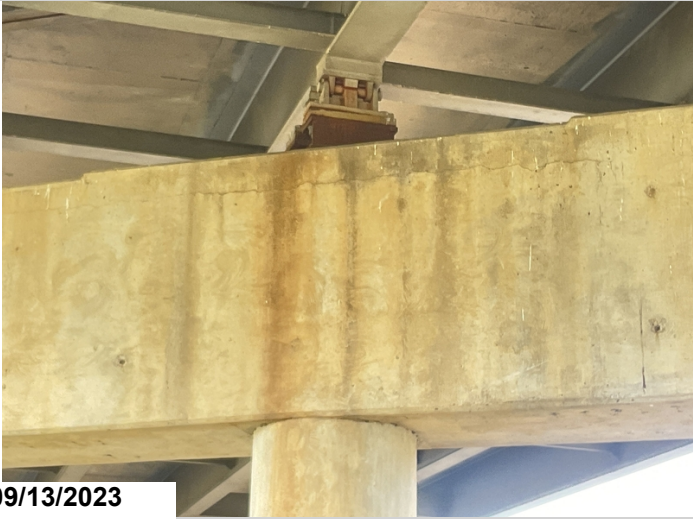
Bent # 4 has a horizontal crack located approximately 6" below the top of the cap.
