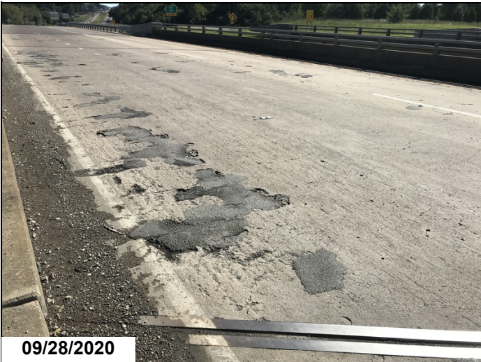
The driving surface of the deck has sealable cracking, large delaminated areas and numerous spalls with exposed reinforcing steel. The temporary asphalt patches have failed in several locations. Span # 2 pictured.
