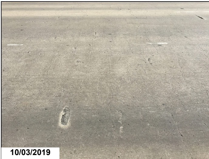
Span # 3 cracking.
