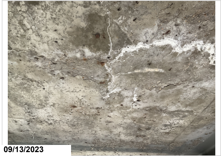
Span 5, bay 1, undersurface scaling and cracking with efflorescence.
