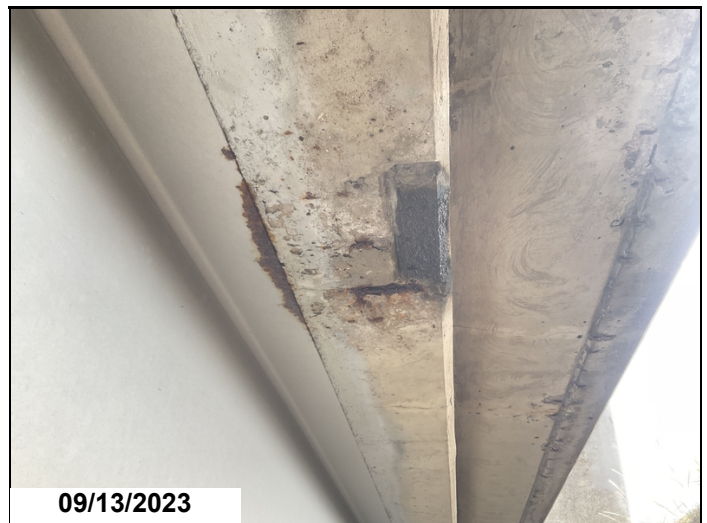
Corrosion to top flange of beam # 1.
