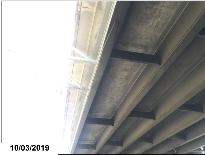
Span # 2 Beam # 1 old traffic impact scar.
