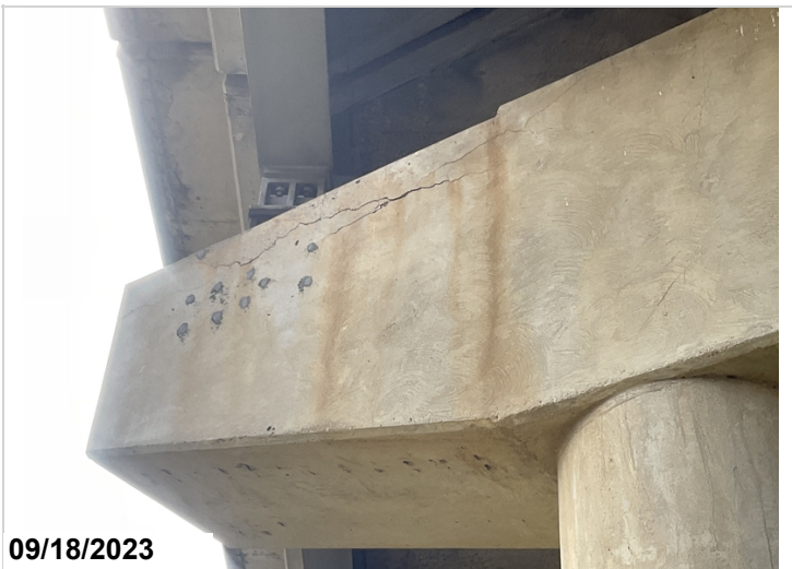
Bent # 3 has horizontal / map cracks located approximately 8" below top of cap in Bays # 1, 4, 5, & 6.
