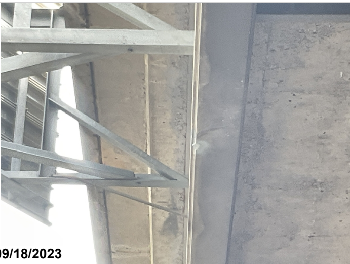
Span # 2, beam # 1 over right lane has a 2" x 2" x 1/2" notch in the bottom cover plate due to traffic impact.
