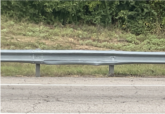
Minor collision damage, left east rail
