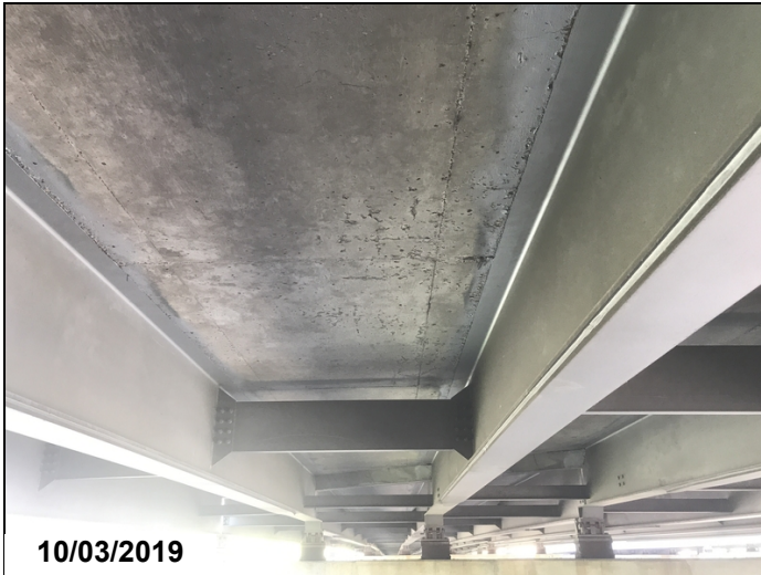
Span # 1 Bay # 2 map cracking and concrete scale on the undersurface of the deck.
