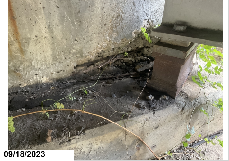
-Abutment # 1 has a 2' spall with exposed reinforcing steel with approximately 1/8" section loss to the reinforcing steel located in the left end of the abutment.
