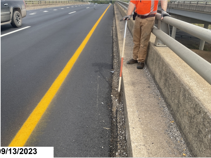
Dirt and debris in gutters
