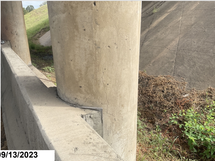
Bent # 5, Column # 3 has vertical cracking near the base of the column
