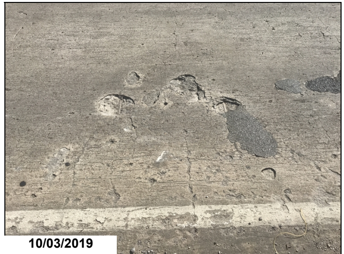
Span # 4 spalling with exposed reinforcing steel.
