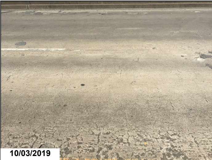
Span # 4 transverse cracking.
