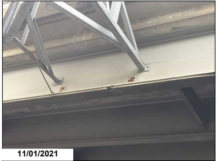
Span # 2, beam # 1 has a 2" X 2" x 1/2" notch in the bottom cover plate due to traffic impact locate above the Rt lane.
