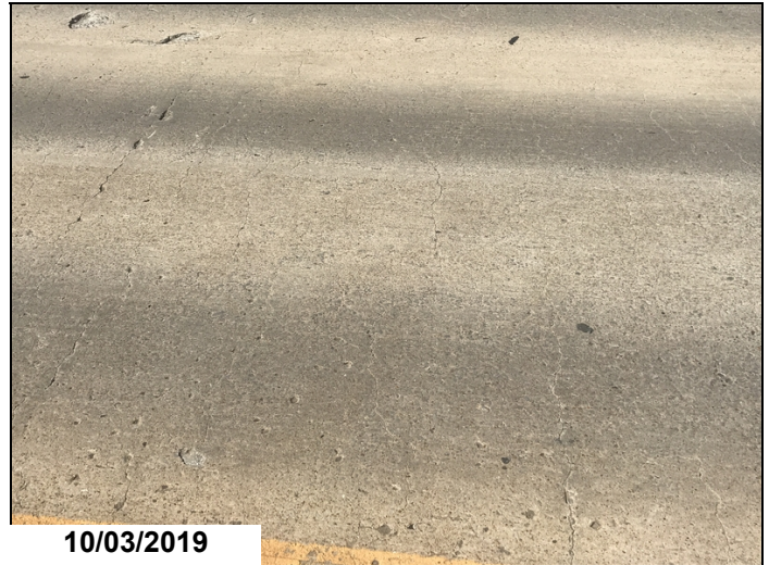
Span # 5 transverse cracking.
