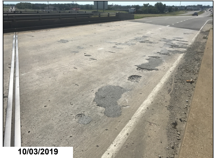
The driving surface of the deck has sealable cracking, large delaminated areas and numerous spalls with exposed reinforcing steel. The temporary asphalt patches have failed in several locations. Span # 1 pictured.
