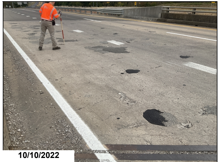
The driving surface of the deck has sealable cracking, large delaminated areas and numerous spalls with exposed reinforcing steel. The temporary asphalt patches have failed in several locations. Span # 5 pictured.
