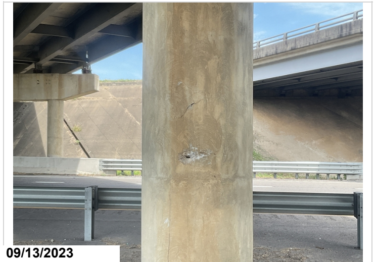
Bent # 4, Column # 2 has a softball sized spall with exposed reinforcing steel and an 8" delaminated area just above the spall.
