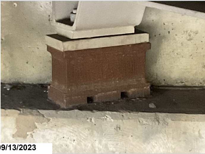
Abutment 2 typical bearing.
