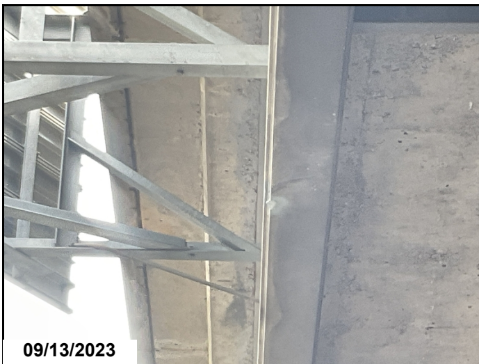
09/13/2023 - RSM - Maintenance forces have painted the area of collision damage to beam # 1 bottom flange cover plate in span # 2 since last inspection.
