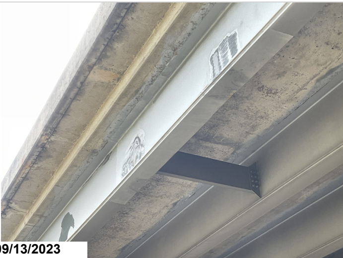
Span # 4, beams # 1 & 2 have old impact scars
