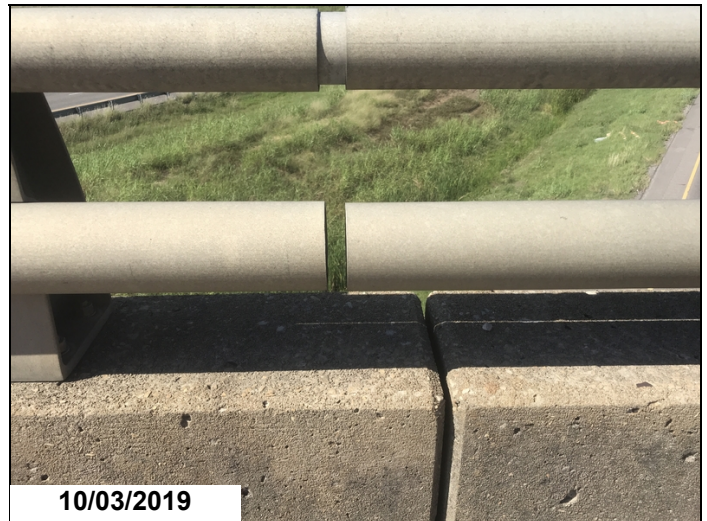
Bridge railings have several loose tube connections that have vibrated out of position.
