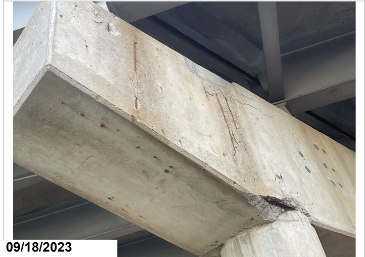
Bent # 5 has several 3' long vertical spalls with exposed reinforcing steel with initial section loss in the Left side of cap.
