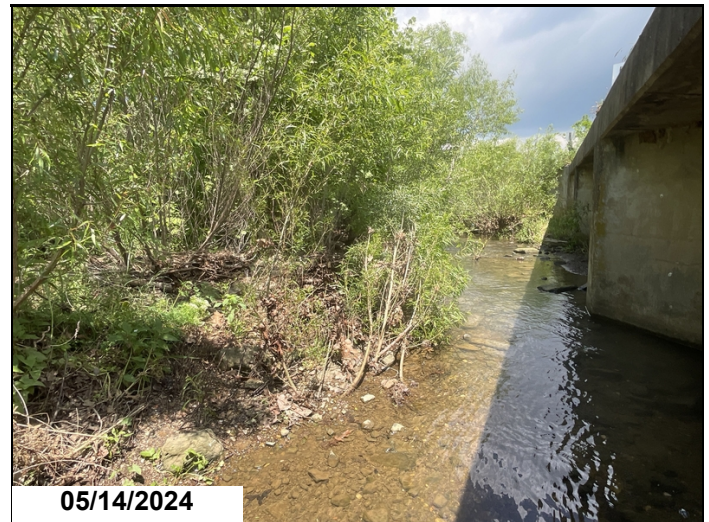
Vegetation and debris restricting the outlet end of channel.
