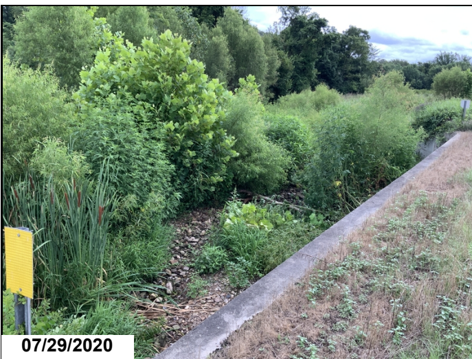
Outlet end small trees restrict the channel flow.
