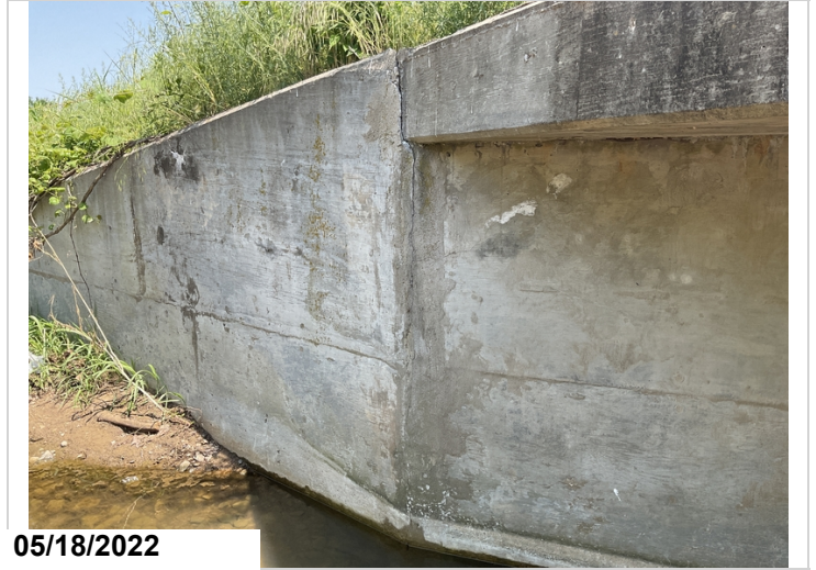
Barrel 1, Right, Wing Wall: Cracking.
