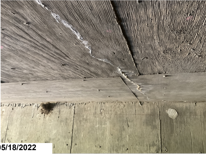
Typical cracking with efflorescence.
