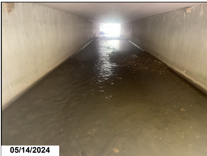
Barrel 1. Gravel accumulation.
