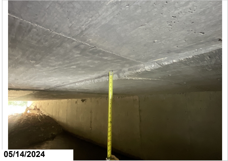
Barrel 3, Top slab, Area where forms sagged approximately 2" during the construction process.
