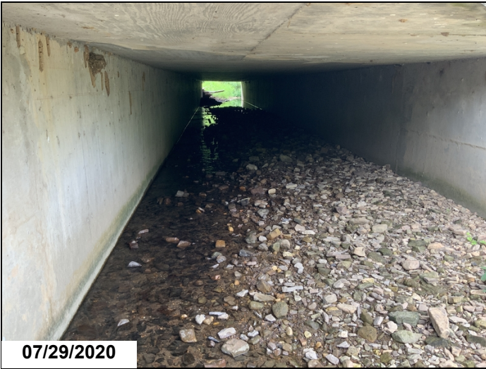
Barrel 3 Debris accumulation.
