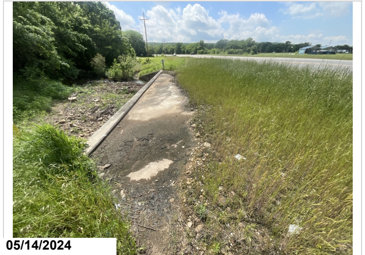
Right side of structure, Up to approximately 7' of the top slab exposed.
