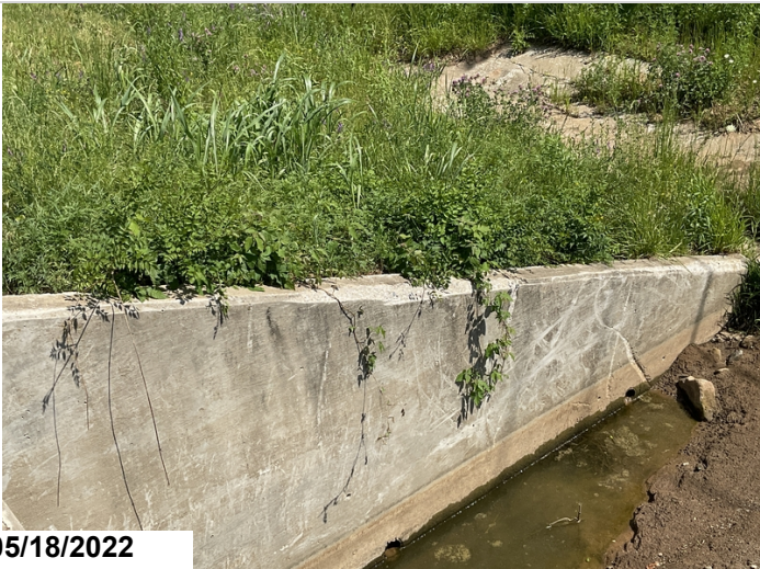
Barrel 3, Right, Wing Wall: Spalling.
