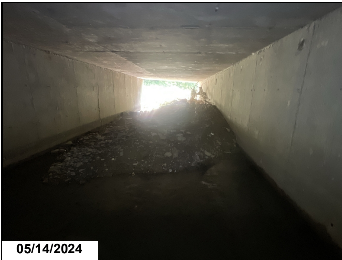
Barrel 3. Up to approximately 3' of gravel accumulation.
