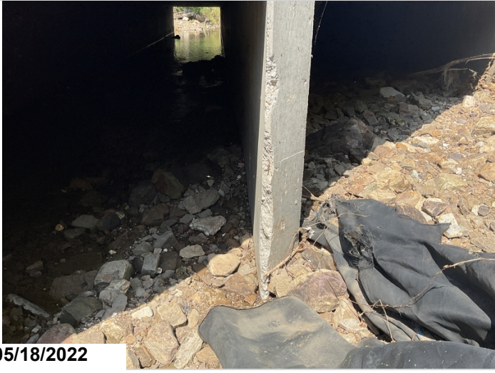
Intermediate Wall: Spalling.
