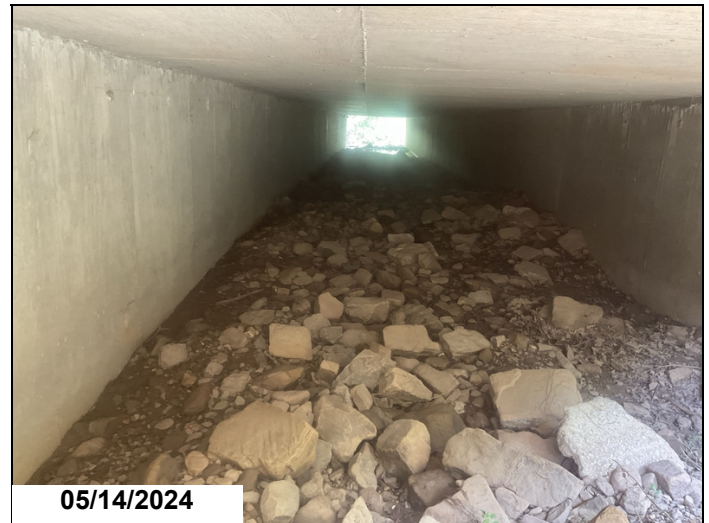
Barrel 2. Gravel accumulation.
