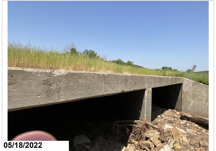
Head Wall, Right: Minor spalling.
