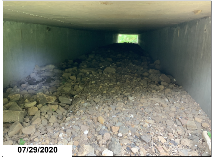
Barrel 2 Debris accumulation.
