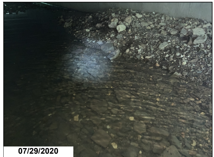
Barrel 3 Debris accumulation.
