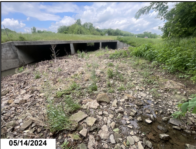
Right side of structure. Gravel accumulation.
