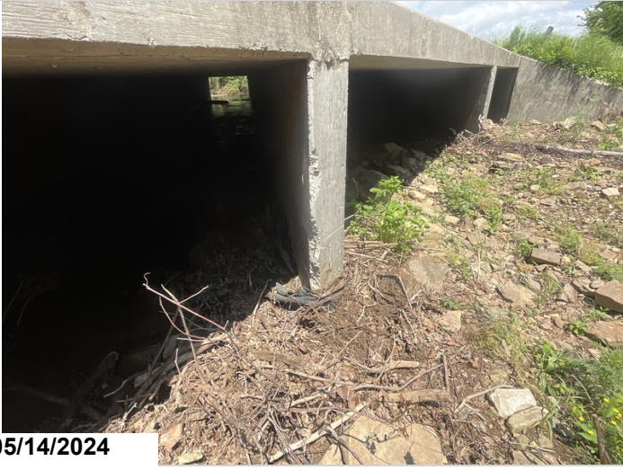
Barrel 1, Right, Wall 2 has a 3' tall spall with no exposed reinforcing steel.
