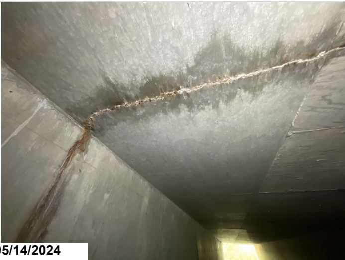
Barrel 2, Top slab, Transverse crack with efflorescence and rust stains.
