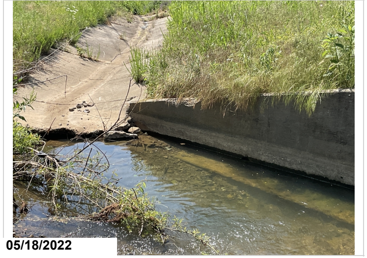
Barrel 1, Right, Wing Wall: Spalling.
