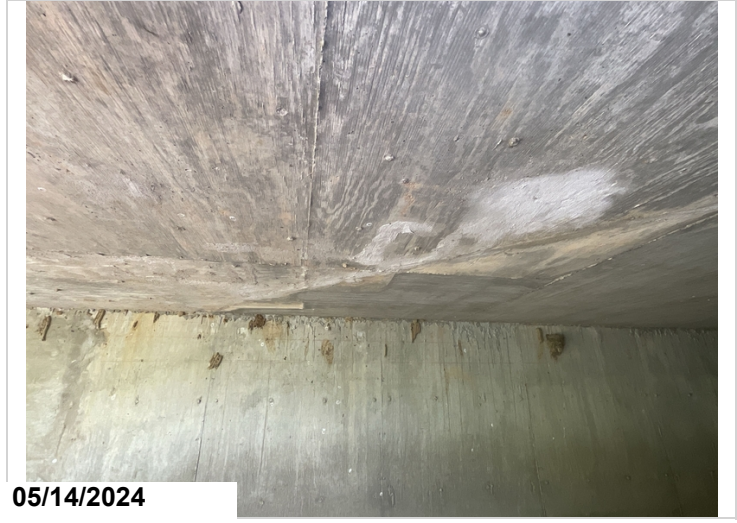
Barrel 1, Top slab, Grouted repairs appear to be functioning as intended.
