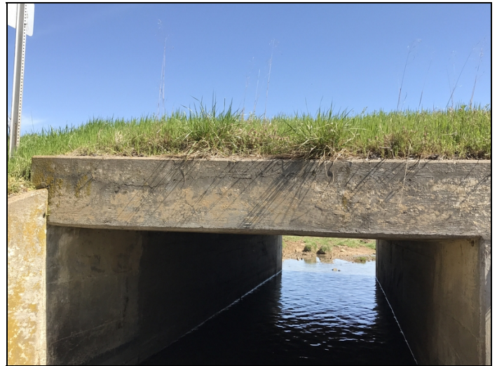
Horizontal cracking. Inlet end of Barrel # 1 headwall.
