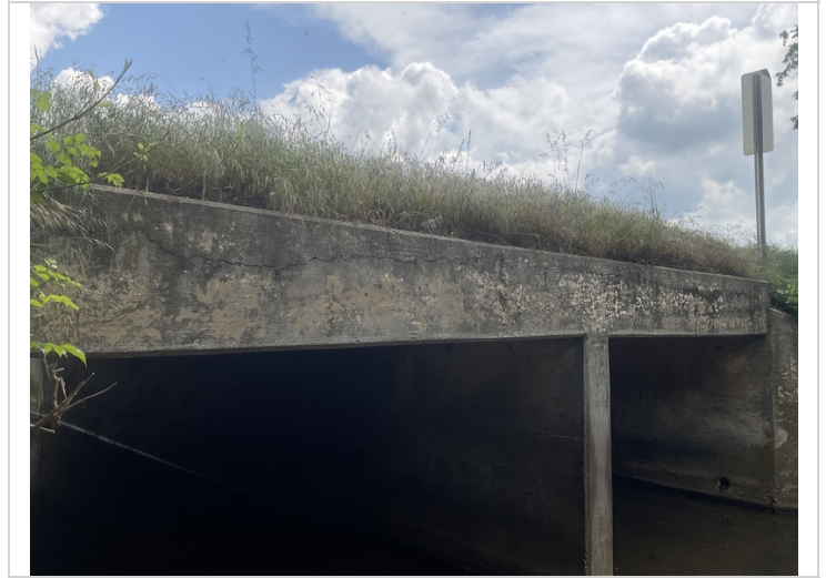
Right head wall horizontal wide cracking.
