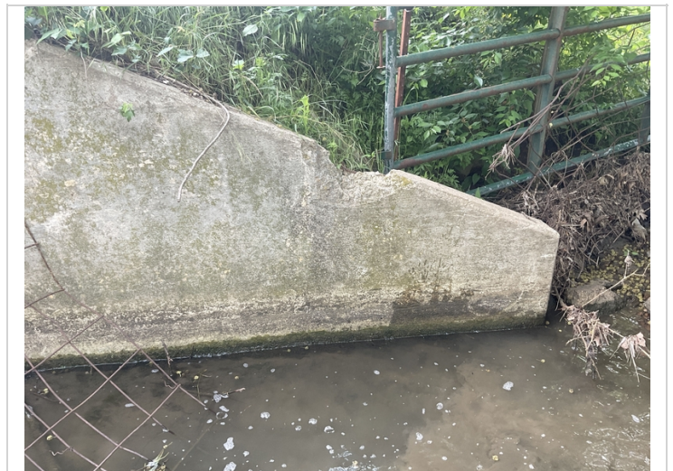
Barrel # 2 Rt wing wall spalling with exposed reinforcing steel.
