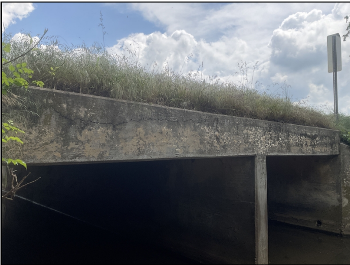
Right head wall with wide horizontal cracking.
