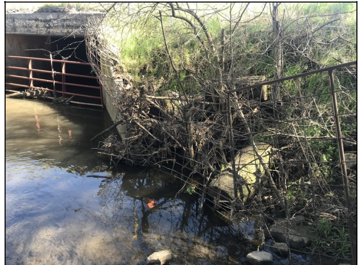
The upstream channel has streambed material accumulation that is directing stream flow into the Southeast wing wall causing minor erosion behind the wing wall.
