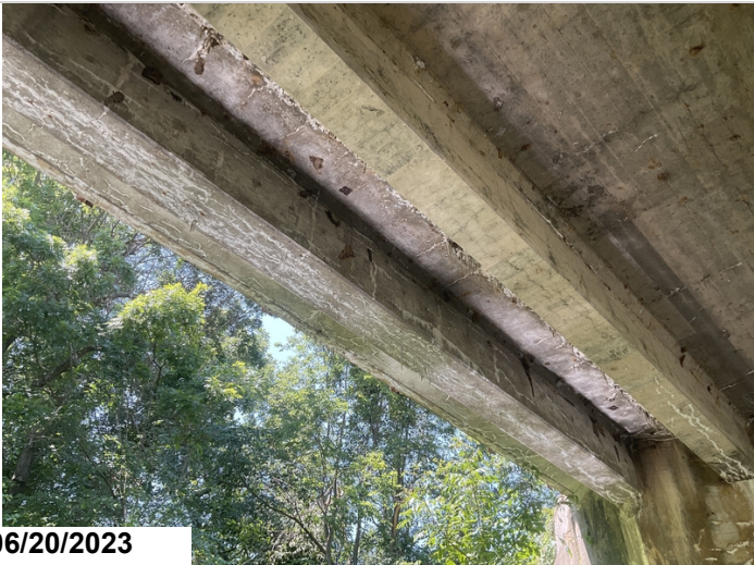
Span # 1 girders # 4 & 5 cracking with efflorescence buildup.
