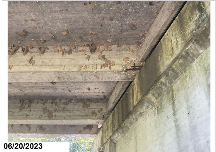
Span # 2 girders # 3 & 4 spalling with exposed reinforcing steel.
