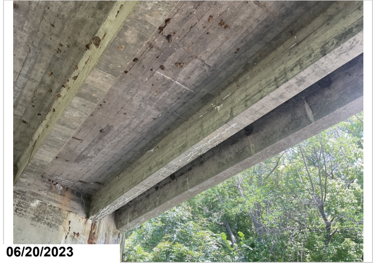
Span # 1 girders # 1 & 2 cracking with efflorescence buildup.
