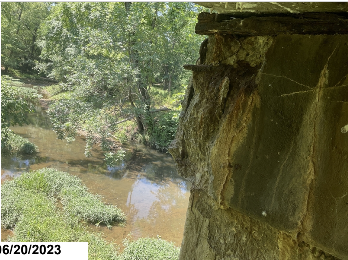
Bent # 3 cap Rt ahead face has concrete deterioration with spalling with exposed reinforcing steel that has caused approximately 2" of bearing area loss to girder # 5 of span # 3. The delaminated areas extend under the bearing device.
