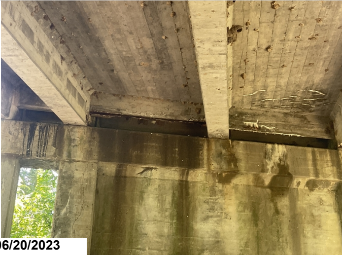
Span # 2 bay # 2 spalling with exposed reinforcing steel in the expansion dam.
