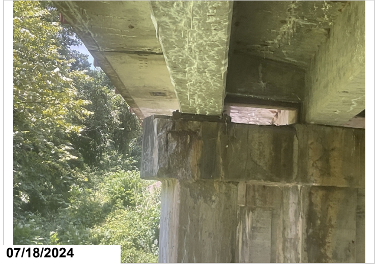
Bent 3. Ahead face, Right side of cap has concrete deterioration.
