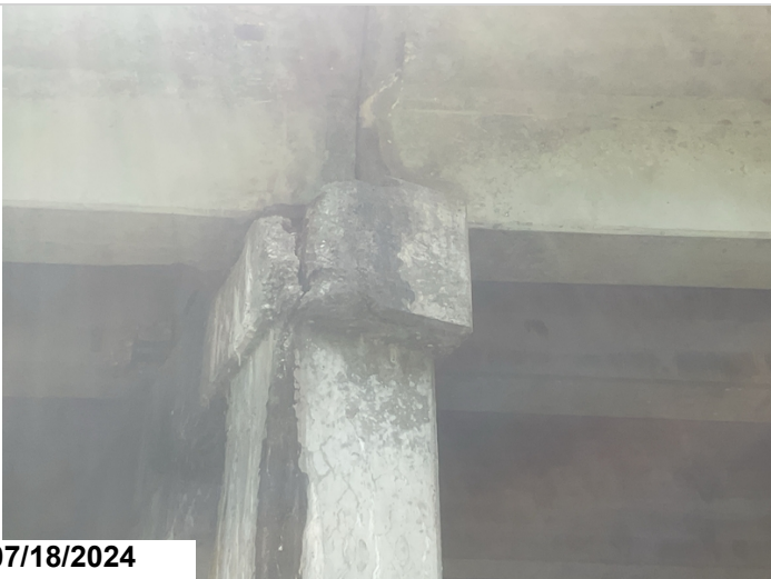
Bent 3. Left side of cap has concrete deterioration.
