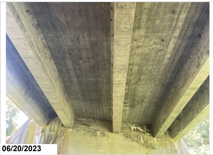
Span 3 typical undersurface of the deck.
