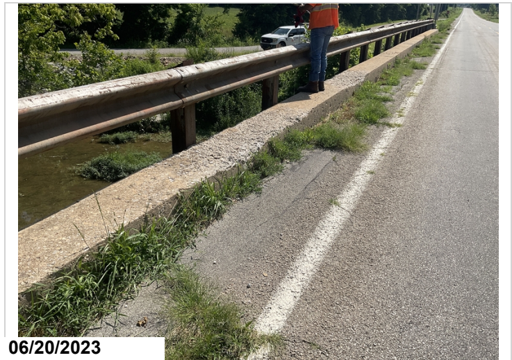
Left curb concrete deterioration.
