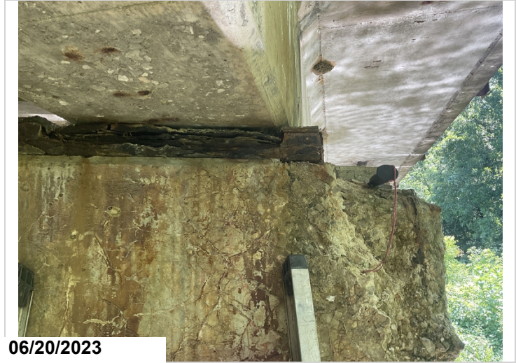
Bent # 2 Rt spalling with exposed reinforcing steel and loss of bearing area.
