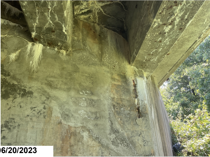
Abutment # 2 Rt spalling with exposed reinforcing steel.
