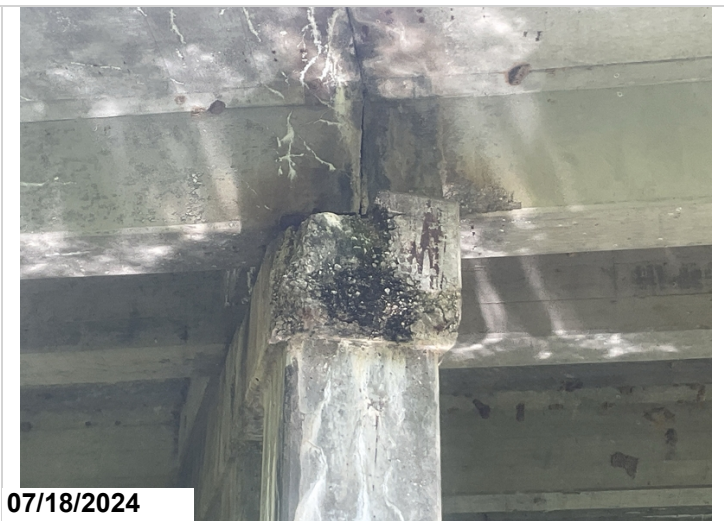
Bent 2 cap. Right end. Concrete deterioration.
