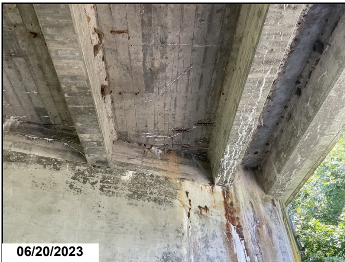
Span 1 bay 2 spalling with exposed reinforcing steel.
