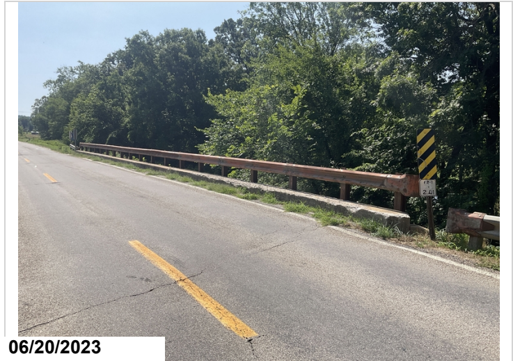
Right bridge rail failing paint system.
