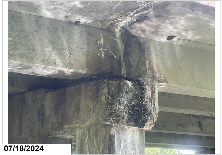
Bent 2 cap. Right end. Concrete deterioration.
