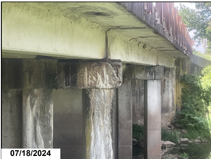
Bent 3 cap, Ahead face, Left end has concrete deterioration with loss of bearing area.
