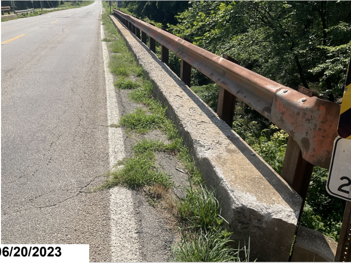
Right curb concrete deterioration.
