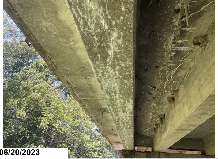
Span # 3 Girder # 5 cracking with efflorescence buildup.
