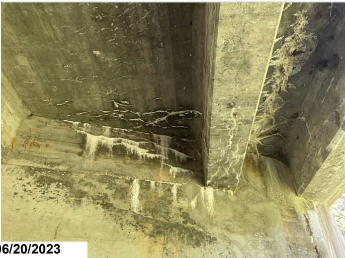
Span # 3 undersurface cracking with efflorescence buildup.
