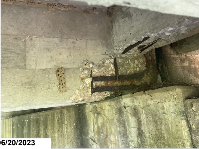
Span # 3 Bent # 3 Girder # 2 spalling with exposed reinforcing steel.
