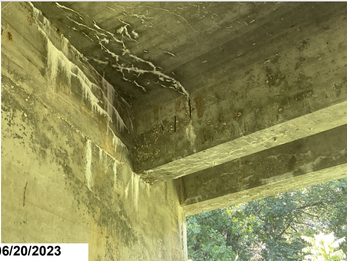
Abutment # 2 Girder # 4 spalling with exposed reinforcing steel.
