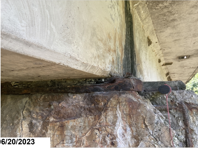
Bent # 3 Girder # 1 bearing with active corrosion and pack rust.
