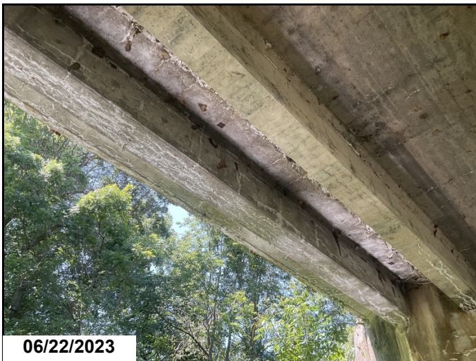
Span 1 girders 4 & 5 cracking with efflorescence buildup.
