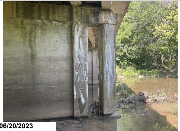
Bent # 3 columns # 1 & 2 cracking with efflorescence buildup.
