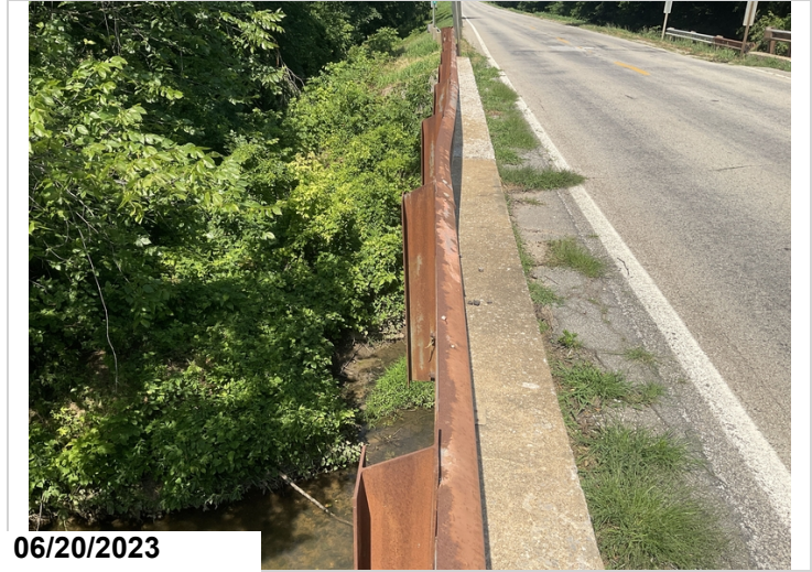
Span # 2 Rt collision damage.
