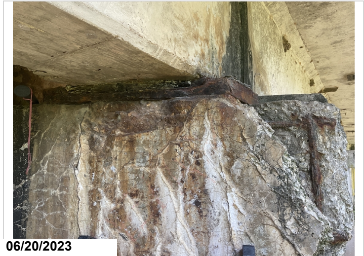
Bent # 3 Lt concrete delamination with bearing area loss under girder # 1.
