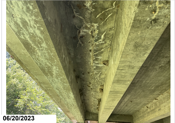
Span # 3 bay # 4 efflorescence buildup.
