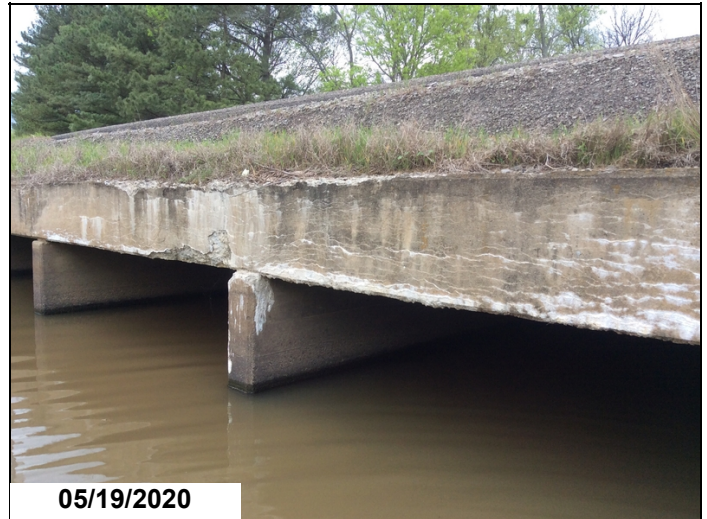
05/19/2020 The Left headwall and vertical face of top slab has soft and deteriorating concrete over Barrels # 1 and 2 with mapcracking and efflorescence. The concrete is beginning to spall along the undersurface edges.
