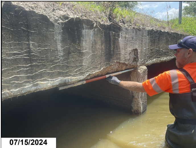
07/15/2024 Barrels # 1 and 2 Top Slab, Left Exterior Edge: Undersurface has a 3' spalled area and concrete deterioration with efflorescence along the Left exterior edge. 1LF Spalling CS3
