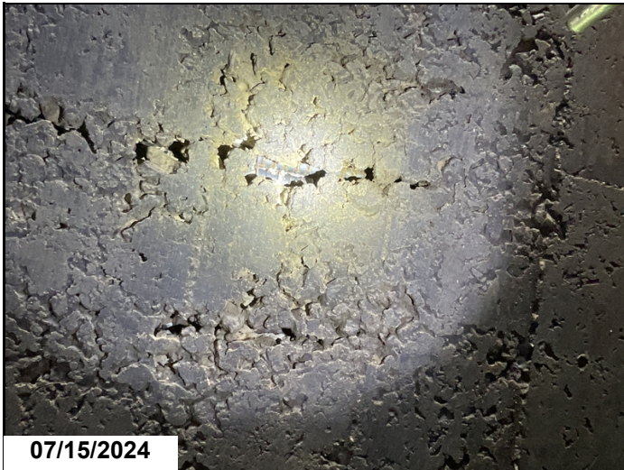
Top Slab Undersurface: Areas of honeycombing that exposes reinforcing steel from the construction process. 1LF Exposed Steel CS2
