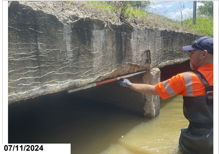
Barrels # 1 and 2 Top Slab, Left Exterior Edge: Undersurface has a 3' spalled area and concrete deterioration with efflorescence along the Left exterior edge. 1LF Spalling CS3
