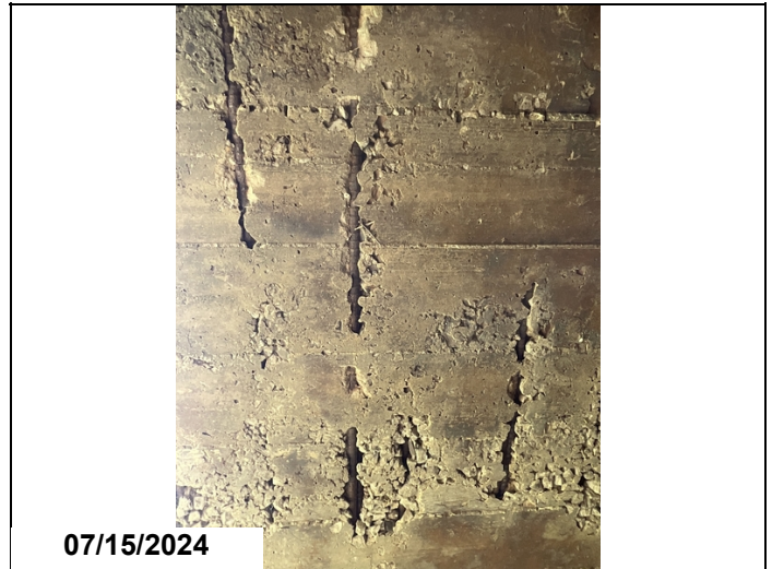
Top Slab Undersurface: Areas of honeycombing from the construction process that exposes reinforcing steel. The most extensive area with honeycombing is in Barrel # 2 at the inlet end of structure. Exposed steel 2LF CS3.
