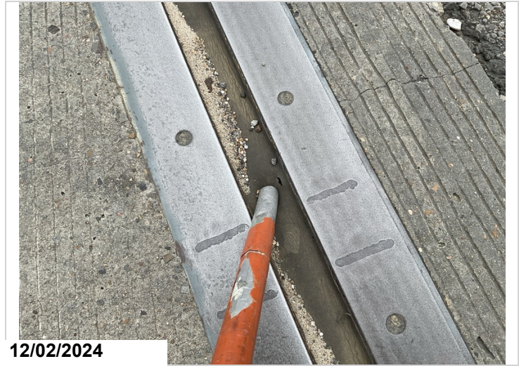
Few isolated areas of tears/ rips in the sealant allowing water to leak onto the substructure and superstructure.
