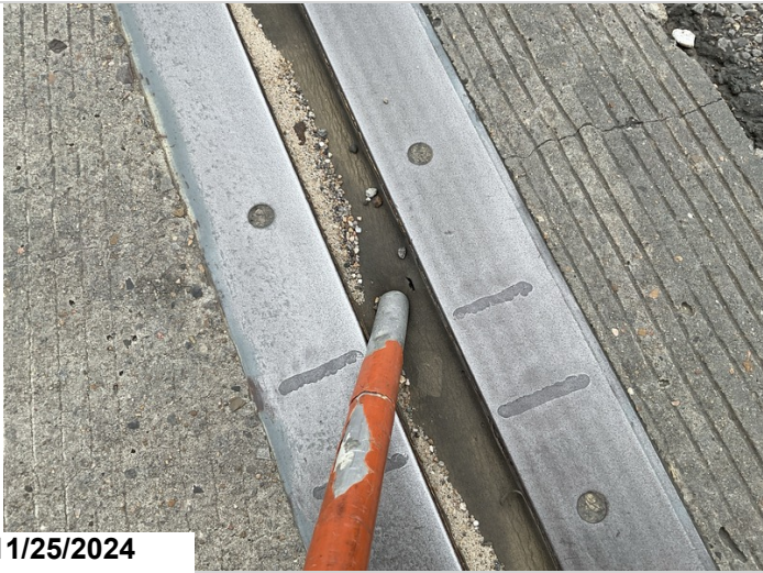
Abutment # 2 Expansion Joint, Right Lane: Full depth rip/puncture. 1LF CS4.
