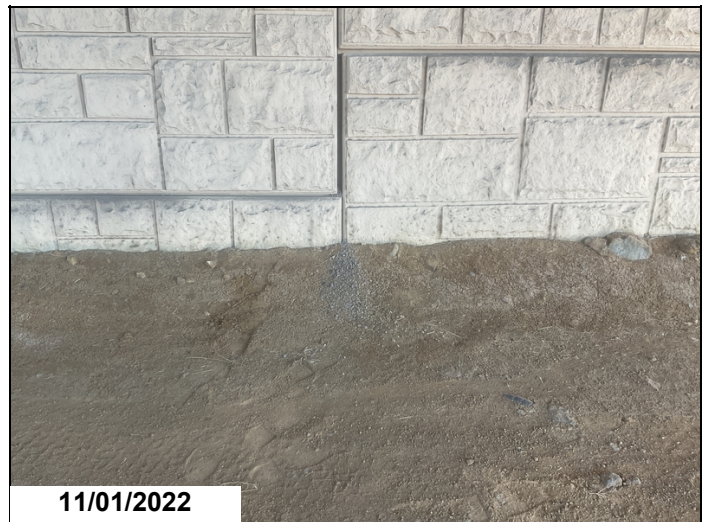
North MSE wall under Beam # 6 has minor leakage of granular fill visible at the base of the wall.
