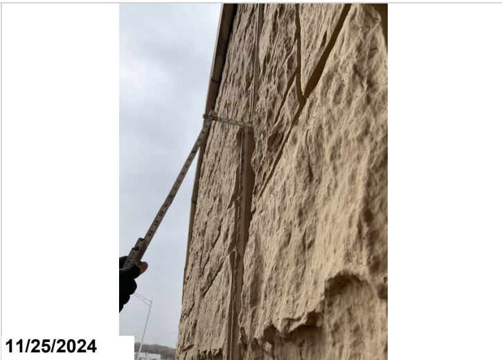
Abutment # 1 MSE wall still appears misaligned and bulging.
