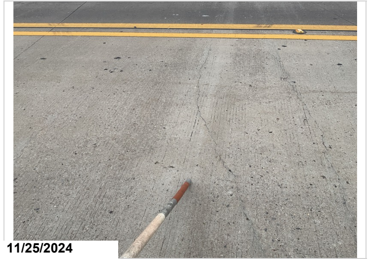
Span # 2, Over Bent # 2: Transverse crack.
