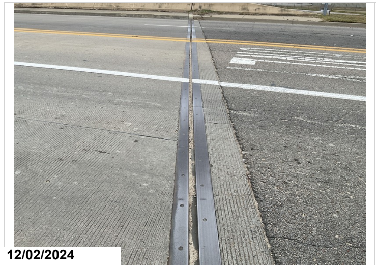
Abutment # 2 Expansion Joint: Dirt and debris in assembly.
