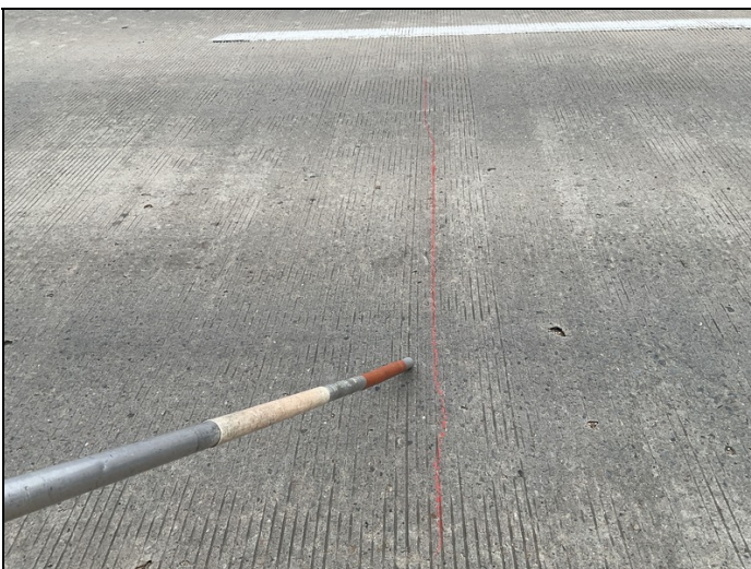
Span # 1, Right Lane: Transverse cracks.
