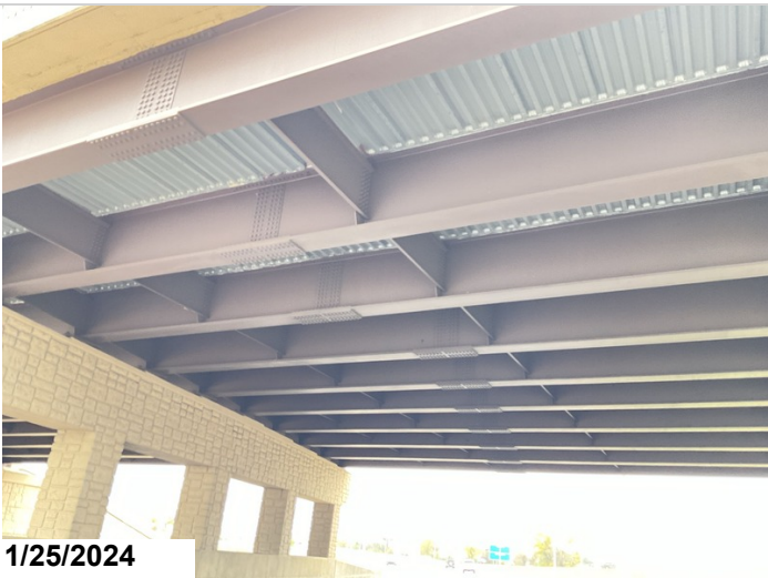
Span # 2 splice connections. General view.
