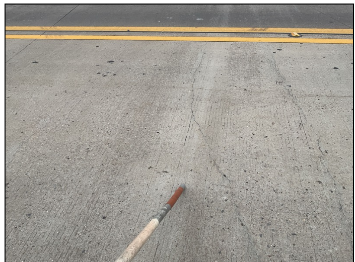
Span # 2, Over Bent # 2: Transverse crack.
