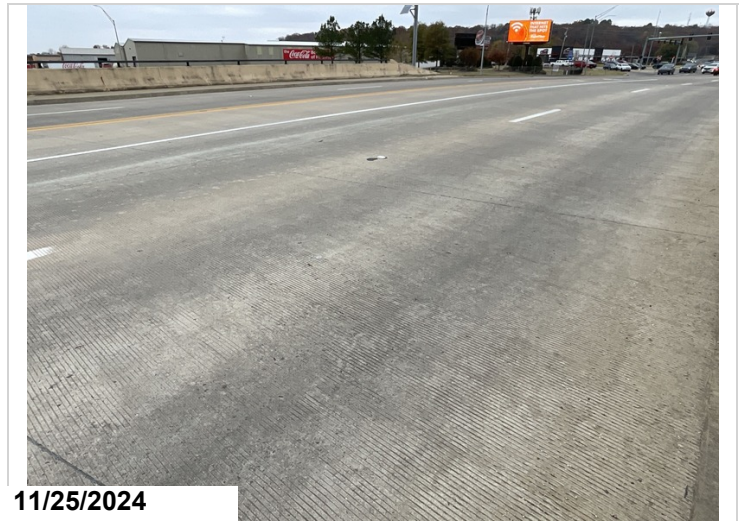
The driving surface of the deck has sealable cracking and appears to be a good candidate for a polymer wearing surface based on the condition of the deck at time of inspection.
