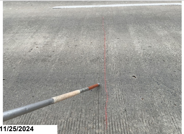
Span # 1, Right Lane: Transverse cracks.
