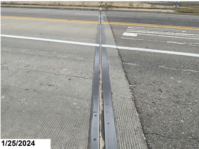
Abutment # 2 Expansion Joint: Dirt and debris in assembly.
