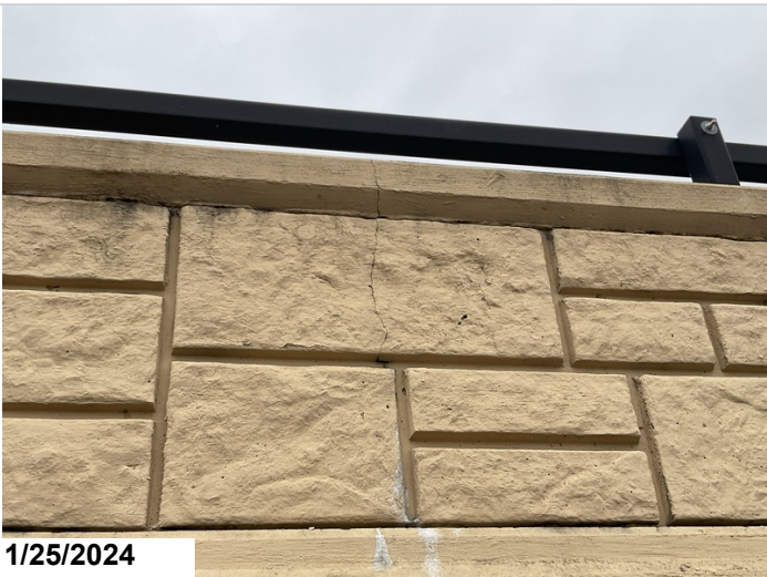
Span # 2, Left Railing: Vertical crack. 1LF CS2.
