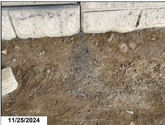
North MSE wall under Girder # 6 has minor leakage of granular fill visible at the base of the wall.
