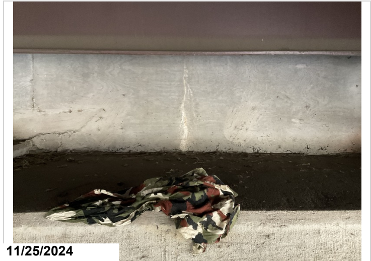
Abutment # 1 Backwall, Bay # 2: Verticrack with efflorescence. 1LF CS2.
