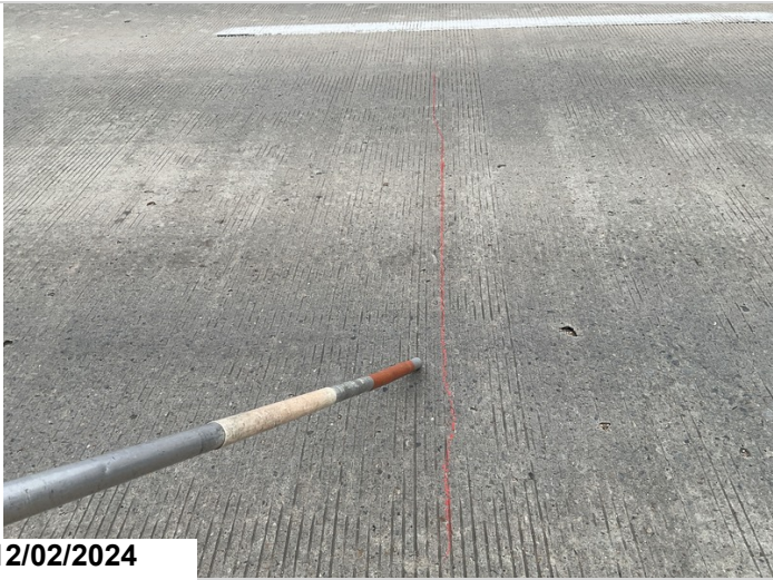
Span # 1, Right Lane: Transverse cracks.
