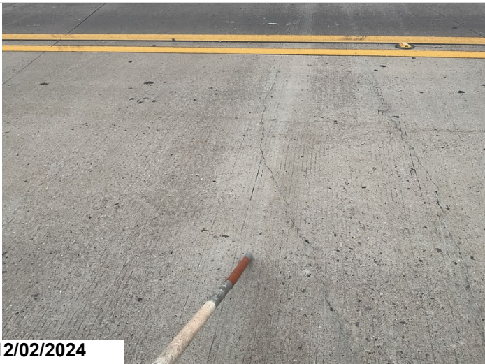
Span # 2, Over Bent # 2: Transverse crack.
