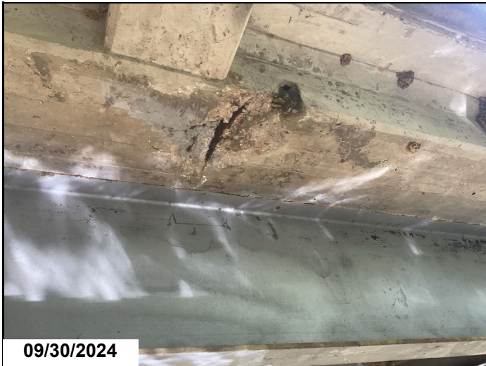
Left Deck Overhang, 8' From Abutment # 2: 16" spall with exposed reinforcing steel. 2SF CS3.
