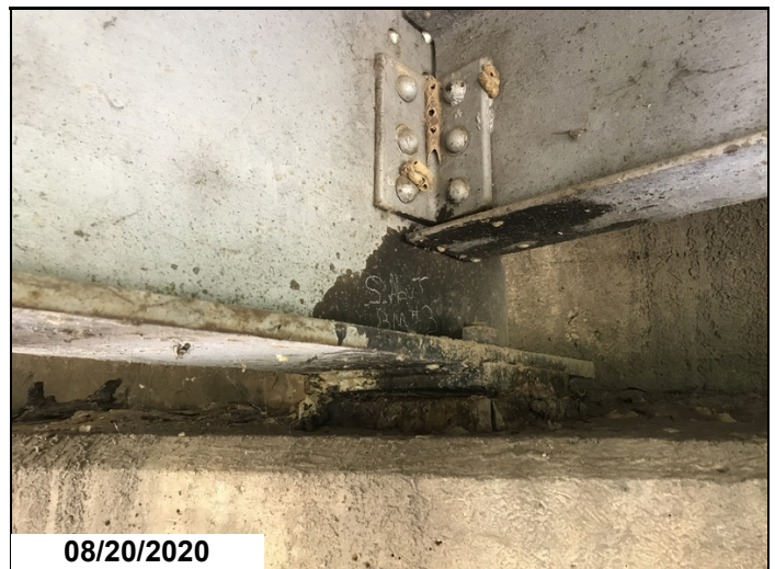
Abutment # 1 bearing #2 active corrosion.
