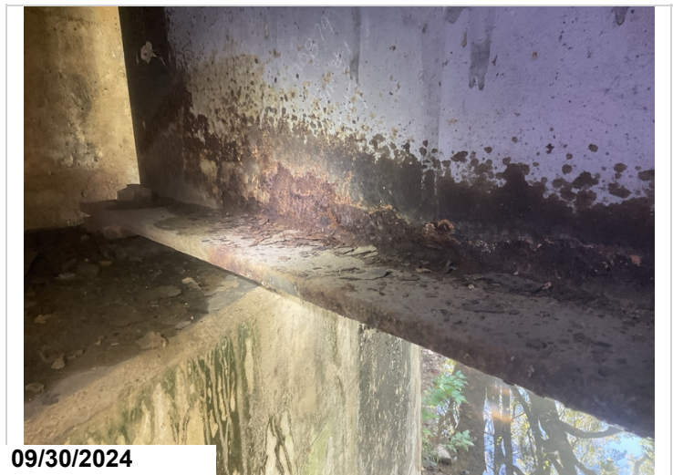
Girder # 1, Abutment # 1: Corrosion with flaking rust. 5LF CS3.
