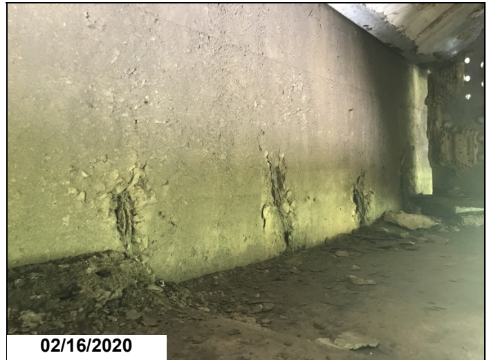
Spalling in abutment # 2 backwall. Photo between girders # 2 and # 3.
