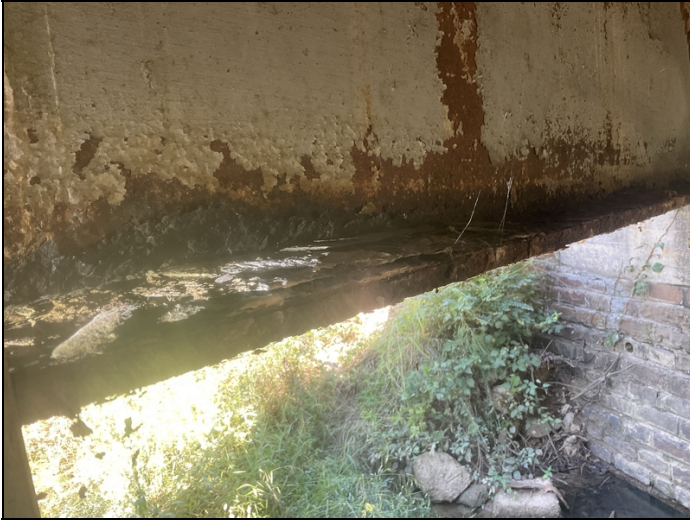
Right exterior girder: Corrosion with flaking rust / section loss.
