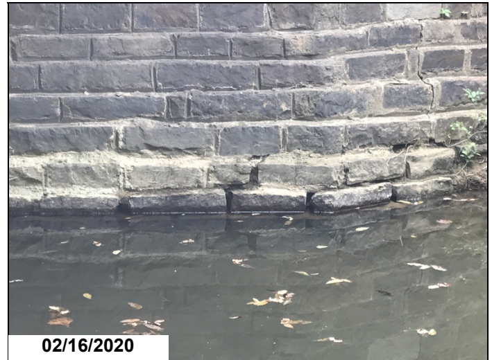
Abutment #1-Grout deterioration between stones.
