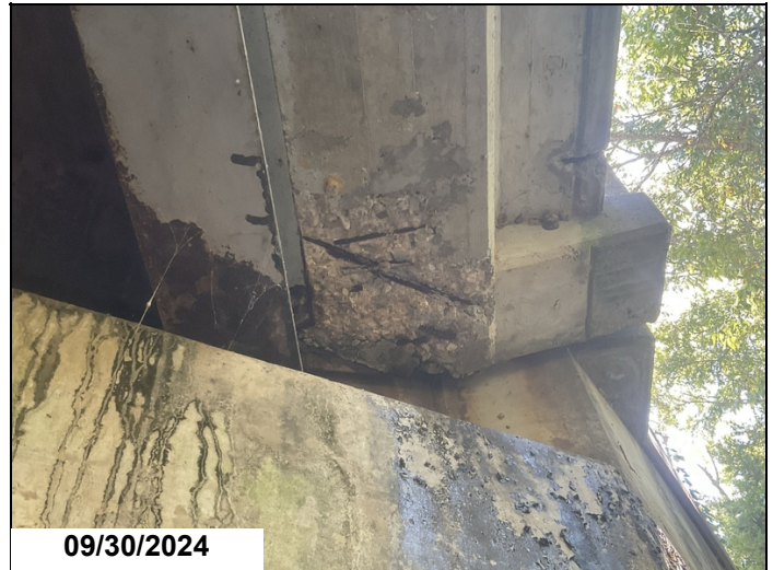
Left Deck Overhang, At Abutment # 1: 4SF CS3.
