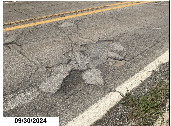
Left Lane: Potholes in asphalt driving surface.
