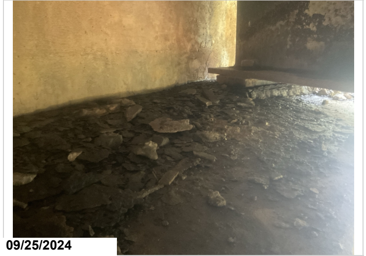
Abutment # 1: Dirt and debris accumulation in bearing area.
