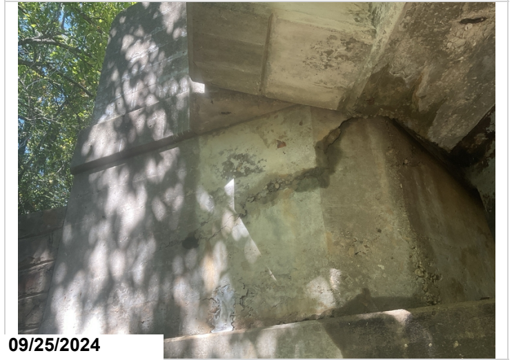
Abutment # 2 Backwall, Left Side: Fractured under the end post from apparent traffic impact. 4LF CS3.
