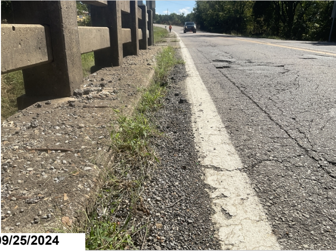
Gutters have heavy dirt and debris accumulation that restricts the deck drains.
