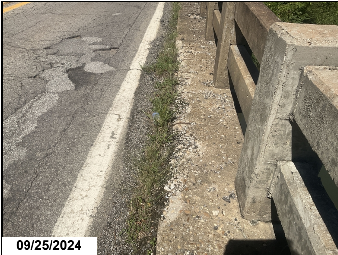
Right Curb: Areas of soft and deteriorating concrete with exposed reinforcing steel throughout. 22LF CS3.
