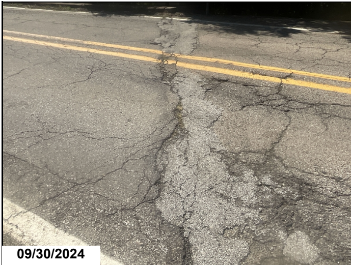
Asphalt breaking apart over abutment # 2.
