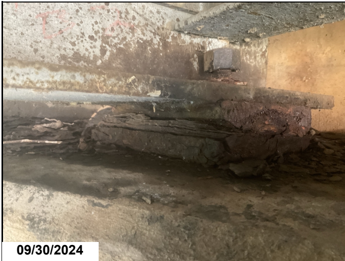
Abutment # 2: Bearing # 2: Corrosion with flaking rust / section loss. 1EA CS3.
