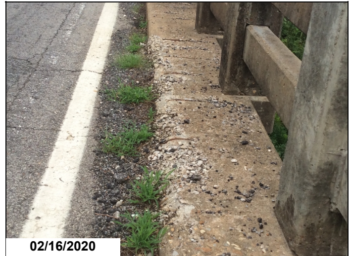
Right curb-Concrete deterioration with spalling that exposes reinforcing steel.
