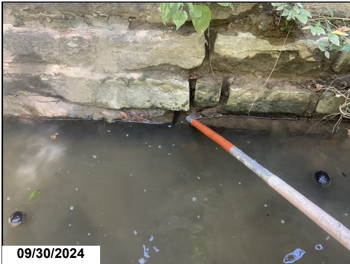
Abutment # 1: Grout deterioration at the water elevation. 23LF CS3.
