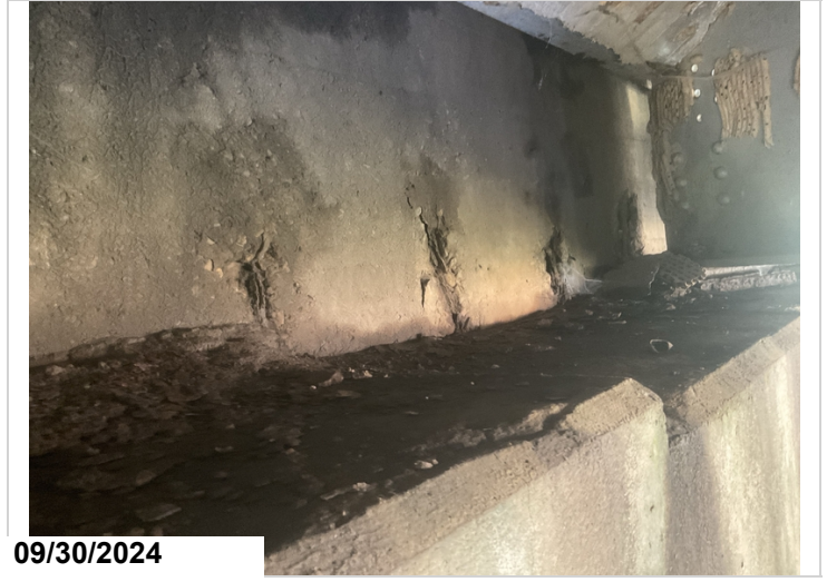
Abutment # 2 Backwall: Spalls with exposed reinforcing steel. 8LF CS3.
