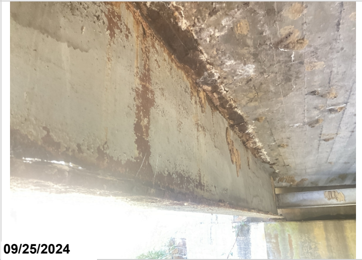
Right exterior girder: Corrosion with flaking rust / section loss.
