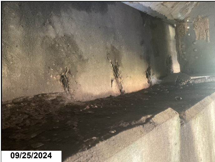
Abutment # 2 Backwall: Spalls with exposed reinforcing steel. 8LF CS3.
