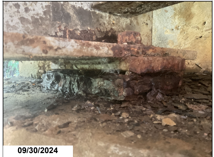
Abutment # 2: Bearing # 1: Corrosion with flaking rust / section loss. 1EA CS3.
