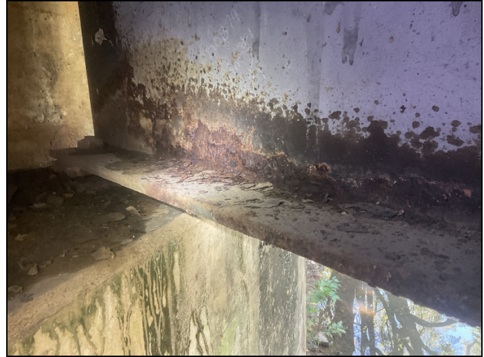
Girder # 1, Abutment # 1: Corrosion with flaking rust. 5LF CS3.
