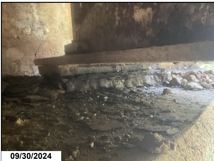
Abutment # 1, Bearing # 1: Corrosion with flaking rust / section loss. 1EA CS3.
