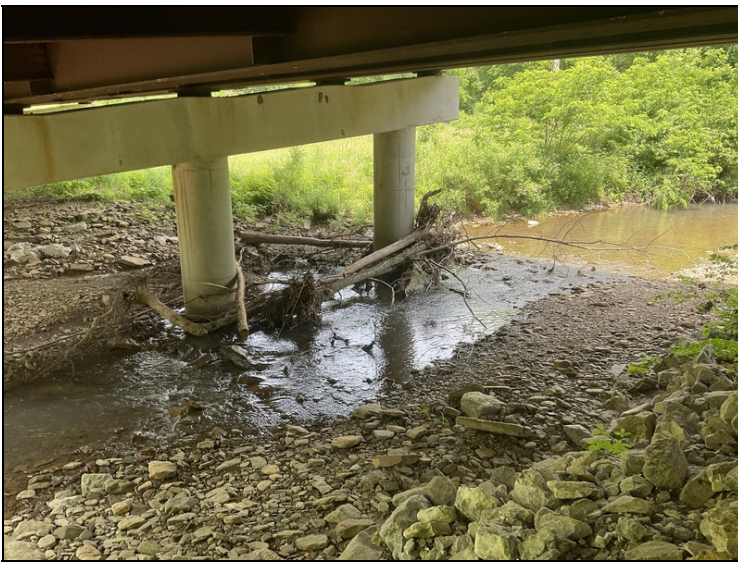
Bent #2 light drift accumulation.
