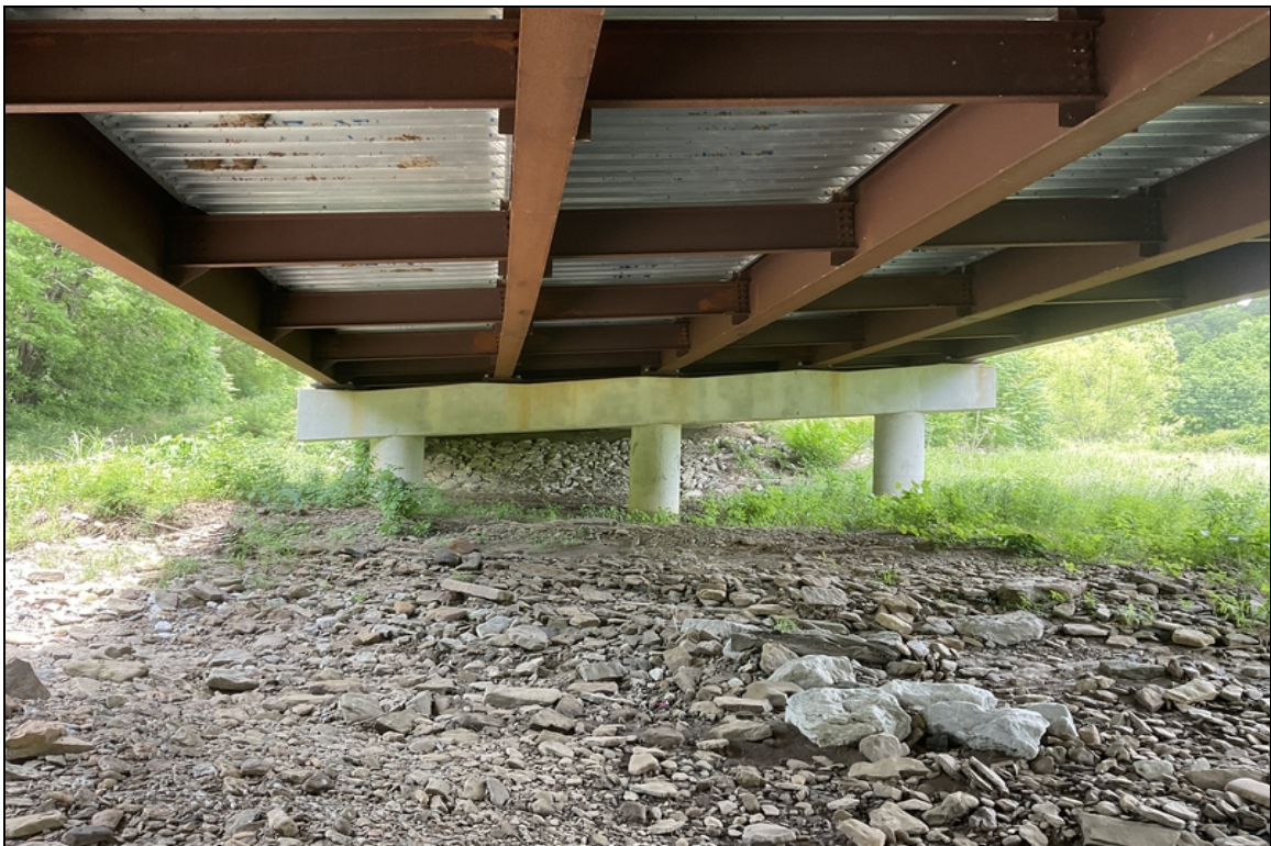
Intermediate bent typical.
