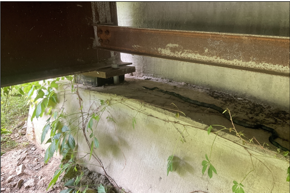
Abutment #1 typical bearings.
