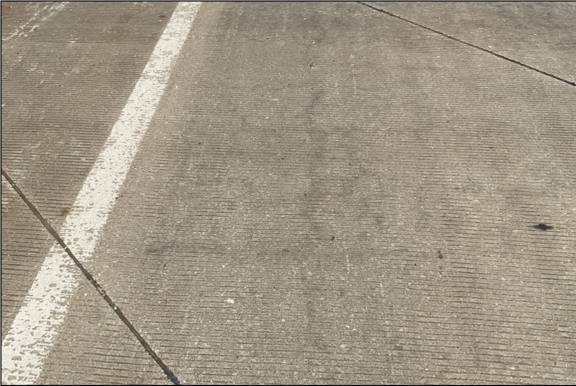
Sealable deck cracking.
