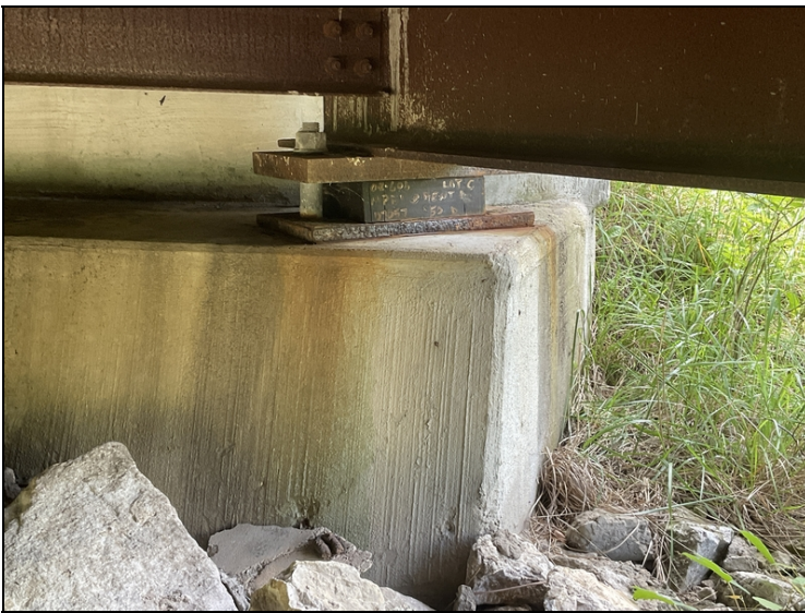
Abutment #1 bearing #1 active corrosion with pack rust.
