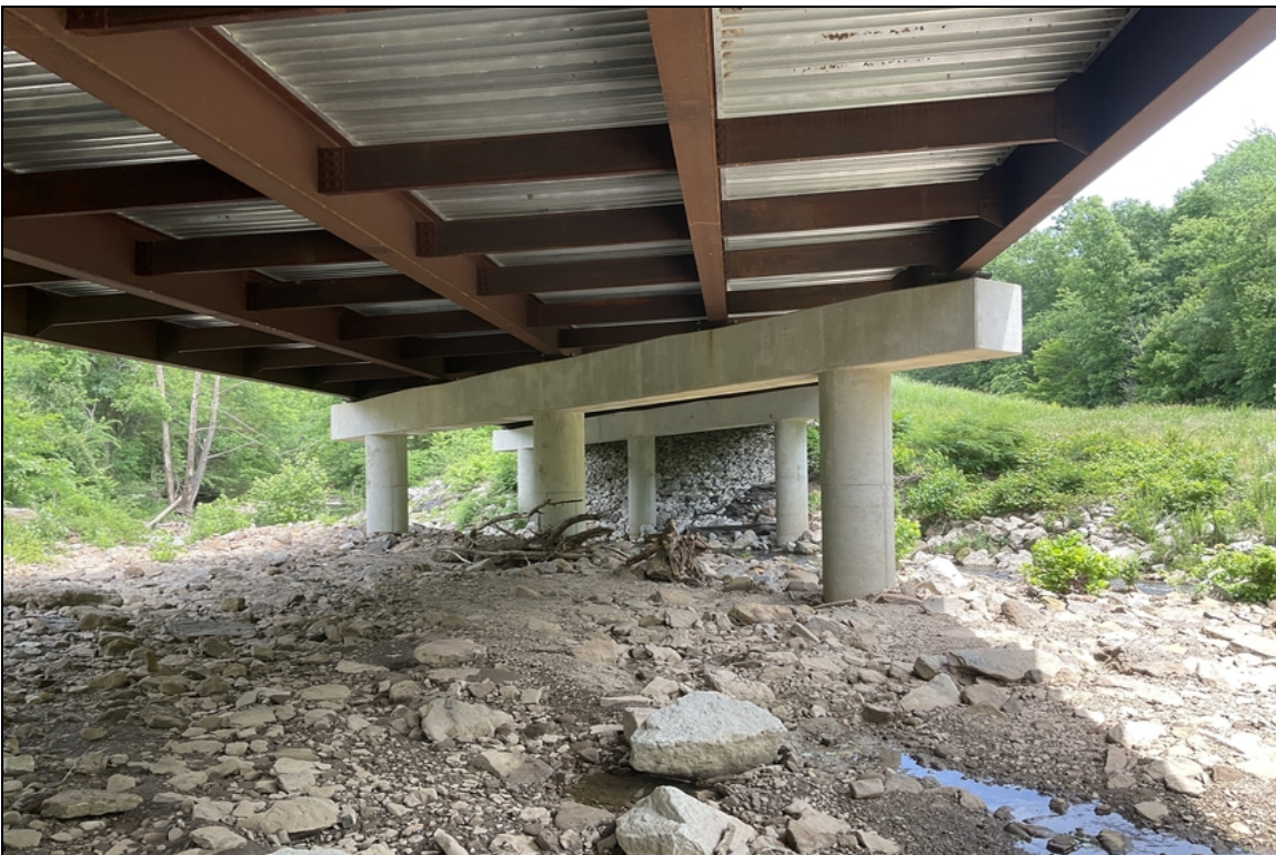
Typical intermediate bent.
