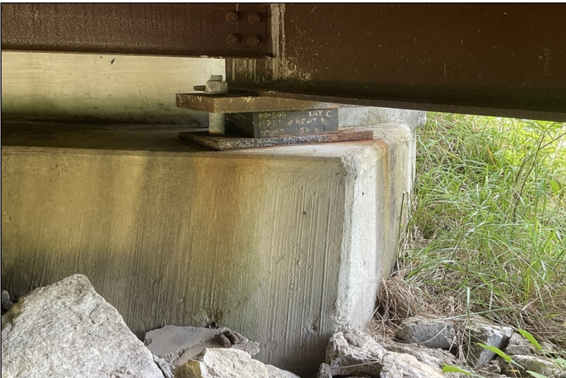
Abutment #1 bearing #1 active corrosion with pack rust.
