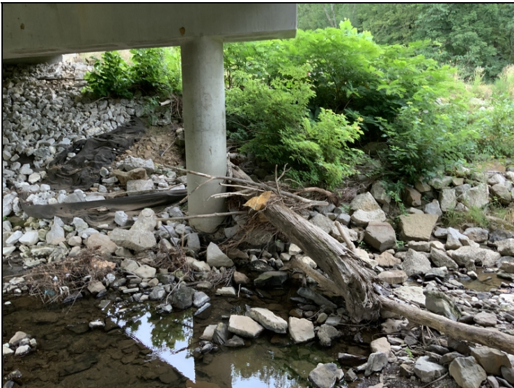
Bent 4 Column 3 Large drift
