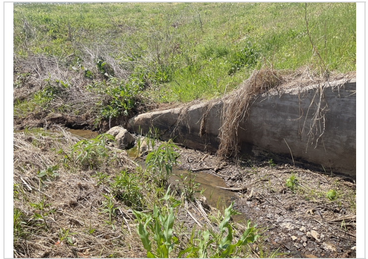
Barrel # 1 Rt fractured wing wall.
