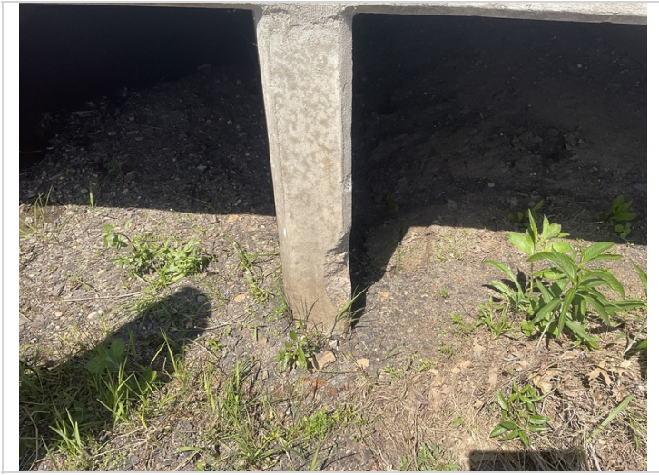
Wall # 2 Rt spalling.
