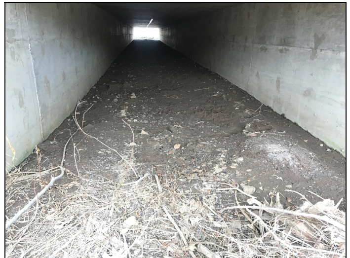
The interior of culvert barrels have up to 30" of silt accumulation.
