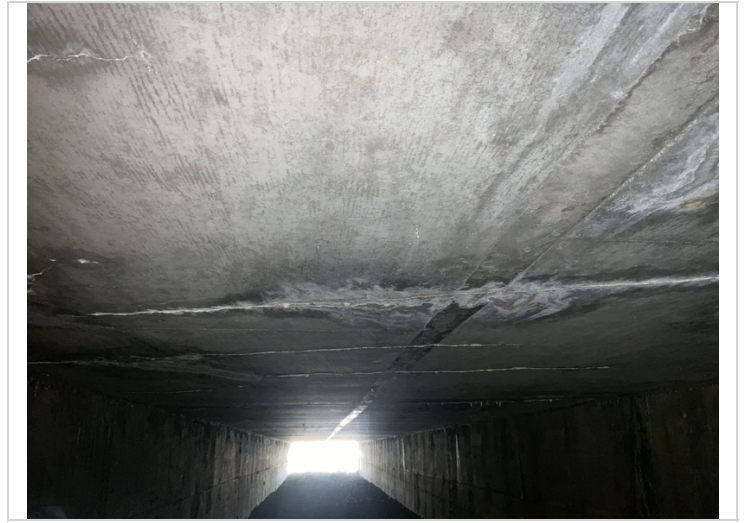
Barrel # 4 top slab cracking with efflorescence buildup.
