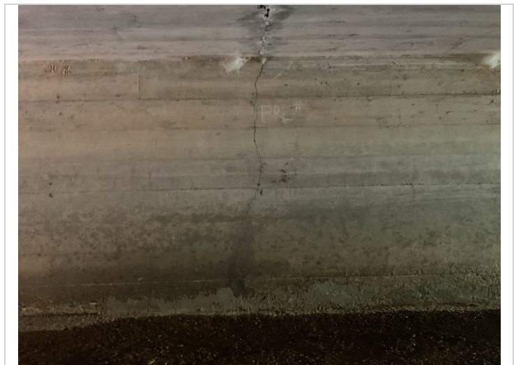
Barrel # 2 wide cracking near the centerline.
