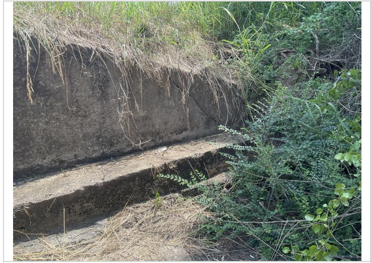
Barrel # 1 Lt end of the Southwest wing wall has a wide diagonal crack.
