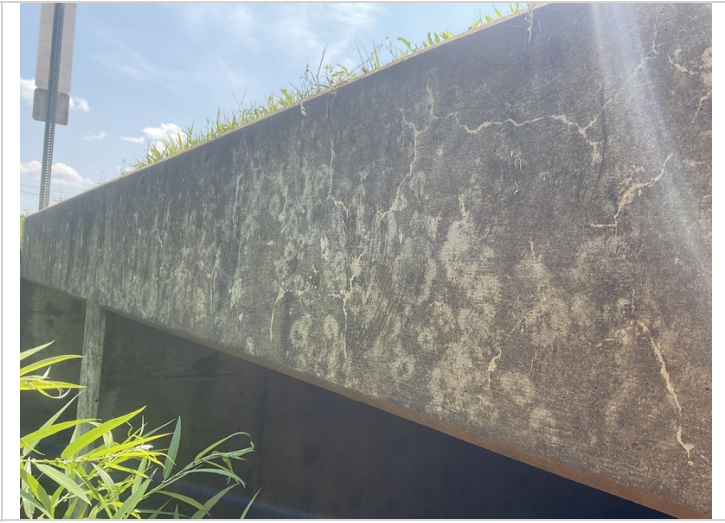
Right head wall map cracking with light staining.
