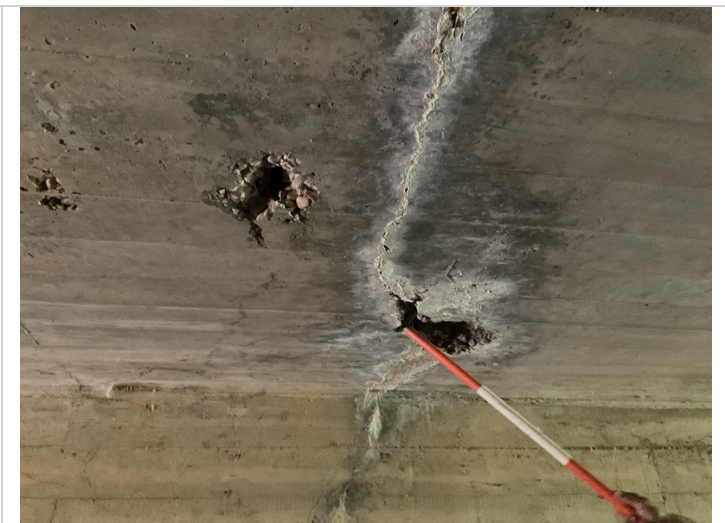
Barrel # 1 top slab has a 2' area and an 8" area with concrete deterioration/spalling with exposed reinforcing steel. Exposed reinforcing steel has active corrosion and measures 5/8" remaining section at this inspection. Concrete section loss up to 4" deep in the larger area of deterioration.
