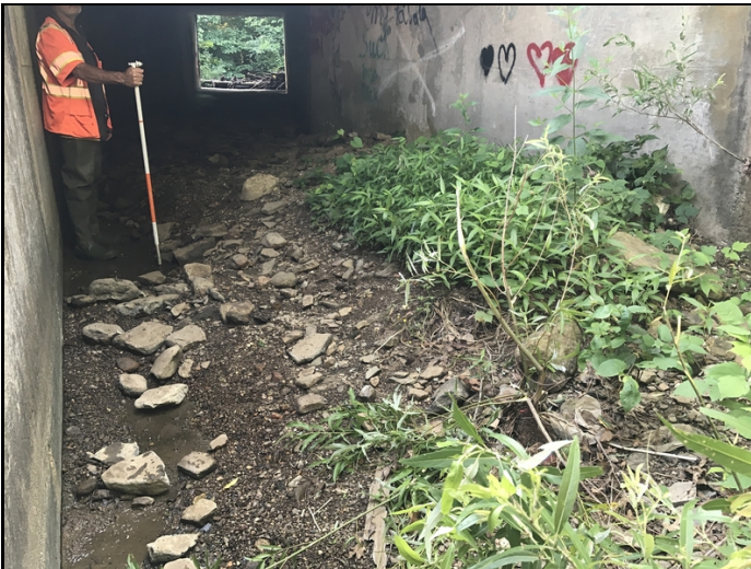
The interior of Barrel # 2 has up to 24" of streambed material in the left side near outlet end.
