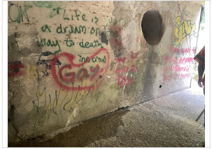
Barrel # 2 Rt diagonal cracking with efflorescence buildup.
