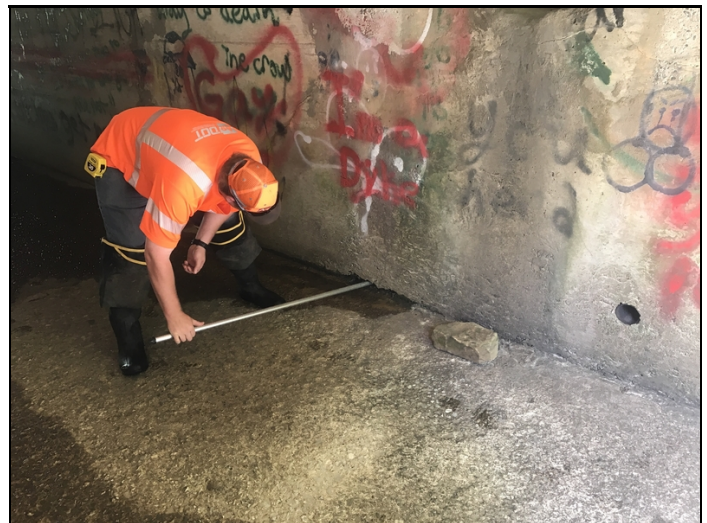
North wall of Barrel # 2. Concrete deterioration.
