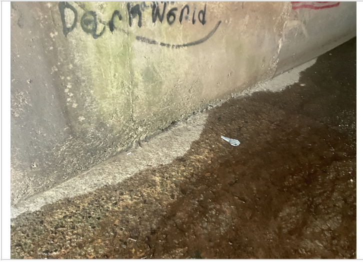
Barrel # 1 Rt concrete deterioration and section loss.
