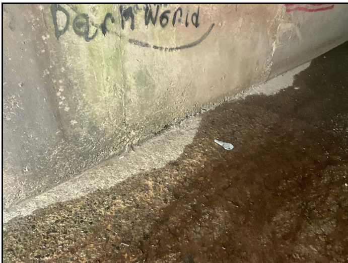
Barrel # 1 Rt concrete deterioration and section loss.
