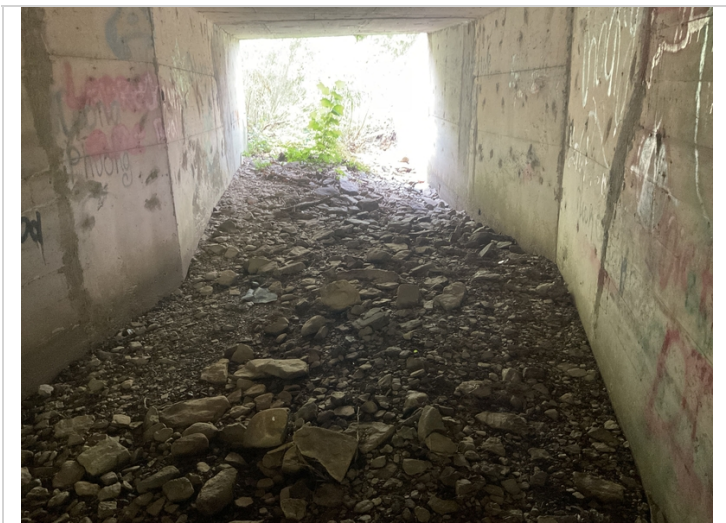
Barrel # 2 Lt stream bed material accumulation.
