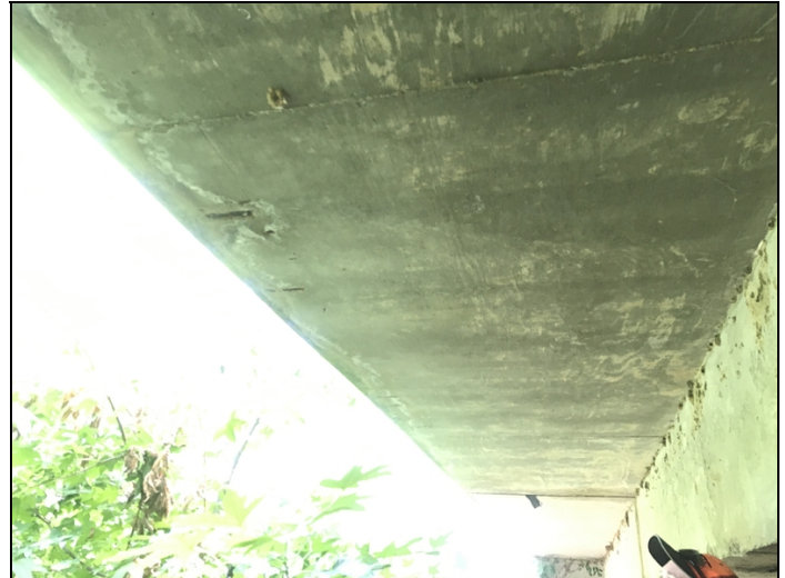
Span # 2. Right overhang. Exposed reinforcing steel.
