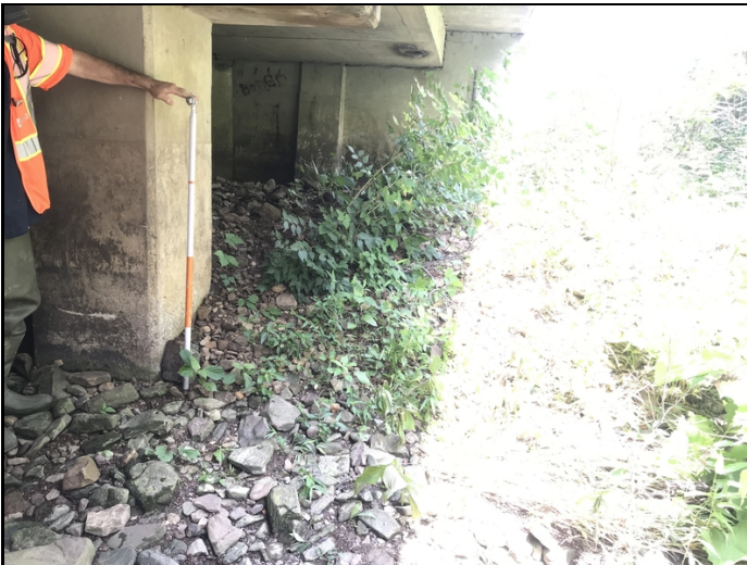
Span # 2 is restricted by approximately 3' of streambed material accumulation.
