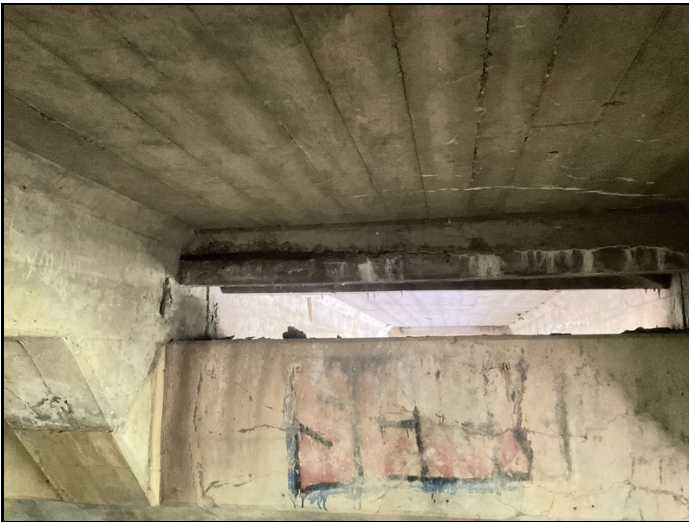
Span # 2 bay # 1 deck haunch over Bent # 2 spalling with exposed reinforcing steel.
