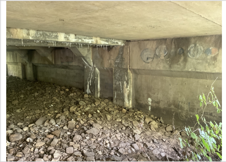
Bent # 2, columns # 2 & 3 have map cracking with efflorescence.
