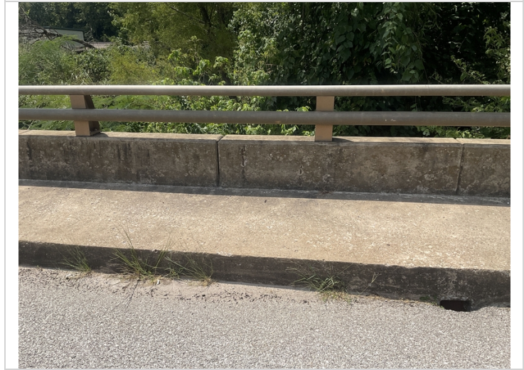
Span # 2 Lt exposed reinforcing steel.
