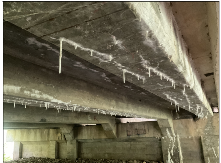
Span # 2 girders # 1 & 2 efflorescence buildup.
