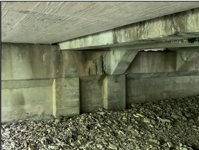
The ahead face of Bent # 2 cap has spalling with exposed reinforcing steel adjacent to girder # 4.
