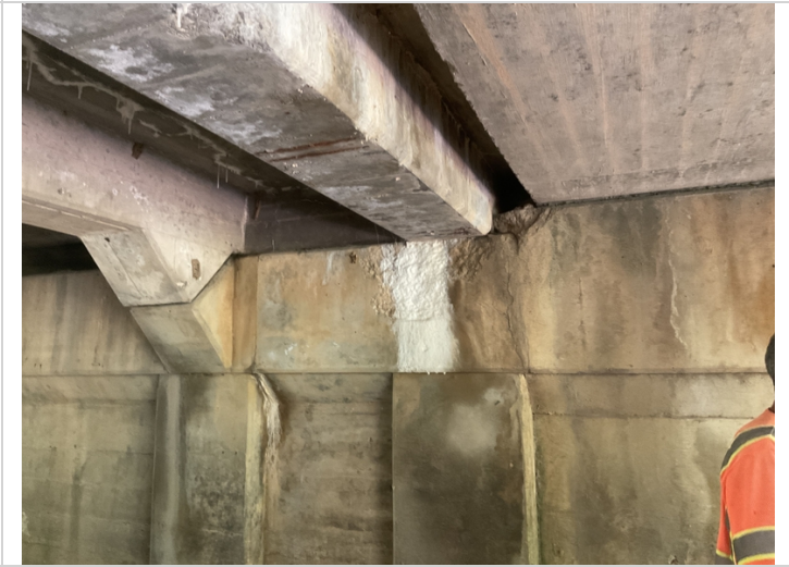
Span # 1 girder # 5 spalling in the bearing area.
