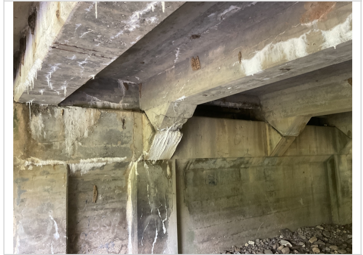
Span # 1 girder # 2 haunch cracking.
