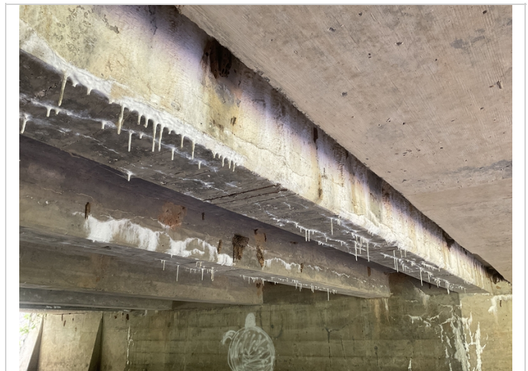
Span # 1 beams # 1 & 2 efflorescence buildup.
