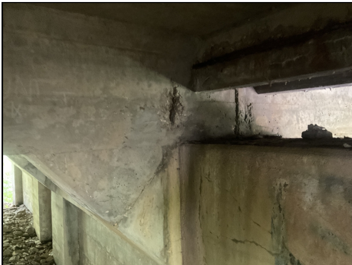
Span # 1 & 2 Girder # 3 spalling with exposed reinforcing steel.
