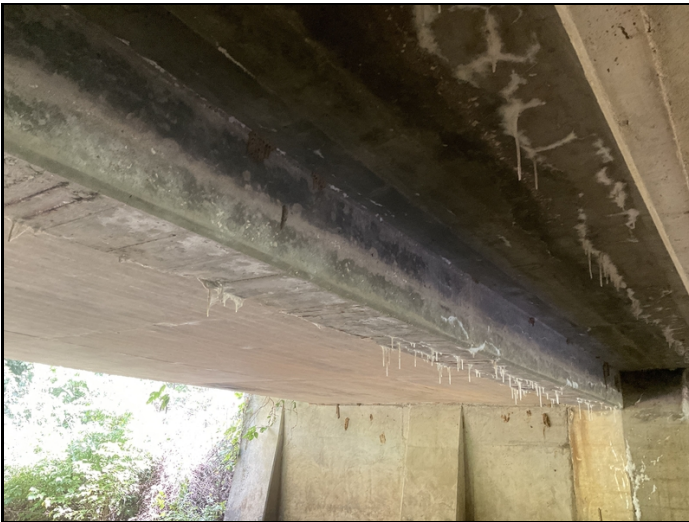
Span # 1 beam # 5 efflorescence buildup.
