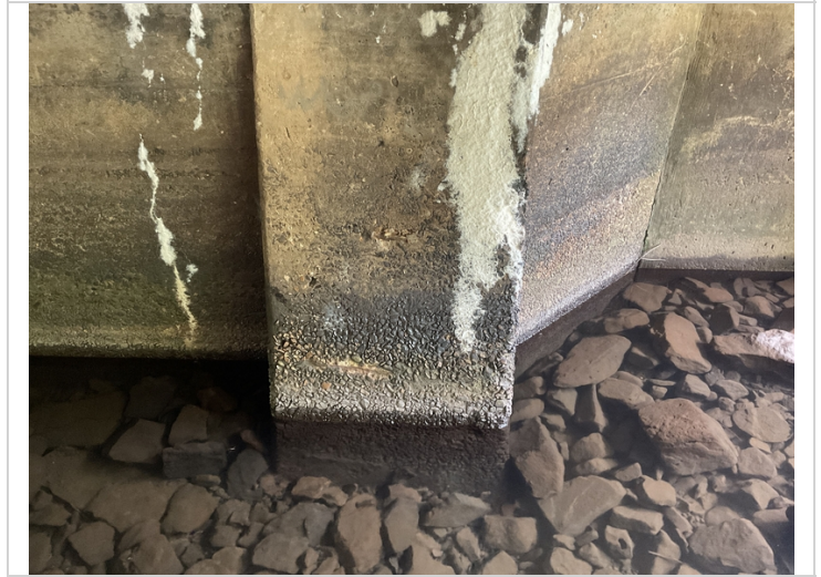
Abutment # 1 column # 3 exposed reinforcing steel.
