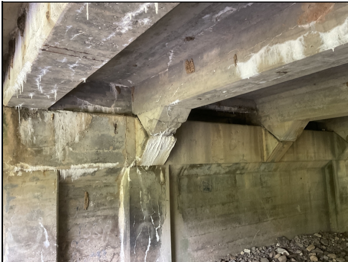
Span # 1 girder # 2 haunch cracking.
