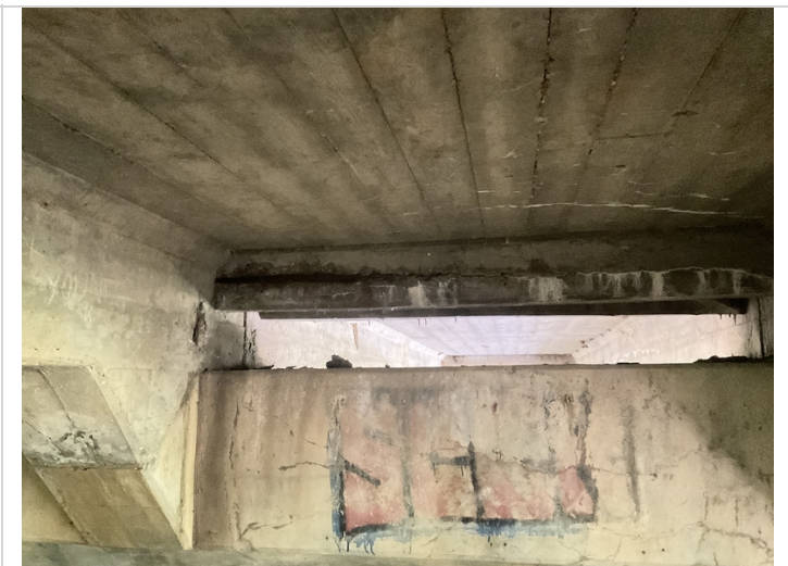
Span # 2 bay # 1 deck haunch over Bent # 2 spalling with exposed reinforcing steel.
