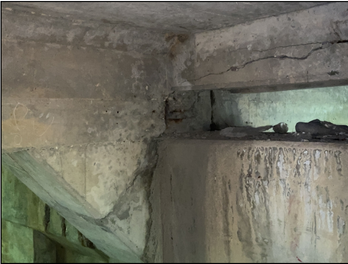
Span # 2 girder # 4 spalling with exposed reinforcing steel over Bent # 2.
