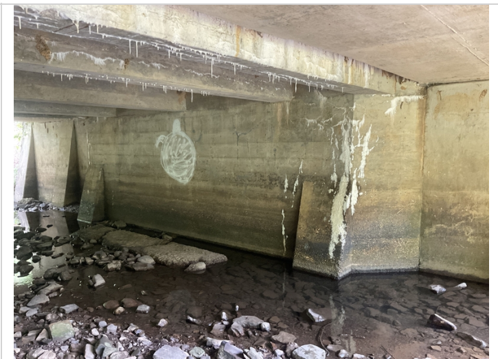
Abutment # 1 cracking with efflorescence buildup.
