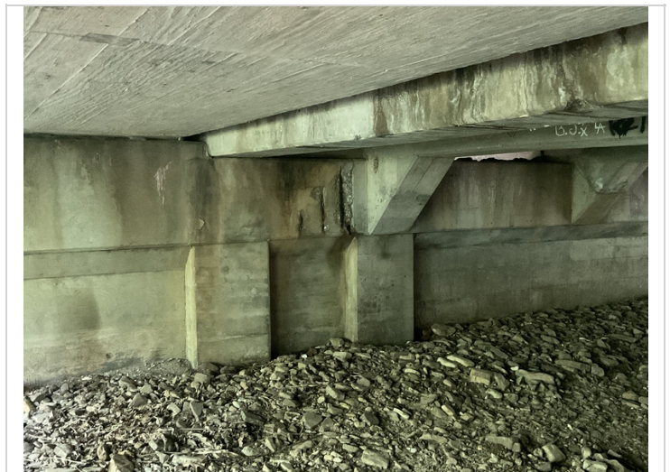
Span # 2 Rt spalling with exposed reinforcing steel.
