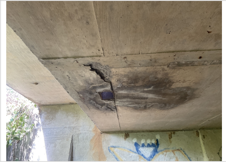
Span # 2 Lt concrete spalling and delaminating adjacent to the deck drains.
