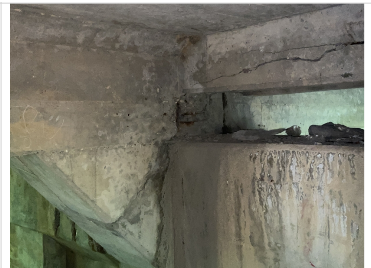
Span # 2 girder # 4 spalling with exposed reinforcing steel over Bent # 2.
