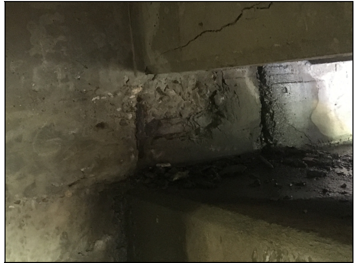
Exposed reinforcing steel in the end of Girder # 4 over Bent # 2.
