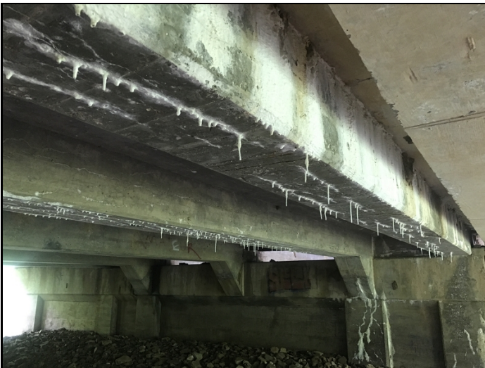
Girders # 1 & 2 in Span # 2-Mapcracking with efflorescence.
