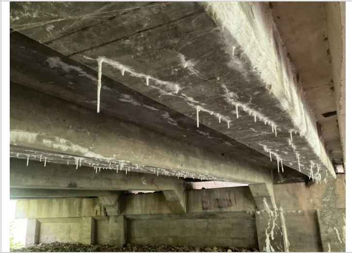
Span # 2 girders # 1 & 2 efflorescence buildup.
