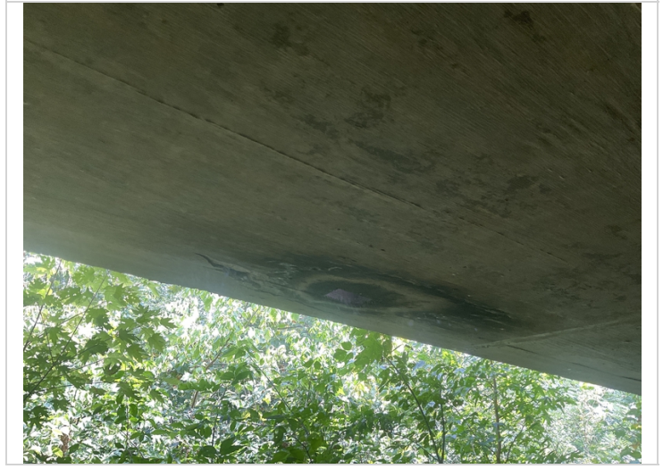
Span # 2 Rt concrete delamination adjacent to the deck drains.
