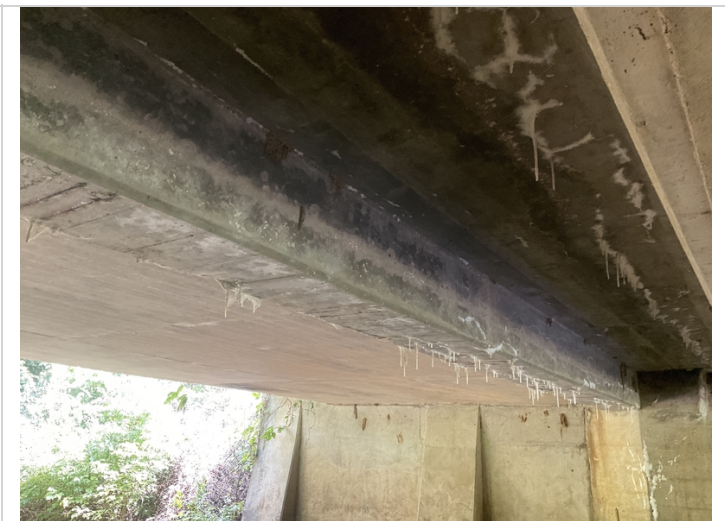
Span # 1 beam # 5 efflorescence buildup.
