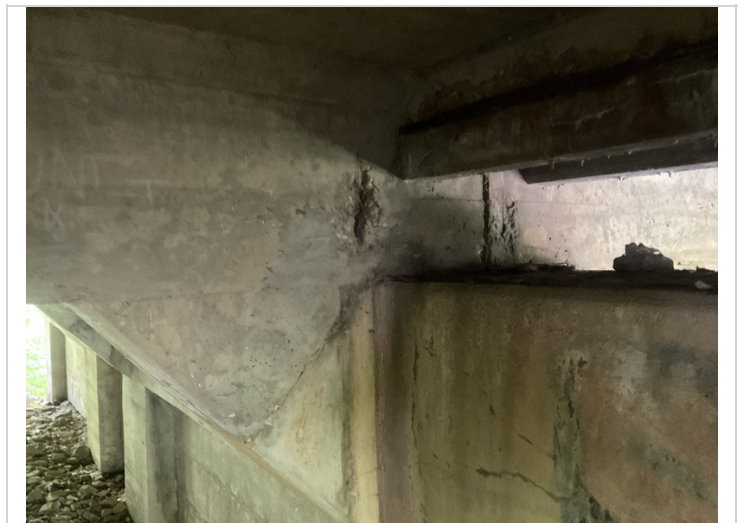
Span # 1 & 2 Girder # 3 spalling with exposed reinforcing steel.
