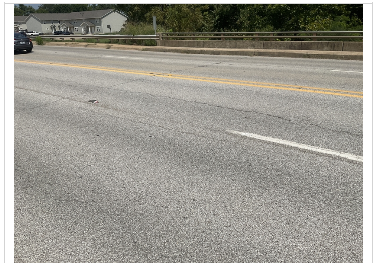
Cracking in the asphalt wearing surface.
