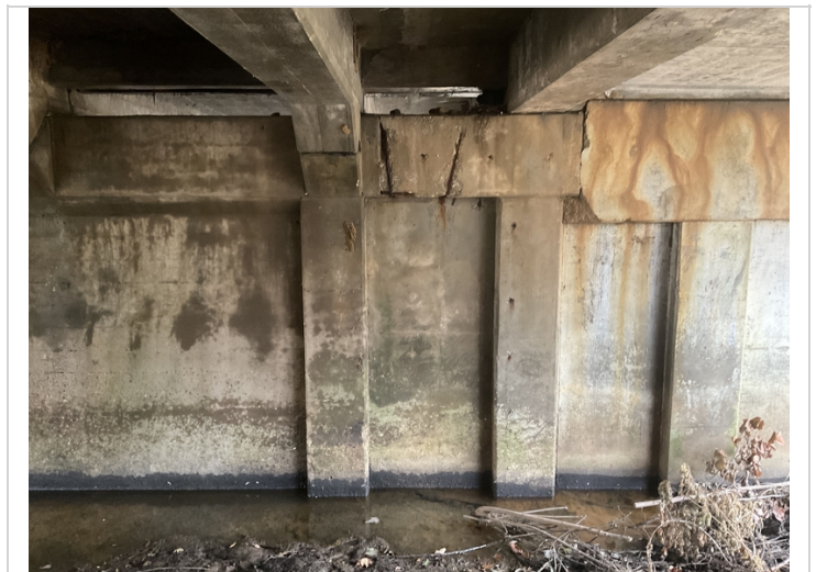
Bent #2 aheadface spalling with exposed reinforcing steel.
