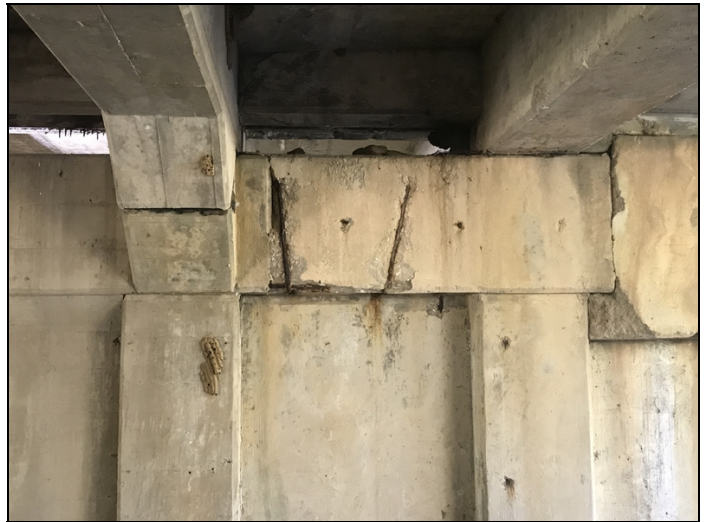
Bent # 2 cap-Spalling with exposed reinforcing in bay 1.
