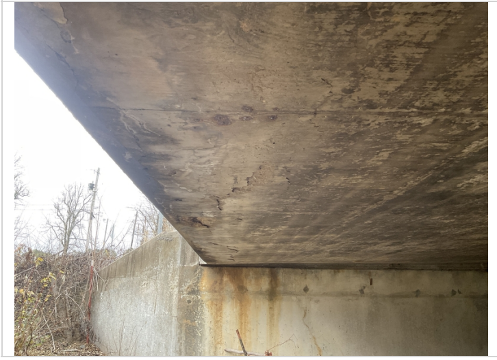
Span #2 Lt concrete delamination and spalling with exposed reinforcing steel.
