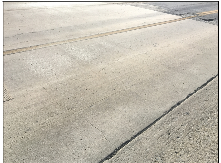
Longitudinal and mapcracking in driving surface of original portion of deck.
