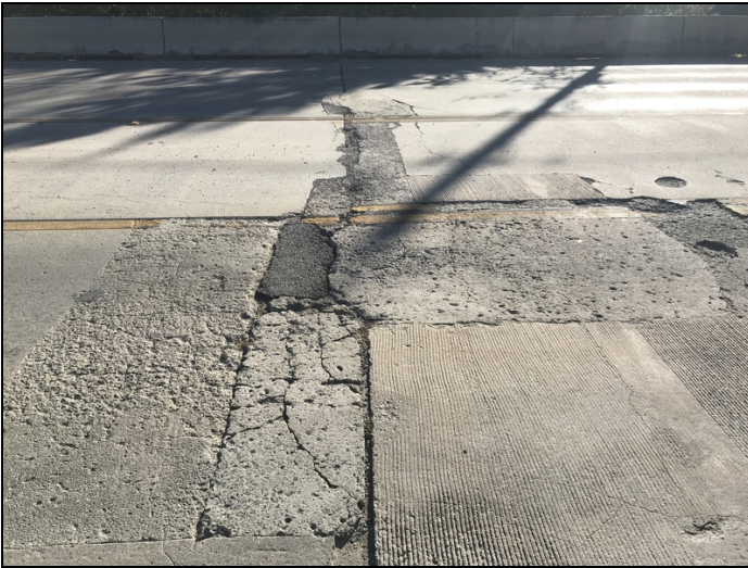
Repairs over bent 2.
