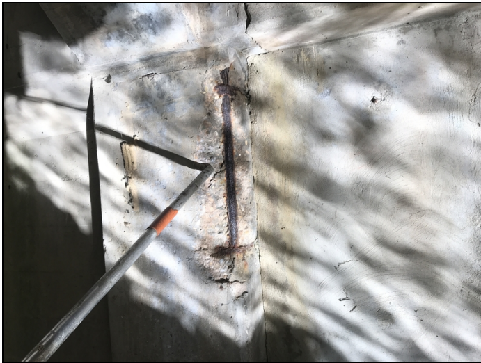
Bent # 2, column # 5-Spalling with exposed reinforcing steel.
