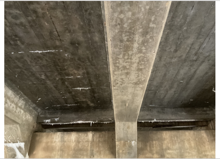
Span #1 adjacent to bent #2 transverse cracking with efflorescence buildup.
