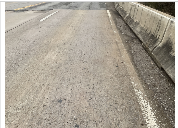
Span #1 Lt map cracking.
