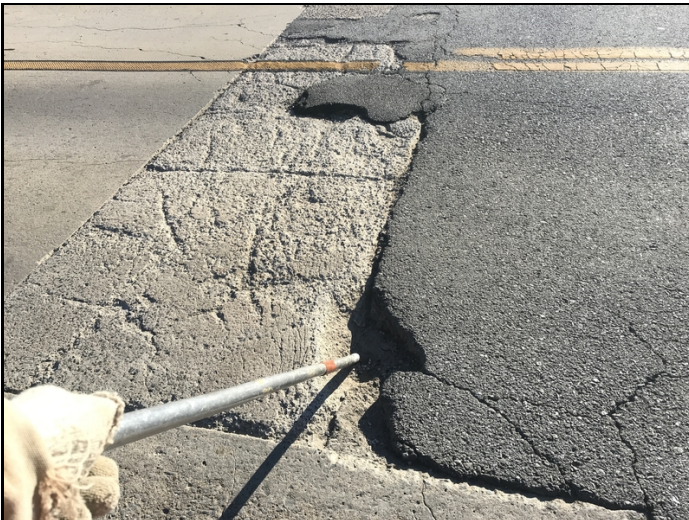
The left lane of the South approach roadway has large potholes at the bridge end.
