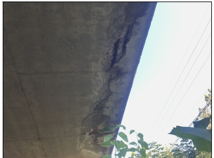
Span 2 slab, right side-Spalling / delaminated areas with exposed reinforcing steel.
