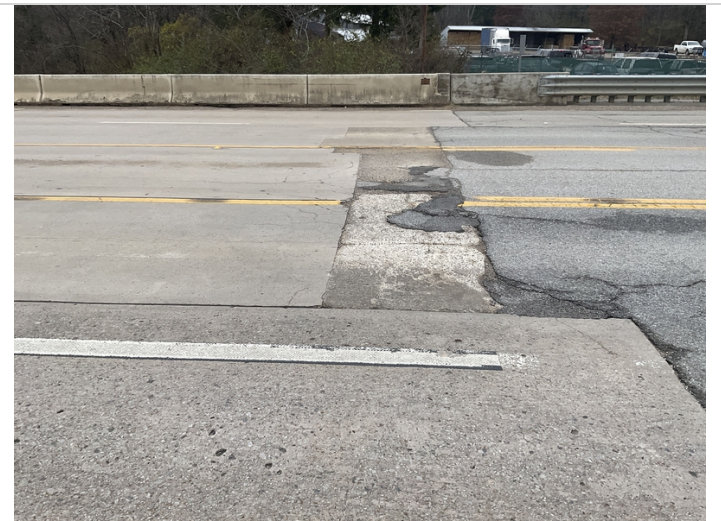
Span #1 wearing surface cracking and failing repairs.
