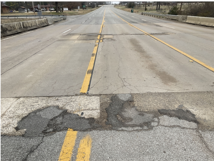
Span #1 cracking on the wearing surface.
