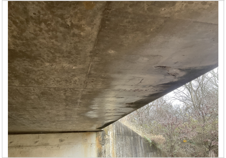
Span #1 Lt concrete delamination along the slab edges.
