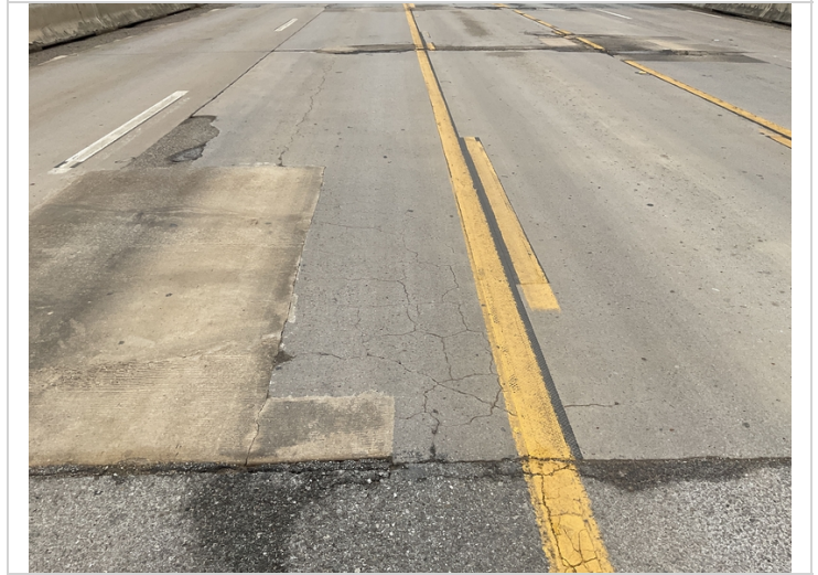
Span # 2 wearing surface cracking.
