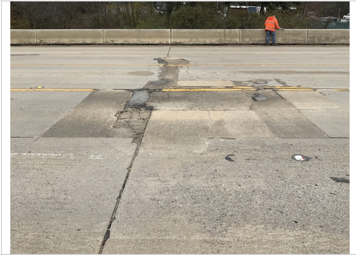
Wearing surface failed repairs over Bent #2.
