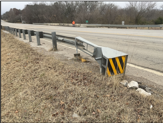
Northeast approach guardrail collision damage.
