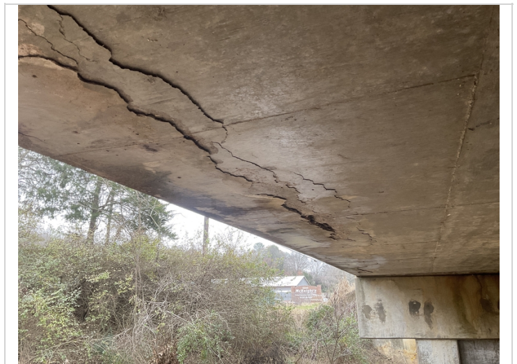
Span #2 Rt concrete delamination and spalling with exposed reinforcing steel.
