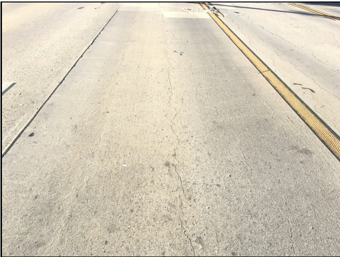
Longitudinal and mapcracking in driving surface.
