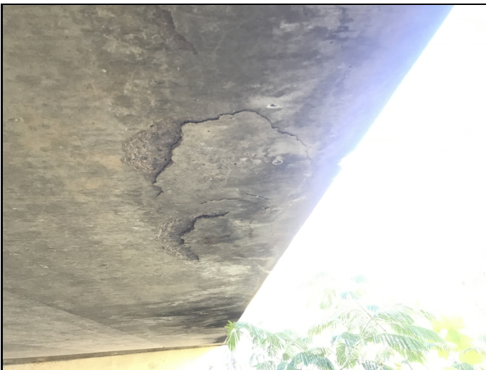
Span 1, left side-Delaminated areas along slab edge.
