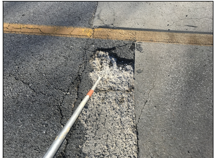
Failing repair over abutment 2.
