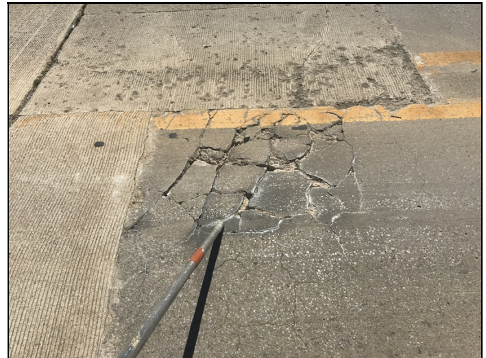
Span # 2 at bent 3-Spalled / delaminated area.
