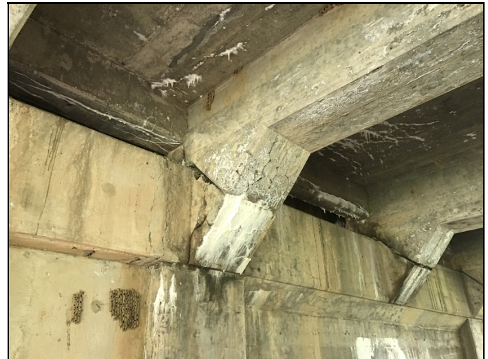
Ahead face of bent # 3 cap under girder # 4 is delaminated.
