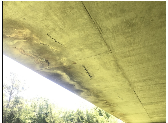
Span # 3, right side-Delaminated areas.
