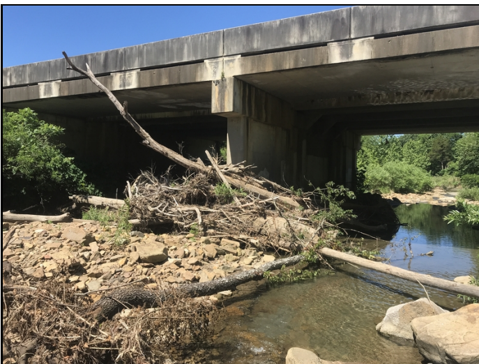
The channel has moderate drift accumulation at bent # 2.
