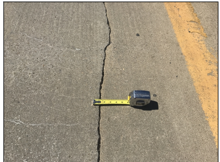
Span # 3, right lane-Wide longitudinal cracking.
