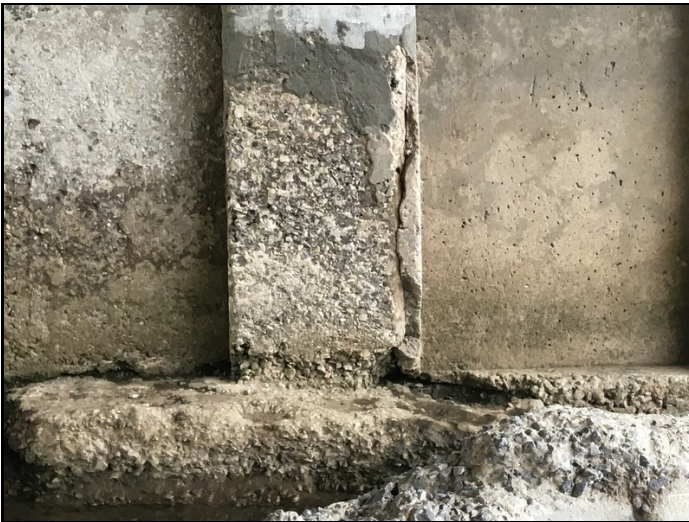
Bent # 3, column # 6-Concrete deterioration.
