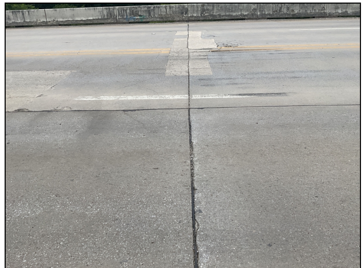
Bent # 2 typical joint seal.
