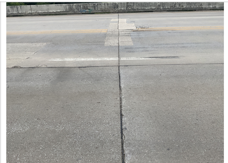
Bent # 2 typical joint seal.
