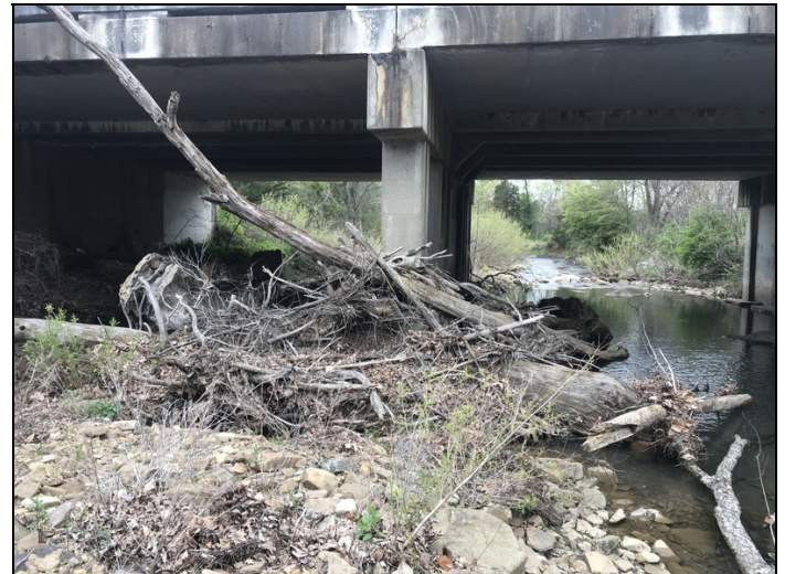
The channel has moderate drift accumulation at bent # 2.
