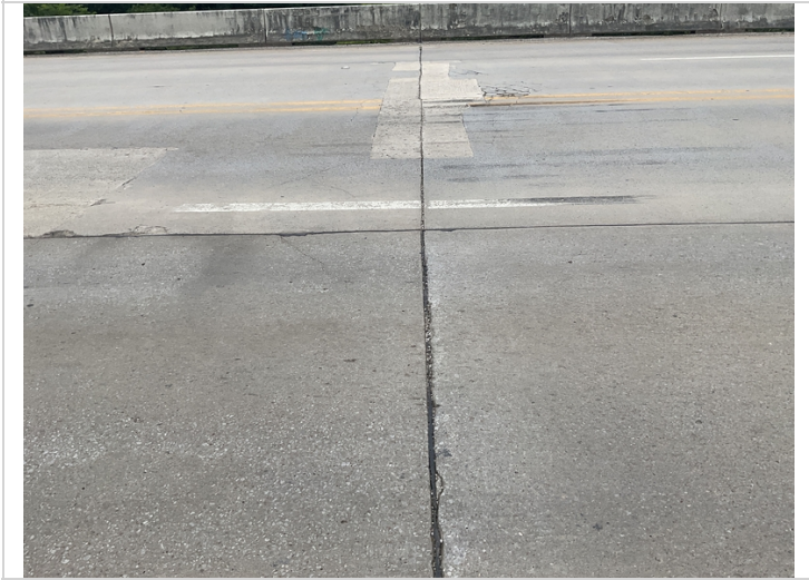
Bent # 2 typical joint seal.
