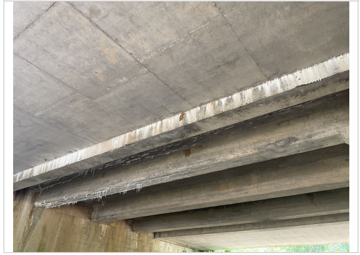
Span # 1 girder # 5 spalling with exposed reinforcing steel.
