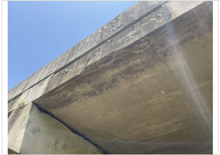
Span # 1 Lt has spalling with exposed reinforcing steel adjacent to bent # 2.
