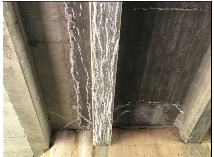
The undersurface of the deck has areas of map cracking with efflorescence adjacent to the bents at the construction joints where the structure was widened.
