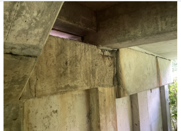
Bent # 3 cap aheadface spalling with exposed reinforcing steel and loss of bearing area.
