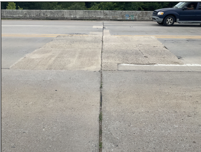
Bent # 3 typical joint seal.
