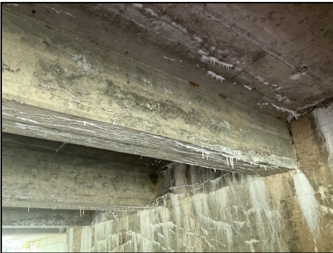
Span # 3 Girder # 4 map cracking with efflorescence buildup and concrete deterioration with section loss adjacent to Abutment # 2.
