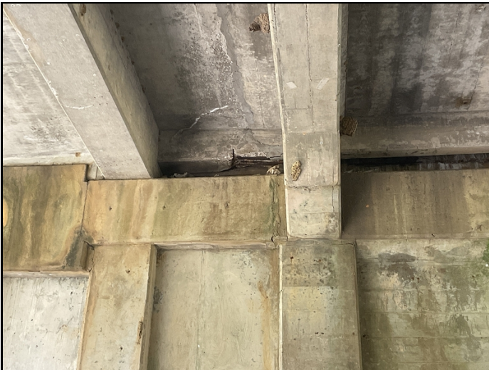
Isolated areas of concrete spalling with exposed reinforcing steel visible in the Expansion joint dams over Bents # 2 & 3.
