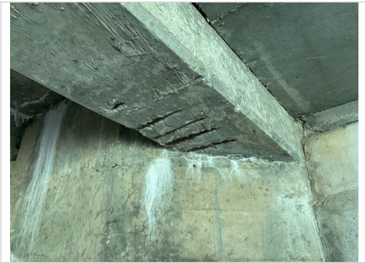
Span # 3 Girder # 5 spalling with exposed reinforcing steel.
