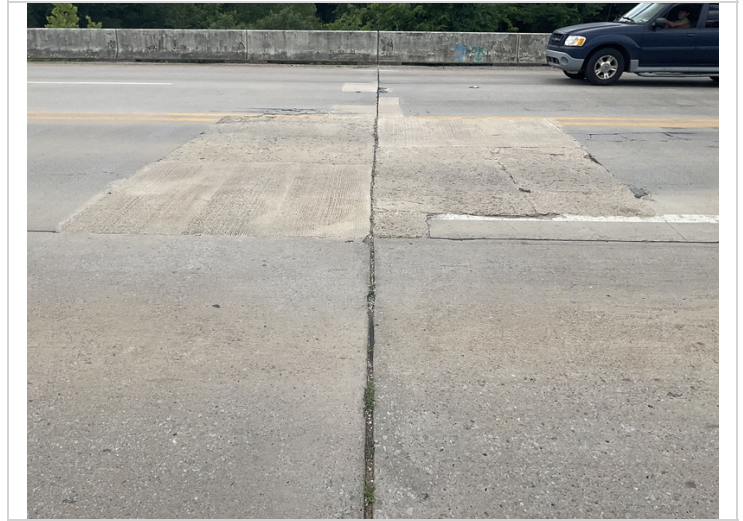
Bent # 3 typical joint seal.
