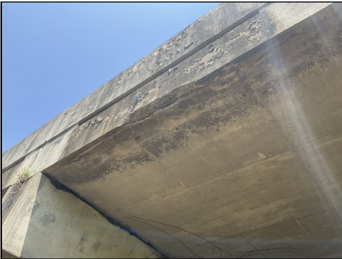
Span # 1 Lt has spalling with exposed reinforcing steel adjacent to bent # 2.
