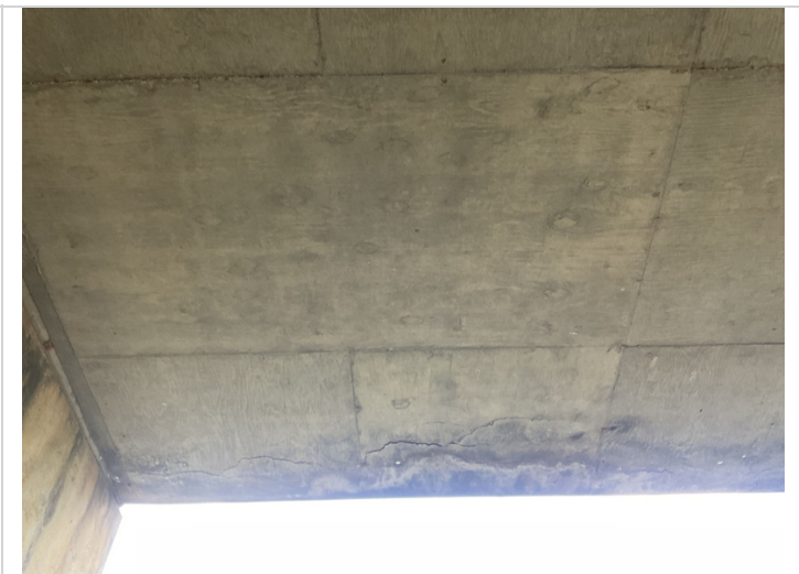
Span # 2 Rt concrete delamination along the edge of the slab.
