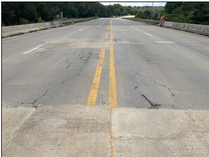
Concrete cracking and spalling on the wearing surface.
