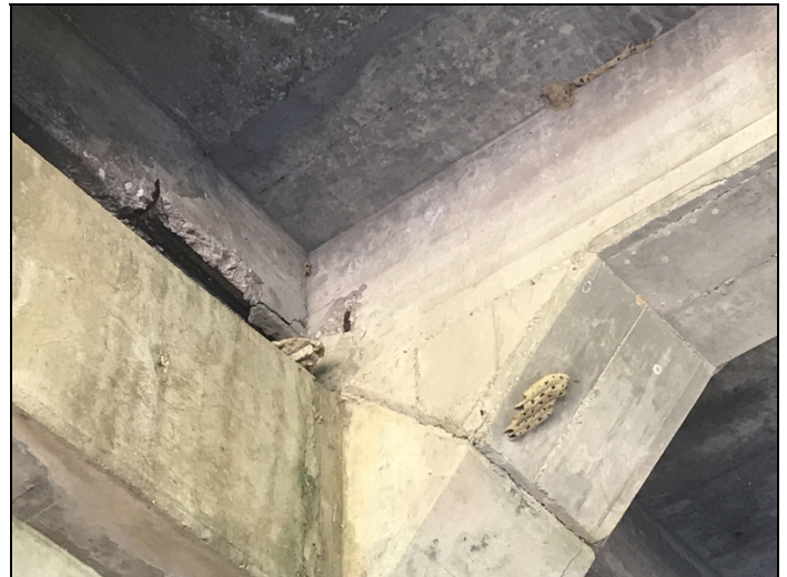
Isolated areas of concrete spalling with exposed reinforcing steel visible in the Expansion dams over Bents # 2 & 3.
