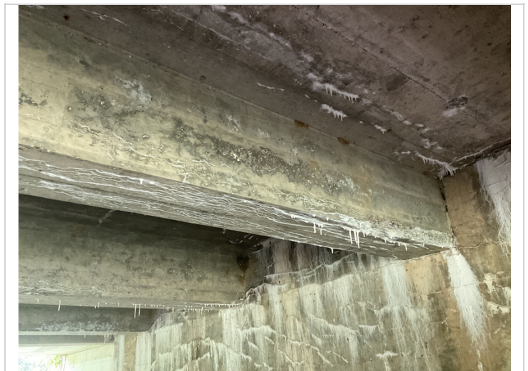
Span # 3 Girder # 4 map cracking with efflorescence buildup and concrete deterioration with section loss adjacent to Abutment # 2.
