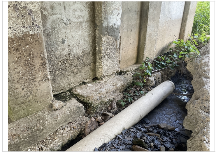
Bent # 3 Column # 6 concrete deterioration along the column base.
