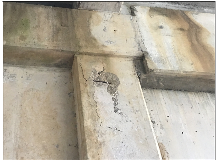
Bent # 2, column # 3-Spalling in ahead face with exposed reinforcing steel.
