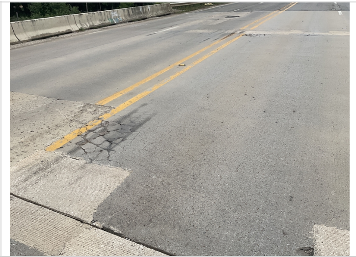
Wearing surface breakup over the intermediate bents.
