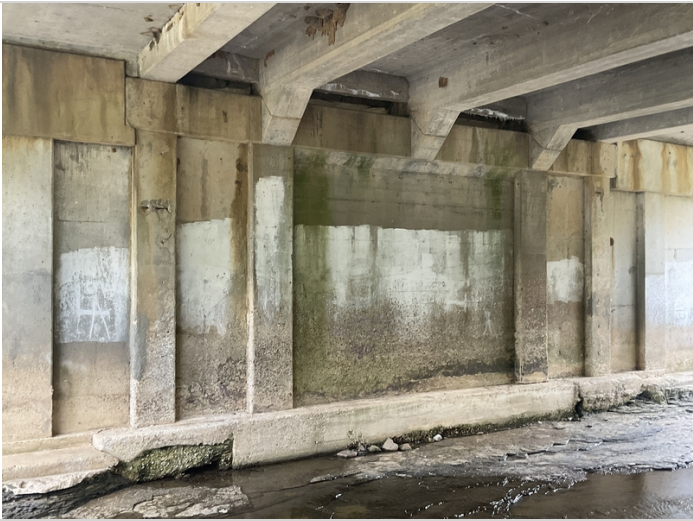
Bent # 2 column # 3 & 6 spalling with exposed reinforcing steel.
