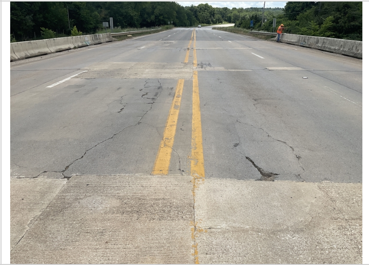
Concrete cracking and spalling on the wearing surface.
