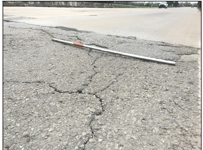
South approach roadway-Settlement in right lane.
