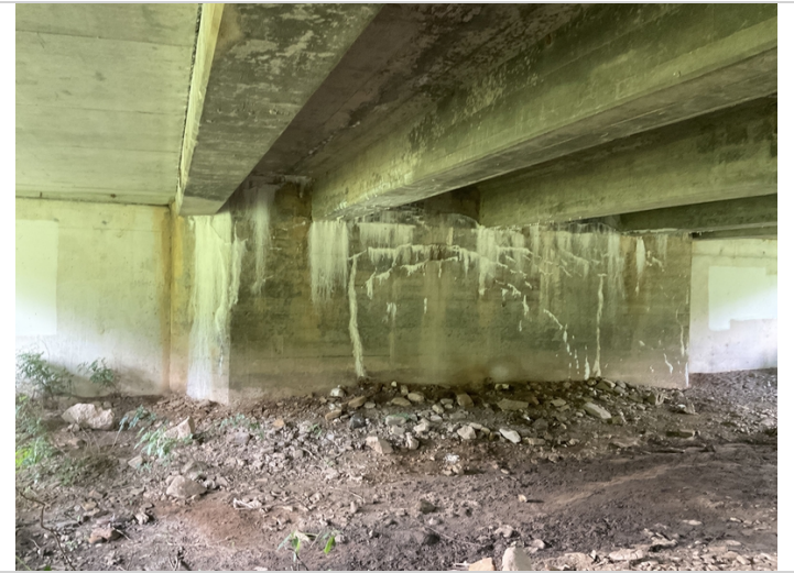
Abutment # 2 cracking with efflorescence buildup.
