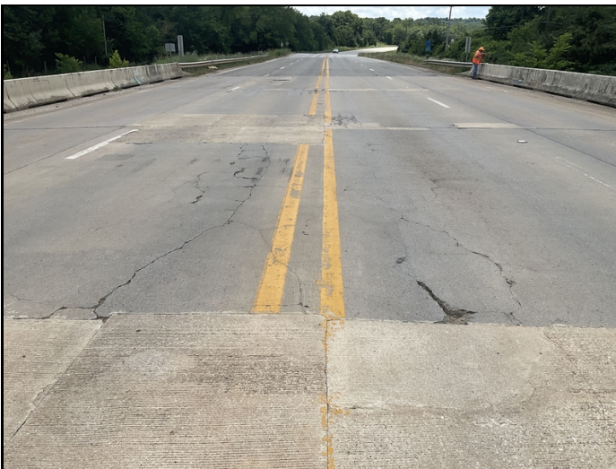
Concrete cracking and spalling on the wearing surface.
