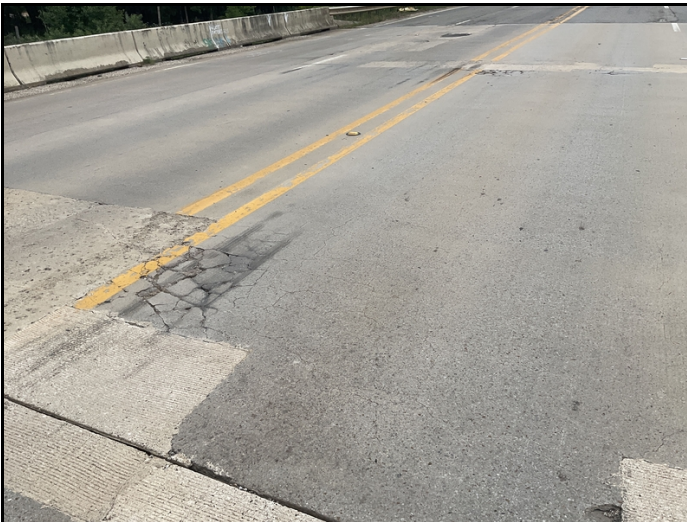
Wearing surface breakup over the intermediate bents.
