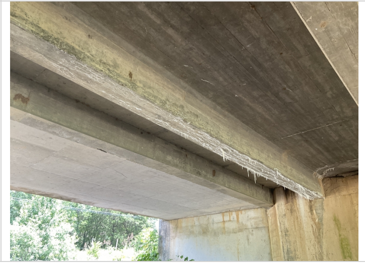
Span # 1 girder # 4 map cracking with efflorescence buildup.
