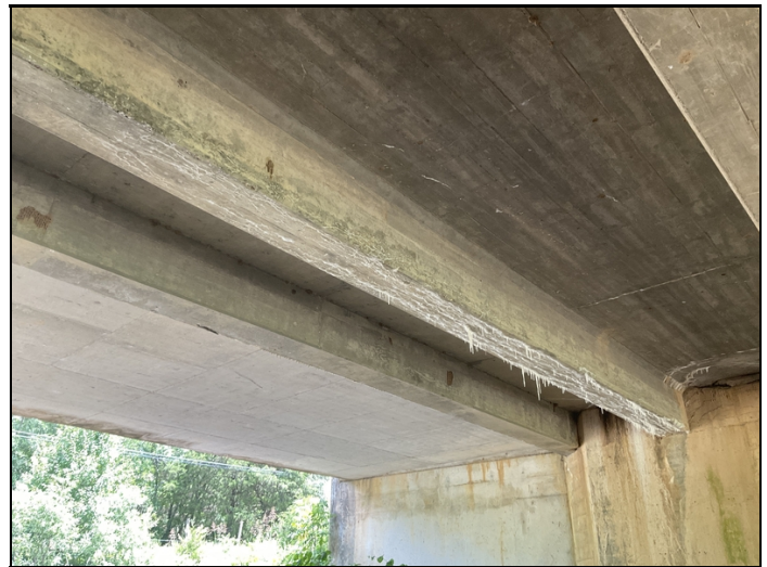
Span # 1 girder # 4 map cracking with efflorescence buildup.
