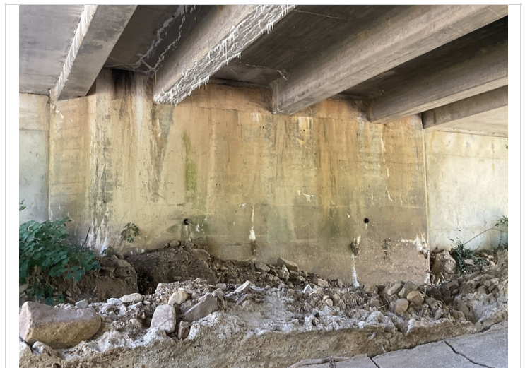
Abutment # 1 cracking with efflorescence buildup.
