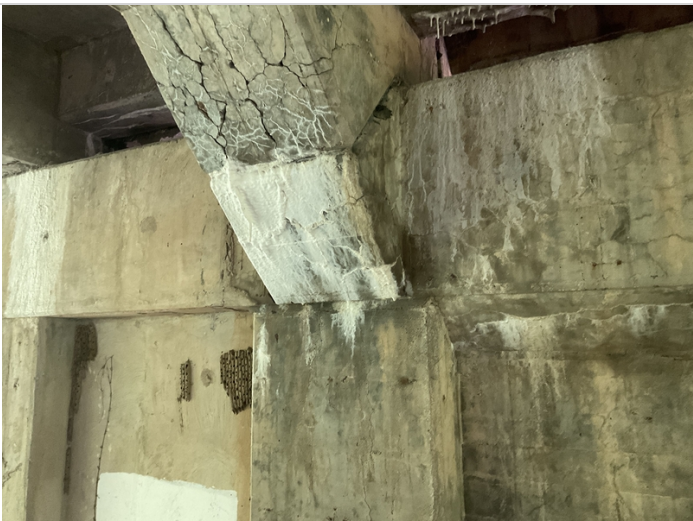
Bent # 3 aheadface wide map cracking with efflorescence buildup under Girder # 4.
