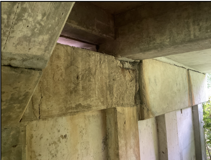
Bent # 3 cap aheadface spalling with exposed reinforcing steel and loss of bearing area.
