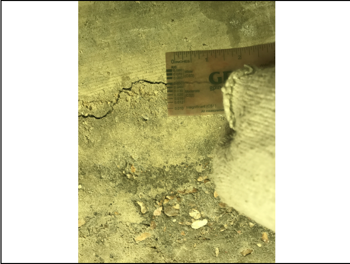
Span # 3, girder 4-Moderate width longitudinal crack.
