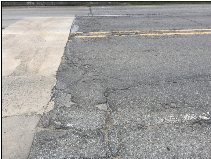
North approach roadway-Mapcracking in asphalt.
