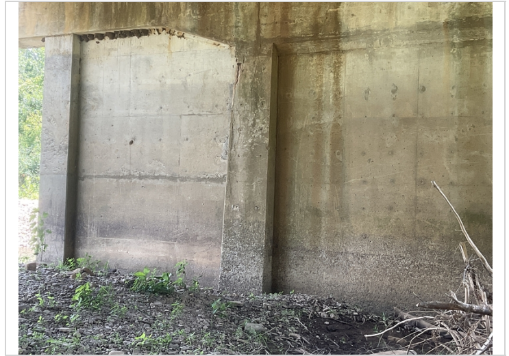
Bent # 6, column # 3 aheadface has an 8' height delaminated/spalled area with exposed reinforcing steel.
