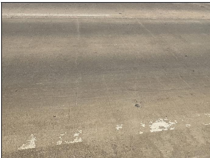
Span # 7 deck cracking.
