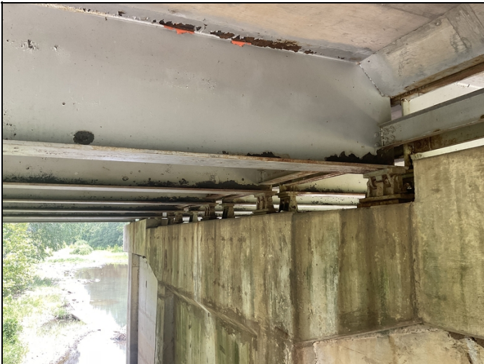
Span # 6 Bent # 6 active corrosion, pack rust and section loss.
