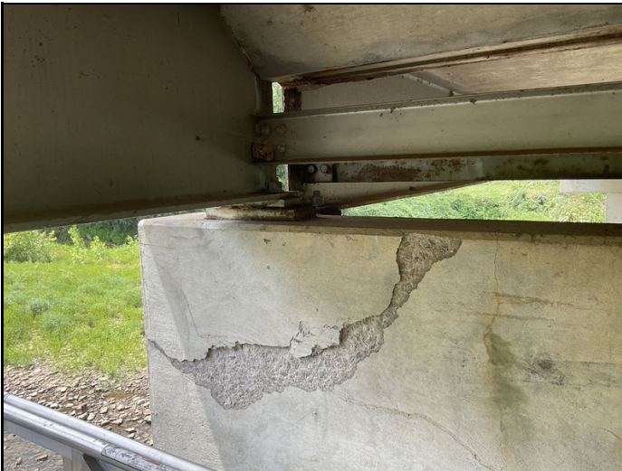
Bent # 4 Lt cap backface with an approximately 4' long X 30" tall concrete delamination that extends from the Lt end of the cap under beam # 1 and appears to extend approximately 2" under the bearing.
