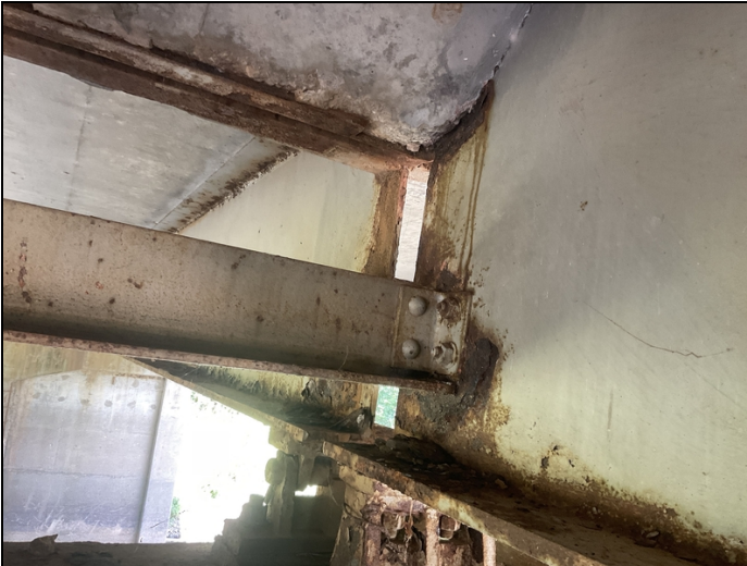
Span # 4, Beam # 7 at Bent # 5 has up to 5/16" section loss at the base of the expansion dam juncture and up to 3/16" section loss at the diaphragm connection.
