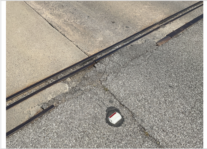
Abutment # 1 Northbound lane cracked welds.
