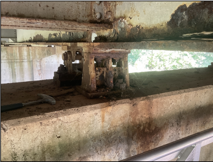
Bent # 5 bearing # 5 active corrosion with pack rust.
