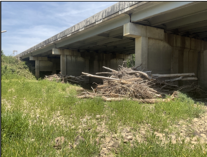
Bents # 5 & 6 drift accumulation.
