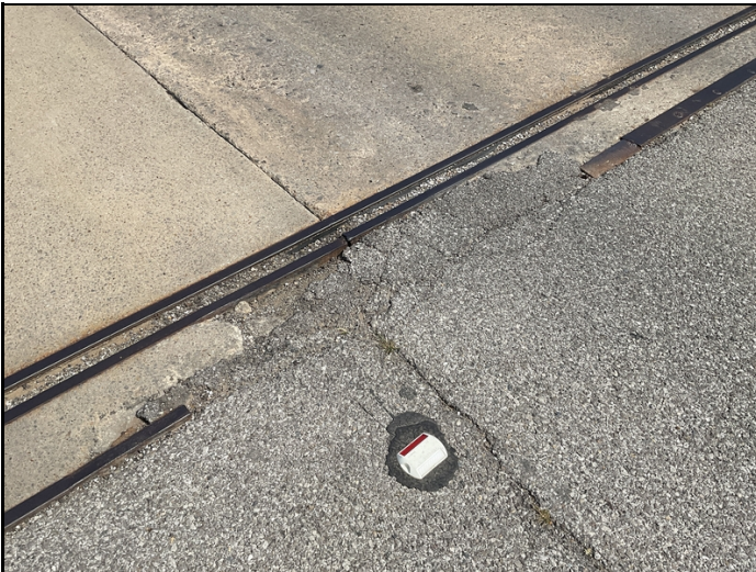
Abutment # 1 Northbound lane cracked welds.
