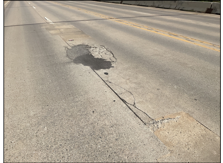
Span # 2 has a 2' wide x 16' long area of delaminated concrete that is breaking apart in the South bound lanes that is raised up approximately 1.5" higher than the surrounding deck area.
