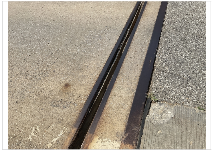
Abutment # 2 strip seals has areas that appear to be pulling out of the extrusion or tearing loose at the extrusion.
