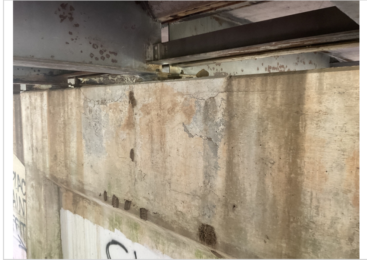
Bent # 2 backface has several moderate sized concrete delaminations and 2 moderate / wide width cracks in the vertical face of the cap located in the original portion of the cap located between beams # 4 - 6.
