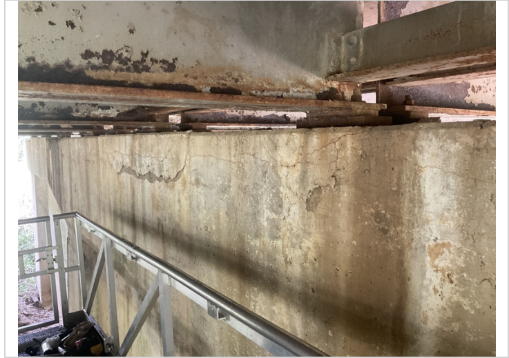
Bent # 3 backface under beams # 4 - 6 has an approximately 9' long X 12" wide concrete delamination in the vertical face of the cap.
