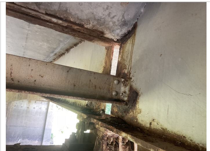
Span # 4, Beam # 7 at Bent # 5 has up to 5/16" section loss at the base of the expansion dam juncture and up to 3/16" section loss at the diaphragm connection.
