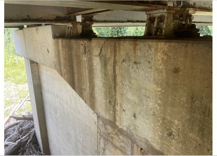
Bent # 5 Lt backface under bay # 3 has a 5' long horizontal crack with a 10" spall with exposed reinforcing steel, the exposed reinforcing steel has active corrosion and initial section loss.
