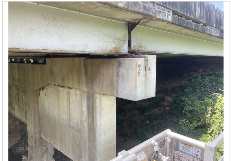
Bent # 7 Rt end of the cap spalling.
