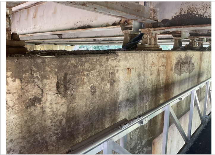
Bent # 4 cap aheadface has a moderate width horizontal crack under beams # 5 - 7 with random delaminations along the crack and a 4' long spall with exposed reinforcing steel under bay # 5 and a 8" spall with exposed reinforcing steel under bay # 6. The exposed reinforcing steel has active corrosion and approximately 20% section loss.
