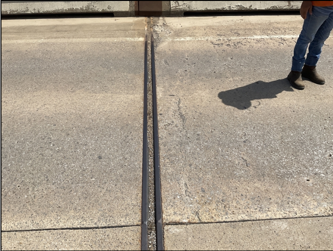
Span # 1 outside lane and shoulder has delaminated concrete and a 5" long area that is breaking apart and extend above the driving surface approximately 1" adjacent to bent # 2.
