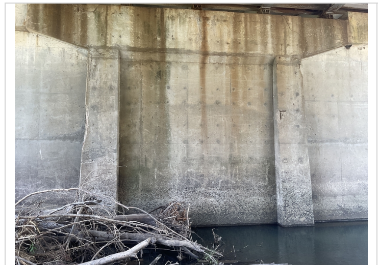
Bent # 5, columns # 2 & 3 backface have multiple spalls with exposed reinforcing steel. Exposed reinforcing steel has active corrosion and pack rust.
