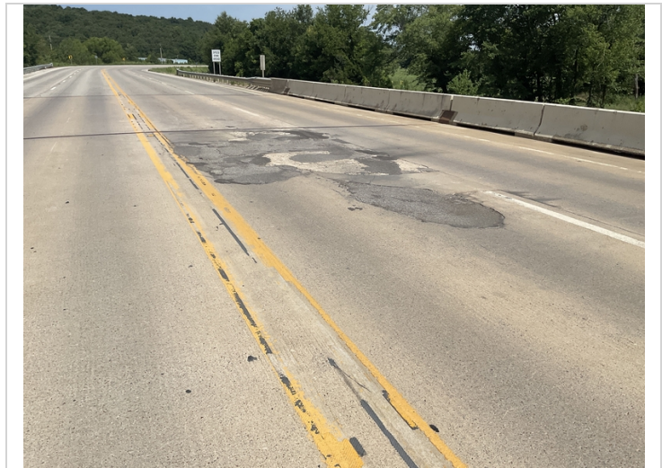
Span # 6 northbound lane with numerous temporary asphalt patches.
