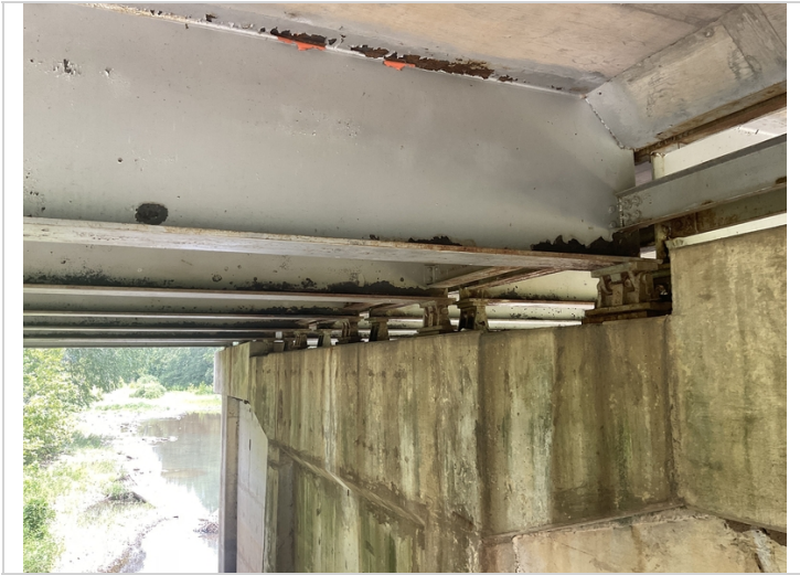
Span # 6 Bent # 6 active corrosion, pack rust and section loss.
