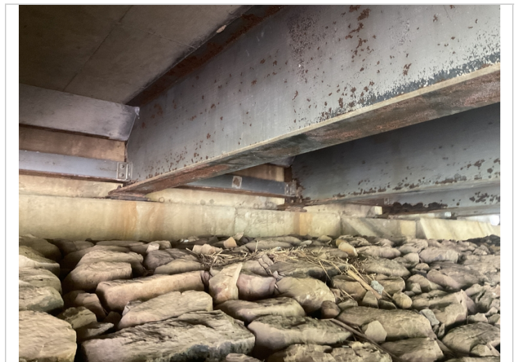
Span # 1, Beams # 3 - 7 have active corrosion, pack rust and up to 1/8" section loss to the webs and bottom flange over Abutment # 1.
