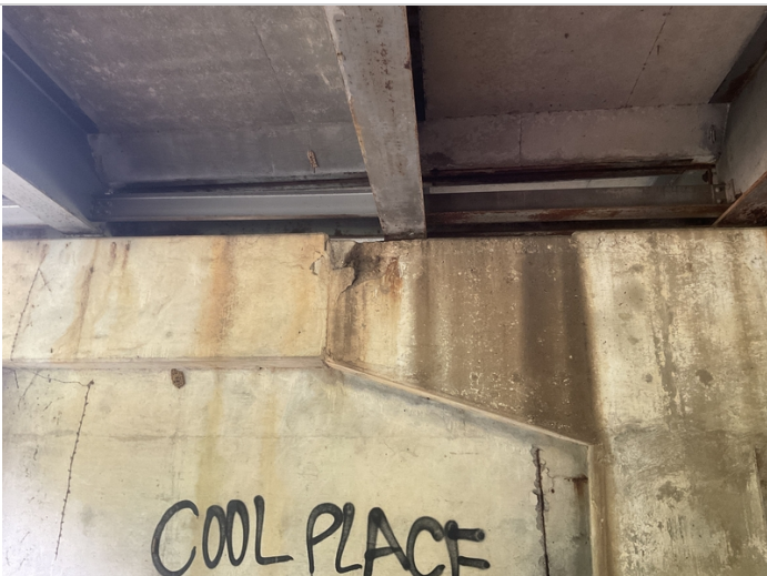
Bent # 2 cap backface has a 1' spall with exposed reinforcing steel in the bearing area of beam # 3.
