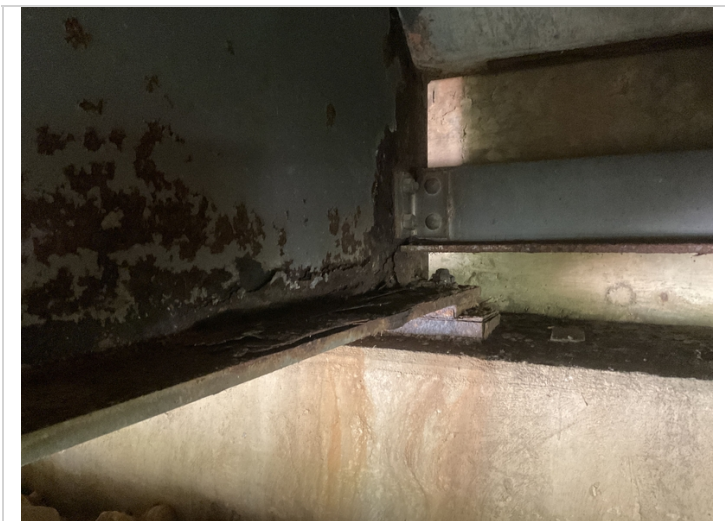
Abutment # 1 beam # 5 active corrosion with pack rust.
