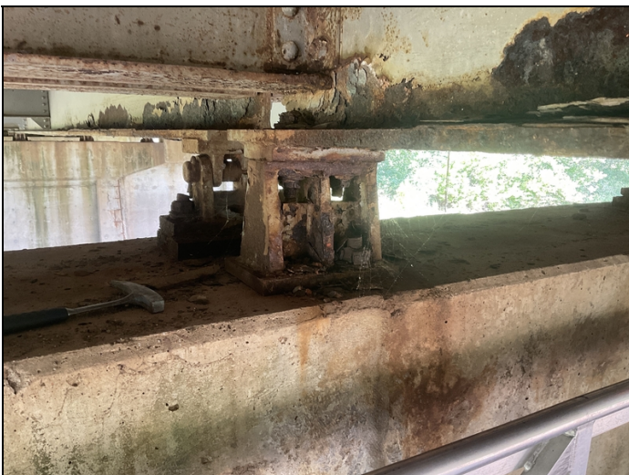
Bent # 5 bearing # 5 active corrosion with pack rust.
