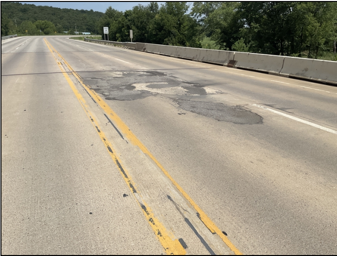
Span # 6 northbound lane with numerous temporary asphalt patches.
