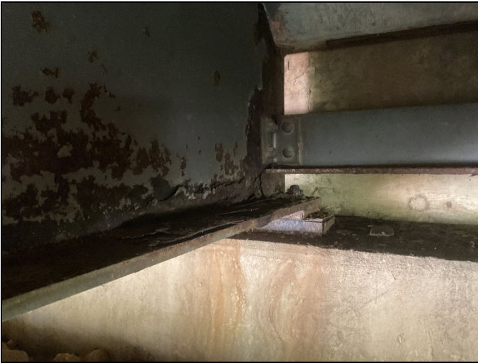
Abutment # 1 beam # 5 active corrosion with pack rust.
