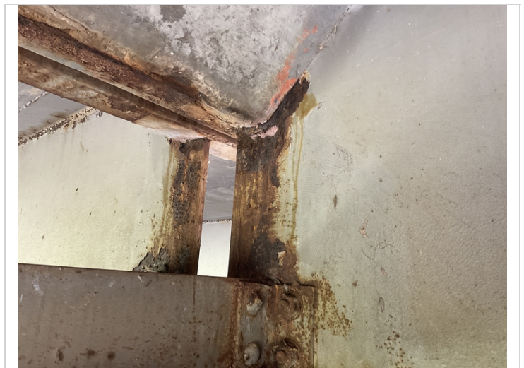
Span # 4, beam # 5 at bent # 5 has a 3" X 1" hole rusted through top of web at the expansion dam juncture.
