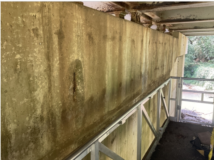
Bent # 6 cap aheadface has a 1' horizontal spall with exposed reinforcing steel over column # 1 and a 2' vertical spall with exposed reinforcing steel located over column # 3.
