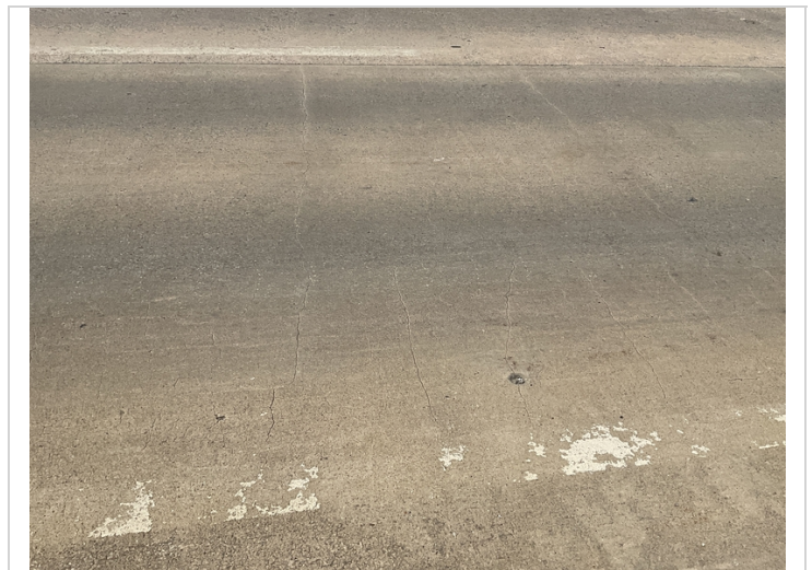
Span # 7 deck cracking.
