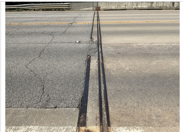
Abutment # 1 strip seal.
