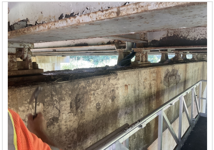
Bent # 4 moveable bearings with active corrosion and minor areas of flaking rust forming.
