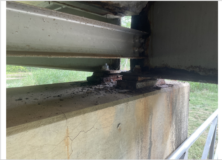
Bent # 2 bearings # 9 active corrosion with pack rust and section loss.
