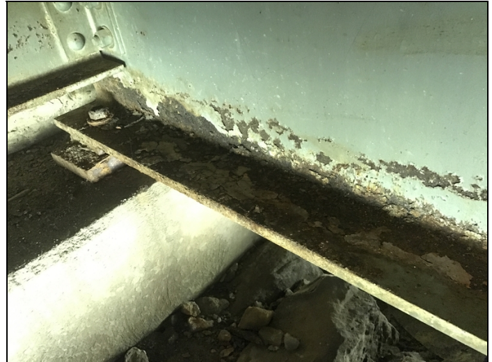
Bent # 1. Beam # 3. Corrosion.
