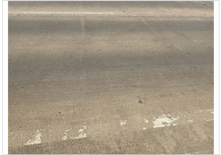
Span # 7 deck cracking.
