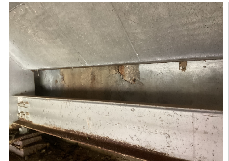
Abutment # 1, bay # 1 spalls with exposed reinforcing steel in the back wall.
