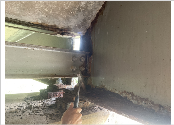
Span # 1, Beam # 9 with up to 3/16" section loss below the expansion dam.
