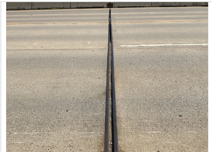
Bent # 4 strip seal typical.
