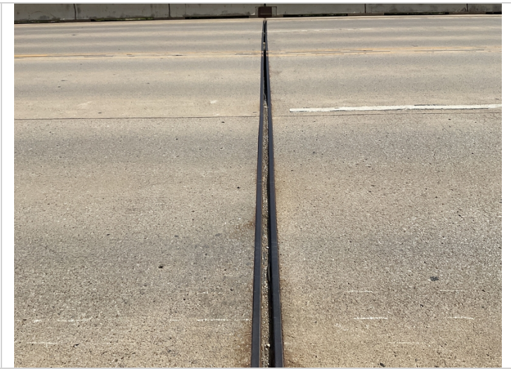
Bent # 4 strip seal typical.
