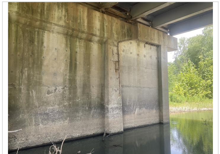
Bent # 6, column # 3 backface has a 10' tall spall with exposed reinforcing steel. The exposed reinforcing steel has active corrosion and pack rust.
