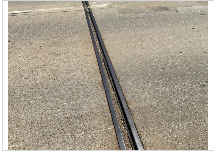
Bent # 3 strip seal working out of the anchorage extrusion.
