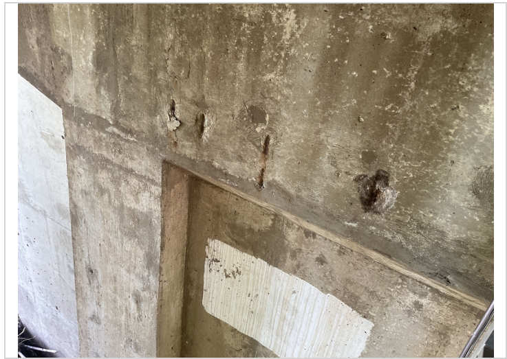
Bent # 4 cap backface has 4 small vertical shallow spalls with exposed reinforcing steel with active corrosion and initial section loss near the bottom edge of the cap adjacent to column # 2.
