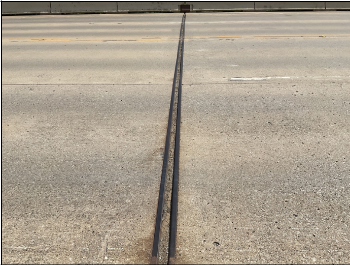
Bent # 6 strip seal typical.
