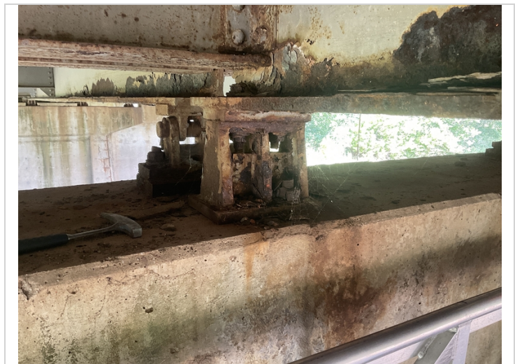
Bent # 5 bearing # 5 active corrosion with pack rust.
