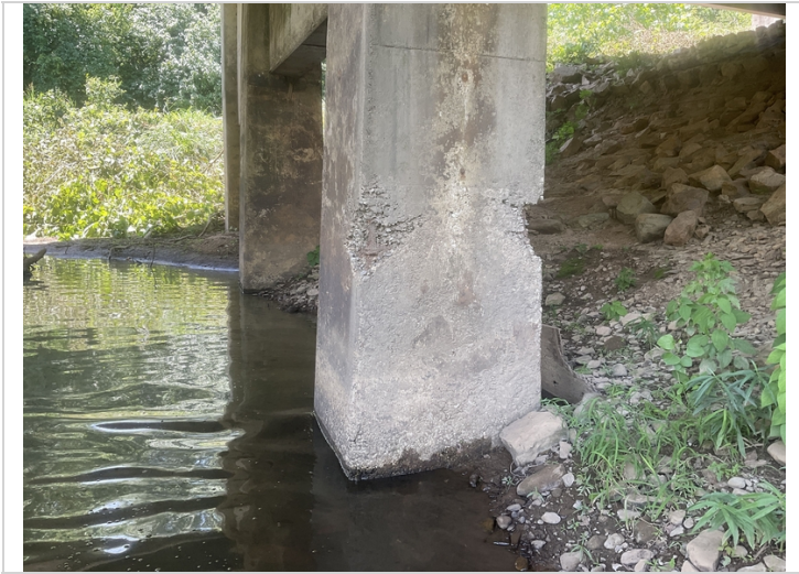
Bent # 7, column # 3 has two 12" tall areas of honeycomb with exposed primary reinforcing steel located 4' above base of column. The exposed steel has corrosion with initial section loss.
