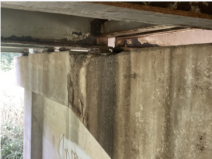
Bent # 3 beam # 3 cap backface spalling with exposed reinforcing steel.
