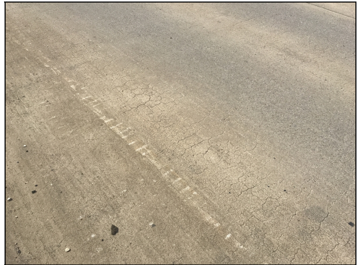
Span 4, right lane-Mapcracking.
