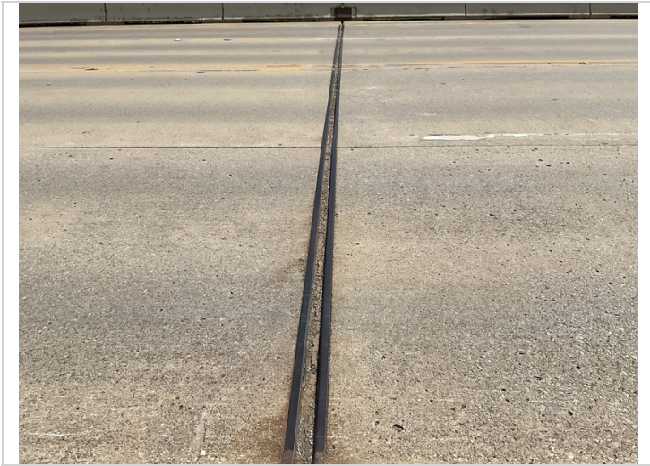
Bent # 6 strip seal typical.
