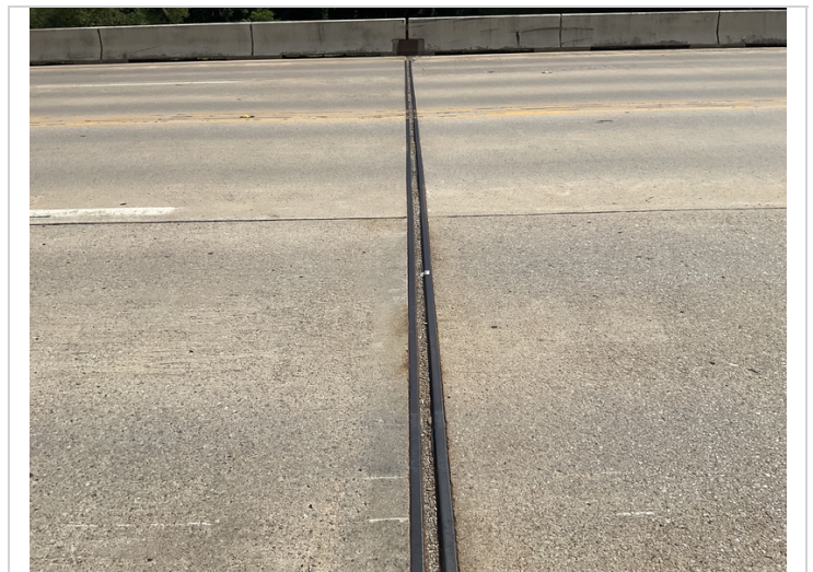
Bent # 2 strip seal typical.
