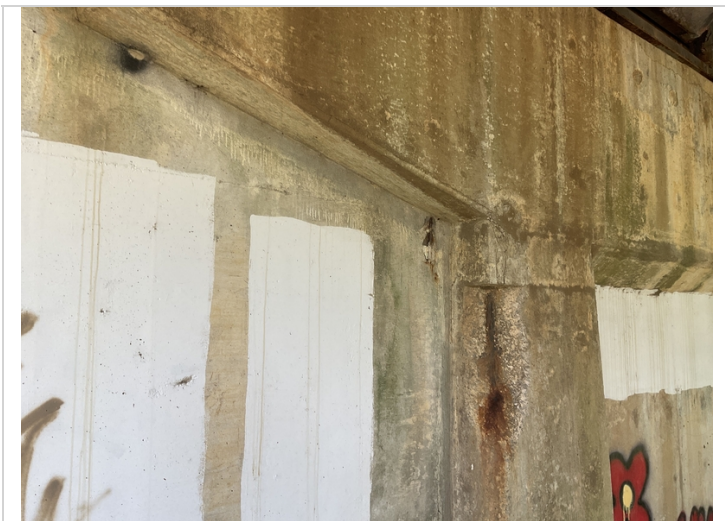
Bent # 3 Rt aheadface has a 6" spall with exposed reinforcing steel adjacent to the top of the Rt edge of column # 3. The exposed reinforcing steel has active corrosion and pack rust.
