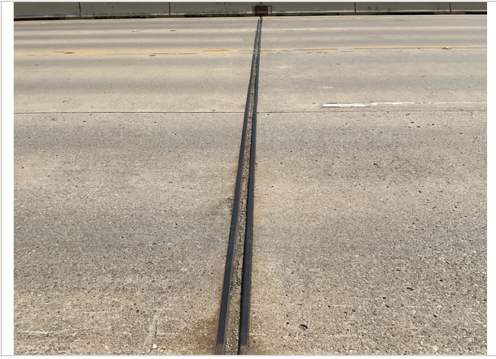
Bent # 6 strip seal typical.
