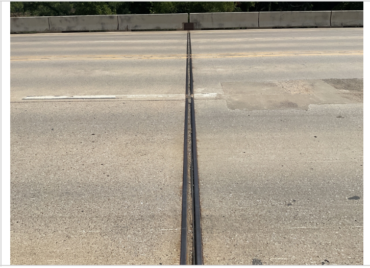
Bent # 3 strip seal typical.
