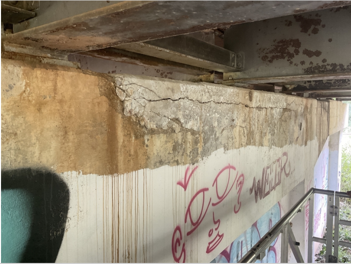
Bent # 2 aheadface under beams 4 - 6 has a 12' long X 13" tall delaminated area with a 5/16" wide horizontal crack, the crack extends approximately 1" under beam # 5 bearing device.
