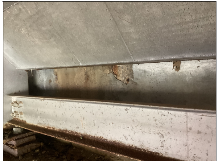
Abutment # 1, bay # 1 spalls with exposed reinforcing steel in the back wall.
