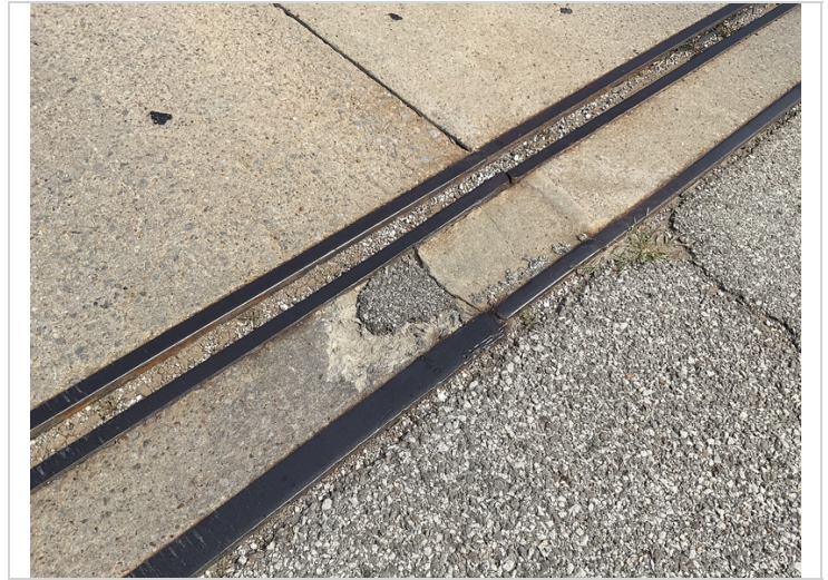
Abutment # 1 Southbound lane cracked weld.
