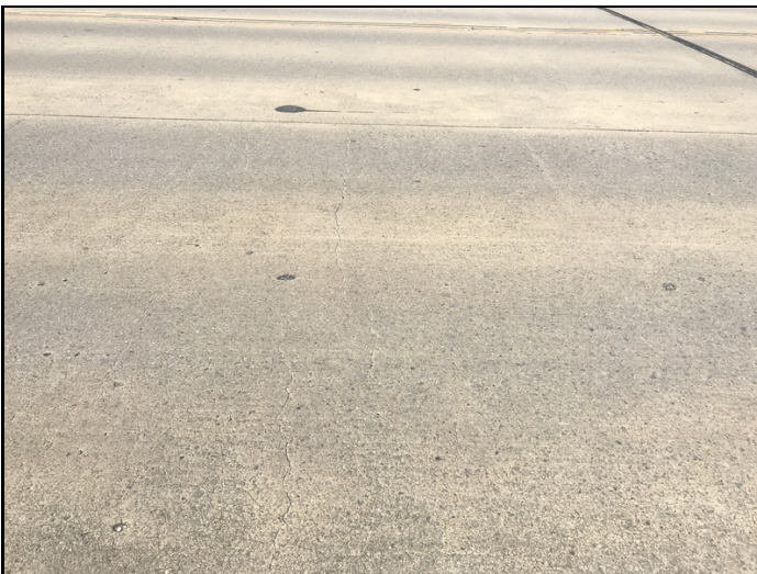
Span 2, right lane-Transverse cracking.
