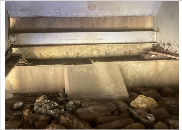
Abutment # 2 fixed bearings with active corrosion and pack rust.
