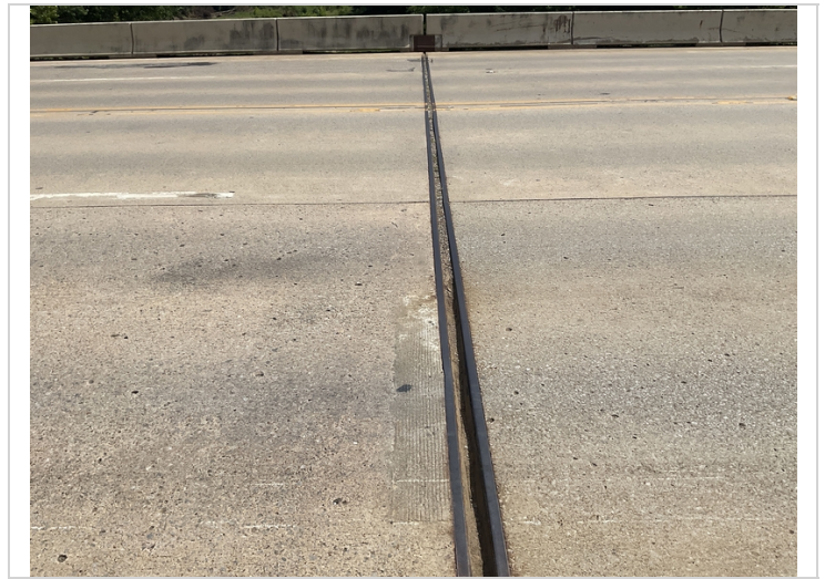
Bent # 5 strip seal typical.
