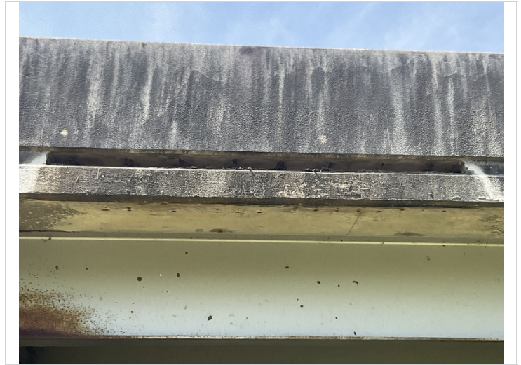
Bridge rail typical spalling with exposed reinforcing steel.
