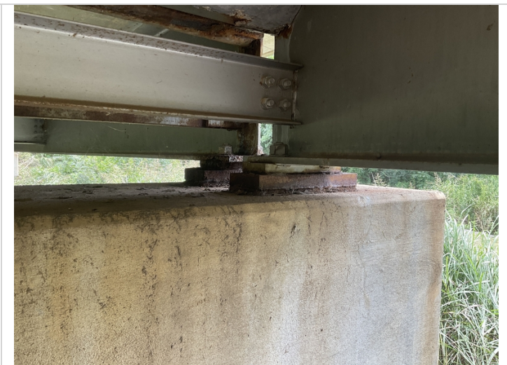
Bent # 3 bearings with active corrosion and pack rust.
