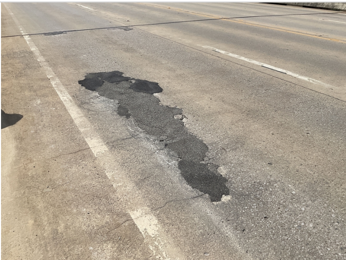
Span # 4 northbound outside lane has a 12' long X 30" wide area of temporary asphalt patches.
