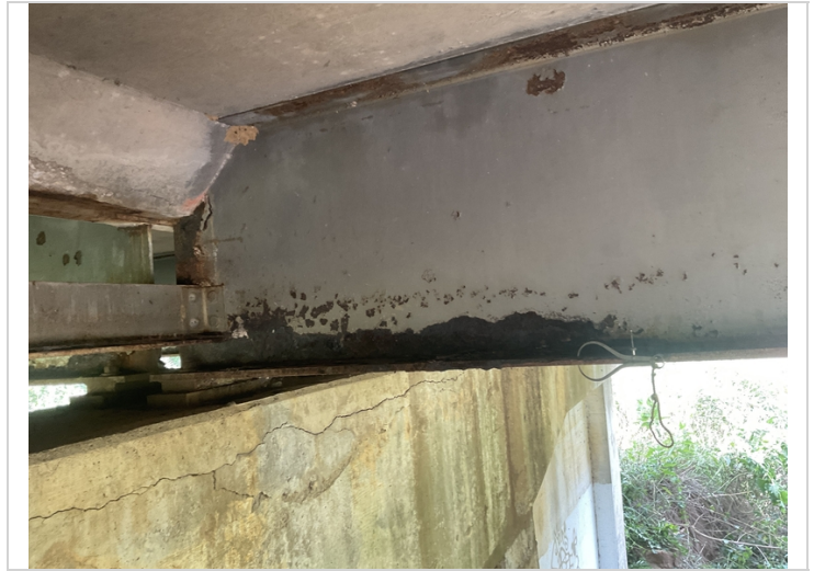
Span # 3, Beam # 5 with up to 2' long area of the bottom flange that has been reduced to approximately 5/8" remaining section.
