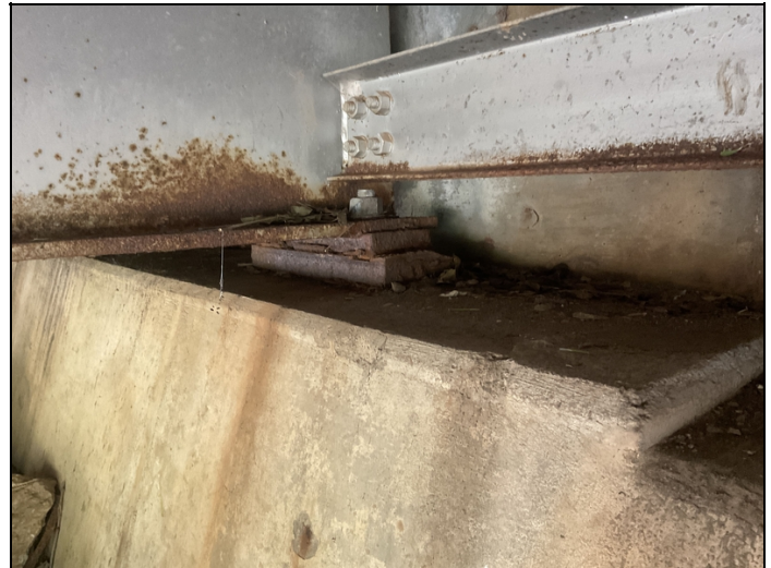
Abutment # 1 bearing # 2 active corrosion with pack rust.
