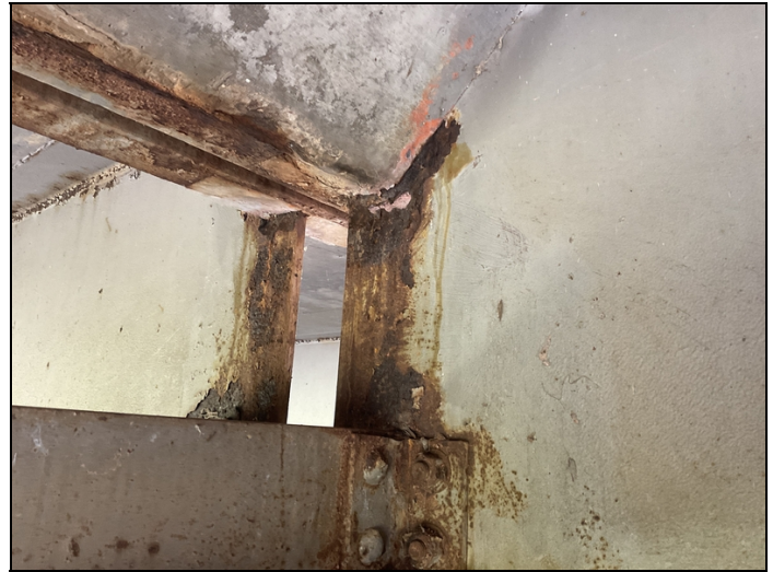
Span # 4, beam # 5 at bent # 5 has a 3" X 1" hole rusted through top of web at the expansion dam juncture.
