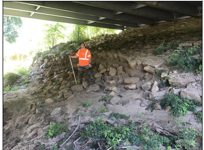
North abutment. Erosion and displacement of hand placed rip rap.
