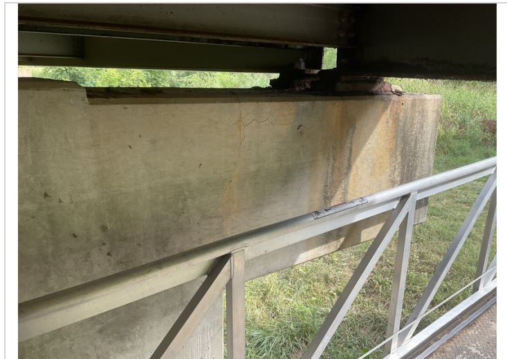
Bent # 2 Rt end of the cap has a semi diagonal crack over the exterior column with horizontal cracks propagating from the diagonal cracking.
