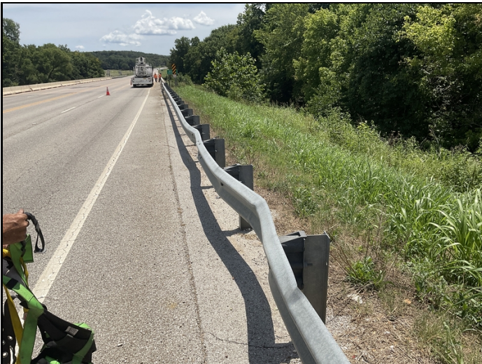
Northwest approach guardrail. Approximately 22' of damaged rail.
