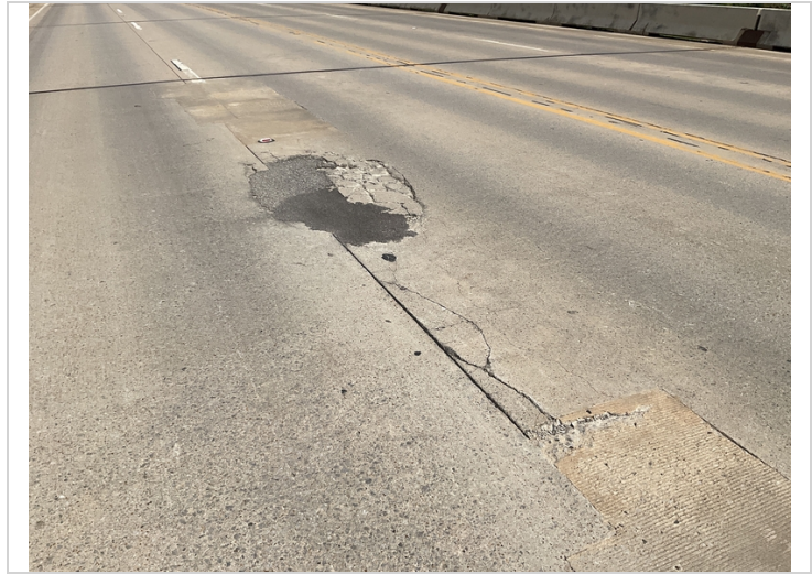
Span # 2 has a 2' wide x 16' long area of delaminated concrete that is breaking apart in the South bound lanes that is raised up approximately 1.5" higher than the surrounding deck area.
