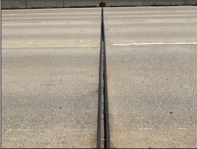
Bent # 4 strip seal typical.
