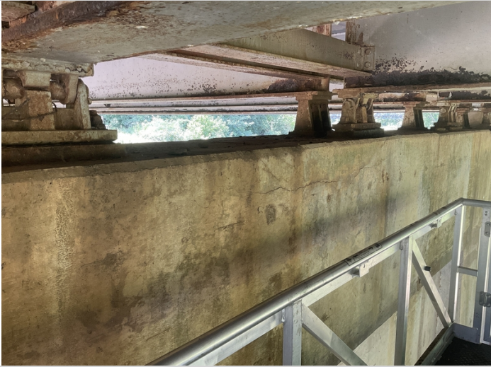
Bent # 5 cap aheadface under bay # 5 has a short duration moderate width horizontal crack with a few small concrete delaminations along the cracking.
