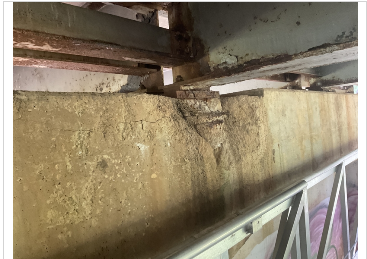
Bent # 3 beam # 7 cap backface spalling with exposed reinforcing steel.
