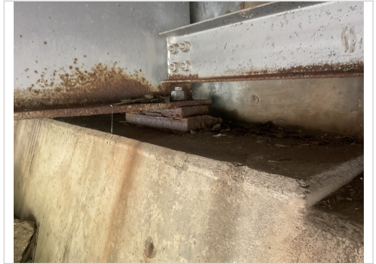
Abutment # 1 bearing # 2 active corrosion with pack rust.
