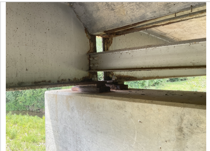
Bent # 5 bearing # 1 active corrosion with pack rust and section loss.
