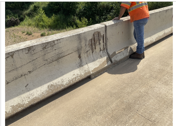
Span # 4 Rt spalling with exposed reinforcing steel in the bridge rail.
