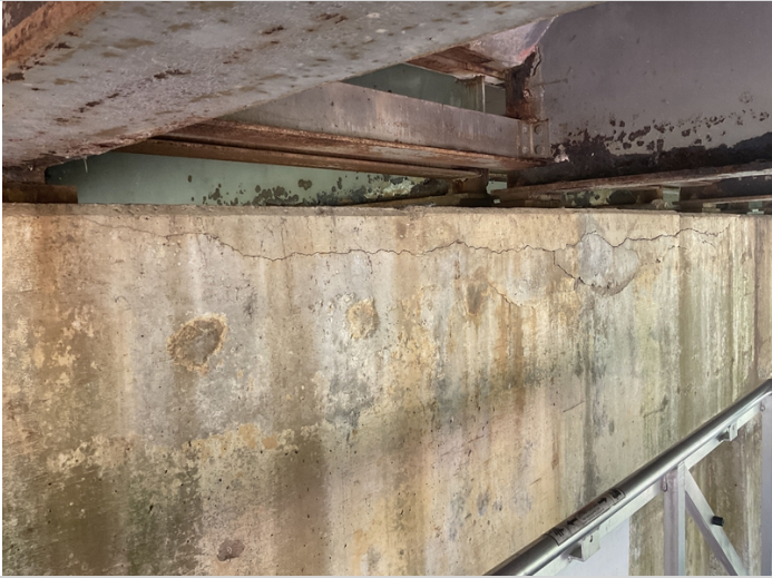
Bent # 3 cap aheadface under beams # 4 - 6 has an approximately 12' long X 13" wide concrete delamination in the vertical face of the cap.
