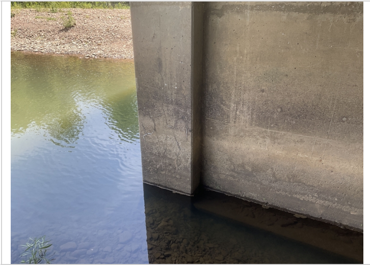
Bent # 5, column # 4 has mapcracking with moderate width vertical cracks and efflorescence buildup in the lower portion of the column.
