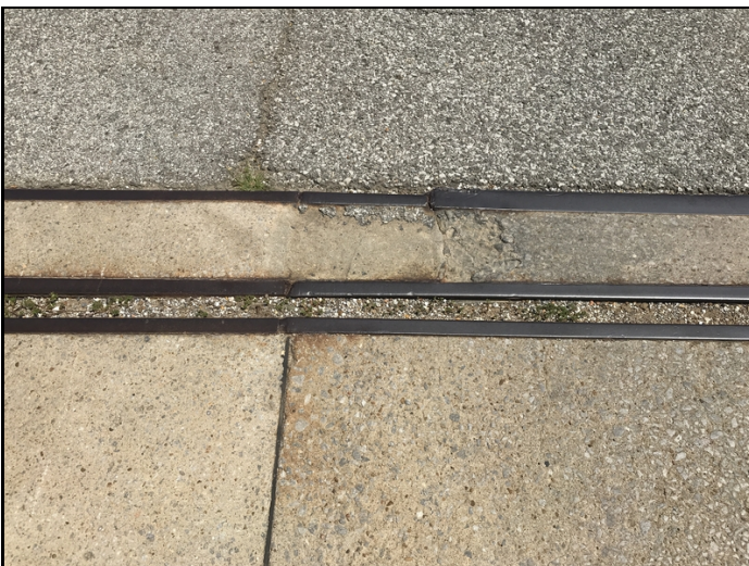
Bent # 1, top of backwall, cracked weld in the angle.
