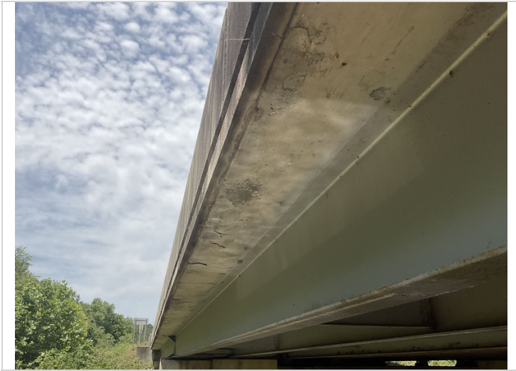
Span # 6 Lt overhang of the deck with numerous concrete delaminations.
