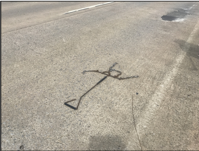
Both wheel paths of the right outside lane of span # 5 has large delaminated areas.
