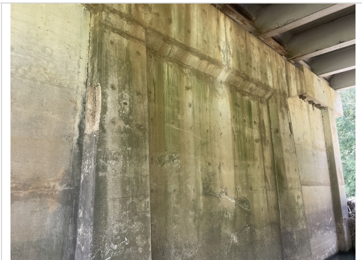
Bent # 6 column # 2 & 3 spalling with exposed reinforcing steel.
