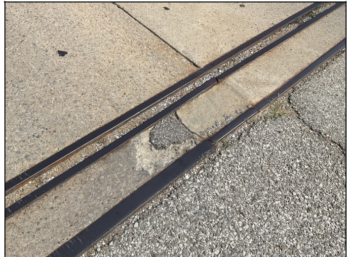
Abutment # 1 Southbound lane cracked weld.
