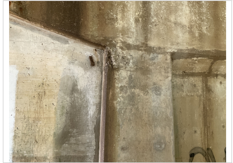
Bent # 3, column # 2 Lt edge of the backface has has concrete deterioration and cracking at the cap juncture.
