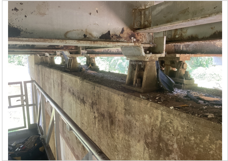
Bent # 4 fixed bearings with active corrosion and pack rust forming.
