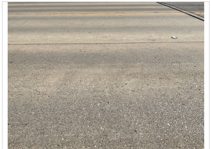
Sealable deck cracking.
