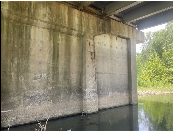
Bent # 6, column # 3 backface has a 10' tall spall with exposed reinforcing steel. The exposed reinforcing steel has active corrosion and pack rust.
