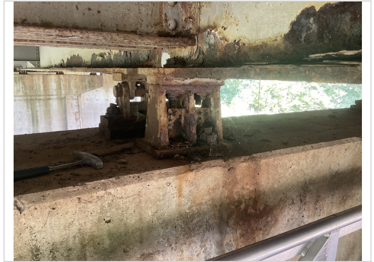
Bent # 5 bearing # 5 active corrosion with pack rust.
