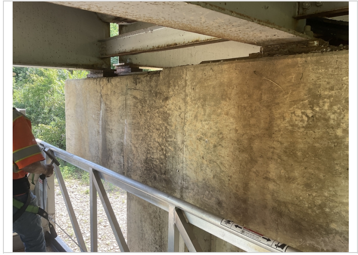
Bent # 4 Rt aheadface end of the cap under bay # 8 has a 5' long area of vertical and horizontal cracks with delaminated concrete and light efflorescence buildup in the vertical face of the cap.
