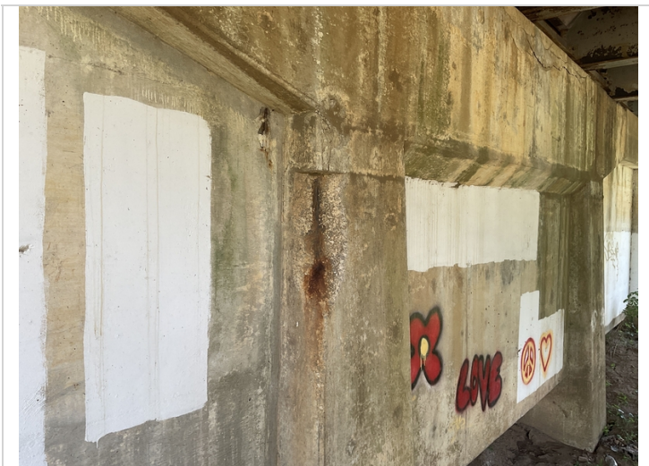
Bent # 3, column # 3 aheadface has a 4.5' tall spall with exposed reinforcing steel. Exposed reinforcing steel has initial section loss.
