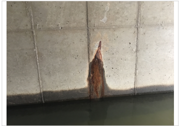
Exterior wall barrel 1, rust staining.
