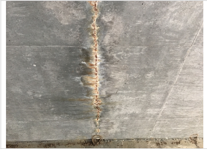
Barrel 4 soffit, rust staining and efflorescence.
