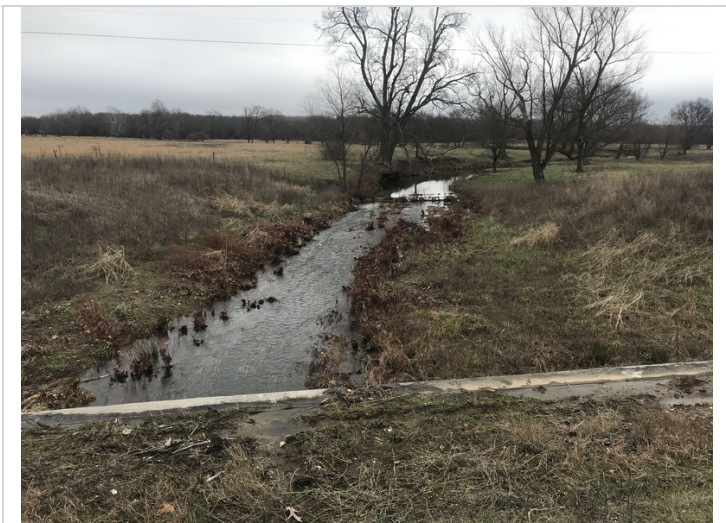
Upstream channel, inlet end of barrels 4 and 5, the channel has silted in.
