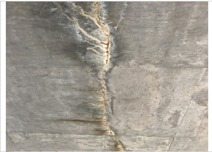
Barrel 1 soffit, rust staining and efflorescence.
