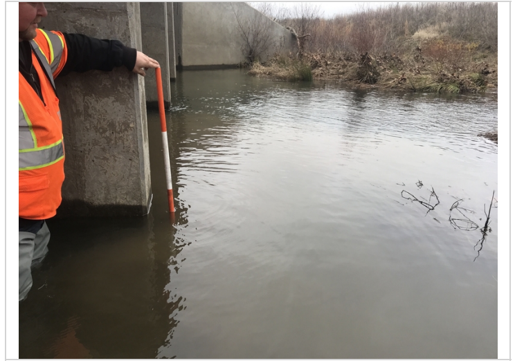
Inlet end at barrel,3, scour
