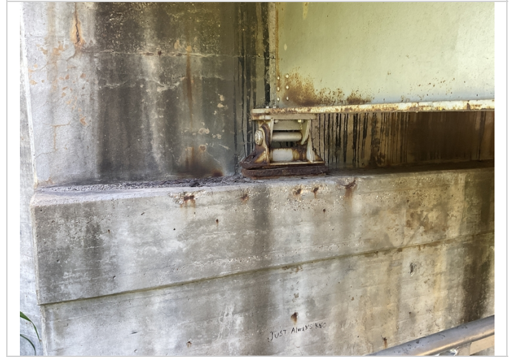
Abutment #1 Rt spalling with exposed reinforcing steel.
