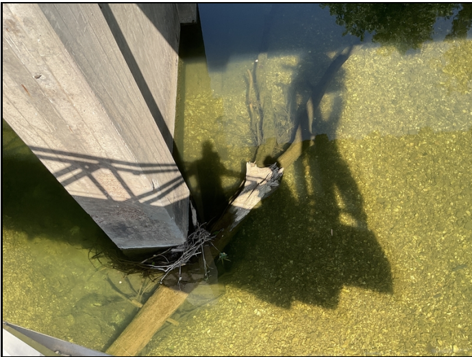
Bent #2 drift accumulation.
