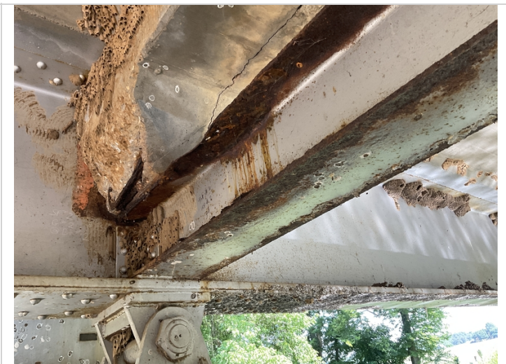
Bent #2 Rt diaphragm holes in the flange.
