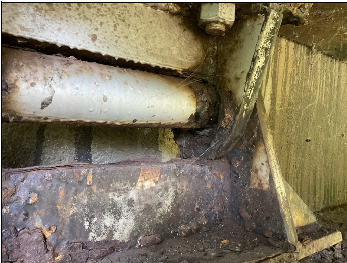
Abutment #2 bearing #1 active corrosion with pack rust and significant section loss to the bearing and pin.
