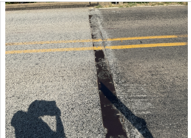
Abutment #1 assembly joint .
