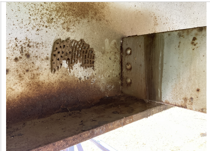
Span #1 girder #1 interior diaphragm connection with 1/16" section loss to the base of the web.
