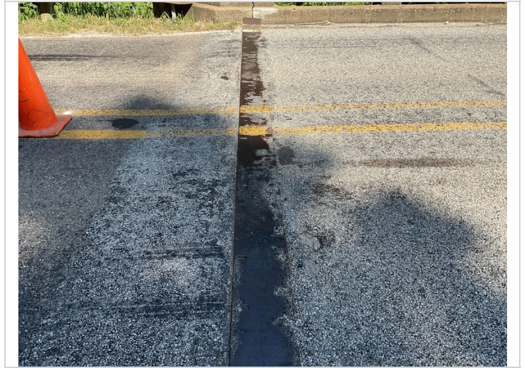
Abutment #2 assembly joint.
