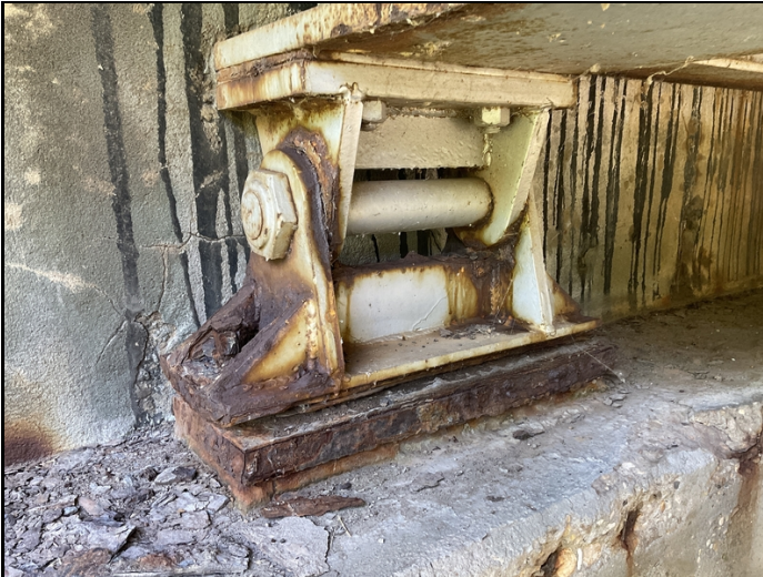
Abutment #1 Rt bearing active corrosion with pack rust.
