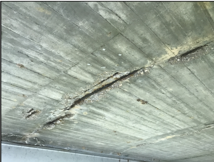
Span 3 undersurface-Spalling with exposed reinforcing steel.
