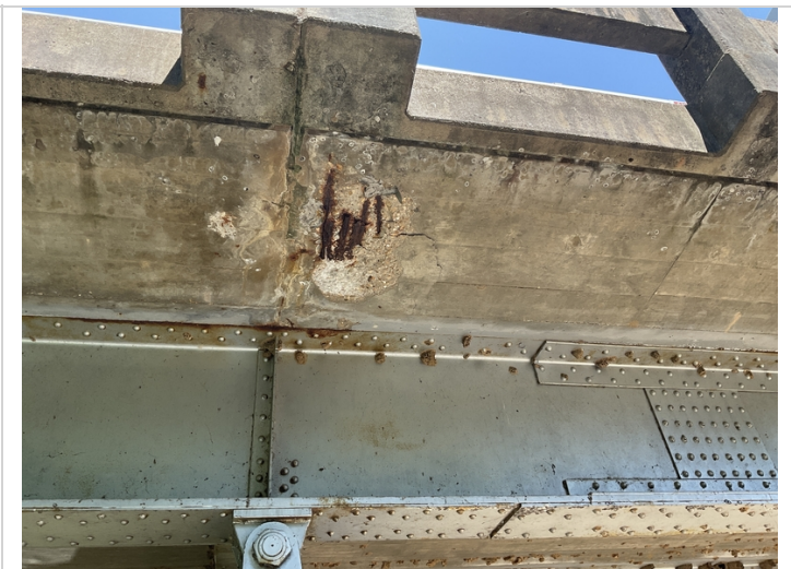
Span #2 Lt spalling with exposed reinforcing steel.
