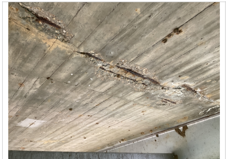
Span #3 undersurface spalling with exposed reinforcing steel.
