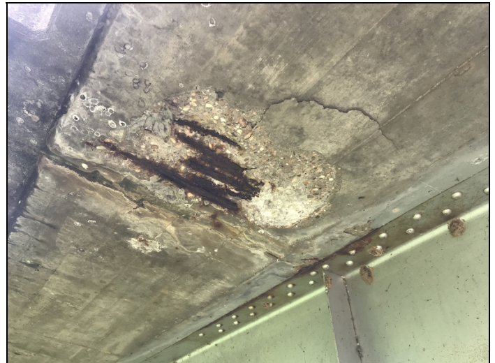
Span 2, left side over bent 3-Spalling with exposed reinforcing steel in deck overhang.
