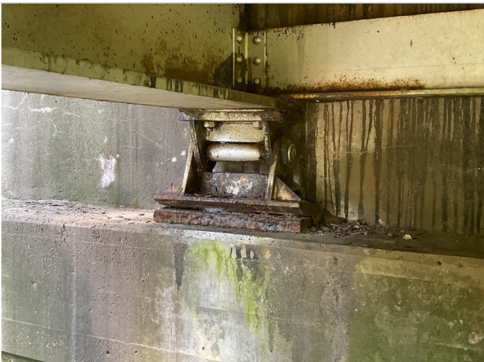
Abutment #2 bearing #1 active corrosion with pack rust.
