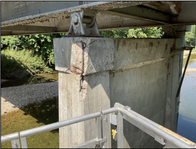
Bent #2 Lt spalling with exposed reinforcing steel.
