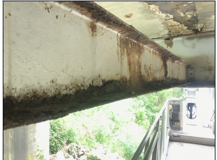
Span 1, diaphragm # 2-Corrosion with section loss.
