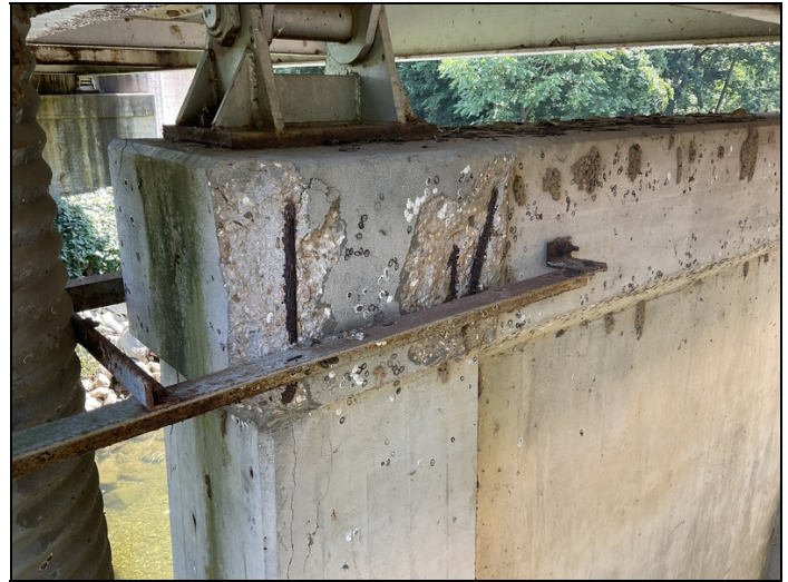
Bent #2 Rt aheadface spalling with exposed reinforcing steel.
