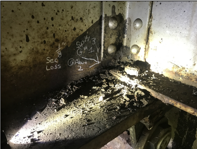
Span # 3, girder # 1 has corrosion to the interior side of web at the diaphragm connection with up to 1/8" section loss. Photo 2.
