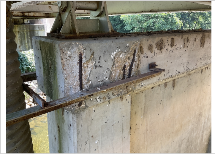
Bent #2 Rt aheadface spalling with exposed reinforcing steel.
