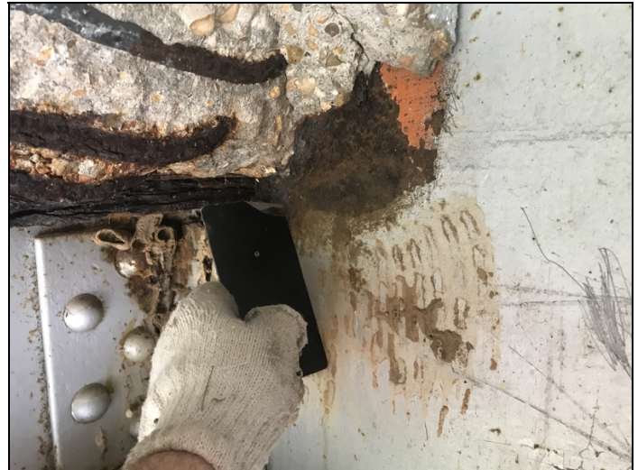
Span # 2, girder # 2 over bent # 3 has corrosion with up to 5/16" section loss to interior side of web at expansion dam juncture.
