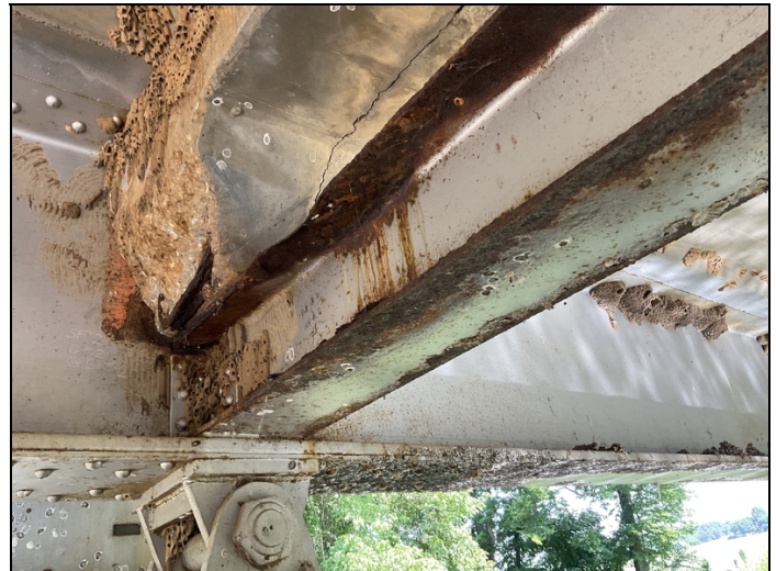
Bent #2 Rt diaphragm holes in the flange.
