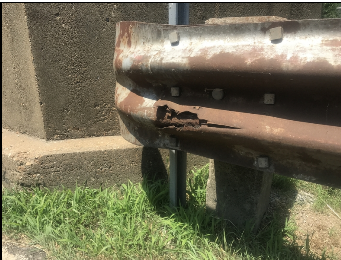
The Northwest approach railing has collision damage that has created sharp jagged edges in the railing near the bridge end.
