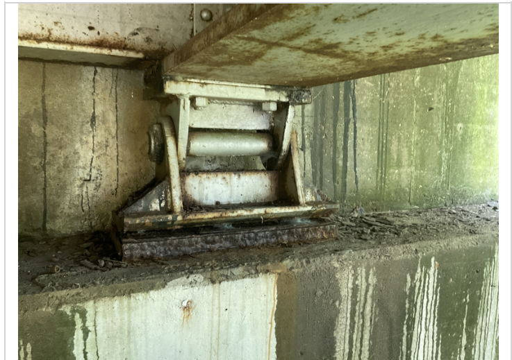
Abutment #2 bearing #2 active corrosion with pack rust.
