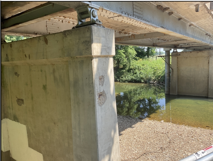
Bent #3 Lt spalling with exposed reinforcing steel.
