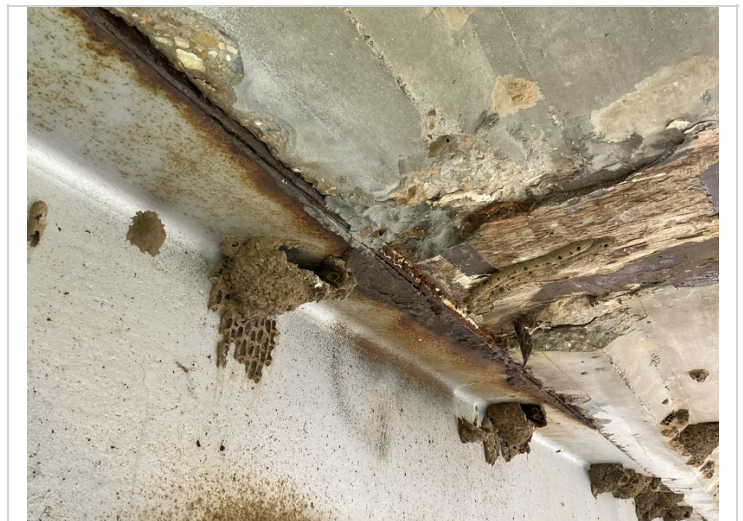
Span #1 Lt top flange active corrosion with pack rust and section loss.
