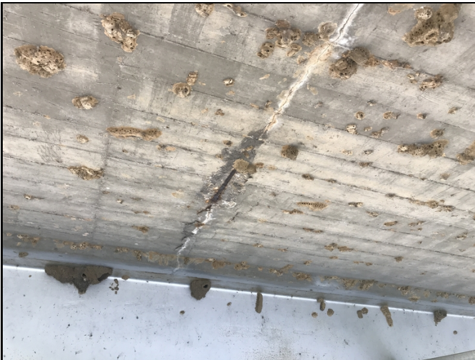
Span 2-Spalling with exposed reinforcing steel.
