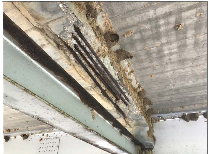
Expansion dam over bent 2-Spalling with exposed reinforcing steel.
