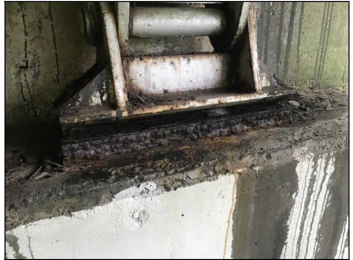
Abutment # 2-Corrosion to bearings.
