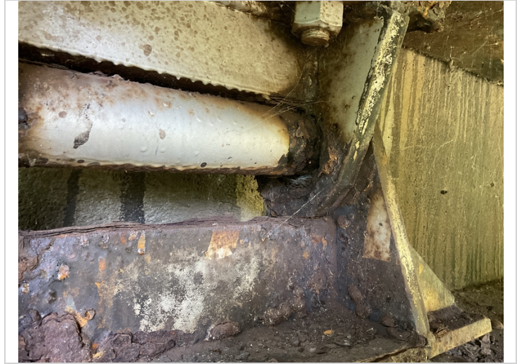
Abutment #2 bearing #1 active corrosion with pack rust and significant section loss to the bearing and pin.
