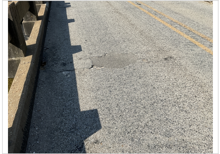
Span #1 temporary asphalt repair.
