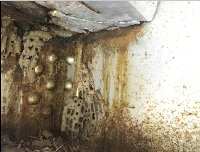
Girder 1 over bent 2-Approximately 1/16" section loss to web.
