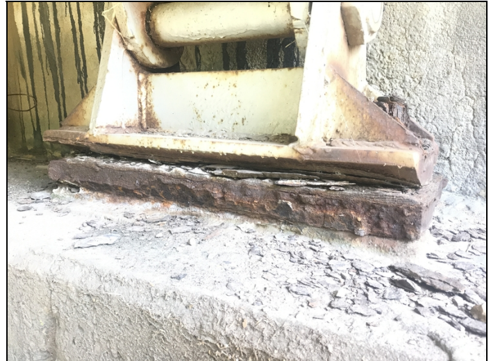
The expansion bearings have active corrosion, layers of rust, and section loss between the masonry plates and the rockers.
