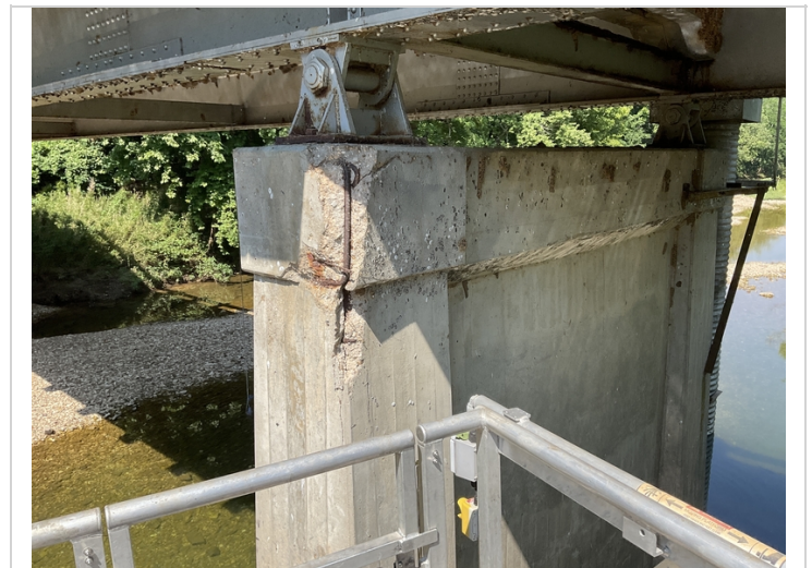
Bent #2 Lt spalling with exposed reinforcing steel.
