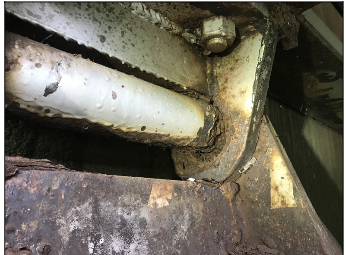
The rocker bearing pins at connections at abutment # 2 have corrosion with significant section loss. The pin at bearing # 1 is the most extreme with up to approximately 1/4" section loss.
