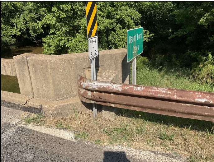
Northwest approach guardrail collision damage.
