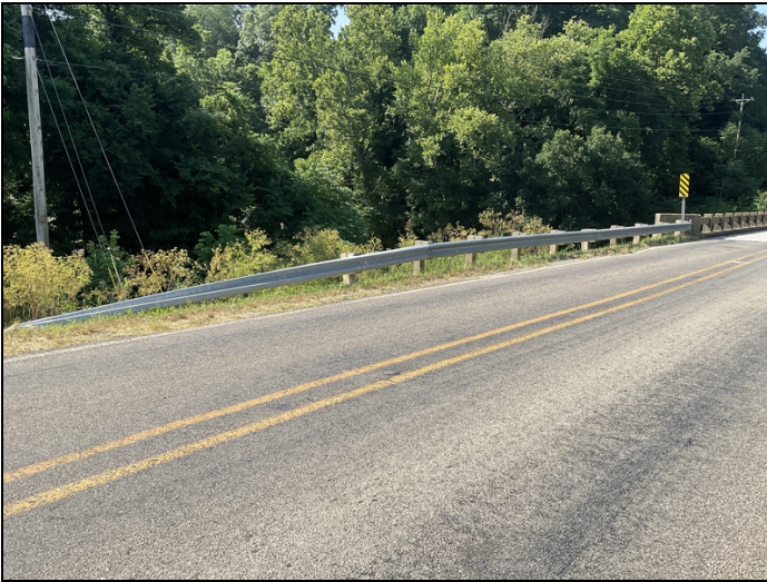
Northeast approach guardrail has been replaced.
