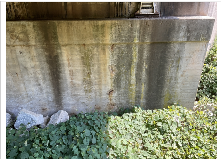
Abutment #1 Lt spalling with exposed reinforcing steel.
