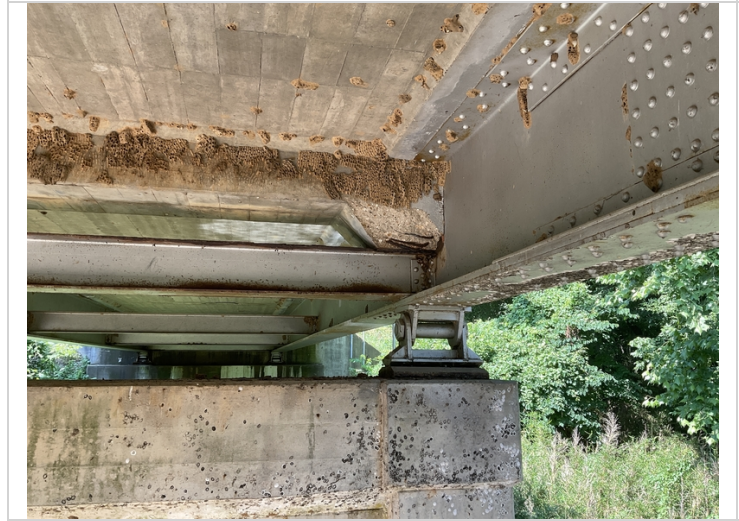
Bent #3 backface spalling with exposed reinforcing steel in the deck haunch.
