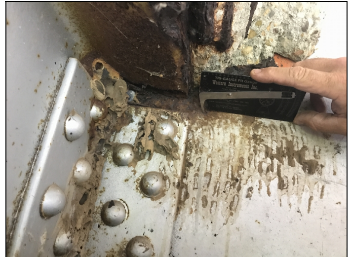
The web of girder # 1 over bent # 3 has up to 5/16" section loss adjacent to the expansion dam.
