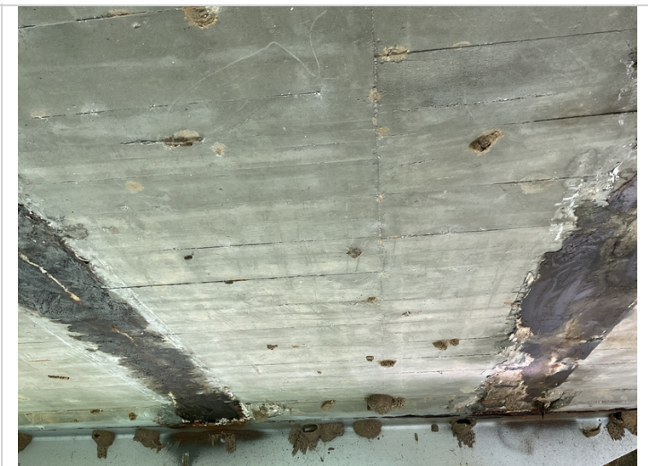
Span #1 transverse cracking repair.
