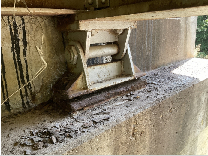
Abutment #1 Lt bearing active corrosion with pack rust.
