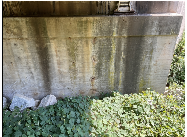
Abutment #1 Lt spalling with exposed reinforcing steel.
