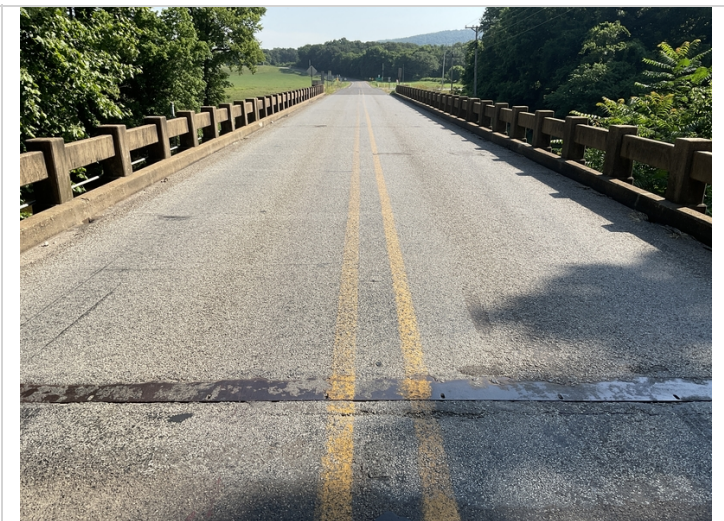
Typical driving surface of the deck.
