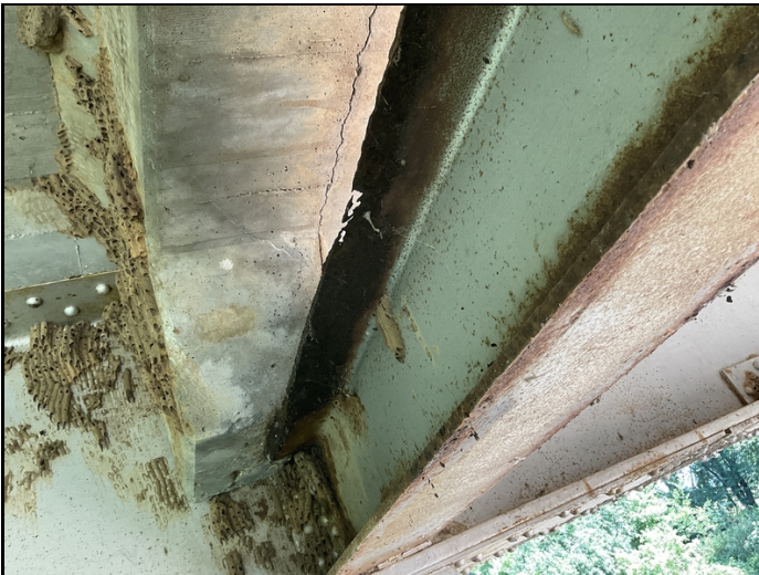
Bent #3 Rt diaphragm with active corrosion and 100% section loss along the top flange.
