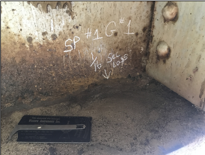
Girder # 1 of span # 1 has approximately 1/16" section loss to base of web located adjacent to diaphragm # 2 connection.
