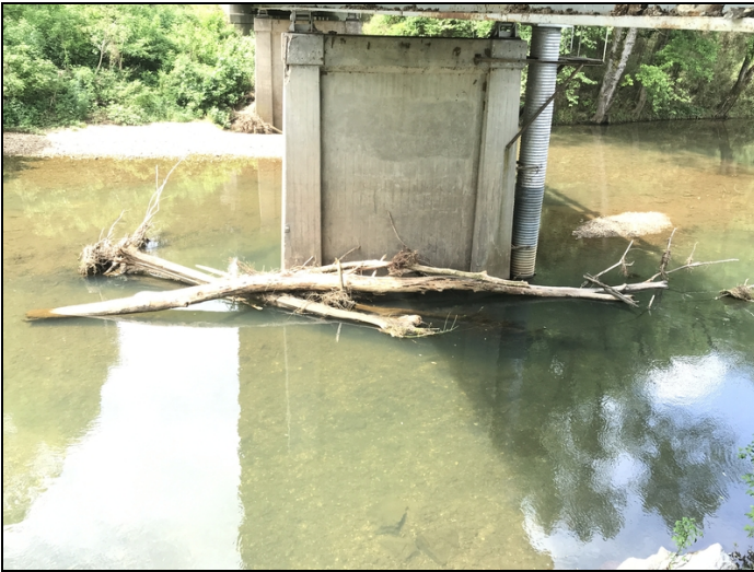
Drift accumulation at bent # 2.
