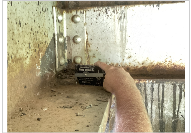
Span 3 girder 1 at abutment 2-Section loss to bottom flange
