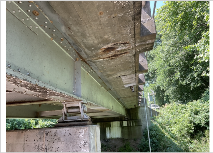
Span #2 & 3 Rt overhang spalling with exposed reinforcing steel.
