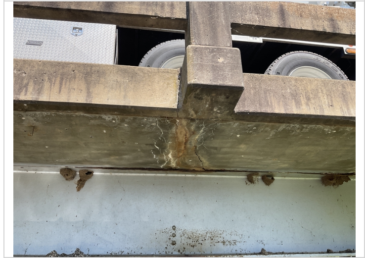
Span #1 Lt transverse cracking under the wheel path over girder #1.
