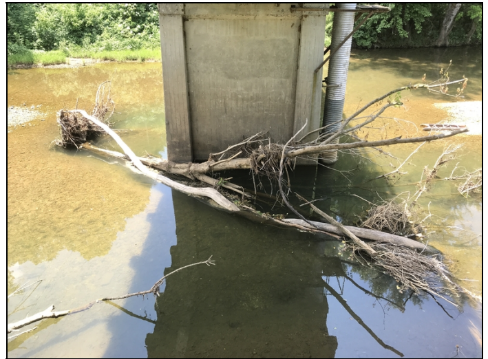
The channel has drift accumulation at bents # 2 and # 3.
