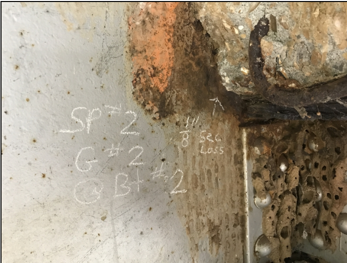
Span 2, girder 2 at bent # 2 has 1/8" section loss to interior side of web at deck haunch juncture.
