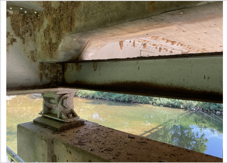
Bent #3 Rt diaphragm with active corrosion and section loss.
