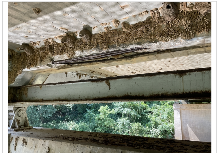
Bent #2 deck haunch spalling with exposed reinforcing steel.
