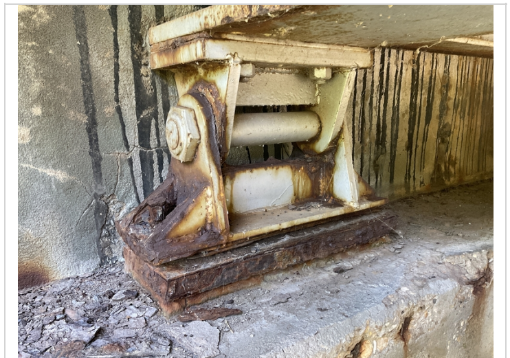
Abutment #1 Rt bearing active corrosion with pack rust.
