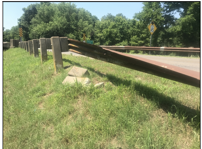
The Northeast approach railing has collision damage that has broken the post that supports the turndown portion of the railing.
