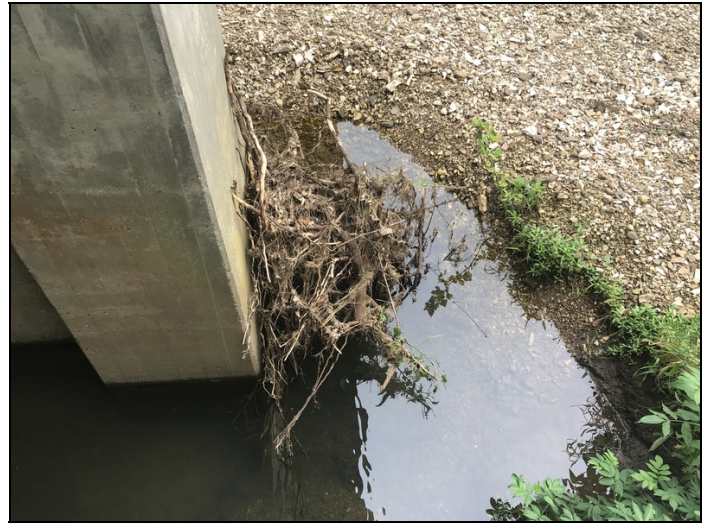
Drift accumulation at bent # 3.
