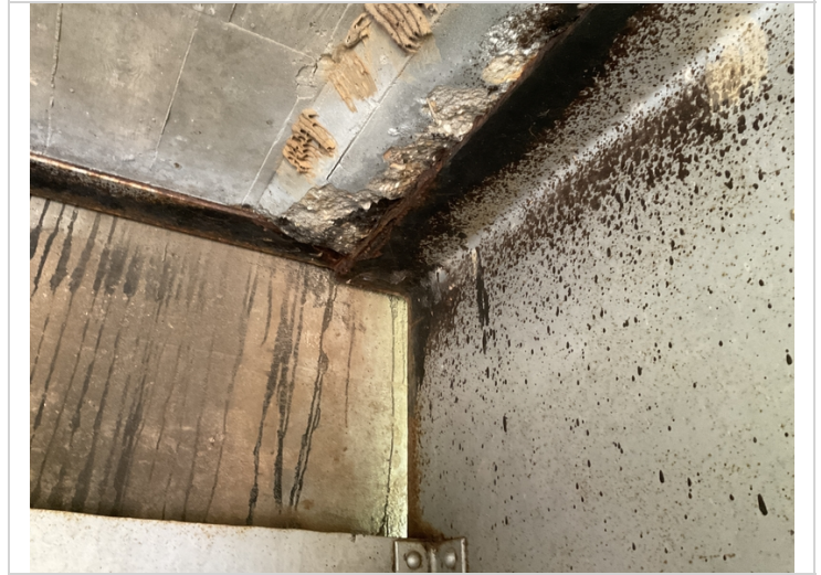
Span #3 Girder #2 @ Abutment #2 active corrosion with pack rust along the top flange.
