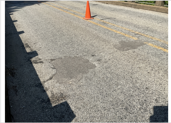
Temporary asphalt patches on the driving surface.
