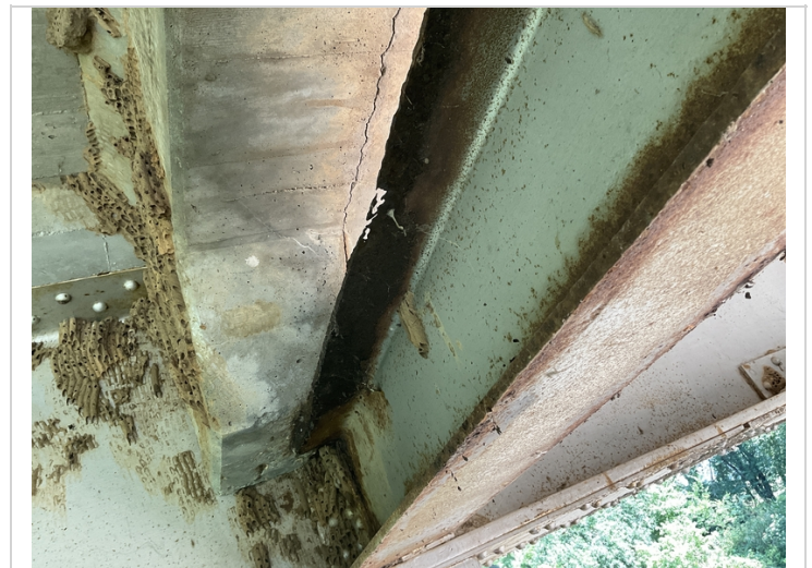
Bent #3 Rt diaphragm with active corrosion and 100% section loss along the top flange.
