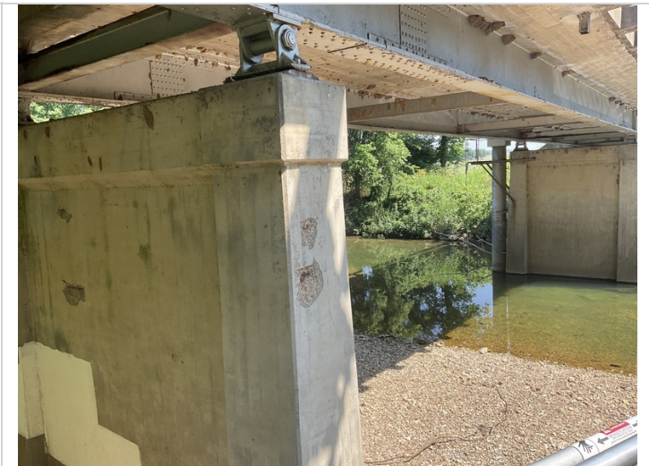
Bent #3 Lt spalling with exposed reinforcing steel.
