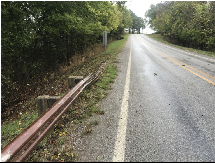
Abutment #2 Lt approach guardrail damage.
