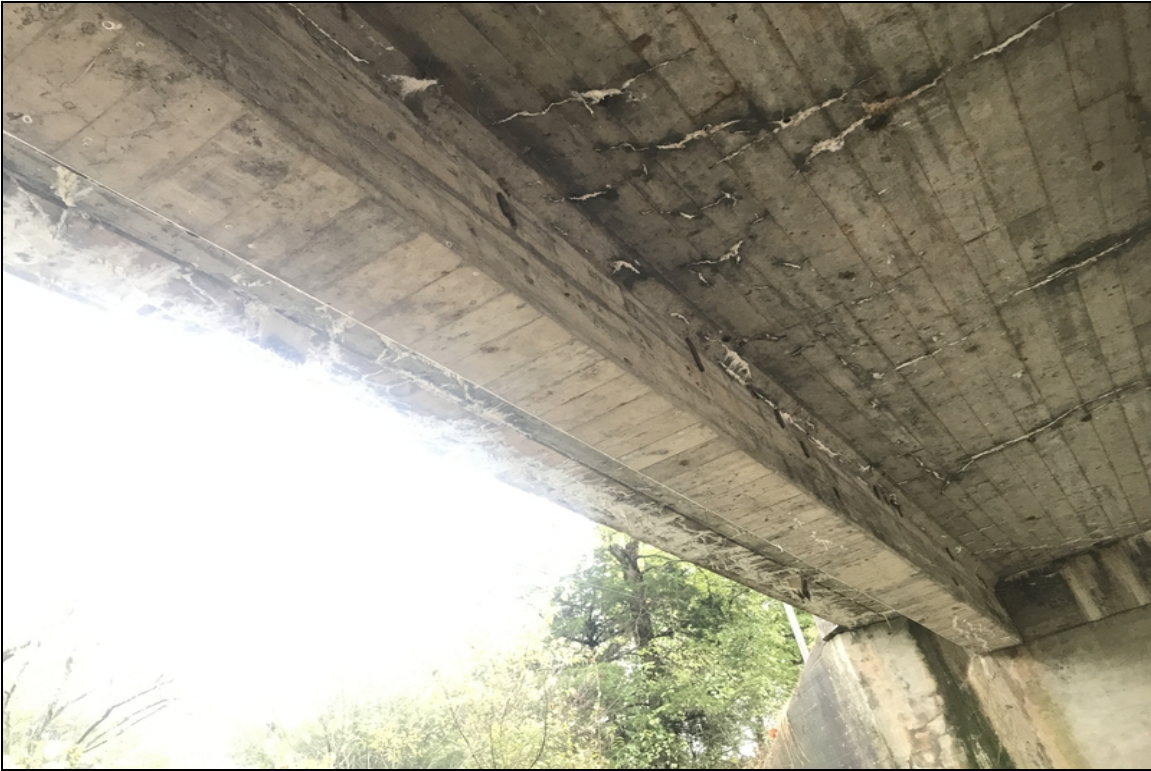
Girder #1 cracking with efflorescence buildup.
