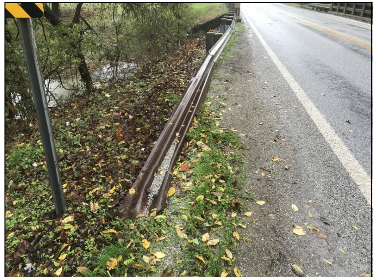
Southwest approach guardrail with minor collision damage.
