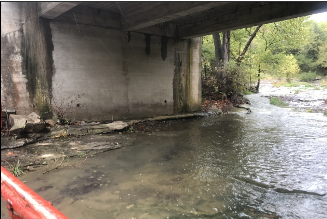
Abutment #1 Lt exposed footing.
