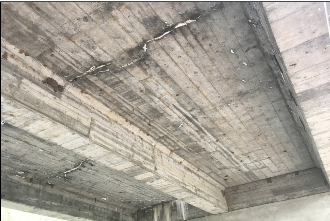
Bay #2 concrete delamination's and spalling with exposed reinforcing steel.
