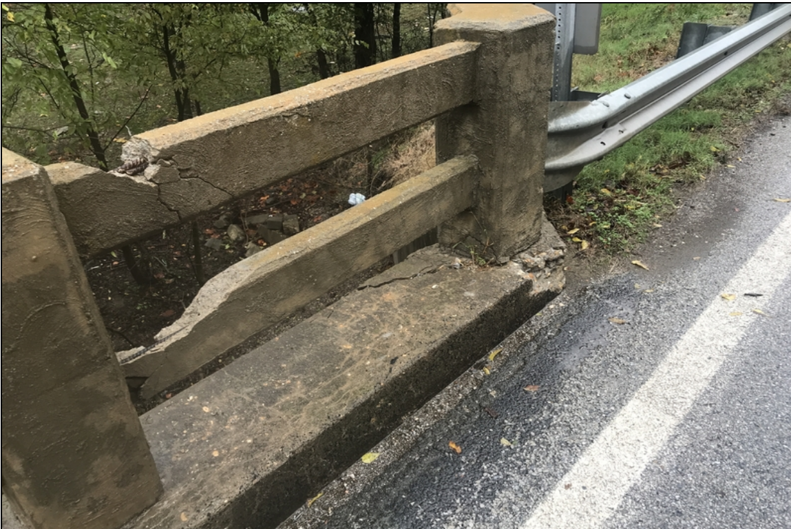
Abutment #1 Rt fractured end post.
