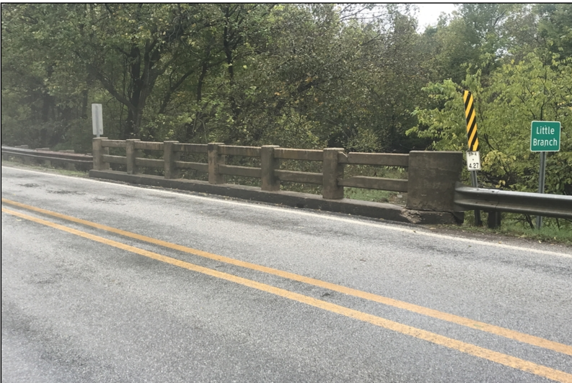
Right bridge rail cracking and spalling with exposed reinforcing steel.
