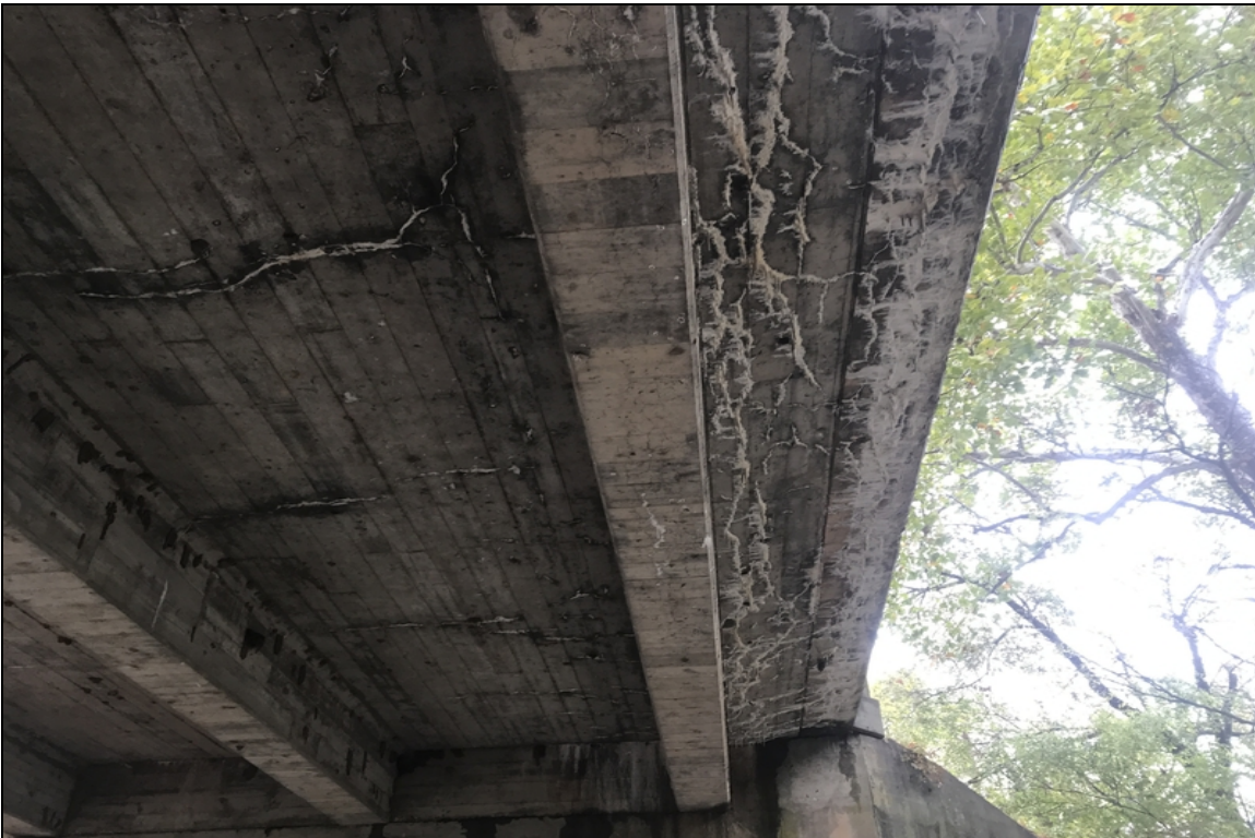
Left overhang and bay #1 cracking with efflorescence buildup.
