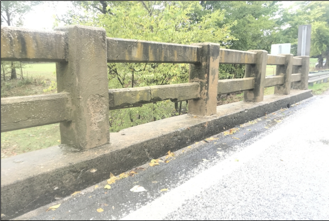
Right bridge rail with exposed reinforcing steel.
