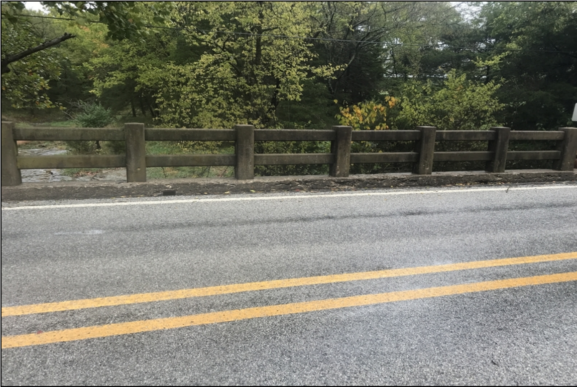
Left curb concrete deterioration.
