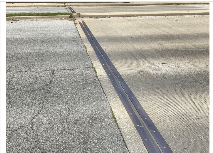
Abutment # 2 joint seal adhesion failure.
