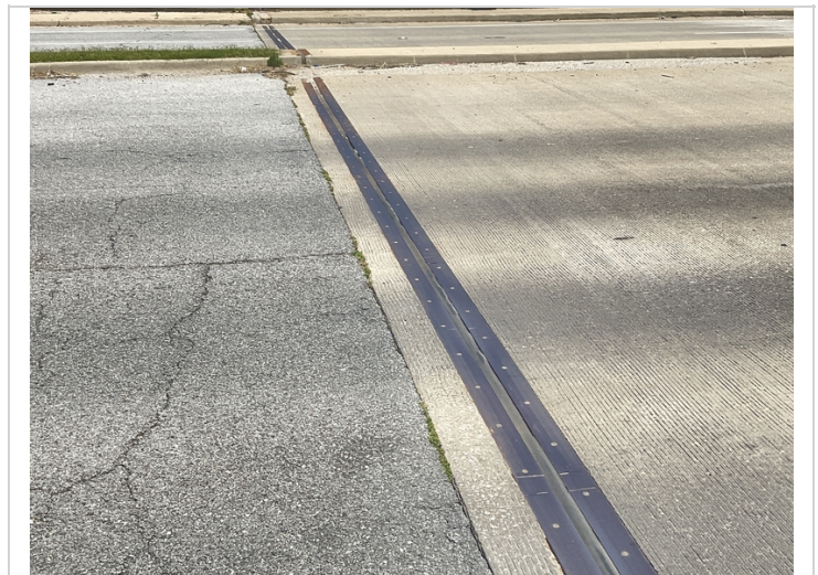
Abutment # 2 joint seal adhesion failure.
