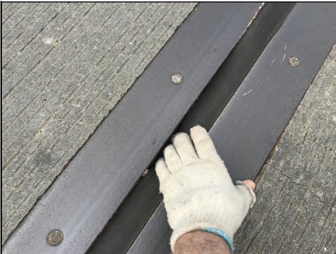
The poured joint sealant at abutment # 2 expansion joint has a few short duration areas of full depth adhesion failure in the Southbound lanes
