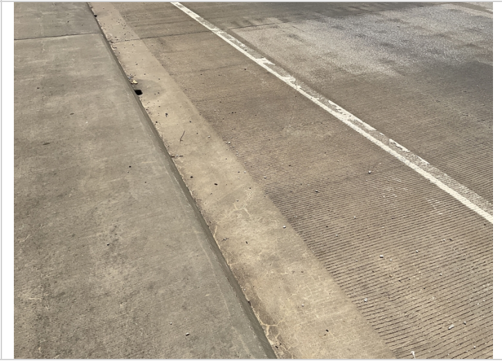
Sealable deck cracking.
