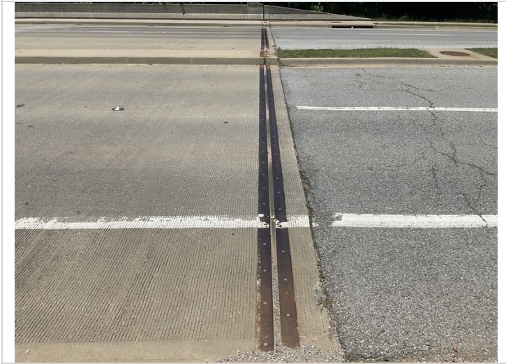
Abutment # 2 typical joint seal.
