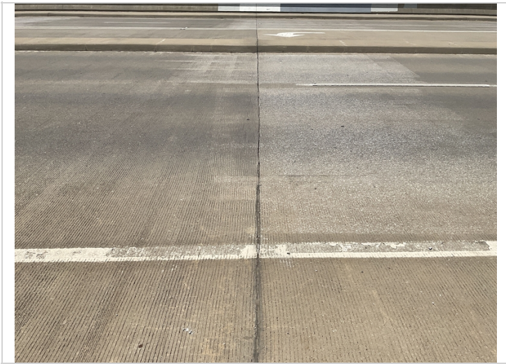
Failing joint sealant.
