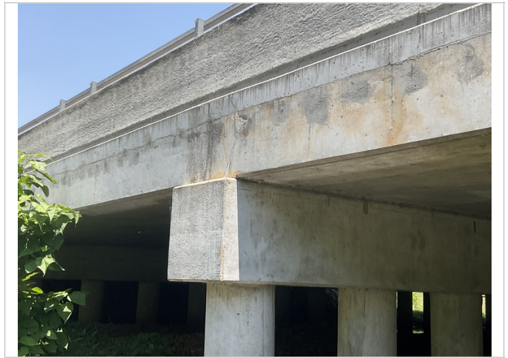
Typical shear type cracking in the edge of the slab over the intermediate bents.
