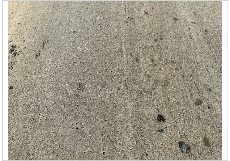
Typical hairline map cracking
