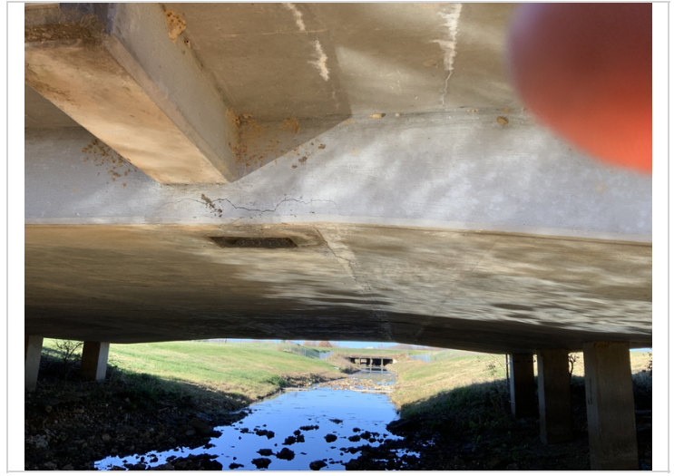
Span 2 Right cracking in edge of deck
