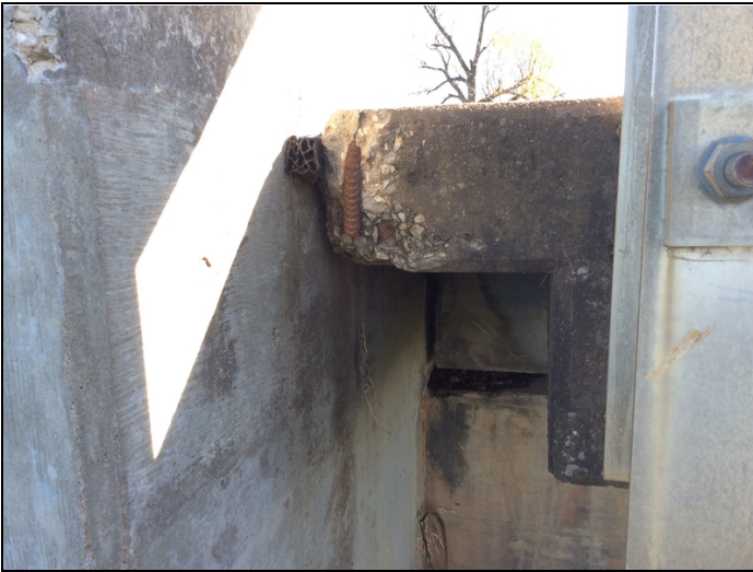
One softball size spall with exposed reinforcing steel at the Northwest edge of deck.
