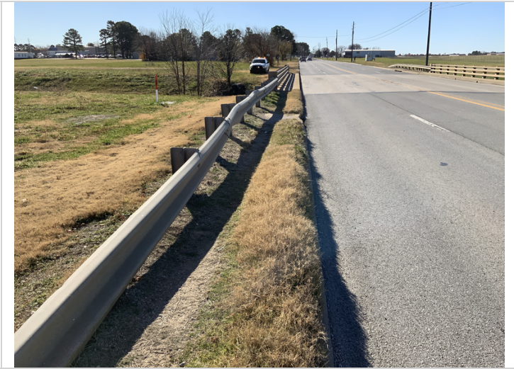
Bent 4 Right minor collision damage to approach bridge railing
