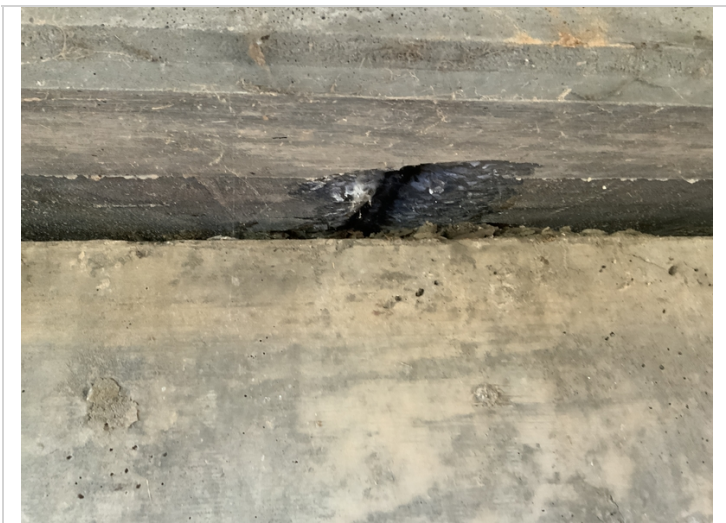
Bent 4 mid span Spalling with exposed reinforcing steel
