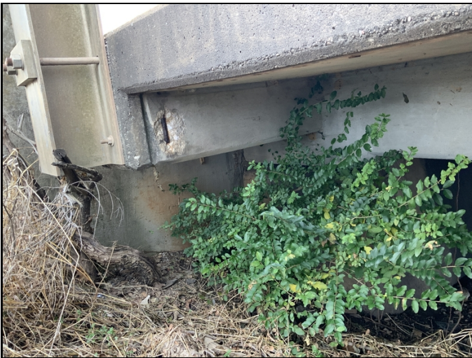
Bent 1 (South Abutment) has spalling with exposed reinforcing steel (Visible from the right side of the structure along the cantilever).
