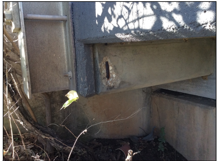
One softball size spall with exposed reinforcing steel at the Southeast edge of deck
