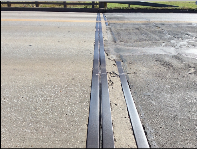
The compression joint seals at the abutments are deteriorated with minor tears on the driving surface and minor adhesion failure that leaks water on the abutments.
