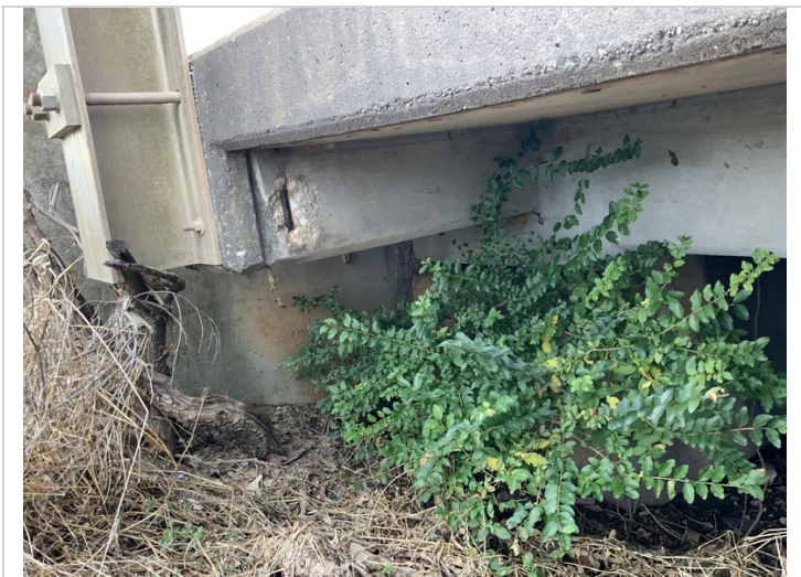
Bent 1 (South Abutment) has spalling with exposed reinforcing steel (Visible from the right side of the structure along the cantilever).
