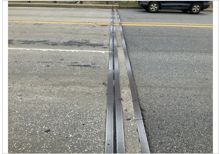
Bent 4 compression joint is cracking and deteriorating. Joints appear to be leaking water on to the abutments.
