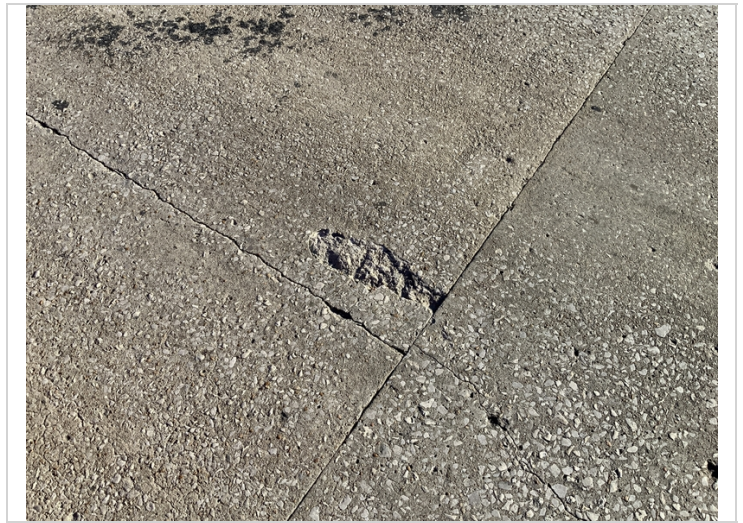
Span 2 Left lane minor Spalling
