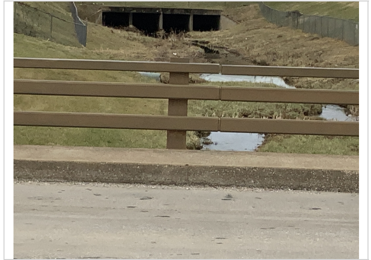
Bent 2 left bridge rail is separated.
