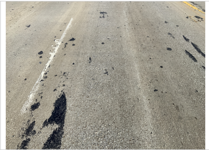
Typical longitudinal cracking
