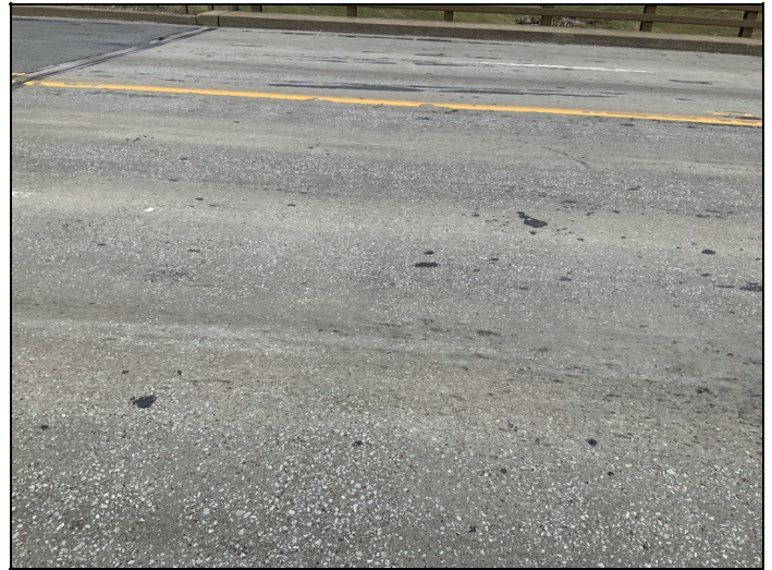
Typical seal-able deck cracking throughout the structure.
