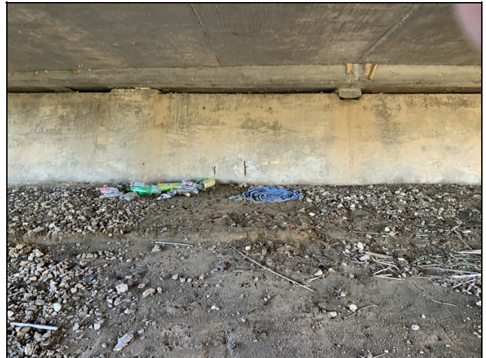
Bent 4 Spalling with exposed reinforcing steel
