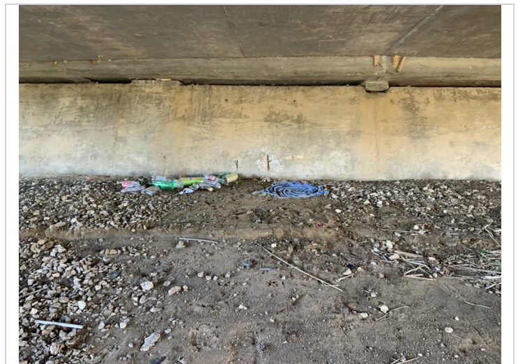
Bent 4 Spalling with exposed reinforcing steel
