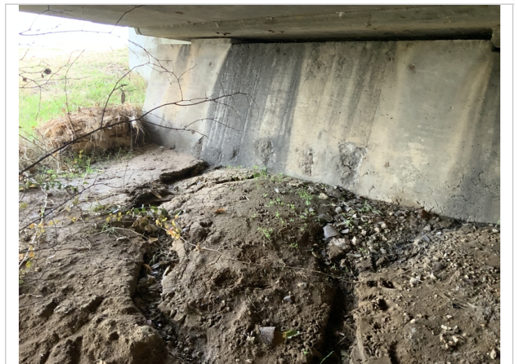
Bent 4 (North Abutment) has 7 spalls with exposed reinforcing steel that has initial section loss at each location.
