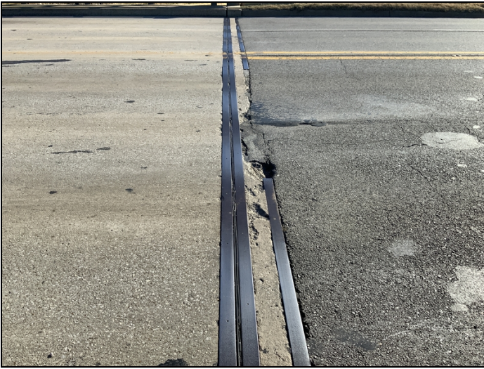
Bent 1 left adhesion failures
