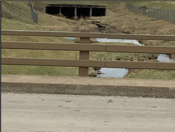
Bent 2 left bridge rail is separated.
