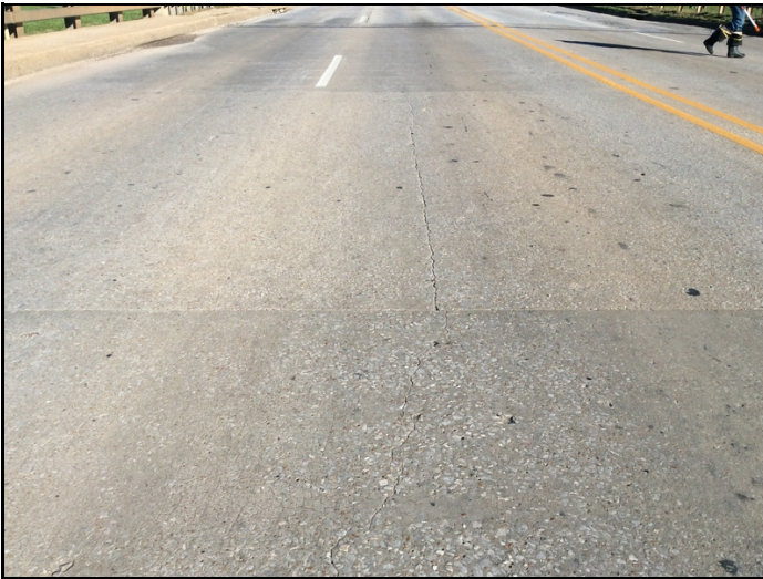
There are sealable map cracks and longitudinal cracks on the driving surface of the deck.
