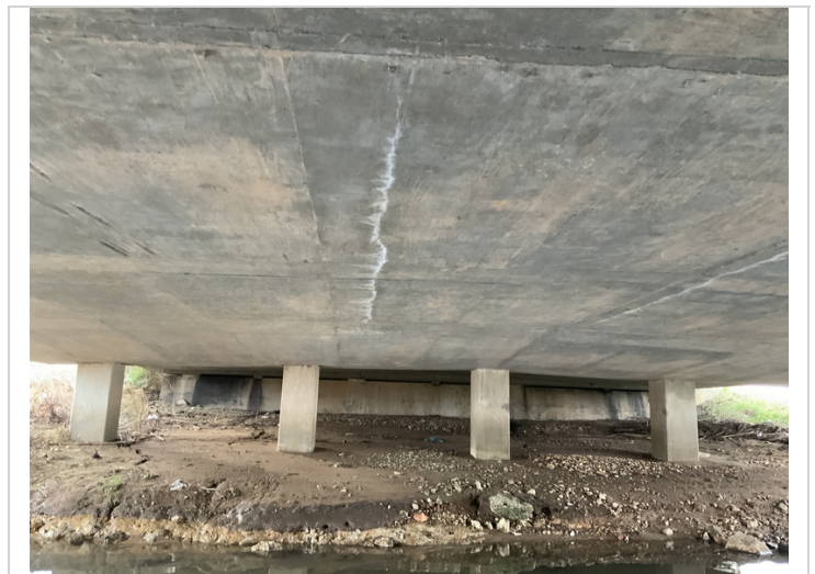
Span 2 has three longitudinal cracking with efflorescence leach through.
