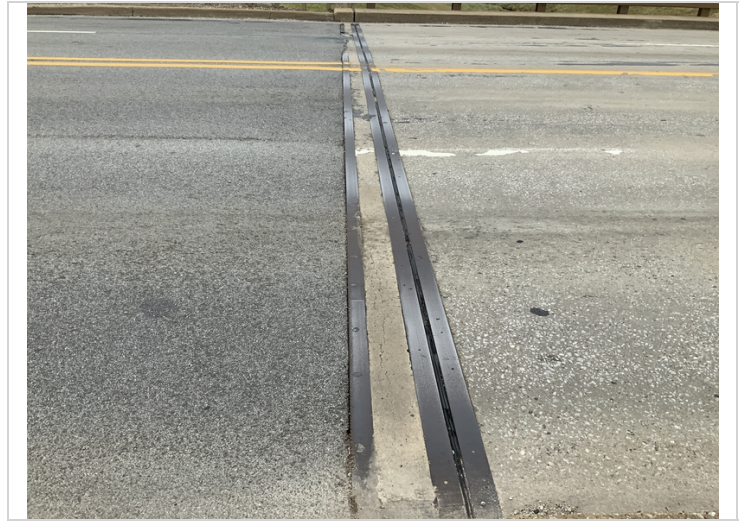
Bent 1 (South Abutment) and Bent 4 (North Abutment) compression joints both have cracking and appear to be leaking.
