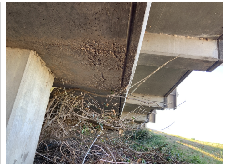
Bent 2 left honeycombing
