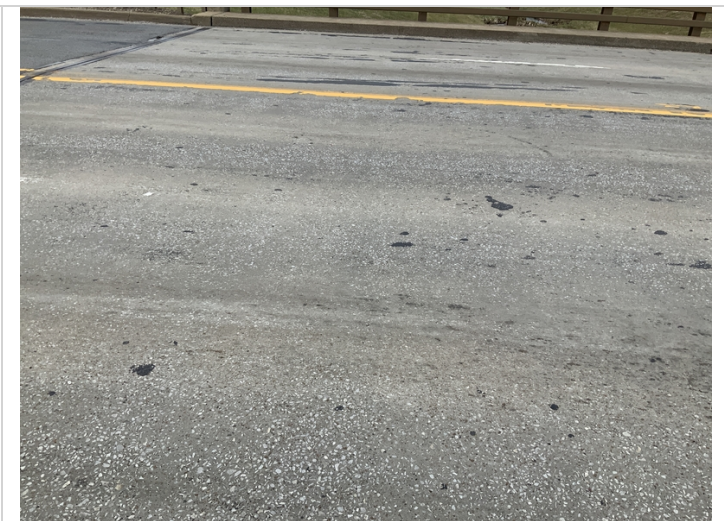
Typical seal-able deck cracking throughout the structure.
