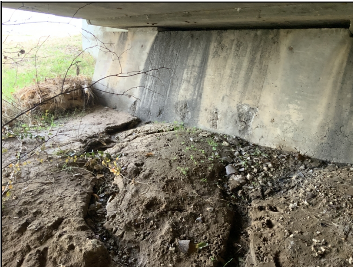
Bent 4 (North Abutment) has 7 spalls with exposed reinforcing steel that has initial section loss at each location.
