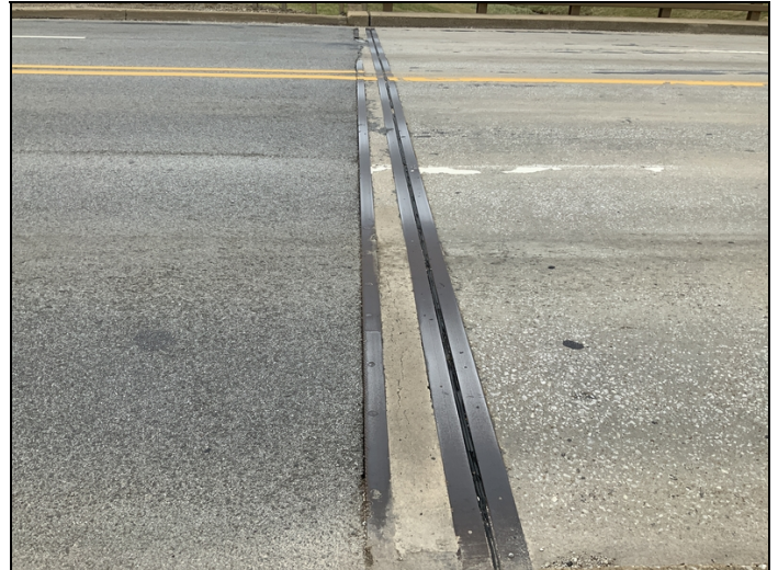
Bent 1 (South Abutment) and Bent 4 (North Abutment) compression joints both have cracking and appear to be leaking.
