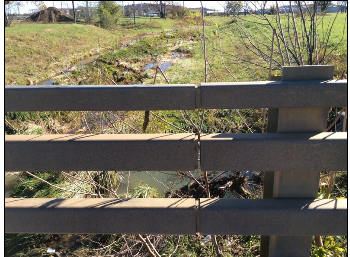
The bridge railing convention joints on the Lt and Rt sides of the bridge are separated.
