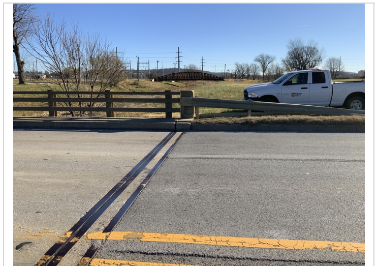
Bent 1 right minor collision damage to approach guardrail
