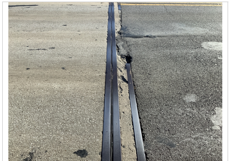
Bent 1 left abut pothole on back wall with approx 12 ft road iron removed
