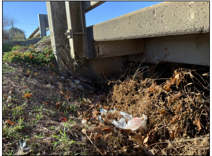
Bent 1 south abutment Spalling with exposed steel
