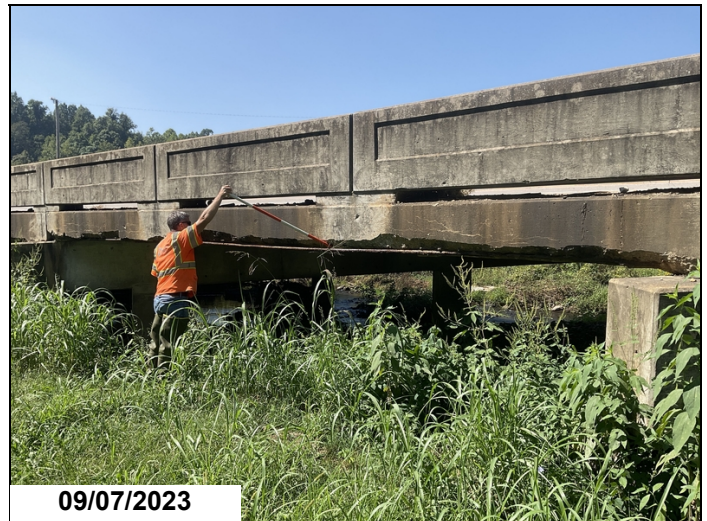
Span # 4 Rt spalling with exposed reinforcing steel.
