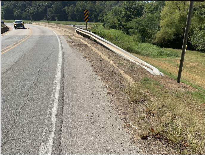
Approach gutters restricted by dirt and debris.
