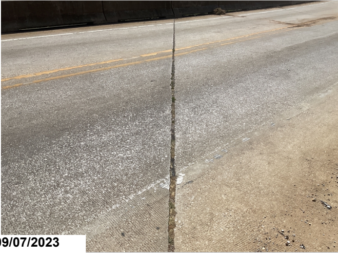
Bent # 5 typical joint seal.
