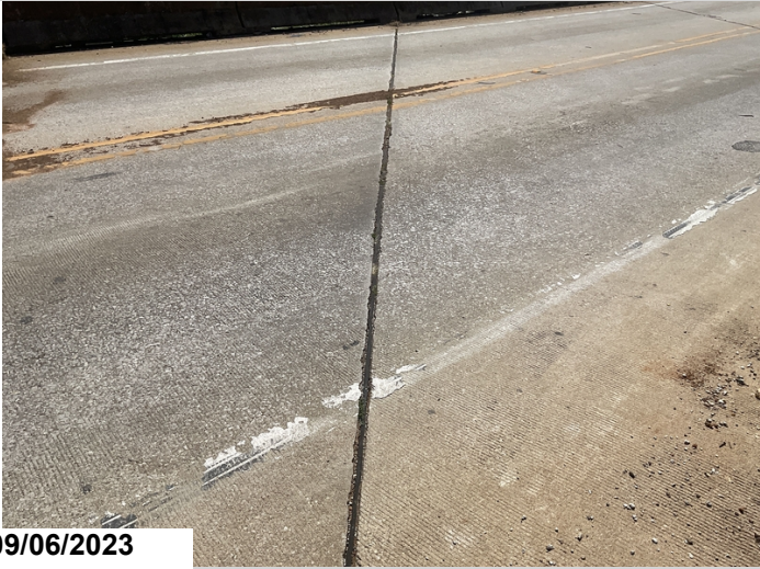
Bent # 4 typical joint seal.
