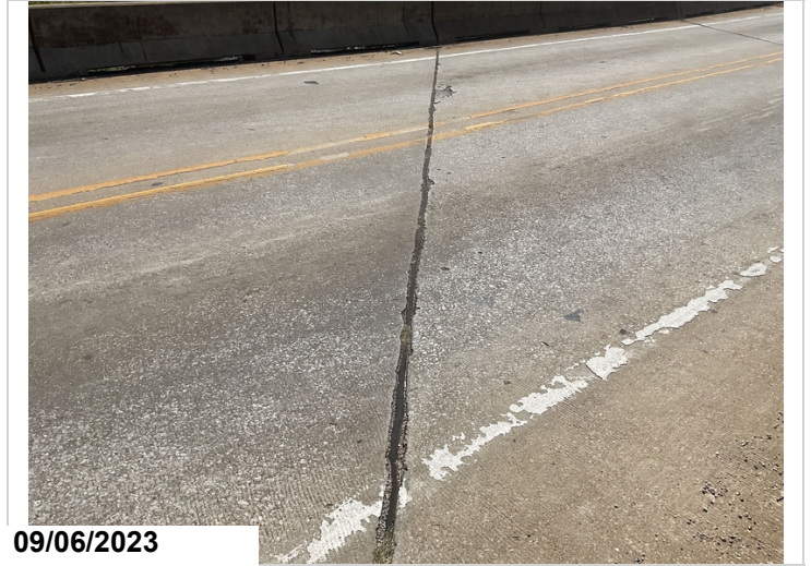
Bent # 3 typical joint seal.
