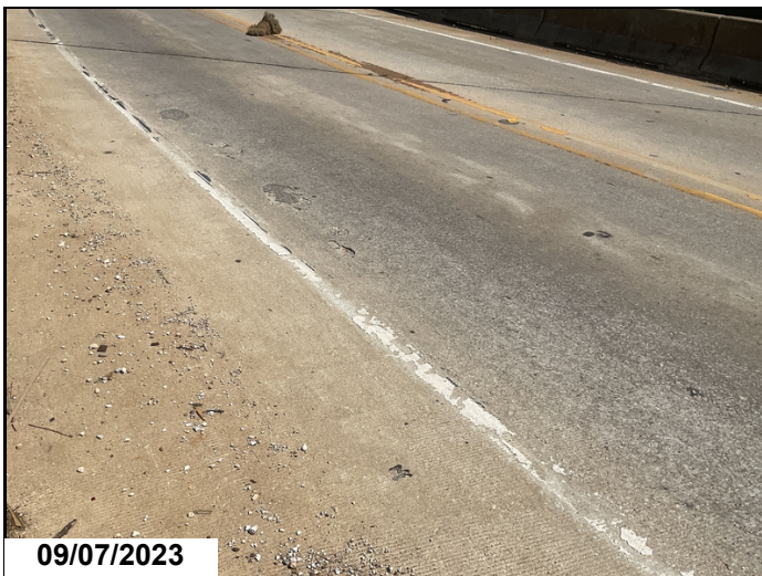
Span # 3 Lt lane spalling and delaminating concrete.
