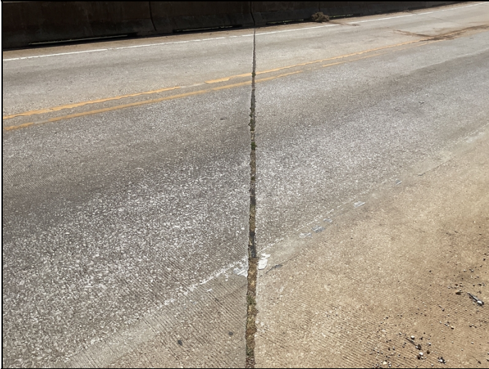
Bent # 5 typical joint seal.
