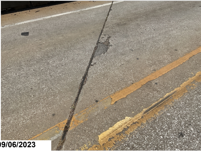
Bent # 3 Span # 2 deck spalling.
