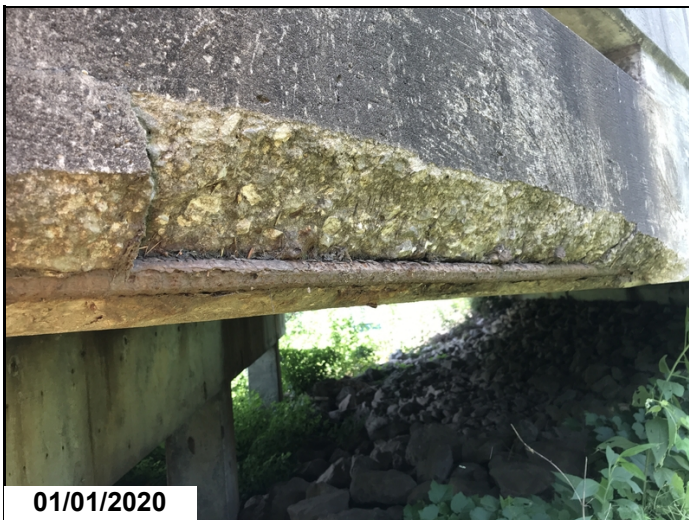
Span # 5-Spalling with exposed reinforcing steel.
