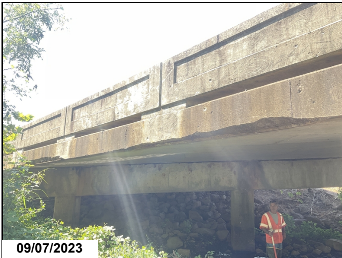
Span # 2 Rt spalling with exposed reinforcing steel.
