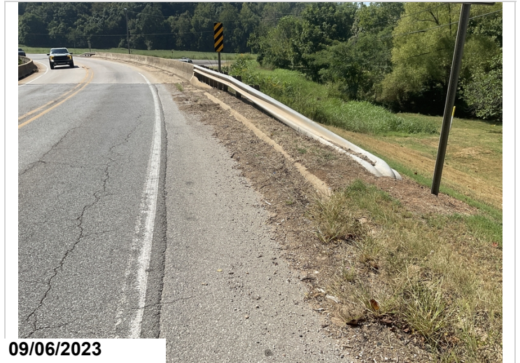
Approach gutters restricted by dirt and debris.
