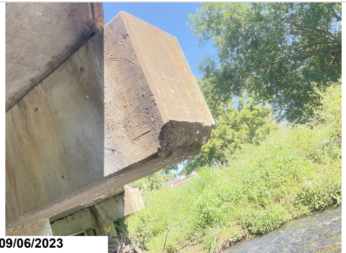
Bent # 3 has a 2' spall with exposed reinforcing steel in the right end of cap.
