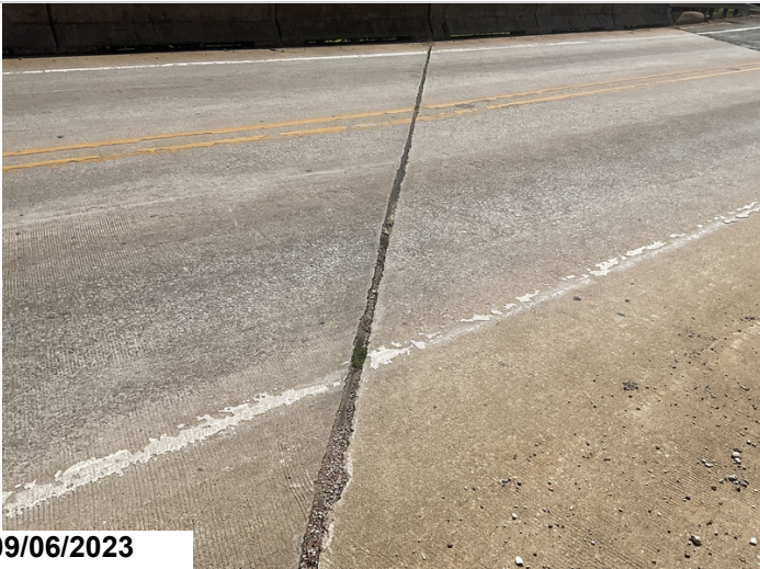
Bent # 2 typical joint seal.
