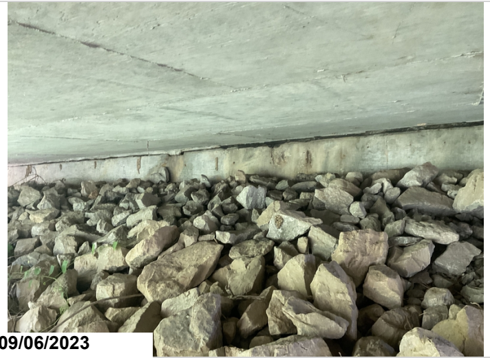
Abutment # 1 spalling with exposed reinforcing steel near the centerline.
