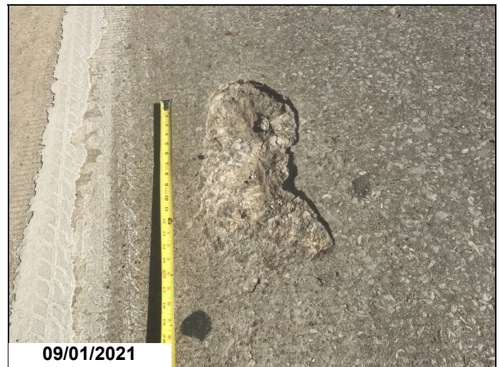
The left lane of span # 3 has delaminated areas in the wheel path with two 15" x 6" spalls that exposed reinforcing steel.
