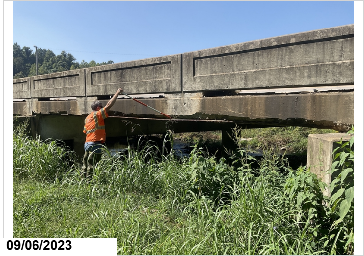
Span # 4 Rt spalling with exposed reinforcing steel.
