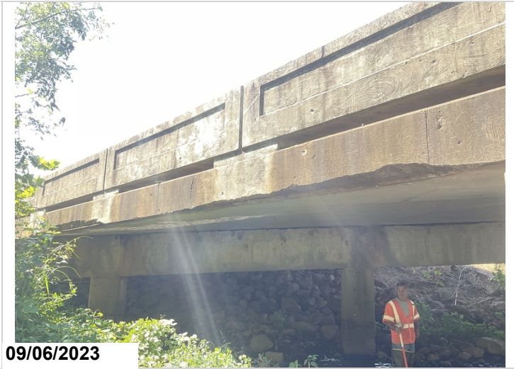
Span # 2 Rt spalling with exposed reinforcing steel.
