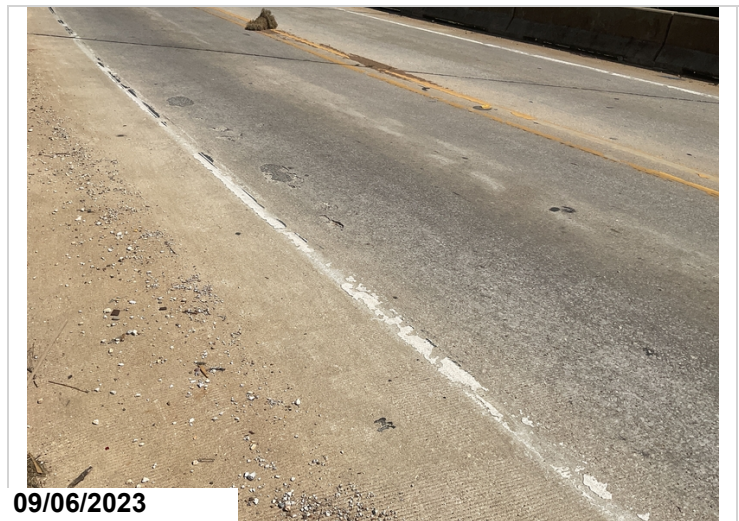
Span # 3 Lt lane spalling and delaminating concrete.
