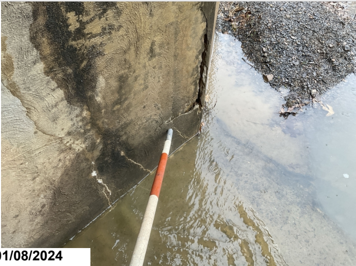
Barrel 1 exterior wall on left side-Delaminated area at wing wall juncture
