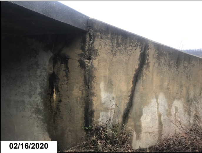
Barrel # 1 exterior wall on left side at the wing wall juncture has spalling that exposes reinforcing steel in the upper portion of the wing wall. The base of wall has a 12" delaminated/ spalled area.
