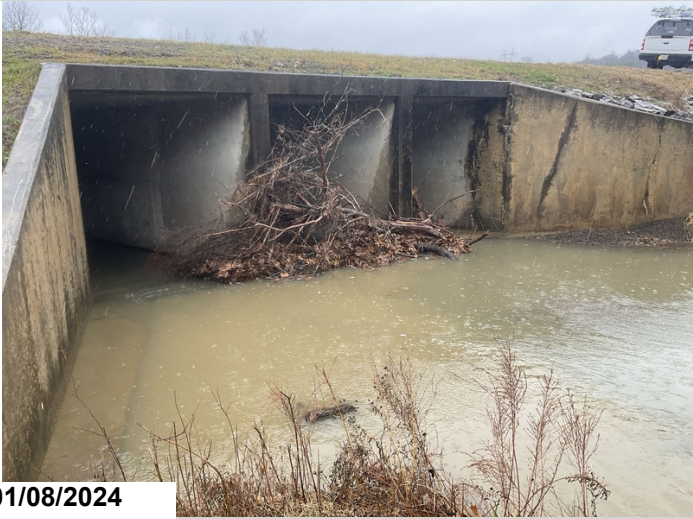
Channel has drift accumulation lodged against the inlet end of culvert that restricts channel flow and promotes additional drift accumulation.
