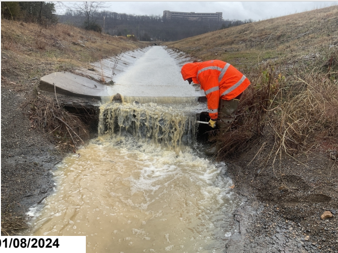
Side drainage ditch paving on Northwest embankment is undermined.
