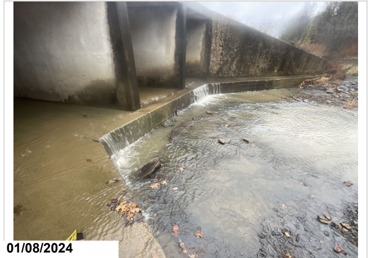
Tow wall exposed on right side
