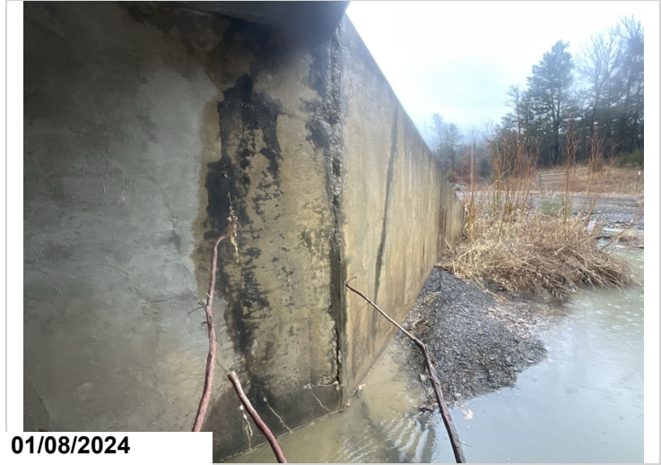
Barrel 1 exterior wall on left side-Spalling with exposed reinforcing steel at wing wall juncture
