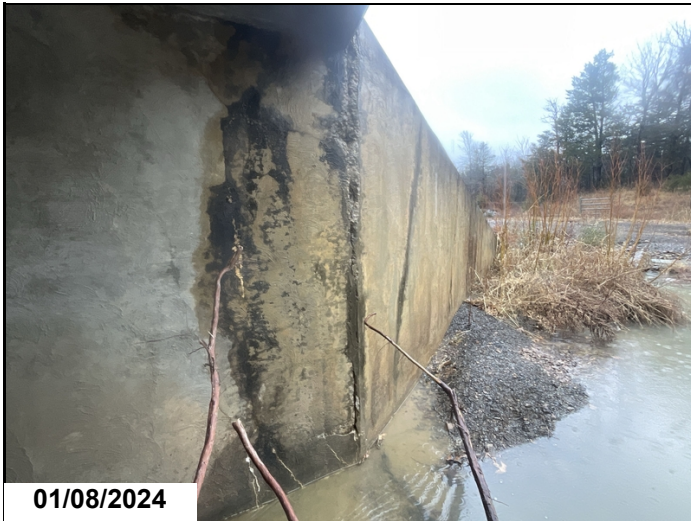
Barrel # 1 exterior wall on left side-Spalling with exposed reinforcing steel at wing wall juncture.
