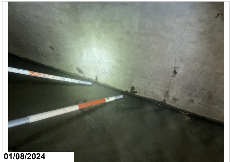
Barrel 3 exterior wall-Shallow spalls with exposed reinforcing steel
