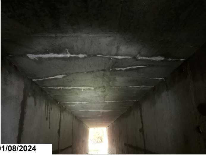
Barrel 1 top slab-Transverse cracks with efflorescence
