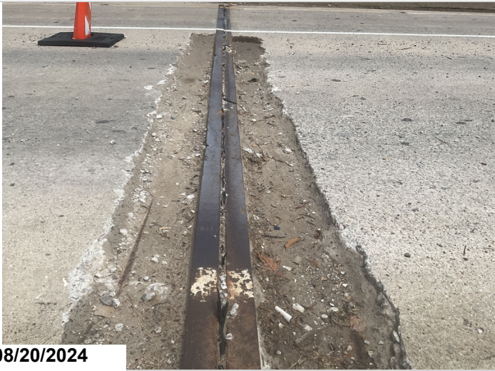
A 12" wide area of the deck has been removed in the outside lanes of the North and south travel lanes adjacent to the expansion joints in preparation for hydro-demolition project. Bent # 6 Northbound Expansion joint pictured.
