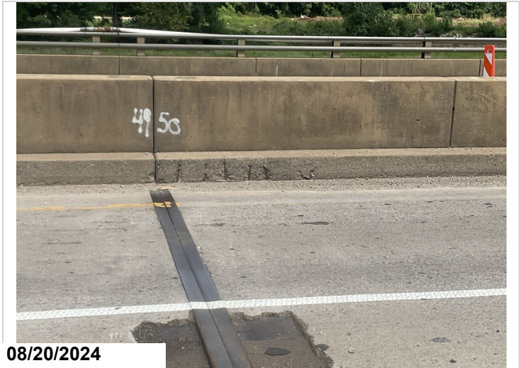
Span # 4, Median Parapet Wall, Adjacent to Bent # 4: Spalls with exposed reinforcing steel. 3LF CS3.
