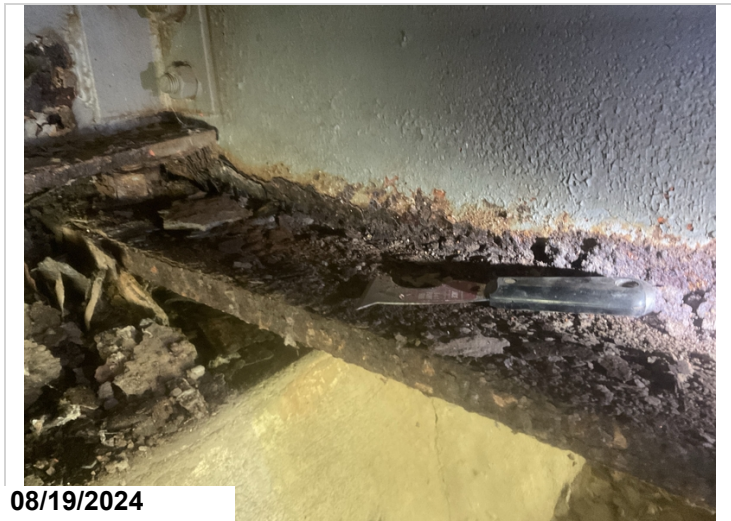
Span # 6, Abutment # 2, Girder # 9: Corrosion / section loss. 3LF CS3.
