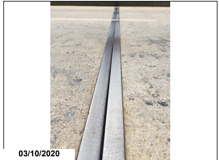
Bent #5 expansion joint seal missing.
