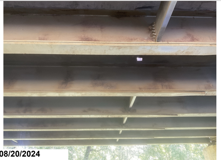
Paint system flaking/ peeling.
