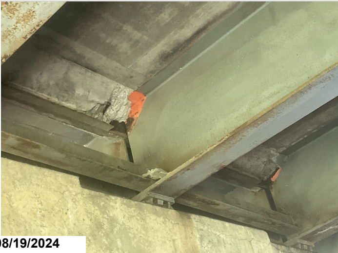
Bent # 5 Expansion Joint Assembly: Assembly is jammed together with distortion visible in assembly from the undersurface. The distortion appears to be spalling the deck expansion dam on the ahead side (Span # 6).
