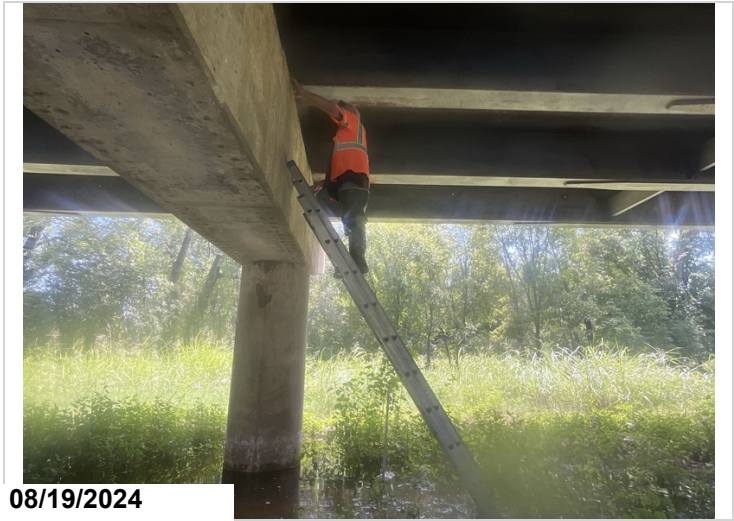
Bearing area inspection method.
