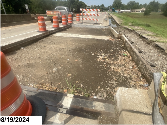
Approach Slabs: The outside Northbound lane of both approach slabs is in the process of being replaced. Approach Slab # 2 pictured.
