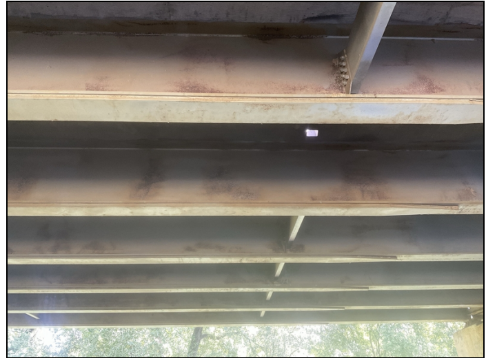
Paint system flaking / peeling.
