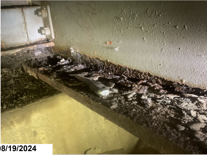
Span # 6, Abutment # 2, Girder # 8: Corrosion / section loss. 4LF CS3.
