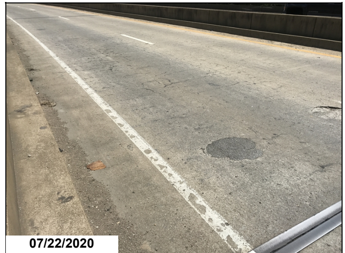
Span #3 SB cracking and spalling with exposed reinforcing steel.
