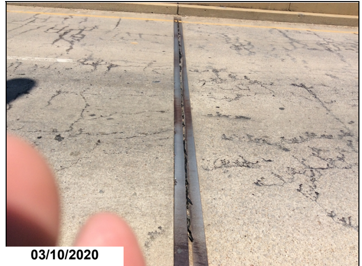
Bent 2 expansion joint
