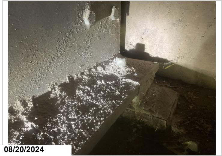
Span # 1, Abutment # 1, Bearing # 6: Missing left anchor bolt nut. 1EA CS2.
