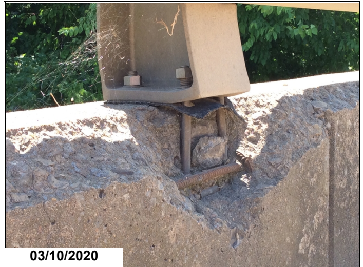
The right concrete bridge railing in span # 3 has a 12" spall that exposes reinforcing steel and the anchorage for one of the steel bridge railing post.
