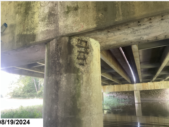
Bent # 5, Column # 2 , Back Side: 21" spall with exposed reinforcing steel with active corrosion / section loss. 1EA CS3.
