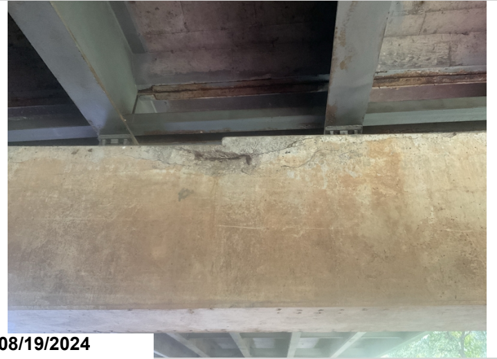
Bent # 2 Cap, Back Right Side: 2 12" spalls with exposed reinforcing steel. Spall, 1LF CS3, Exposed Steel, 1LF CS3.
