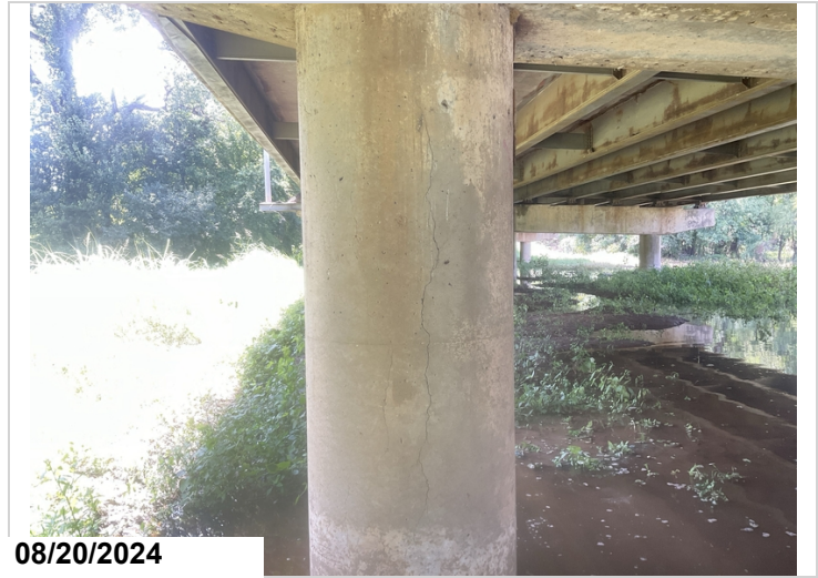
Moderate width vertical cracking in column.
