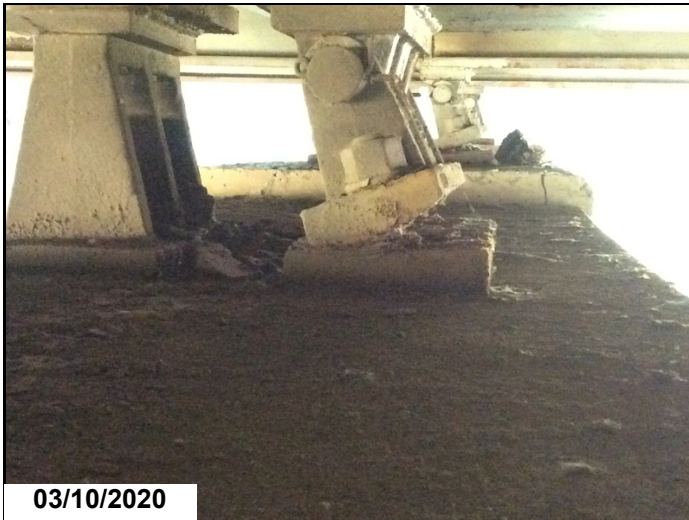
Bent # 2 bearings-Full expanded.
