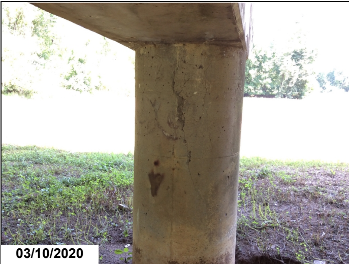
Cracking / delaminated area in column.
