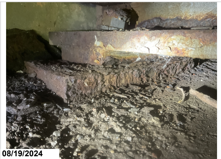
Span # 1, Abutment # 1, Bearing # 9: Corrosion with pack rust between sole and masonry plate. 1EA CS3.
