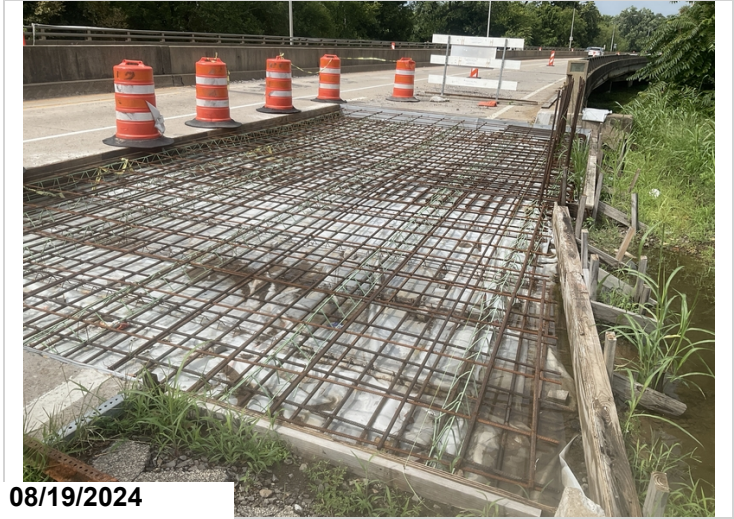
Approach Slab # 2: The outside Eastbound lane is in the process of being replaced.
