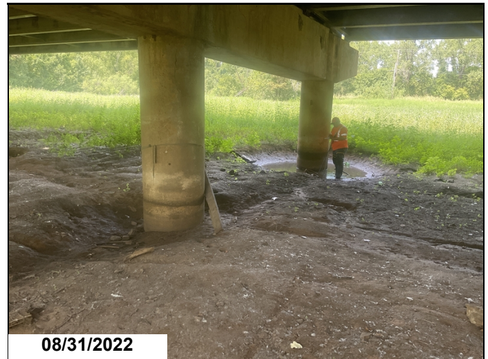
Localized scour around Bent # 6, Column # 1.
