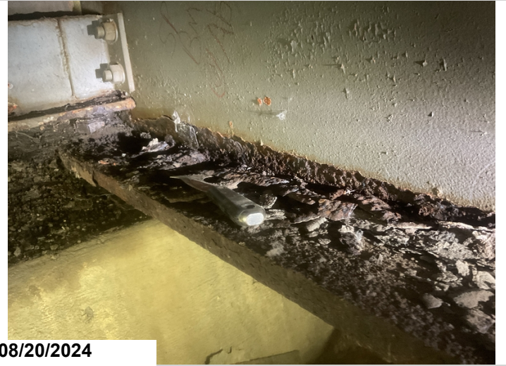
Span # 6, Abutment # 2, Girder # 8: Corrosion / section loss. 4LF CS3.
