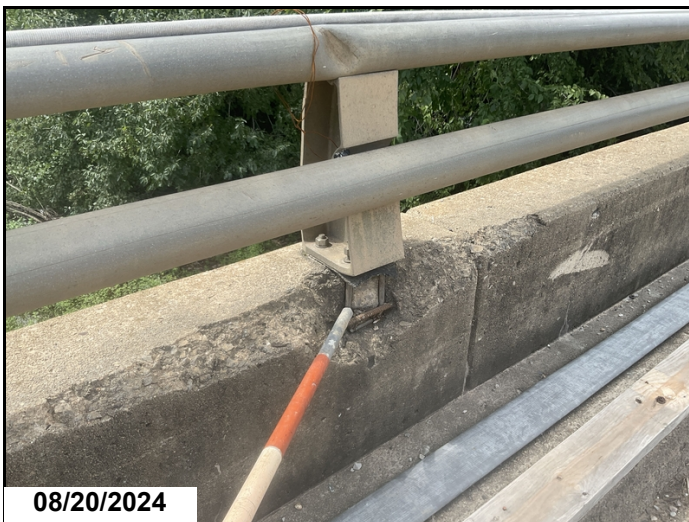
Span # 3, Right Railing, Eastbound Lane: Collision damage with a spall with exposed reinforcing steel at the base of the metal bridge rail post where the post is anchored to the concrete portion of the rail. 1EA CS4.
