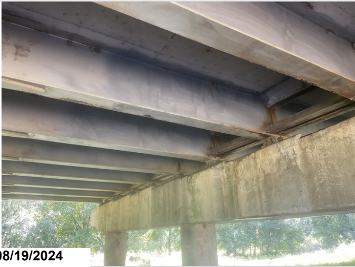
Spans # 4, 5 and 6: Ends of Girders have been painted in the past. Span # 5 girders pictured.
