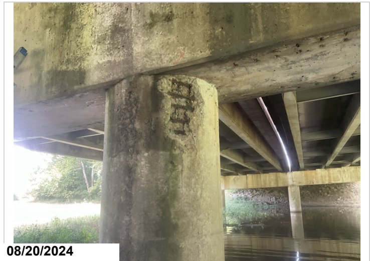
Bent # 5, Column # 2 , Back Side: 21" spall with exposed reinforcing steel with active corrosion / section loss. 1EA CS3.
