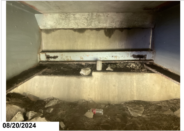
Abutment # 2, Bay # 8: Holes rusted through diaphragm.
