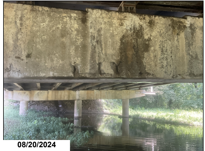
Bent # 5 Cap: Vertical 24" long delaminated area / spall with exposed reinforcing steel and numerous small delaminated areas with three 8" spalls with exposed reinforcing steel on the left side of the back face of cap. 4LF CS3.
