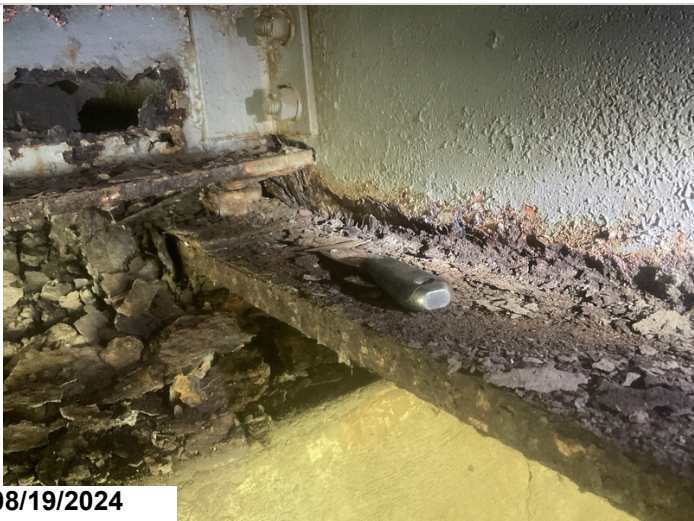
Span # 6, Abutment # 2, Girder # 9: Corrosion / section loss. 3LF CS3.
