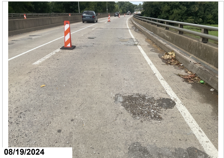
Span # 6, Westbound Outside Lane: Spalling with asphalt repairs.
