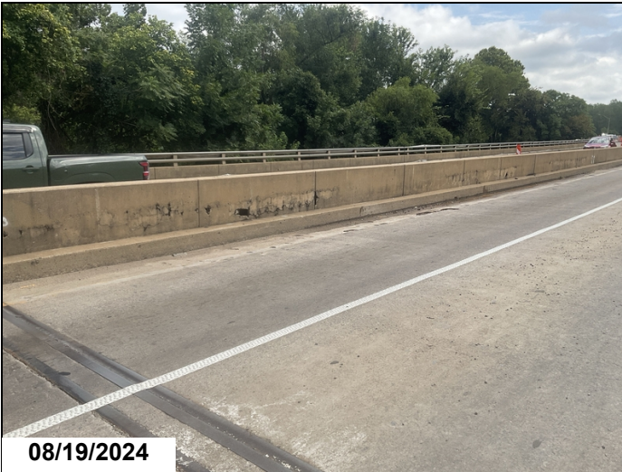
Span # 1: Median Barrier Wall: Concrete deterioration with spalling that exposes reinforcing steel and voids in the wall.
