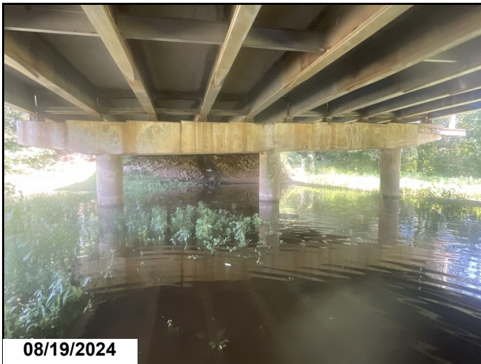
Past high water events has caused areas of minor localized scour around the bent columns.
