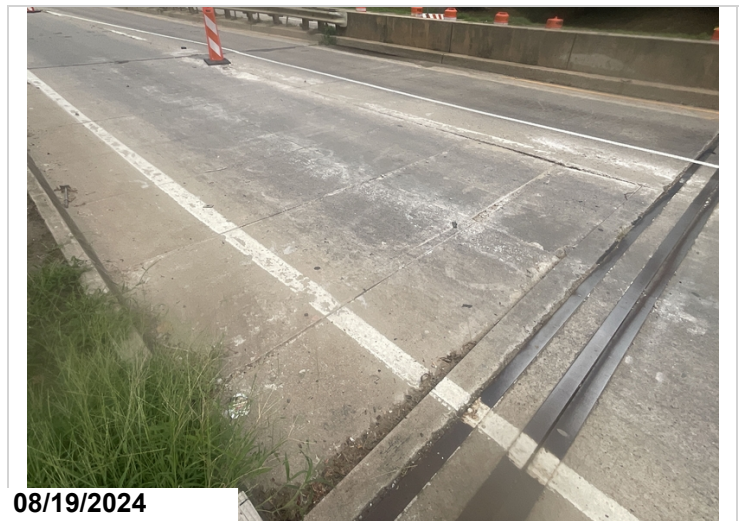
Approach Slab # 1 of Northbound Outside Lane has been prepped for removal with saw cuts visible throughout.
