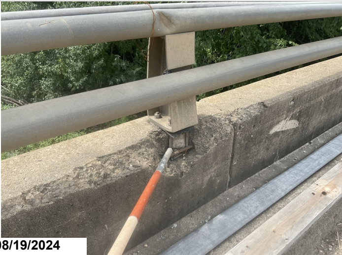
Span # 3, Right Railing, Eastbound Lane: Collision damage with a spall with exposed reinforcing steel at the base of the metal bridge rail post where the post is anchored to the concrete portion of the rail. 1EA CS3.
