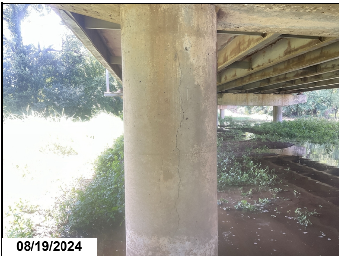
Moderate width vertical cracking in column.
