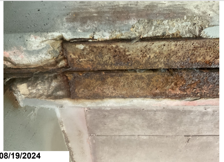
Bent # 2 Expansion Joint Assembly is jammed together in locations.
