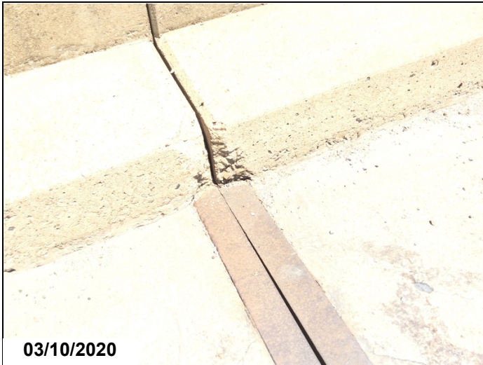
Bent #4, West bound side-Expansion joint assemblies jammed together.
