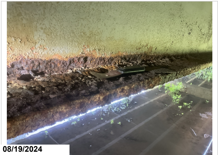
Span # 3, Bent # 3, Girder # 6: Corrosion to web and bottom flange in an area approximately 5' in length. Bottom flange has an estimated 1/16" section loss. Base of web and upper portion of web at expansion dam have an estimated 3/6" section loss. 5LF CS3.
