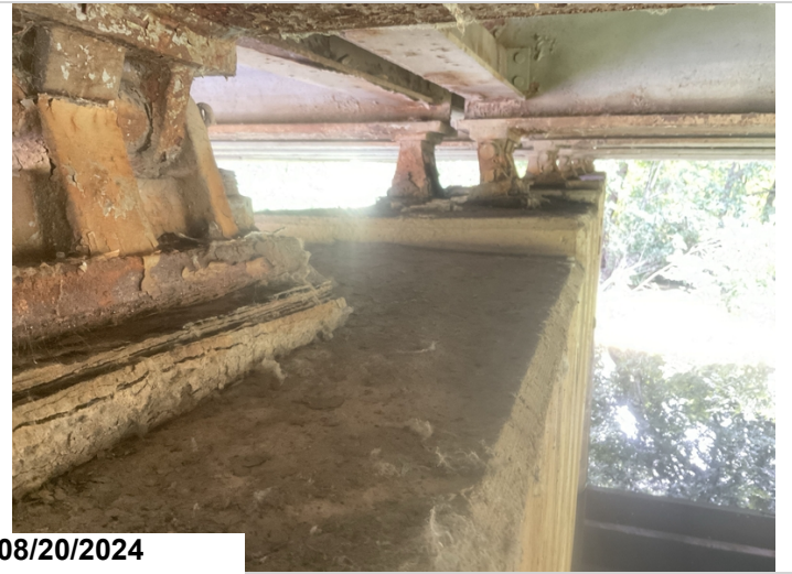
Bent # 3 Bearings: Failing paint system with pack rust between bearing plates.
