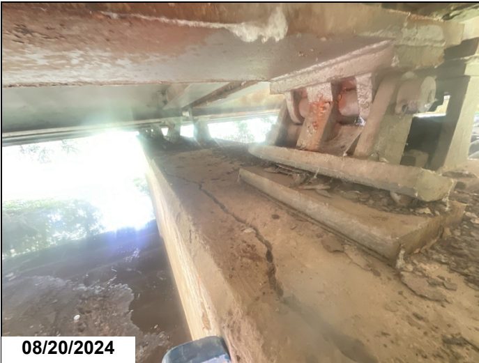
Bent # 2 Cap: Delaminated area.
