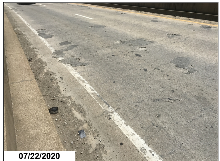
Span #1 SB concrete deterioration, delaminations and spalling.
