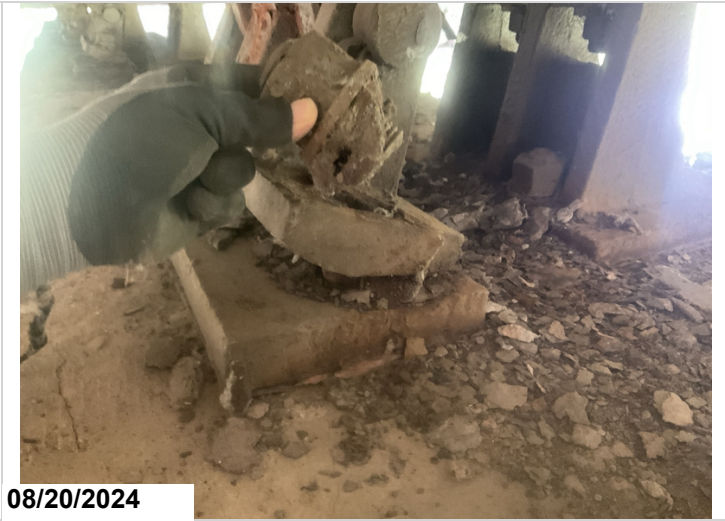
Span # 1, Bent # 2, Bearing # 9: Right anchor bolt sheared off. 1EA CS3.
