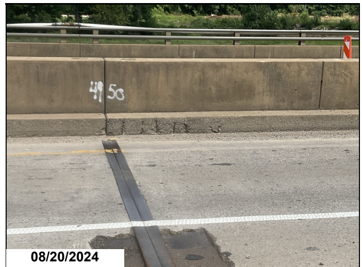
Span # 4, Median Parapet Wall, Adjacent to Bent # 4: Spalls with exposed reinforcing steel. 3LF CS3.
