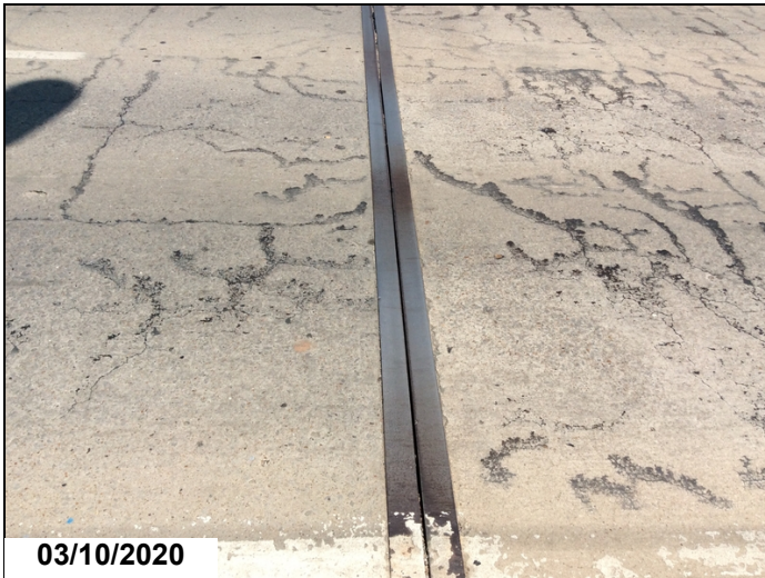
Bent 6. Deck joint seal
