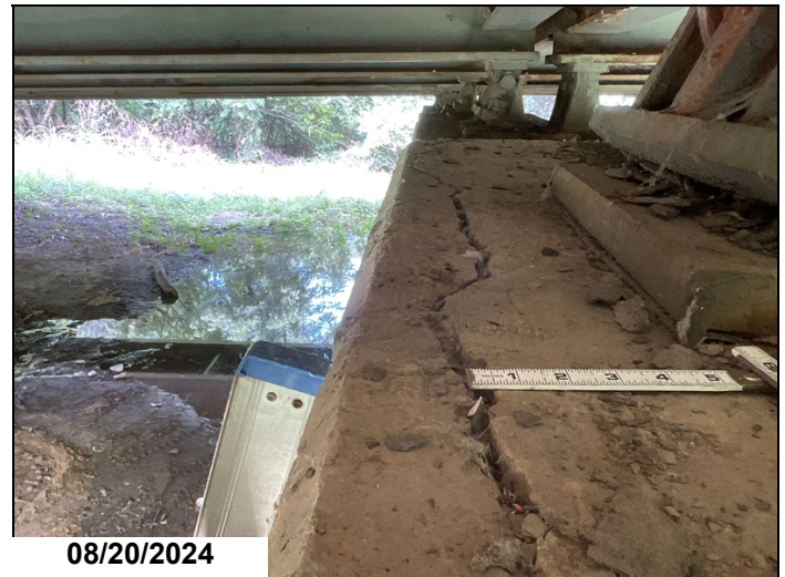
Bent # 2 Cap: Delaminated areas with wide longitudinal cracking visible in top of cap on right side. 14LF CS2.
