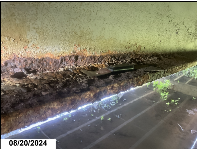
Span # 3, Bent # 3, Girder # 6: Corrosion to web and bottom flange in an area approximately 5' in length. Bottom flange has an estimated 1/16" section loss. Base of web and upper portion of web at expansion dam have an estimated 3/6" section loss. 5LF CS3.
