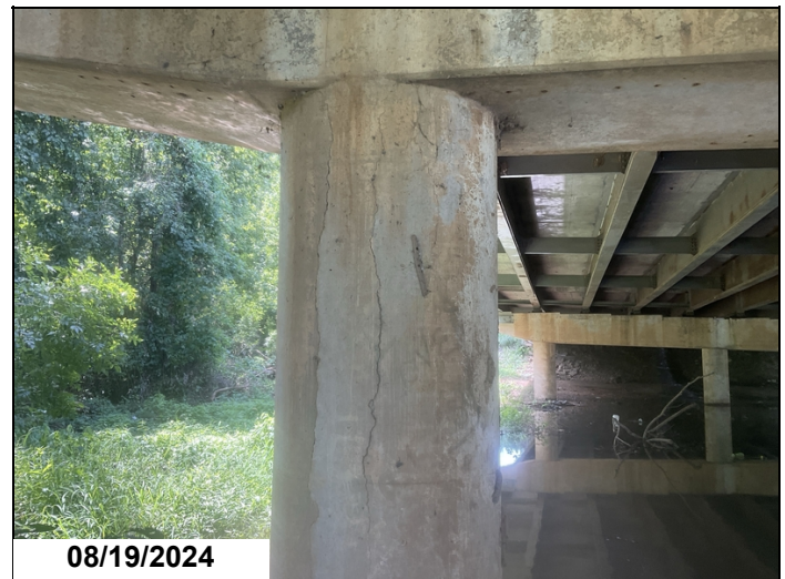
Bent # 3, Column # 3: 12" spall with exposed reinforcing steel in ahead side at the base of the column. Column has delaminated areas and vertical cracking in ahead side and back side. 1EA CS3.
