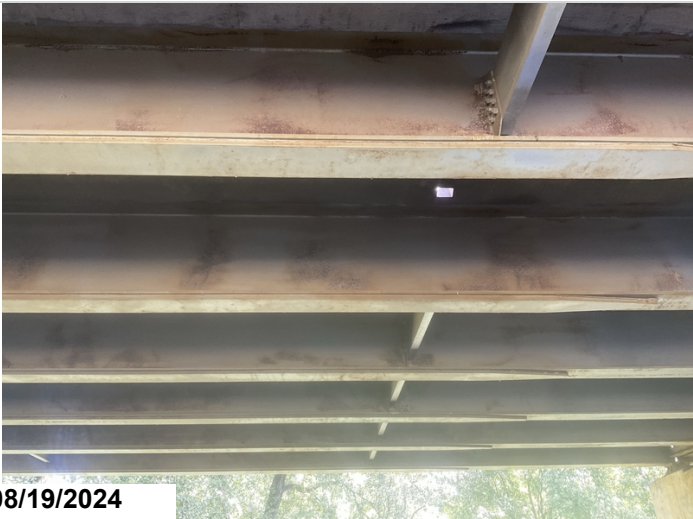
Paint system flaking / peeling.
