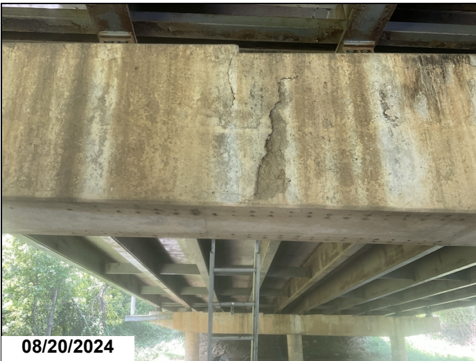
Bent # 3 Cap, Ahead Side, Between Columns # 2 and 3: Delaminated / spalled area. 1LF CS2. 1LF CS3.
