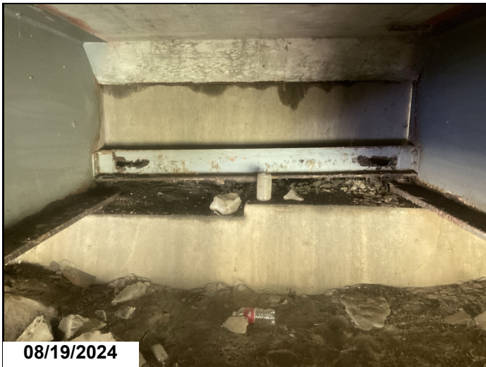
Abutment # 2, Bay # 8: Holes rusted through diaphragm.
