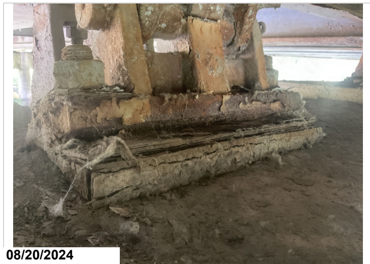
Span # 2, Bent # 3, Bearing # 2: Heavy pack rust between rocker and masonry plate. 1EA CS3.
