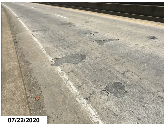
Span #2 SB concrete deterioration, delaminations and spalling.
