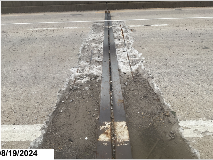
Repairs underway at expansion joints. Bent # 6 pictured.
