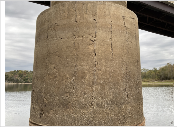
Bent 3, column 1-Wide vertical cracking.
