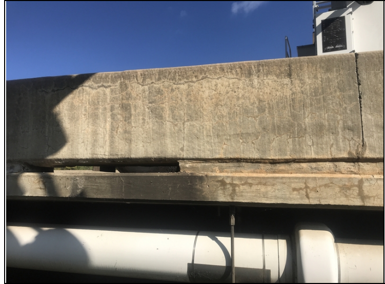
Map cracking with efflorescence in the exterior surface of the Parapet wall.
