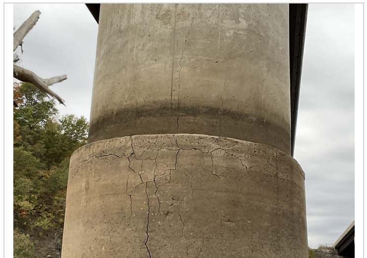
Bent 4, column 1-Mapcracking.
