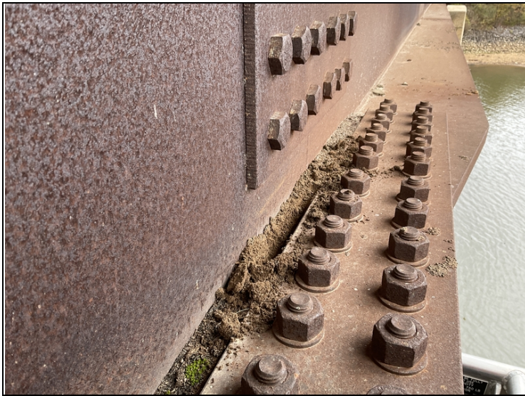
The exterior girders have dirt and debris accumulation adjacent to the splice plate connections potentially causing corrosion / abnormal weathering to girders.
