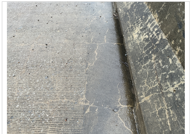
Span 1-Mapcracking in right gutter.
