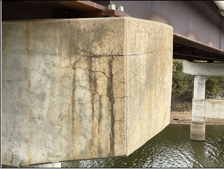
Bent # 4 cap, right side-Wide mapcracking.
