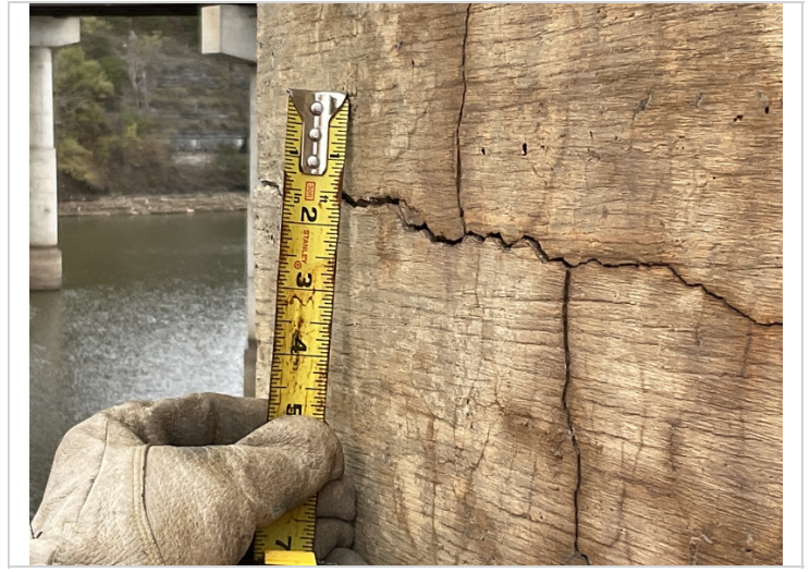
Bent 5 cap, right end-1/8" wide horizontal cracking.
