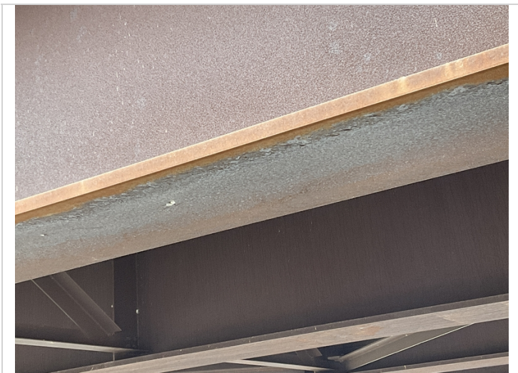
Span 4, beam 4-Abnormal weathering.
