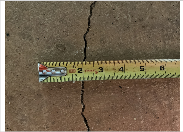
Abutment # 2 has a wide transverse crack that propagates across the bridge seat in bay # 2 located approximately 2' from girder # 3. The crack is 1/8" wide at this inspection. Photo 1.
