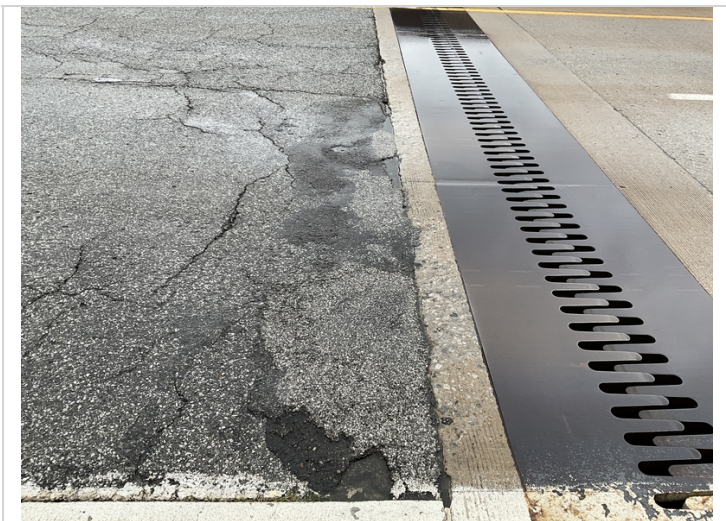
Asphalt mapcracking with repairs in West approach roadway.
