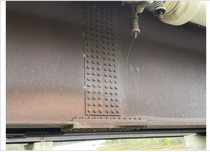
Span 1, girder 4 splice connection.
