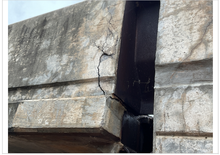
Wide cracking in exterior side of right parapet at abutment # 2
