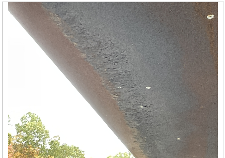
Span 2, girder 4-Abnormal weathering.
