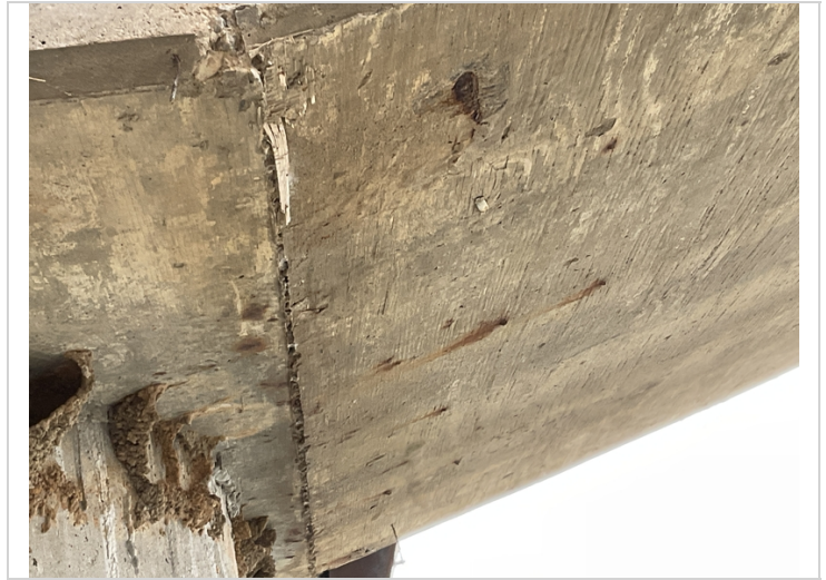
The undersurface of bent # 3 cap has two 3" shallow spalls with exposed reinforcing steel on the right side adjacent to column # 2.
