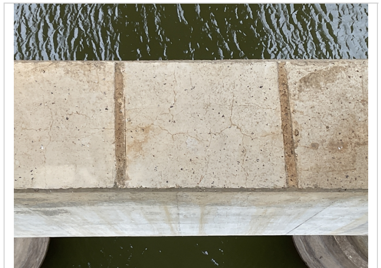
Bent 5 strut has mapcracking in the top surface.
