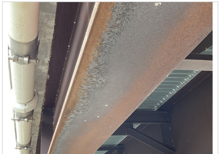
Span 5, girder 4-Abnormal weathering with large flakes.
