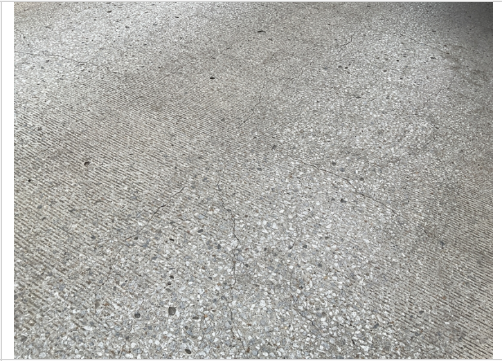
Span 1, right lane-Deck cracking.
