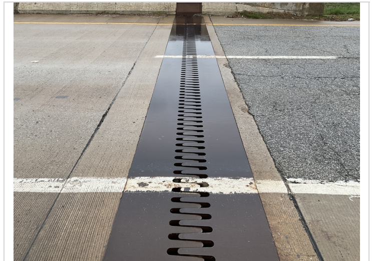
Abutment # 2 finger joint assembly.
