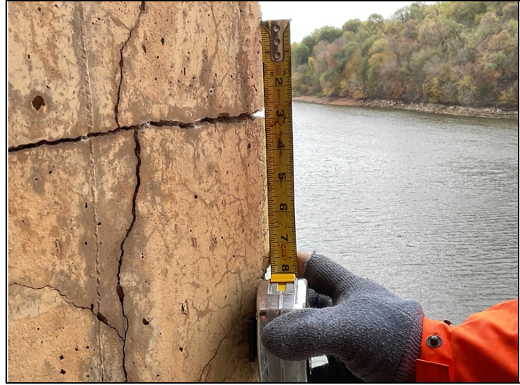
Bent # 4 cap, right side-Wide mapcracking.
