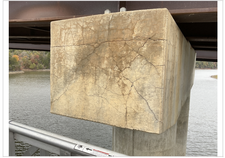
Bent 4 cap, right end-Mapcracking.
