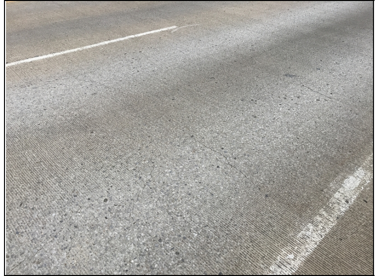
Map cracking.
