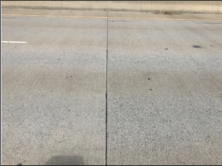
Transverse saw joint sealant is deteriorated.
