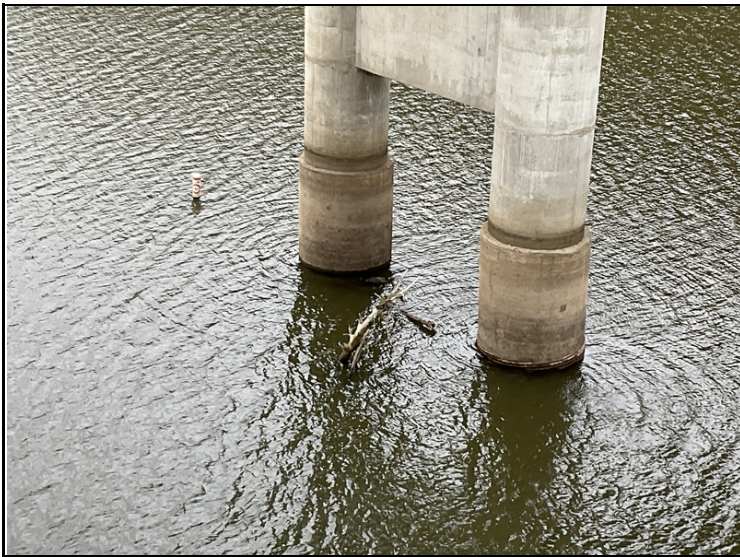
Submerged drift at bent # 4.
