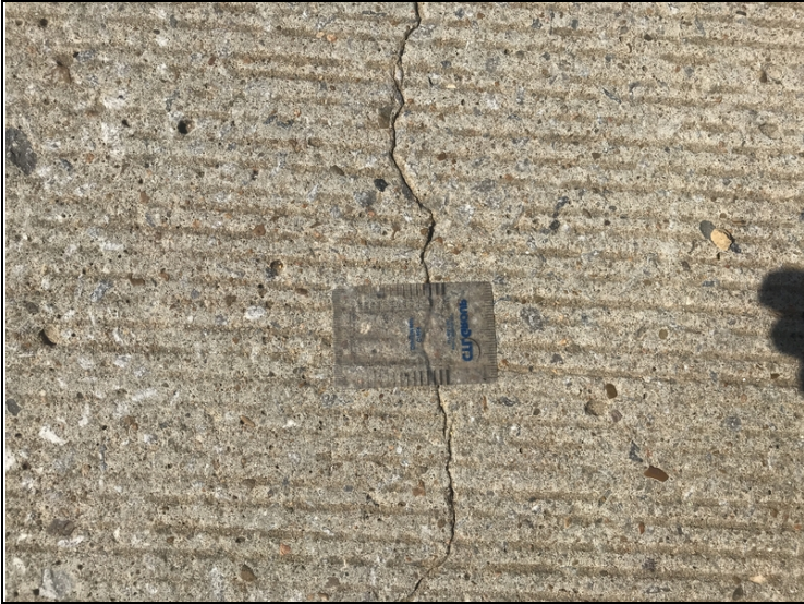
Sealable crack in the deck.
