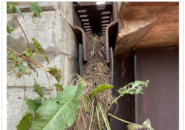
The expansion joint drainage trough on the left side of abutment # 2 has debris accumulation that restricts drainage.
