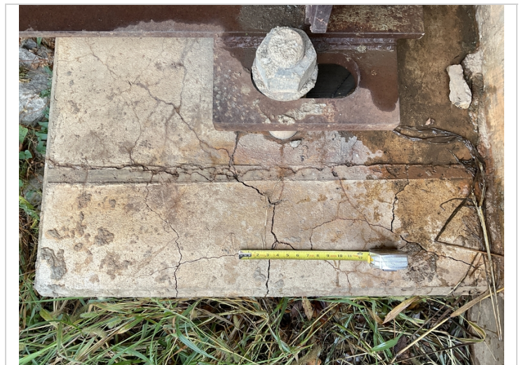
Wide mapcracking on right end of abutment # 2 bridge seat.
