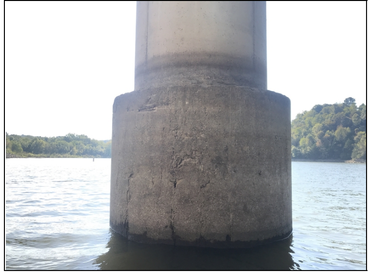
Bent # 3 right column. Exposed reinforcing steel.
