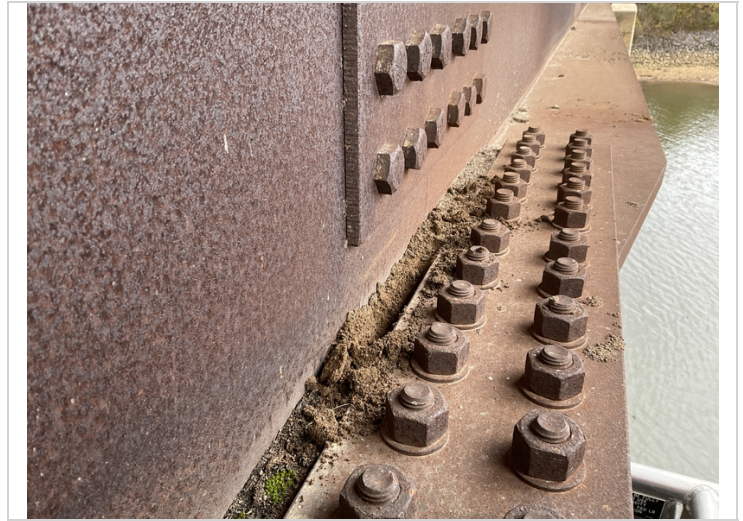
The exterior girders have dirt and debris accumulation behind the splice plate connections potentially causing corrosion / abnormal weathering to girders.
