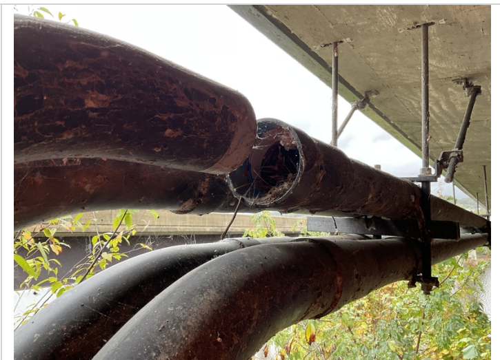
Unused conduit on left side has a failed connection at abutment # 1.
