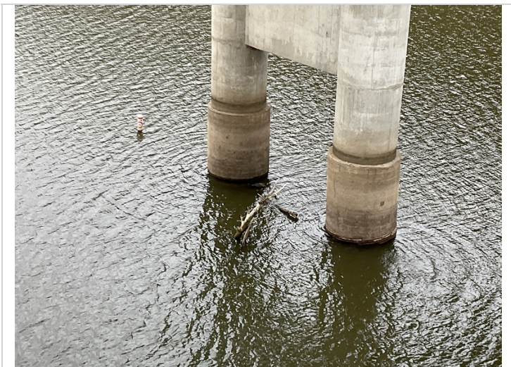
Submerged drift at bent 4.
