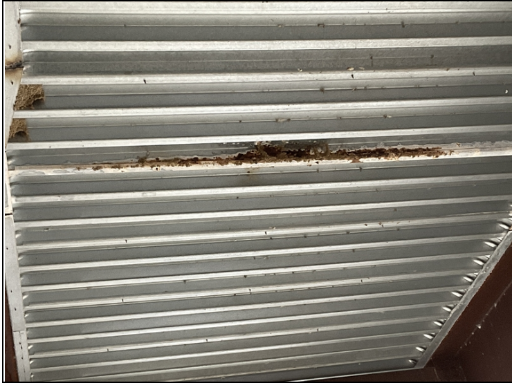
Span # 2, bay # 3-Corrosion to SIP forms.
