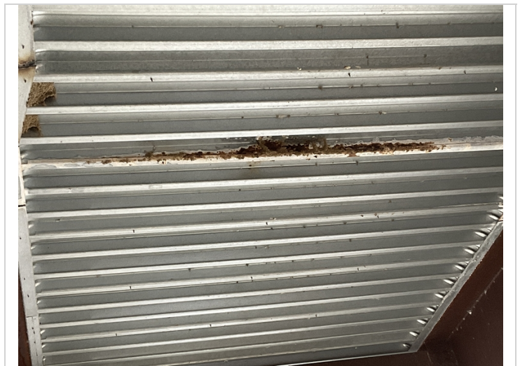
Span 2, bay 3-Corrosion to SIP forms.
