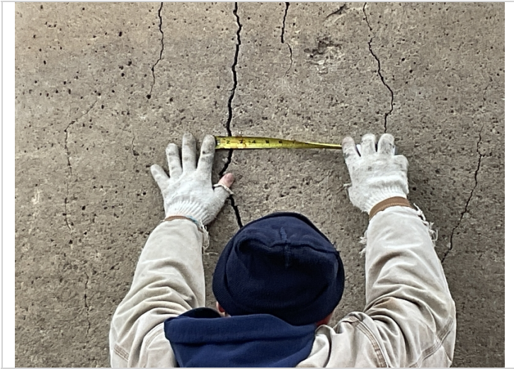
Bent 4, column # 1 has wide vertical cracks in the drilled shaft up to approximately 3/8" wide.
