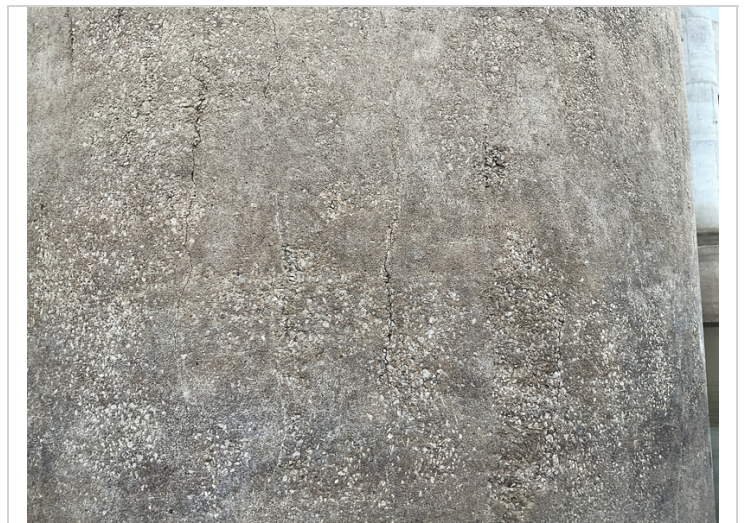
Bent 2, column 1-Vertical cracking.
