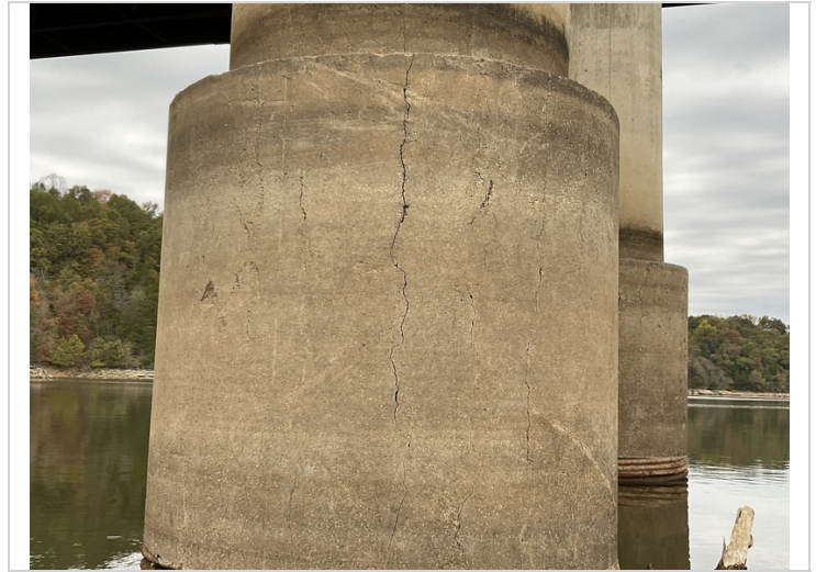
Bent 3, column 2-Wide vertical cracking.
