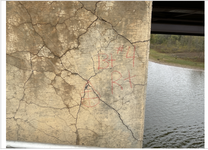
Bent 4 cap, right end-Delaminated area.
