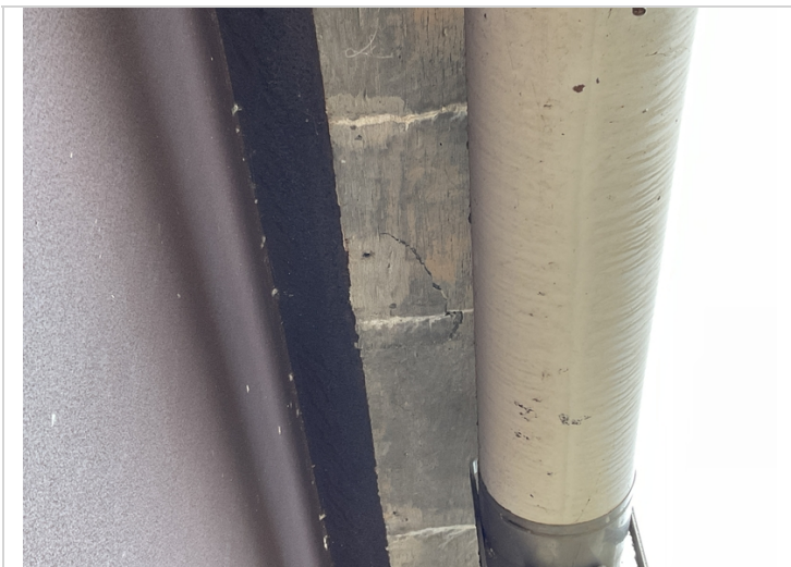
Span # 5, right side-Delaminated area in deck overhang adjacent to girder top flange.
