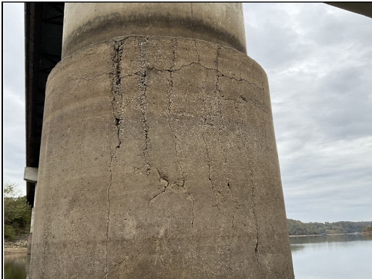
Bent # 4, column # 1-Wide vertical and horizontal cracking.
