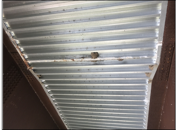
Corrosion in SIP forms.
