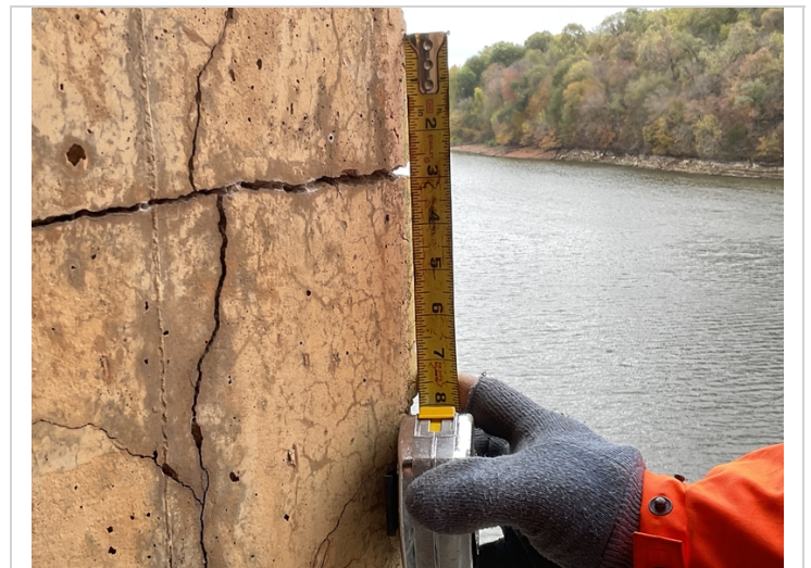
Bent 4 cap, right side-Wide mapcracking.
