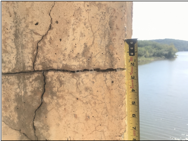
Right end of Bent # 4 cap has 3/8" wide map cracking.
