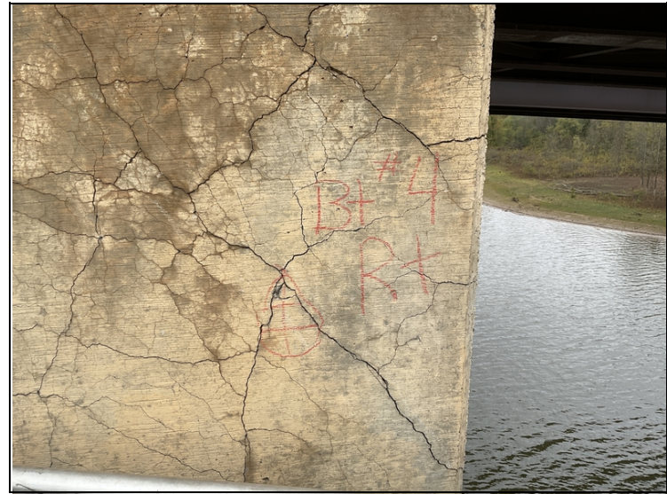
Bent # 4 cap, right end-Delaminated area.
