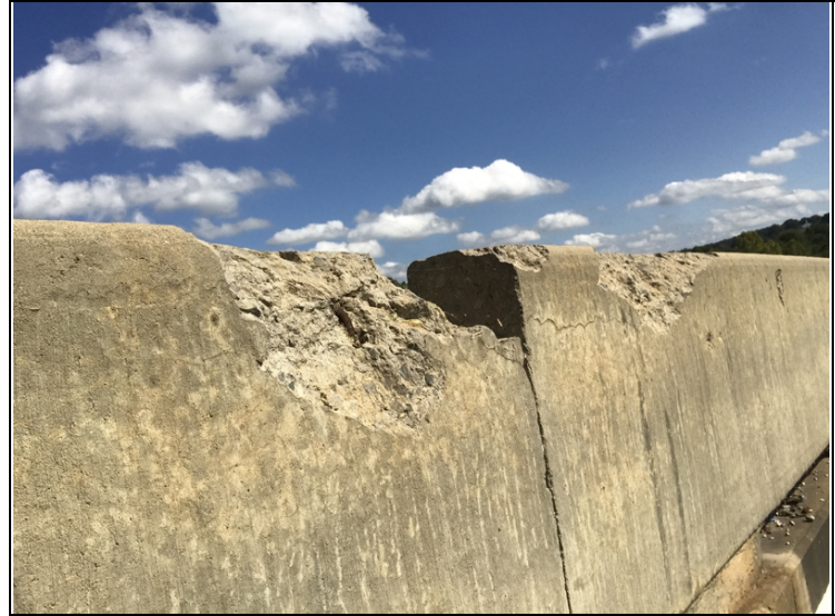
Spall in the Right parapet wall.
