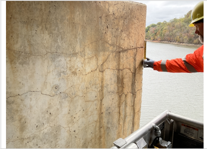
Bent 4 cap, right side-Wide mapcracking.
