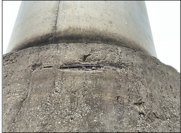
Bent # 3, column 2-Exposed reinforcing steel.
