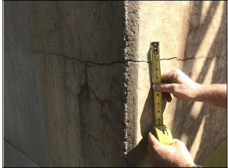
Right end of Bent # 5. 1/8" crack.
