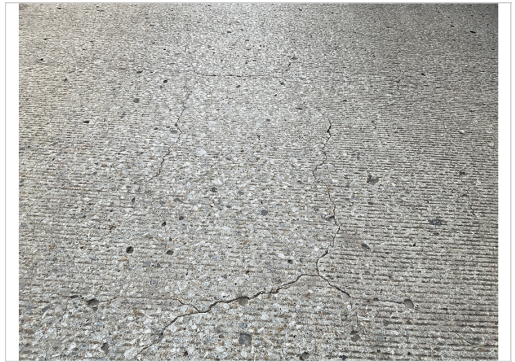
Span 1, right lane-Deck cracking.
