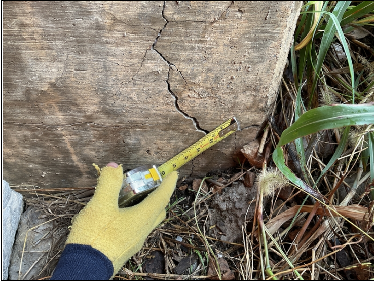
Wide mapcracking on right end of abutment # 2 bridge seat.
