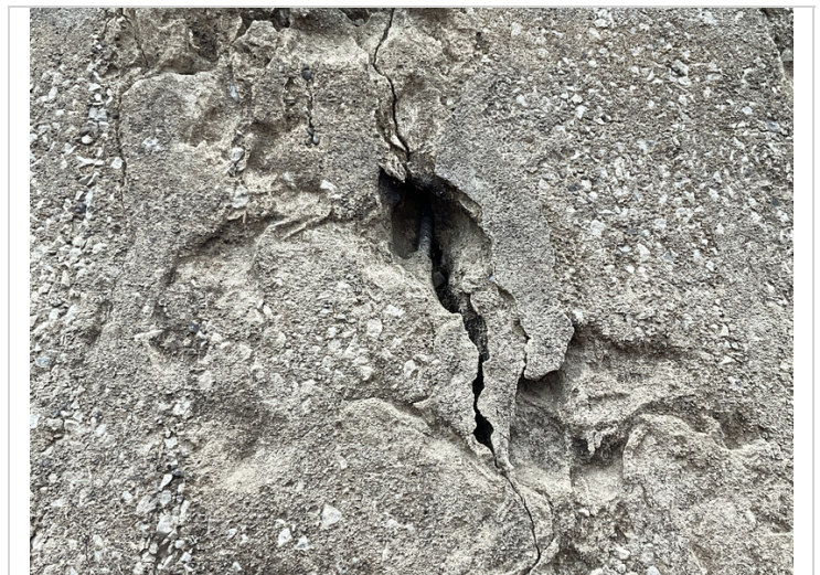
Bent # 3, column # 1-Honeycombing with exposed reinforcing steel.
