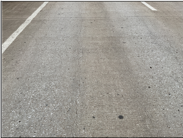
Longitudinal deck cracking.
