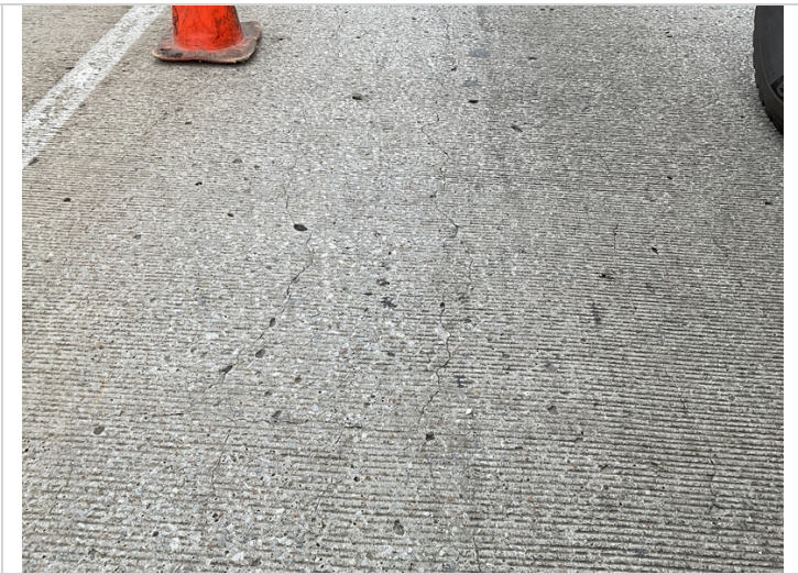
Span 1, right lane-Longitudinal cracking.
