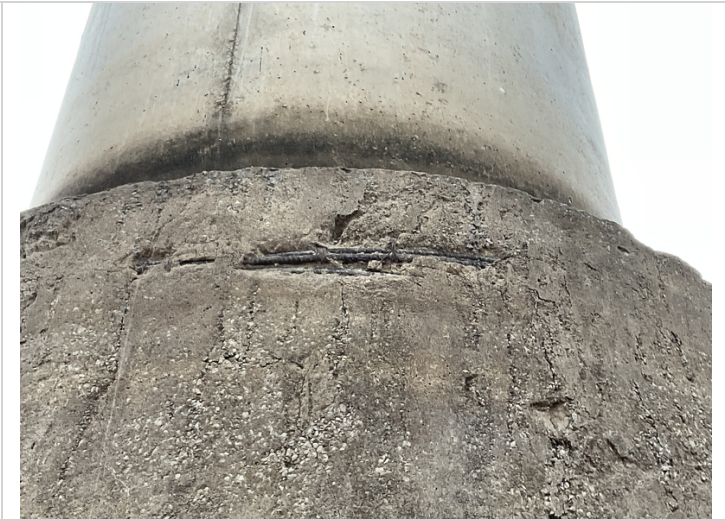
Bent 3, column 2-Exposed reinforcing steel.
