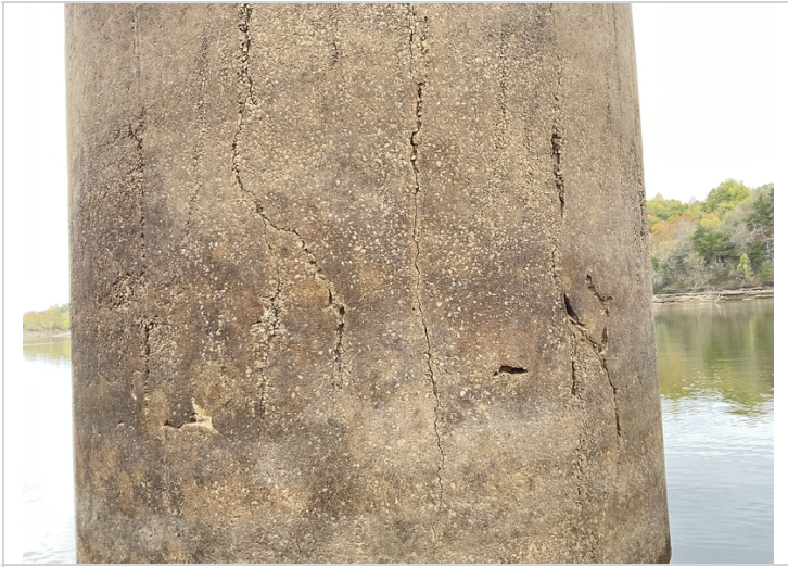
Bent 5, column 2-Vertical cracks.
