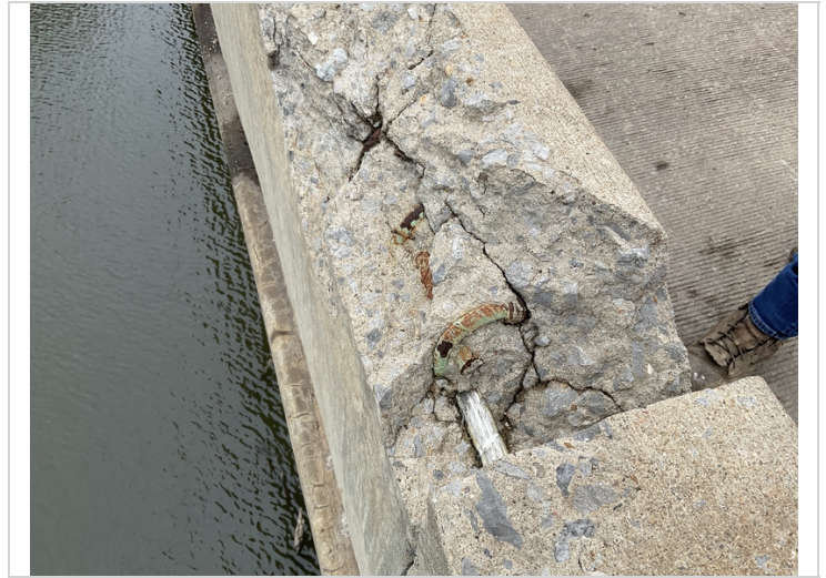
The right parapet in span # 3 has a large spall with exposed epoxy coated and fiberglass reinforcing bar.
