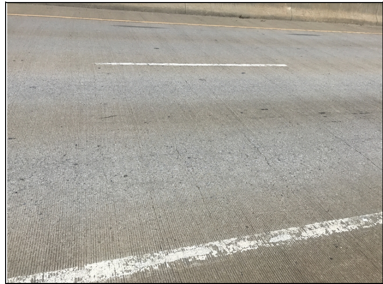
Sealable transverse cracks in the deck.
