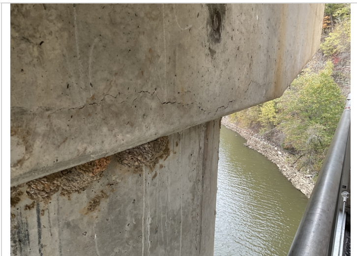
Bent 2 cap backface-Delaminated area over column 2.
