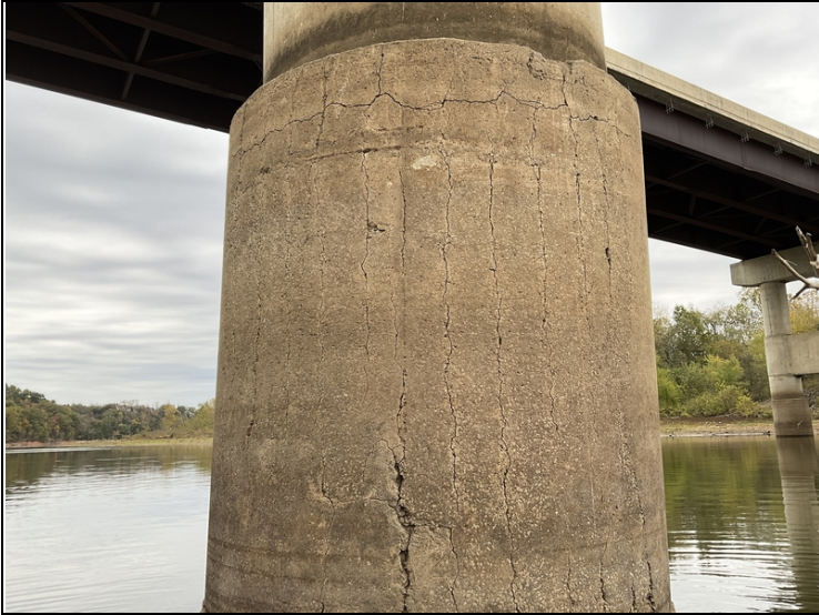
Bent # 4, column 1-Wide vertical cracking.
