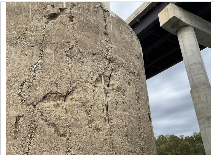
Bent # 3, column 1-Exposed reinforcing steel.
