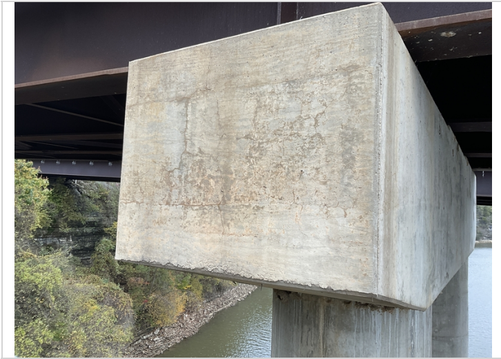
Bent 2 cap, right side-Mapcracking.
