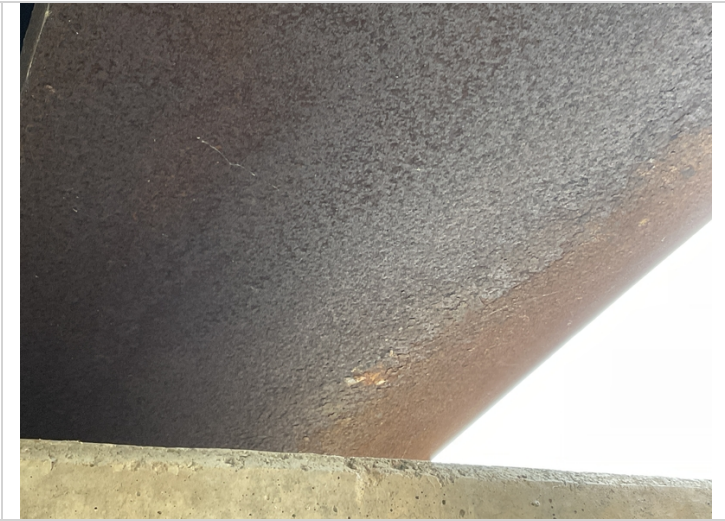
Span 2, girder 4-Abnormal weathering.
