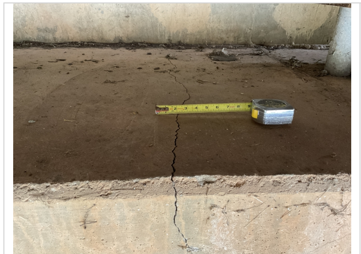
Abutment # 2 has a wide transverse crack that propagates across the bridge seat in bay # 2 located approximately 2' from girder # 3. The crack is 1/8" wide at this inspection. Photo 2.
