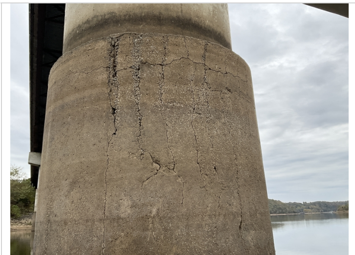
Bent 4, column 1-Wide vertical and horizontal cracking.
