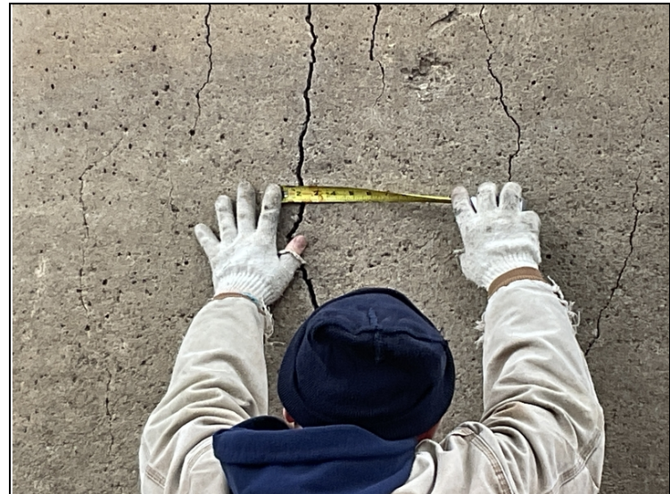
Bent # 4, column # 1 has wide vertical cracks in the drilled shaft up to approximately 3/8" wide.
