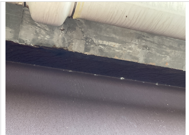
The undersurface of the deck overhang in span # 4 has a 12" delaminated area adjacent to girder # 4 top flange located adjacent to splice connection # 1.
