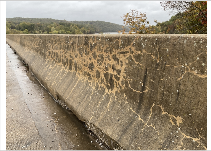
Span 1, right side-Mapcracking in parapet.
