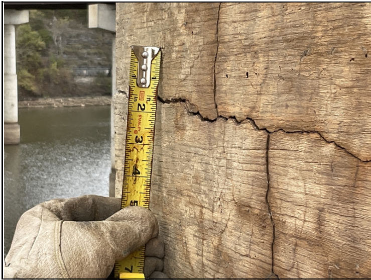
Bent # 5 cap, right end-1/8" wide horizontal cracking.
