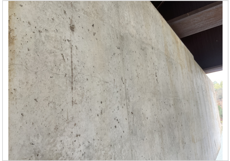
Bent 4 cap-Horizontal hairline crack.
