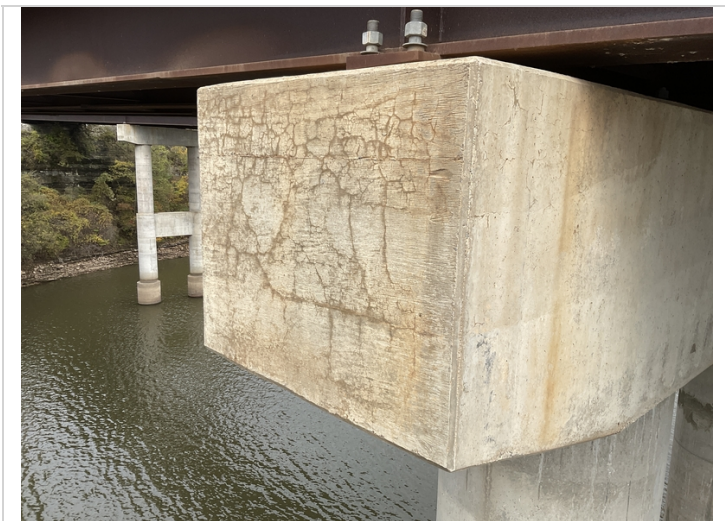
Bent 3 cap, right end-Mapcracking.
