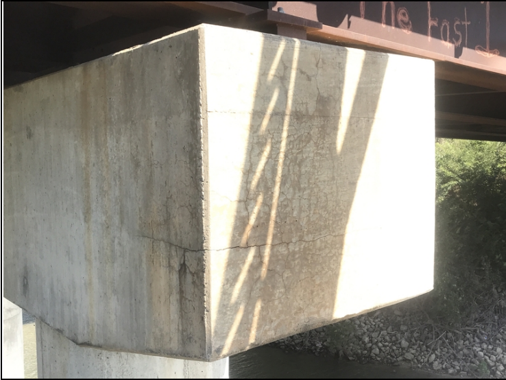
Right end of Bent # 5 Cap. Map cracking.
