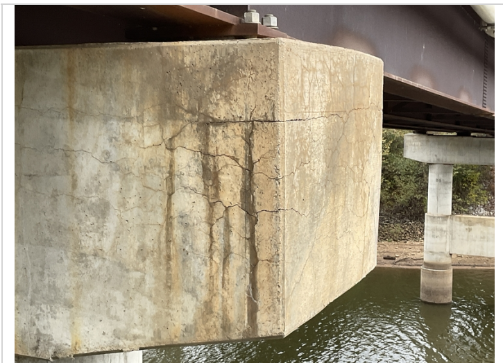
Bent 4 cap, right side-Wide mapcracking.
