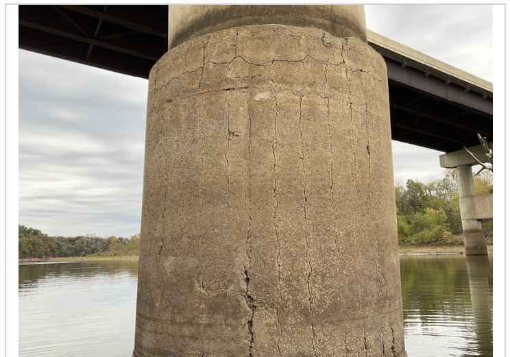
Bent # 4, column 1-Wide vertical cracking.
