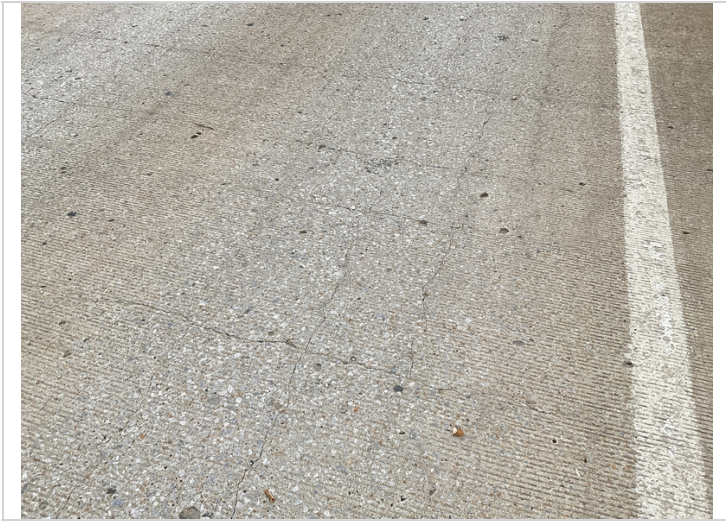
Span 3, right lane-Mapcracking.
