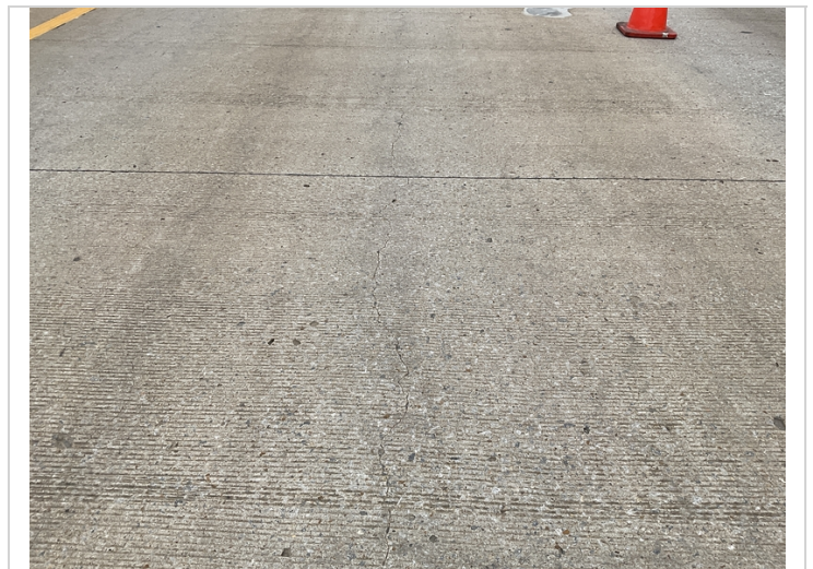
Span 4, left lane-Longitudinal cracking.
