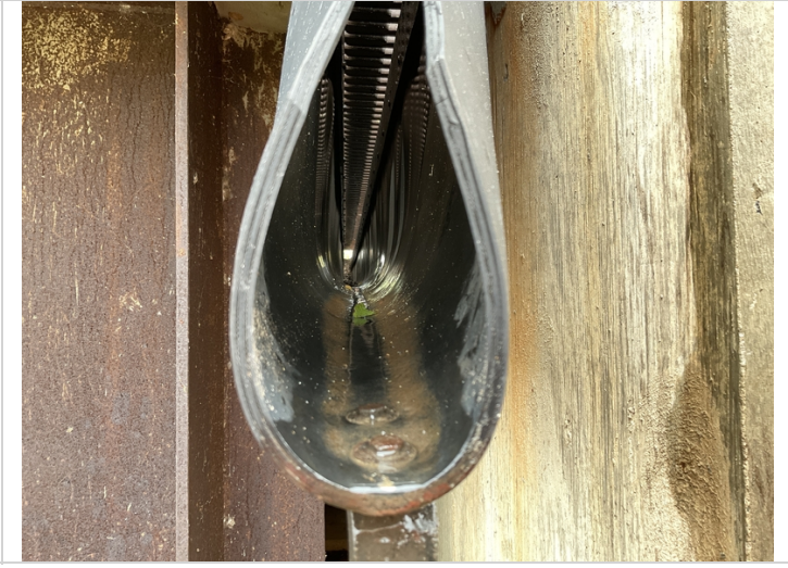
Expansion joint trough at abutment 1.
