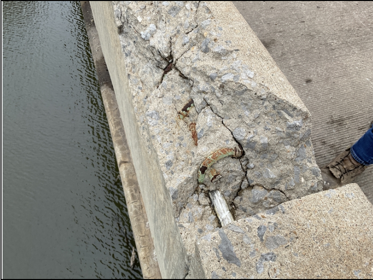
The right parapet in span # 3 has a large spall with exposed epoxy reinforcing steel.
