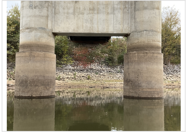
Bent 5 drilled shafts.
