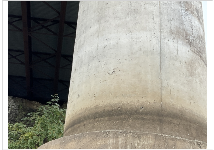
The lower portion of bent # 2 columns have 4" shallow delaminated areas in the ahead face.
