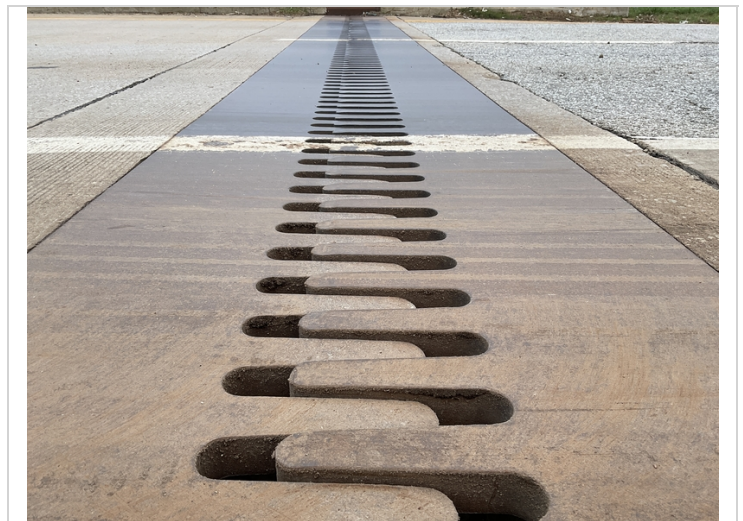
The finger joint over abutment # 2 has a height differential of approximately 3/8" from the portion of assembly at abutment # 2 side to the portion of assembly on the span # 5 side.
