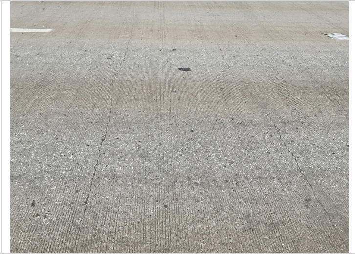
Span 5, right lane-Transverse cracking.
