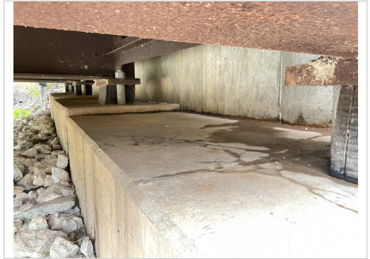
Abutment # 2 bearing area.
