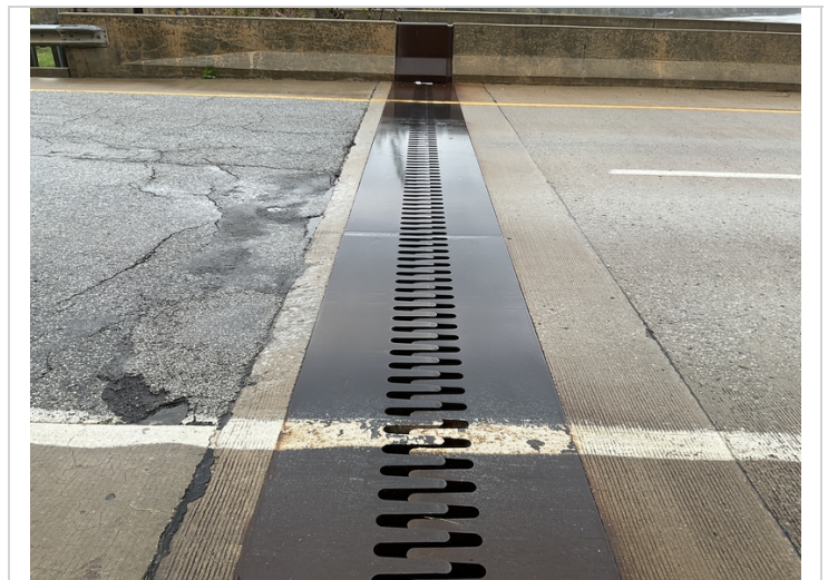
Abutment 1 finger joint assembly.
