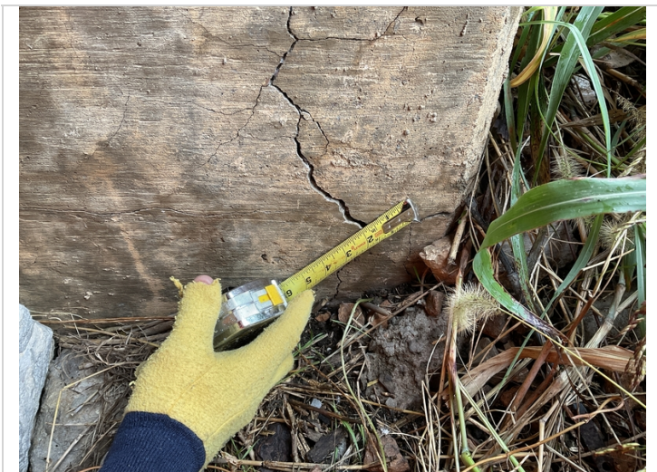
Wide mapcracking on right end of abutment # 2 bridge seat. Photo 2.
