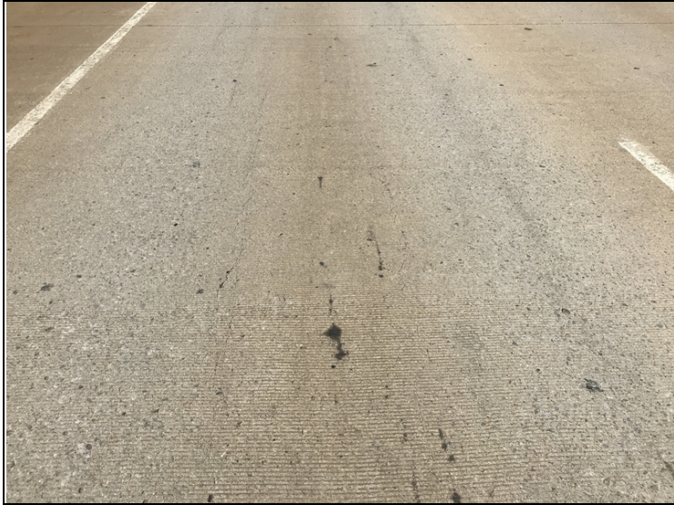
Sealable Longitudinal cracking in the deck.
