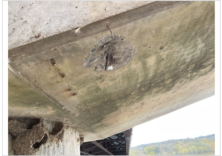
The undersurface on bent # 2 cap has a 6" spall with exposed reinforcing steel on the right side adjacent to column # 2. Exposed steel has initial section loss.
