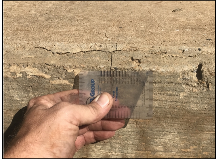
Bent # 3 cap, right side-0.035" cracking.
