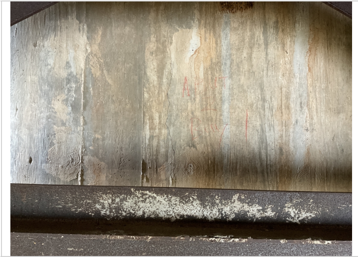
Abutment 2, bay 1-Vertical crack in backwall.
