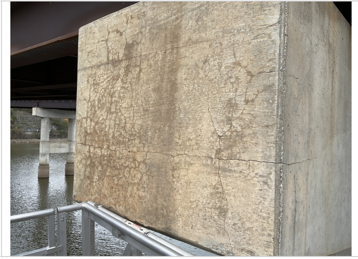
Bent 5 cap, right end-Mapcracking.
