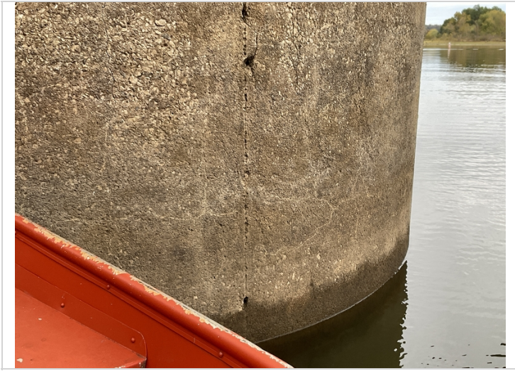
Bent 2, column 1-Light mapcracking.
