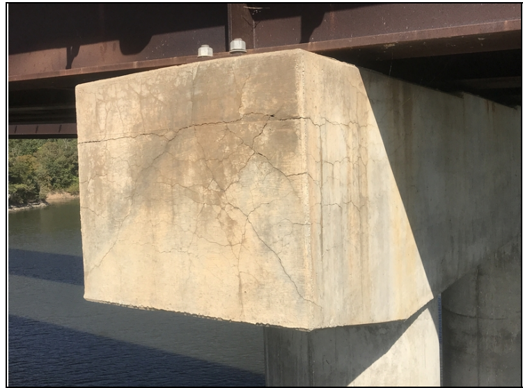
Right end of Bent # 4 cap-Mapcracking.
