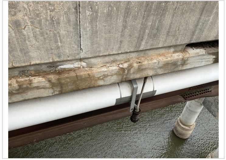
The exterior edges of the deck have mapcracking with areas of scaling and concrete deterioration.
