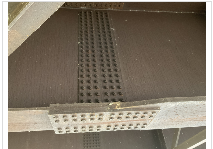
Typical of span 1 splice connections.
