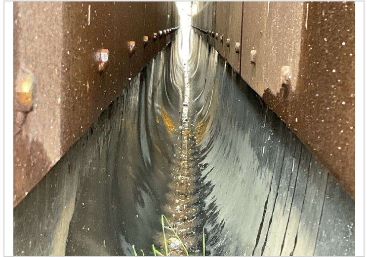
Expansion joint trough at abutment 1.
