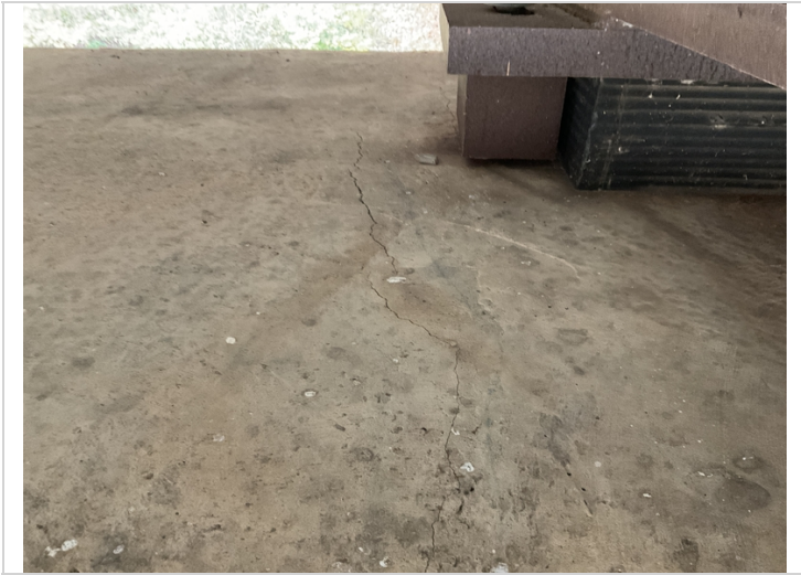
Bent # 5 cap-Transverse crack in top of cap adjacent to beam 2.
