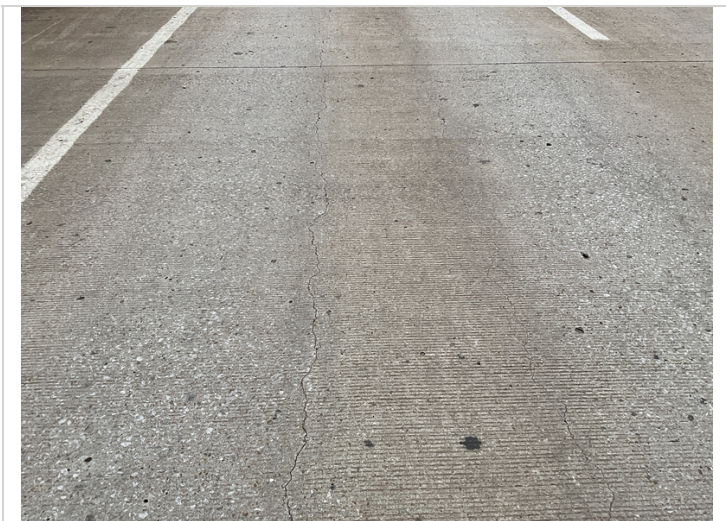
Longitudinal deck cracking.
