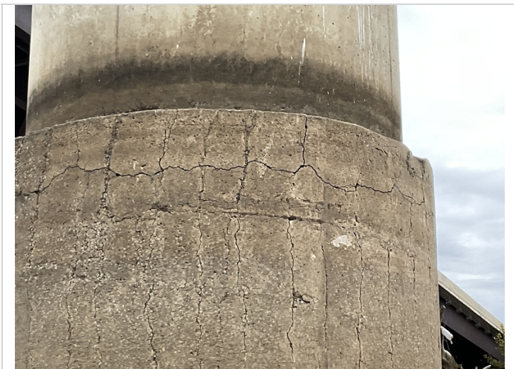
Bent 4, column 1-Wide horizontal cracking.
