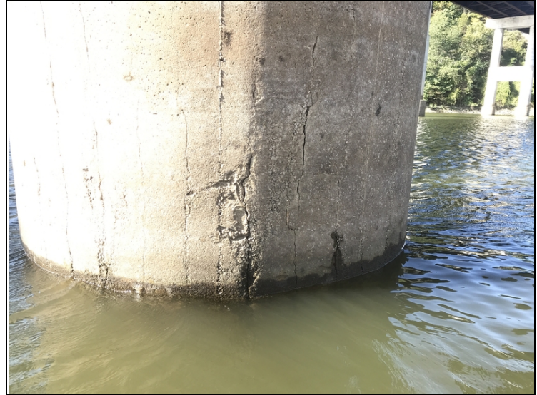
Exposed reinforcing steel in the Right column of Bent # 4.
