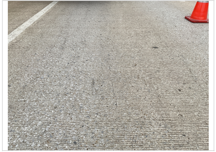
Span 1, left lane-Longitudinal cracking.
