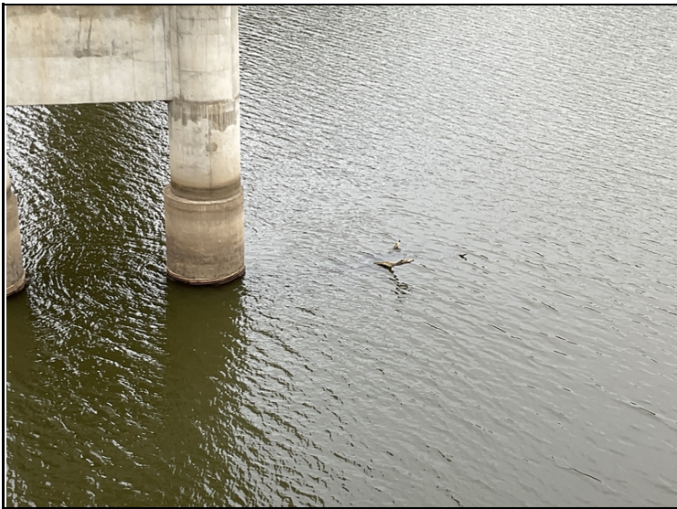
Submerged drift at bent # 4.
