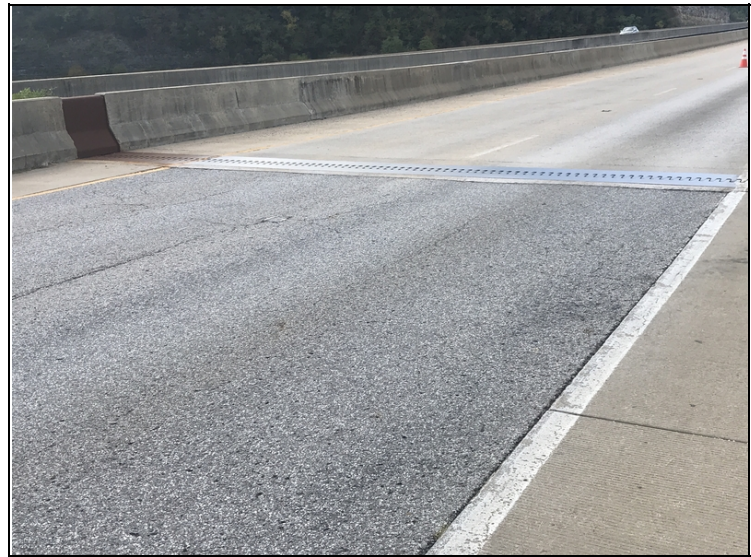
Asphalt settlement at the East bridge end.
