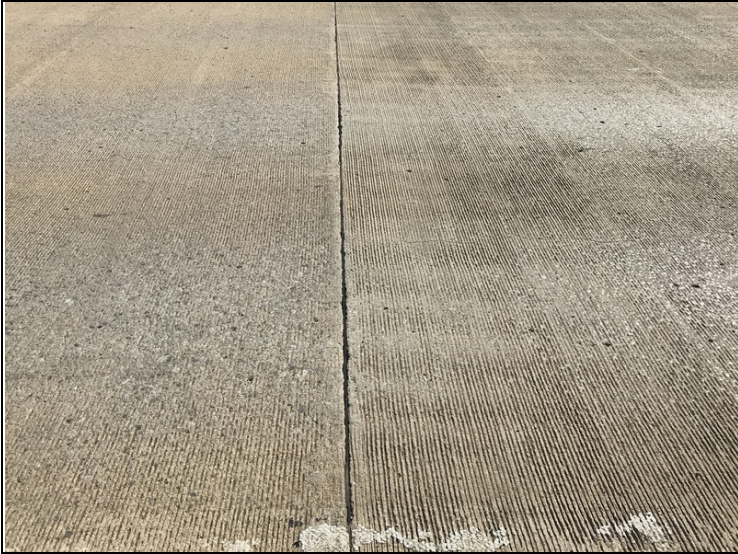
Transverse saw joint sealant.
