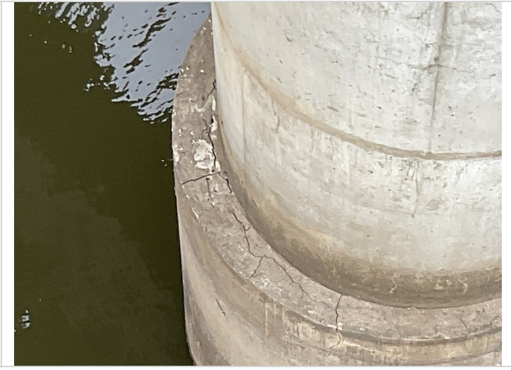
Bent # 5, column # 1-Wide cracking in top of drilled shaft.
