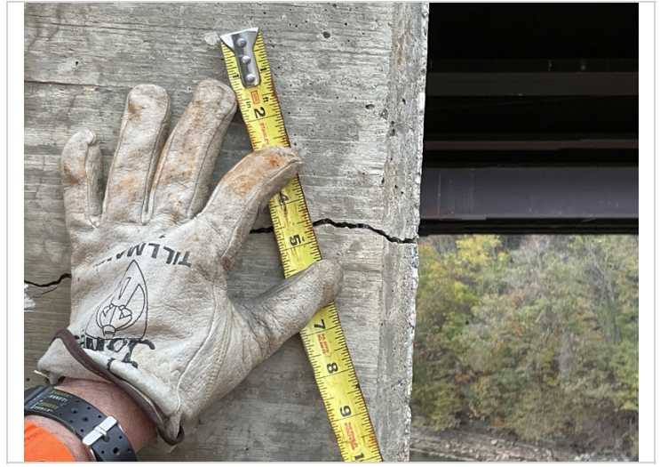
Bent 3 cap, Left end-1/8" wide mapcracking.
