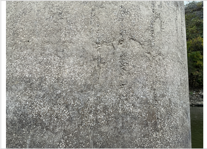
Bent 2, column 1-Exposed steel.
