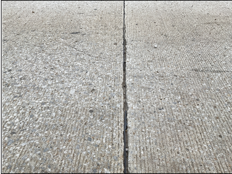
Saw joint material missing.
