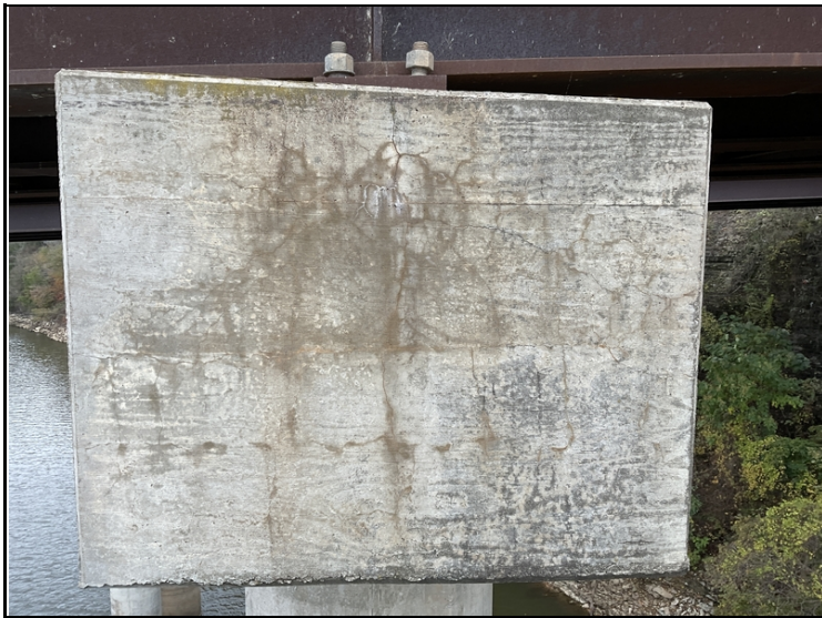
Bent # 2 cap, left end-Mapcracking.
