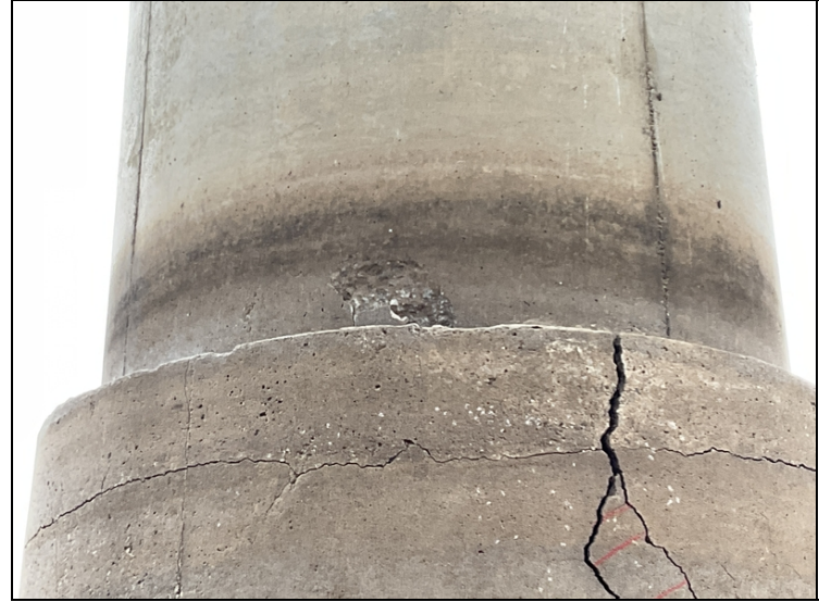
Bent # 4, column # 1-Wide vertical cracking shallow 10" spall.
