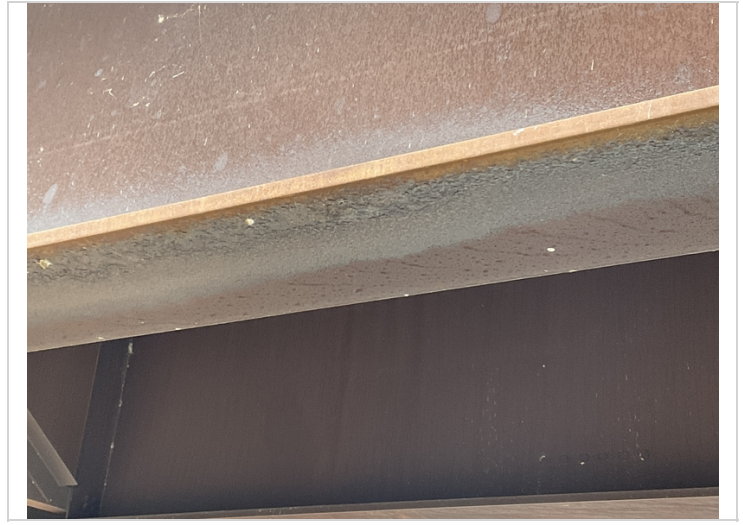
Span 5, girder 1-Abnormal weathering.
