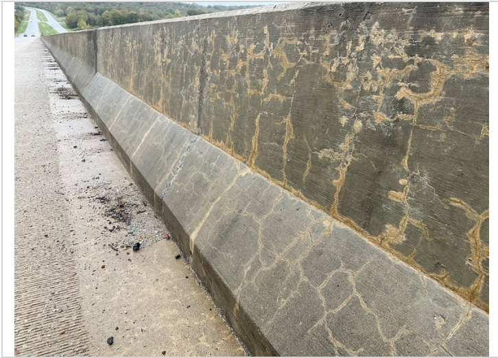
Span 1, right side-Mapcracking in right parapet.
