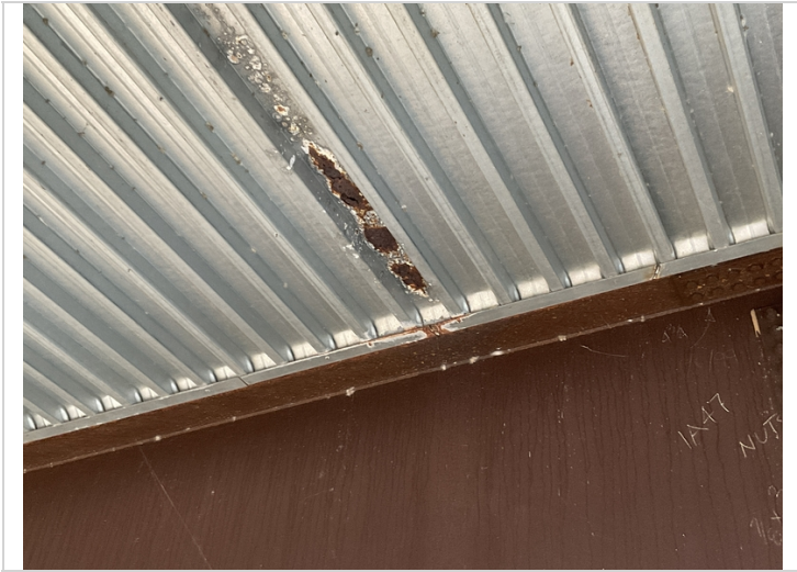
Span 5, bay 3-Corrosion to SIP forms.
