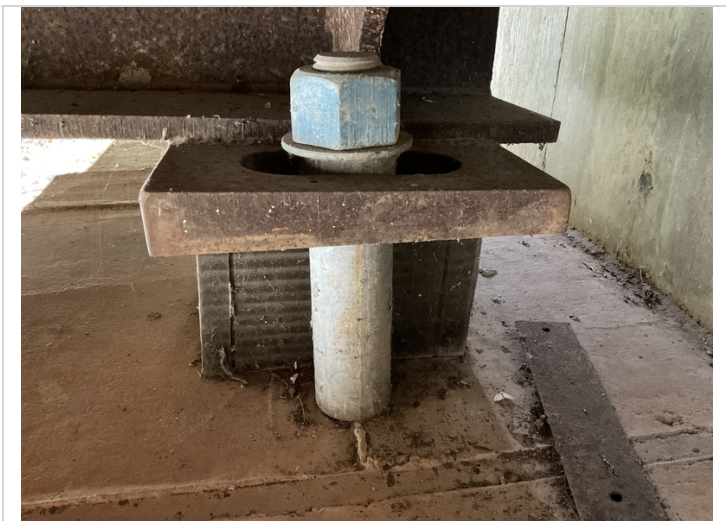
Abutment 2-Bearings at neutral position with ambient temperature approximately 55 Degrees Fahrenheit at time of inspection.
