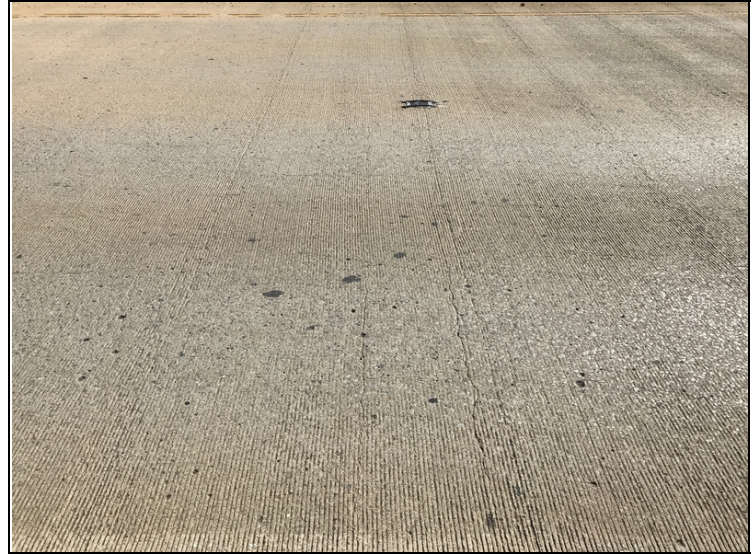
Sealable transverse cracks.
