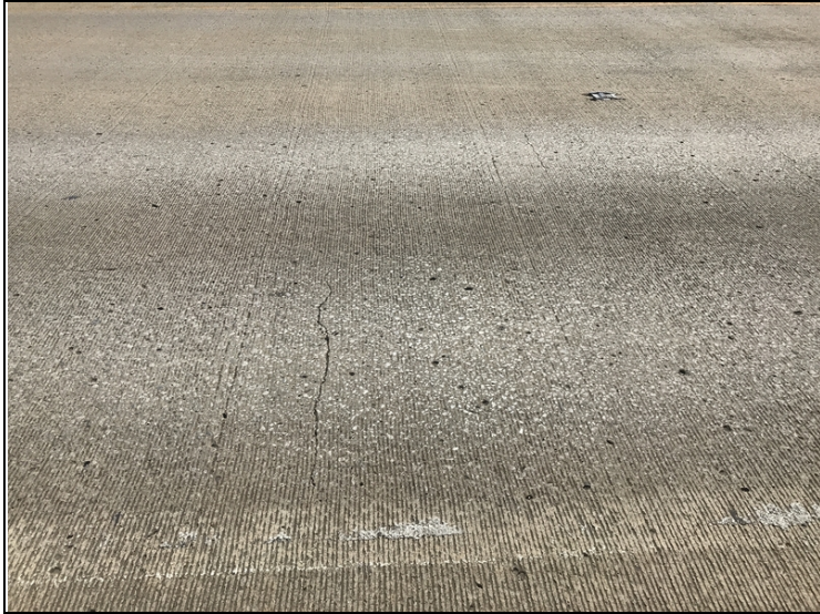
Transverse cracking in the deck.
