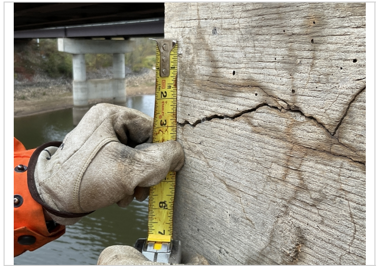
Bent 4 cap, left end-1/8" wide mapcracking.
