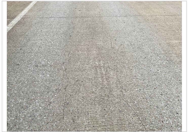
Span 2, left lane-Longitudinal cracking.
