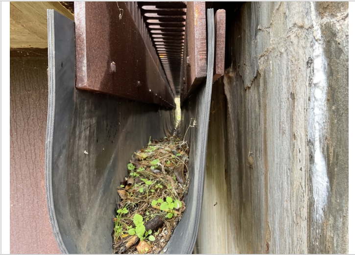
The right end of the expansion joint drainage trough at abutment # 2 has debris accumulation that restricts drainage.
