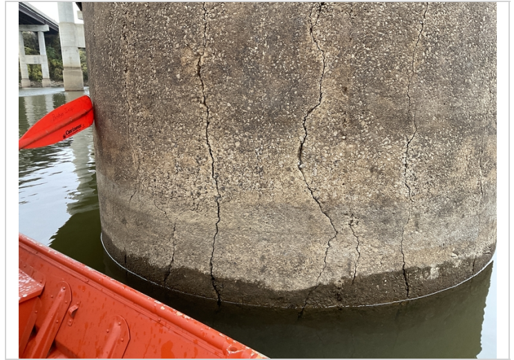
Bent # 5, column # 1-Wide vertical cracking.
