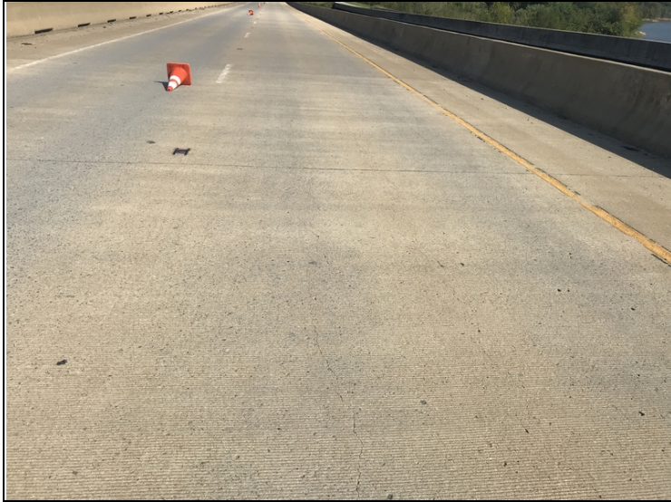
Longitudinal deck cracks.
