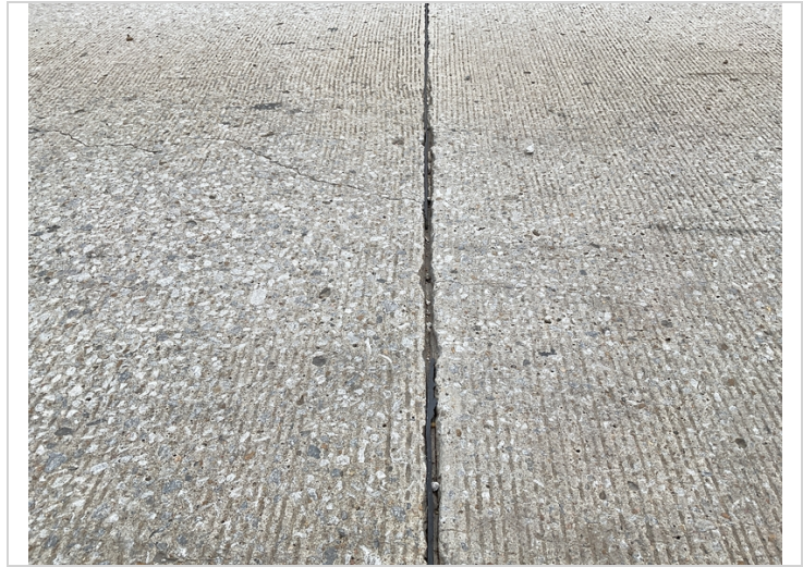
Saw joint material missing.
