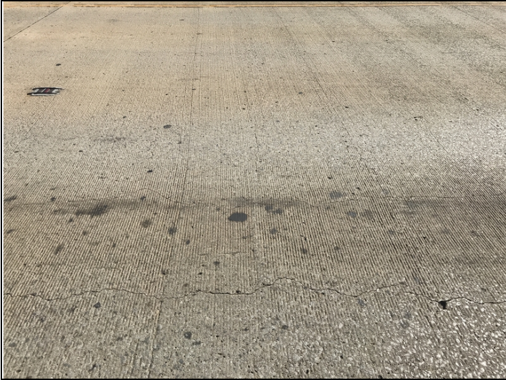
Longitudinal and Transverse cracks.
