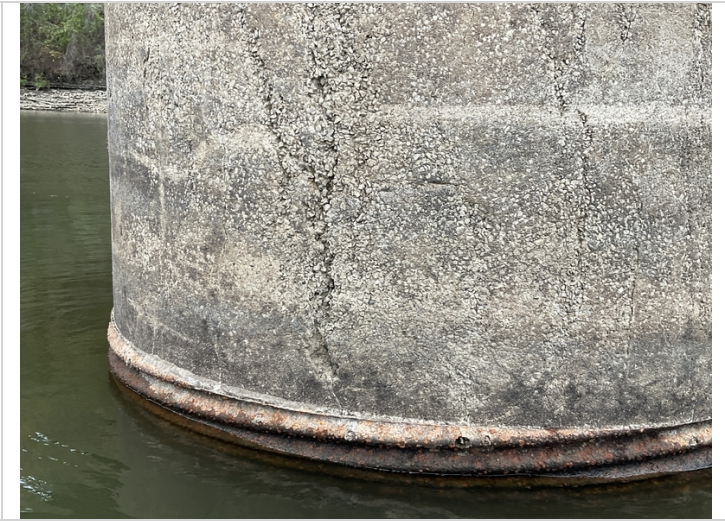
Bent 3, column 1-Honeycombing / concrete deterioration.
