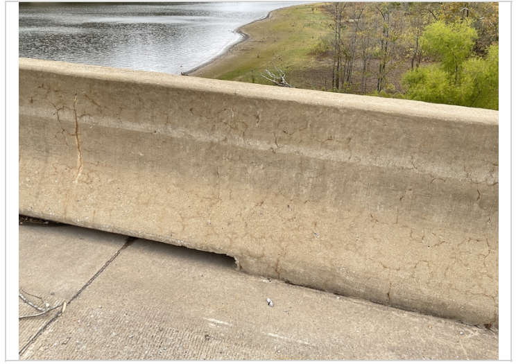
Mapcracking in parapets.
