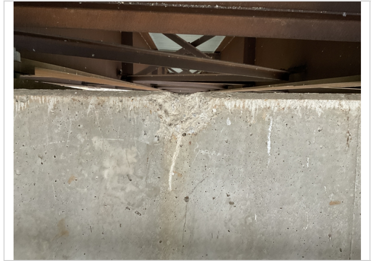
Bent 2 cap-Shallow 6" spall near centerline of cap.
