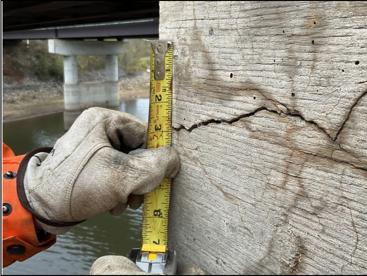
Bent # 4 cap, left end-1/8" wide mapcracking.
