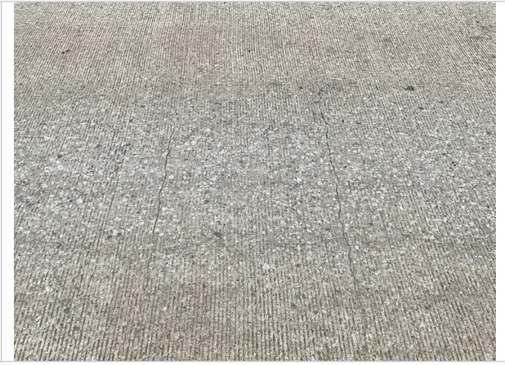
Span 2, left lane-Transverse cracking.
