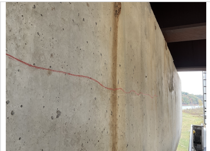
Bent 5 cap-Hairline horizontal crack.
