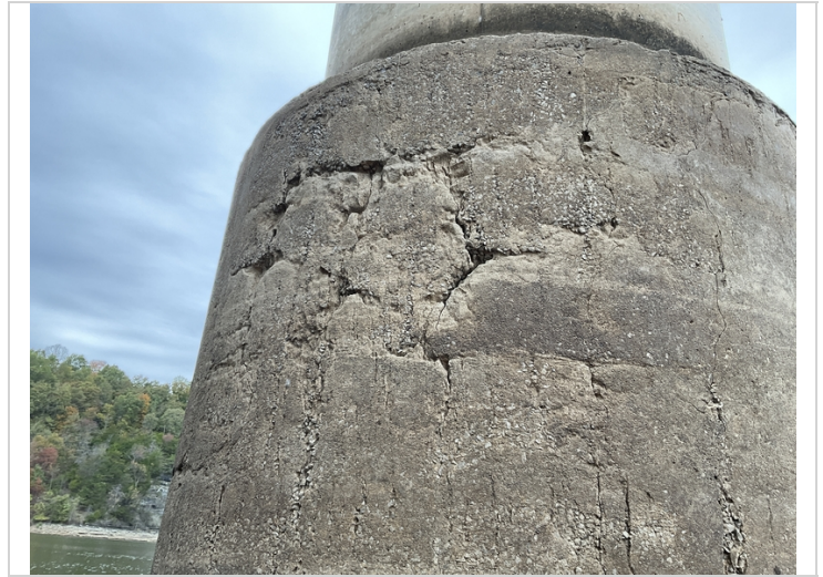
Honeycombing / concrete deterioration in drilled shaft.
