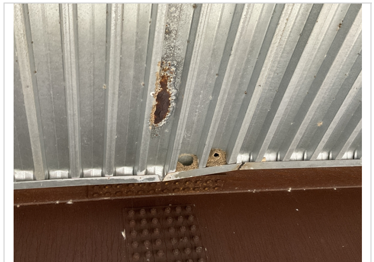
Span 2, bay 3-Corrosion in SIP forms.
