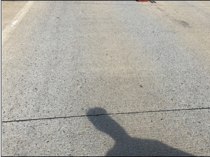
Longitudinal deck cracks.
