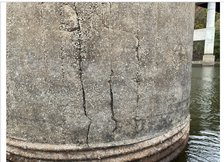
Bent 4, column 2-Concrete deterioration.
