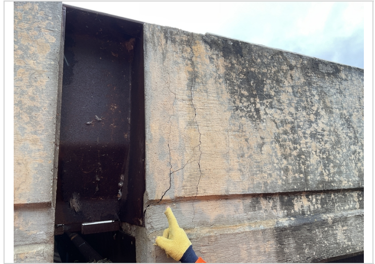
The right side of parapet in span # 1 at abutment # 1 has wide vertical and mapcracking on the exterior side.
