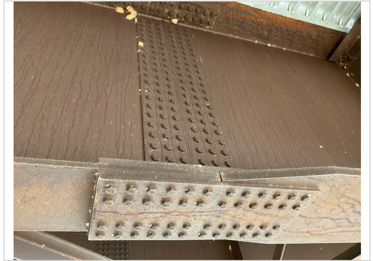
Typical of span 5 splice connections.
