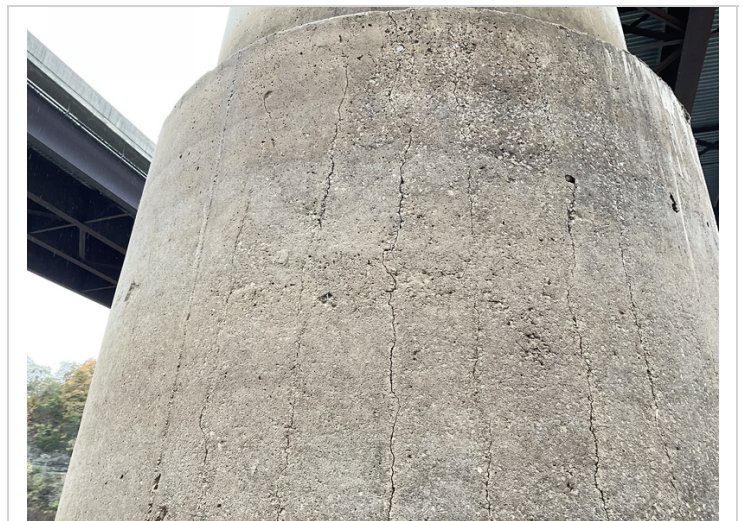
Bent 5, column 1-Vertical cracking.
