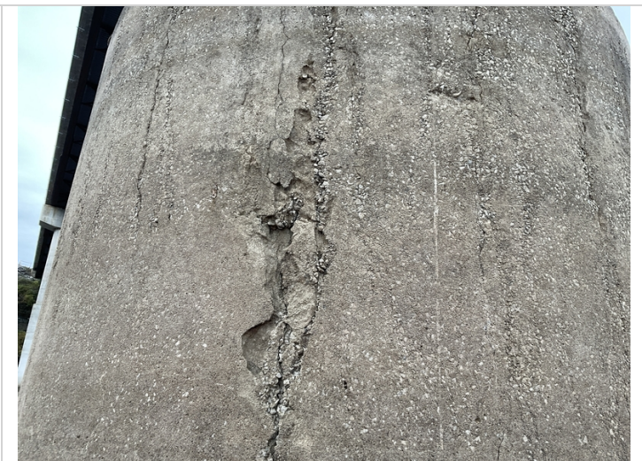
Bent 3, column 2-Honeycombing / concrete deterioration.
