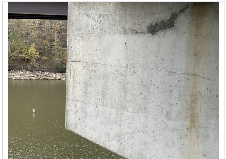
Bent 4 cap, right side-Horizontal cracking.
