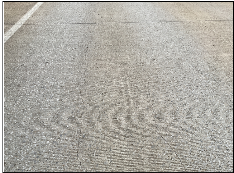
Span 2, left lane-Longitudinal cracking.
