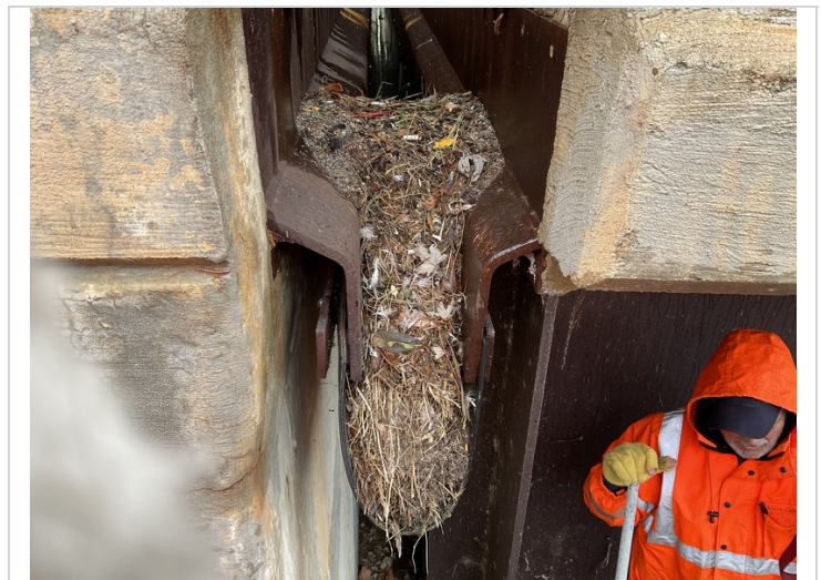
The expansion joint trough at abutment # 1 has debris accumulation on the right side.
