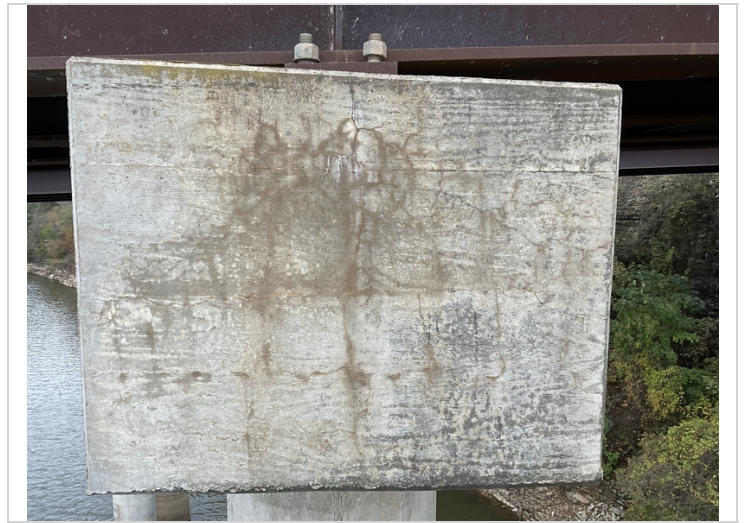
Bent 2 cap, left end-Mapcracking.
