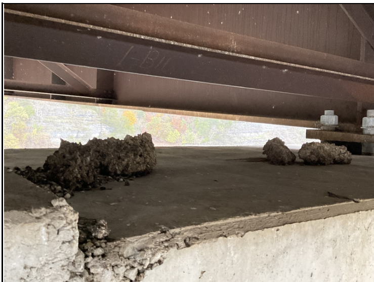
Pigeon droppings-Bent # 4 cap.
