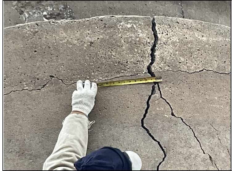
Bent # 4, column # 1-Wide vertical cracking with delaminated areas.
