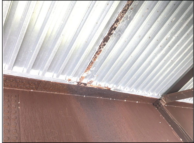
Span # 3. Girder # 3. Splice # 1. Corrosion.
