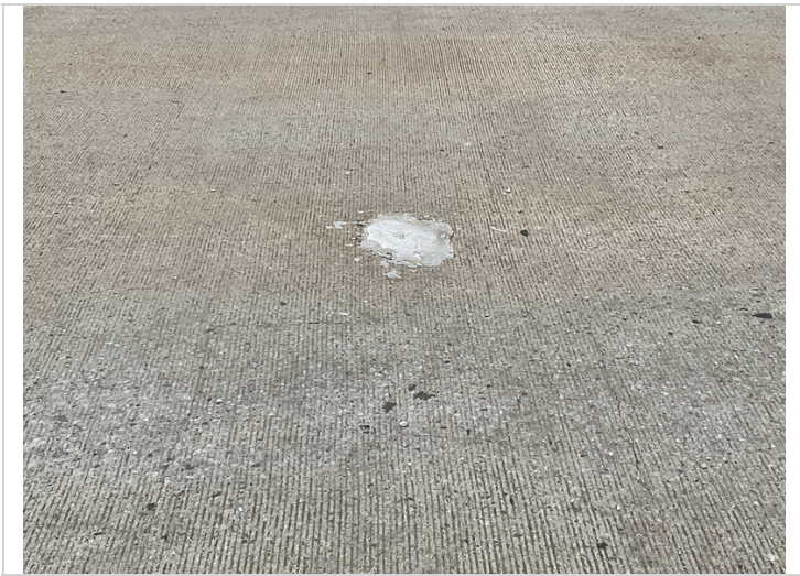
Span 3-Plowable pavement markers removed.
