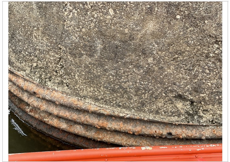
Bent 2, column 1-Concrete deterioration.
