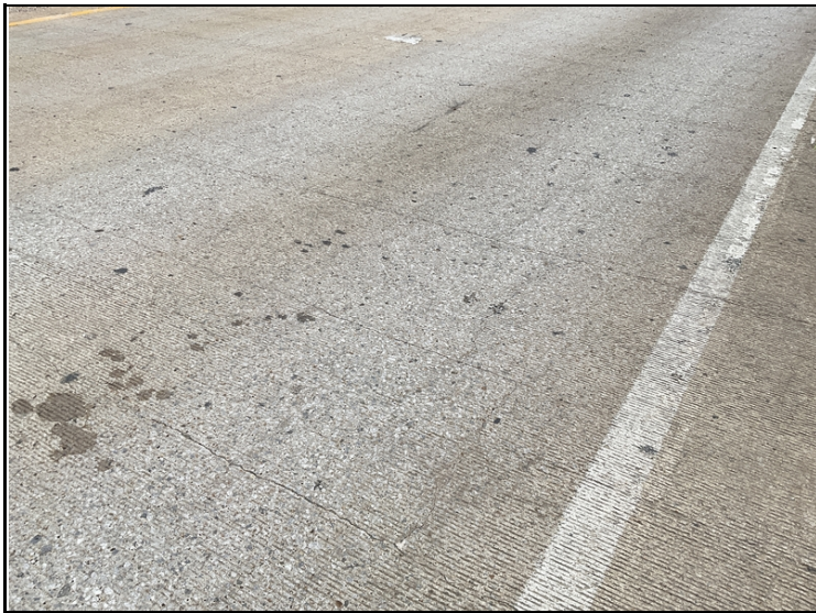
Span 4, left lane-Transverse deck cracking.
