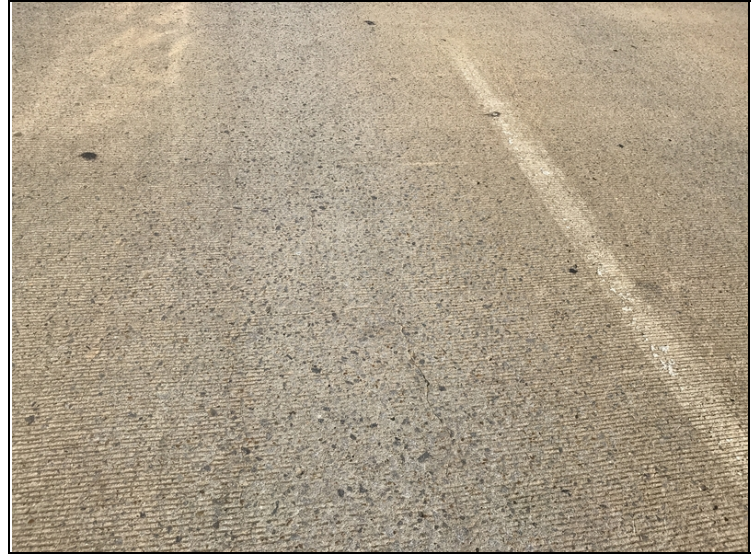
Sealable deck cracks.
