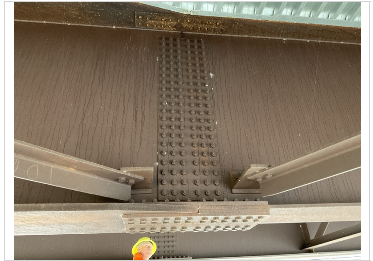
Span 4, girder 3-splice connection.
