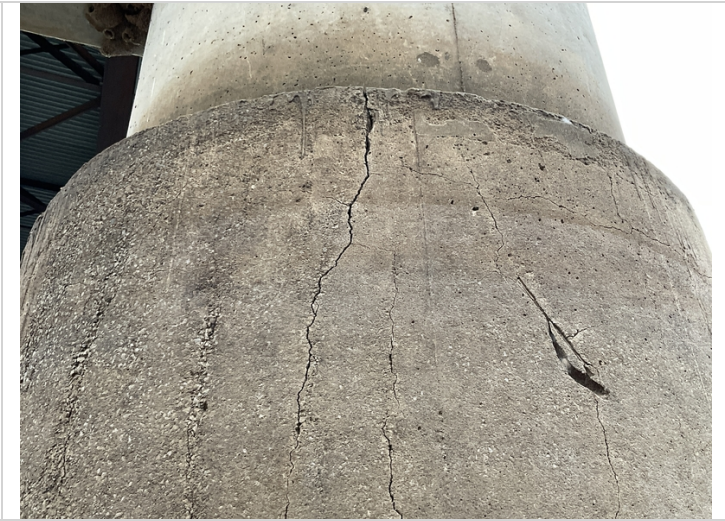
Bent # 5, column # 1-Wide vertical cracking.
