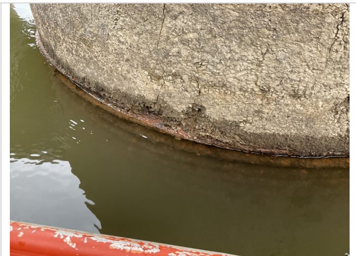
Bent 5, column 1-Concrete deterioration.
