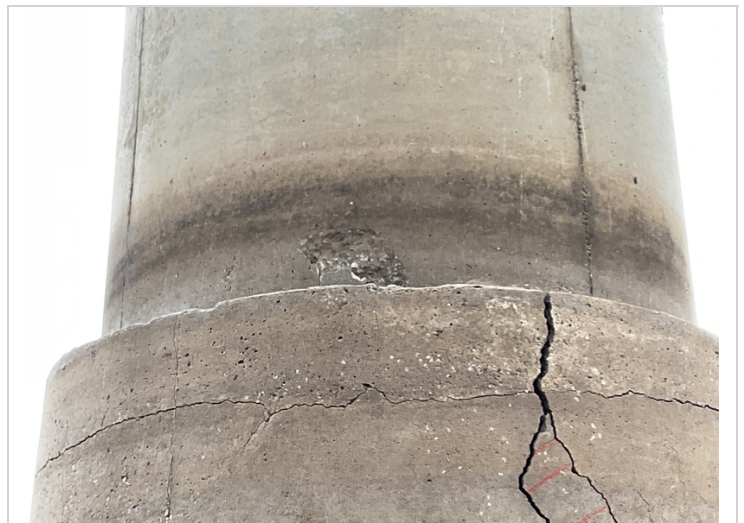
Bent 4, column 1-Wide vertical cracking shallow 10" spall.
