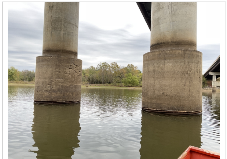
Bent 3 drilled shafts.
