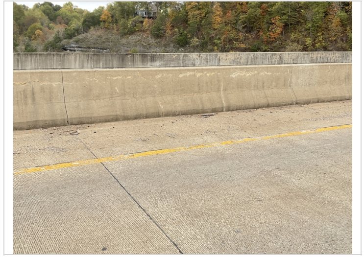
Cracking in right parapet.
