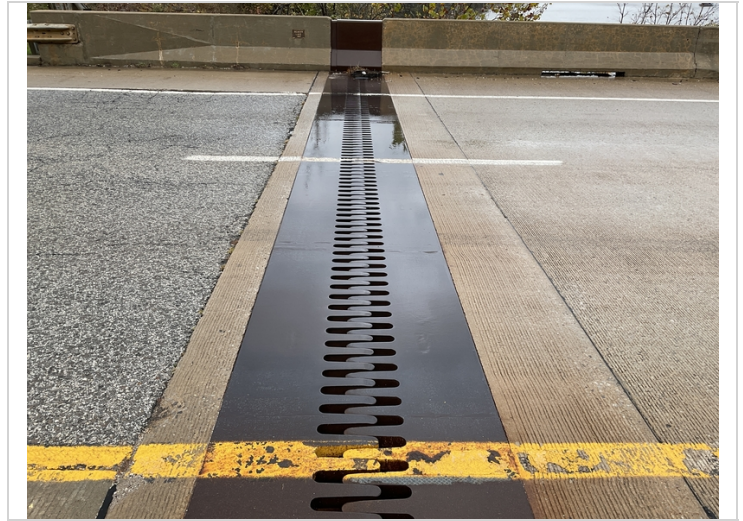
Abutment 1 finger joint assembly.
