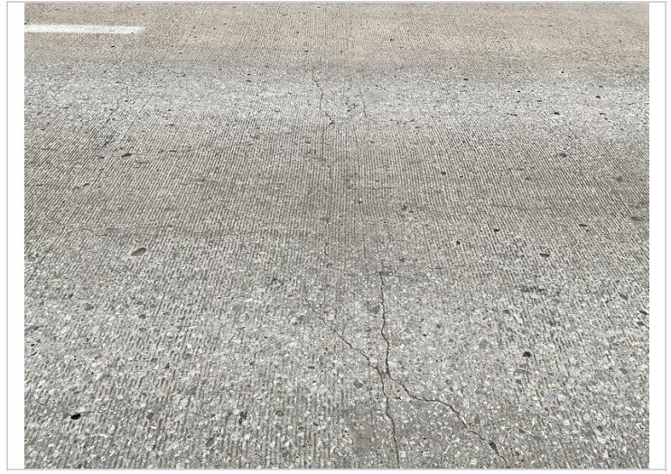
Span 5, left lane-Transverse cracking.
