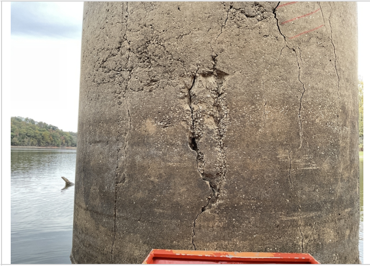
Bent 4, column 1-Concrete deterioration.
