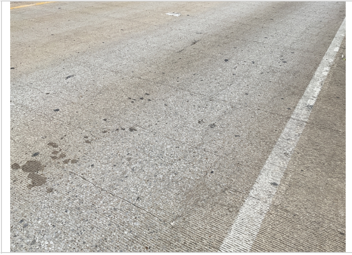
Span 4, left lane-Transverse deck cracking.
