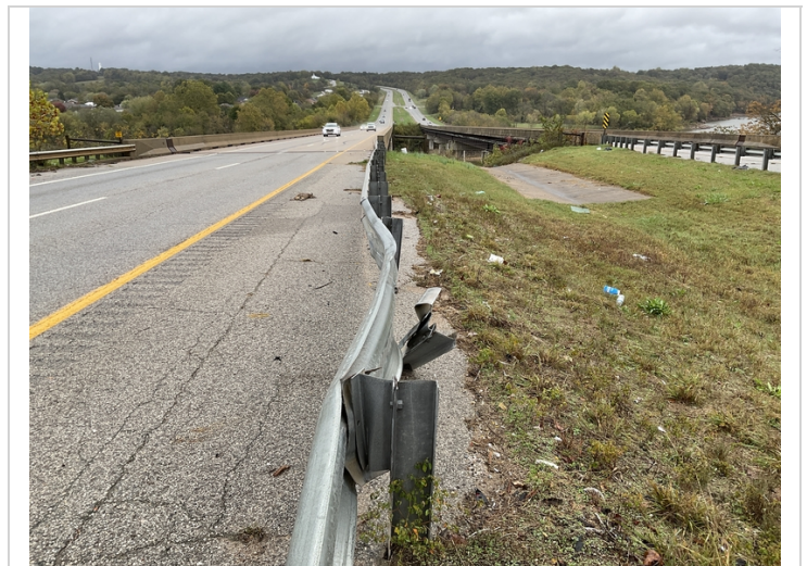
Collision damage to the Southwest approach railing has destroyed approximately 15' of the railing and two railing posts. The collision damage has created a "pocket" in the railing.
