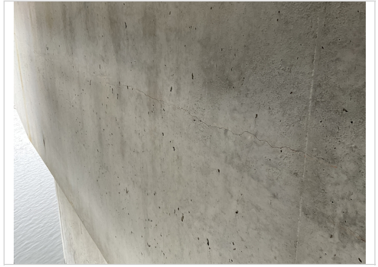
Bent 4 cap-Horizontal cracking.
