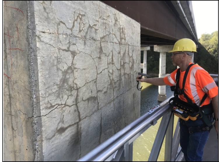
Left end of Bent # 4 cap sounds delaminated in areas.
