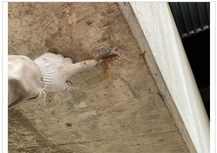
The left end of cap has a 3" spall in the undersurface with exposed reinforcing steel.
