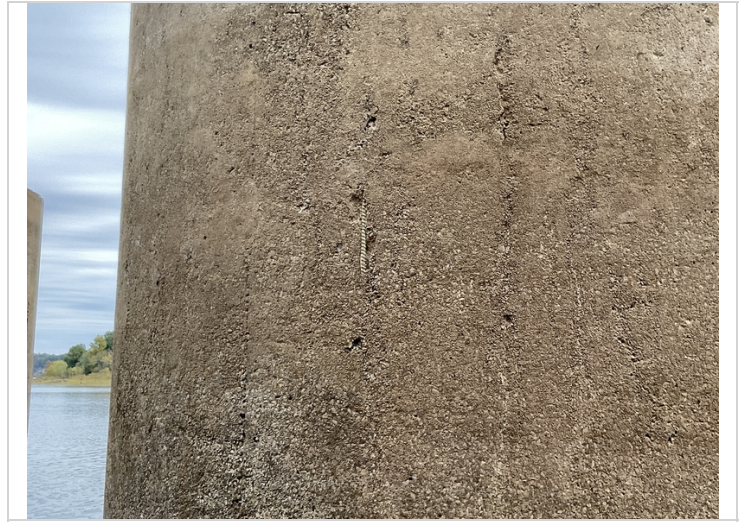
Bent 2, column 2-Exposed reinforcing steel.
