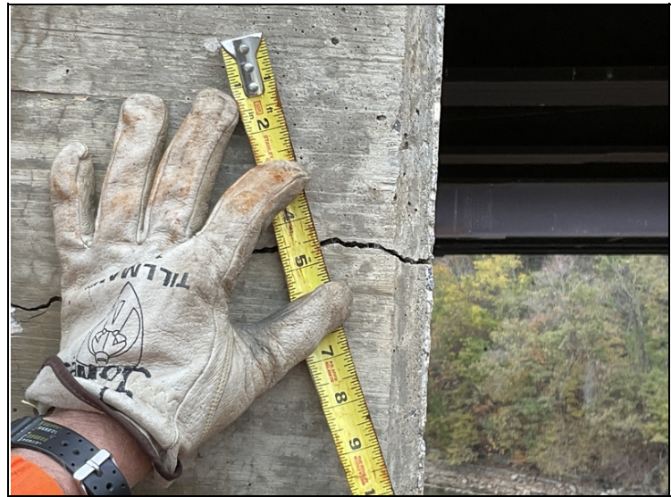
Bent # 3 cap-Left end-1/8" wide mapcracking.
