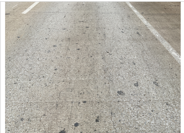
Span 5, left lane-Longitudinal cracking.
