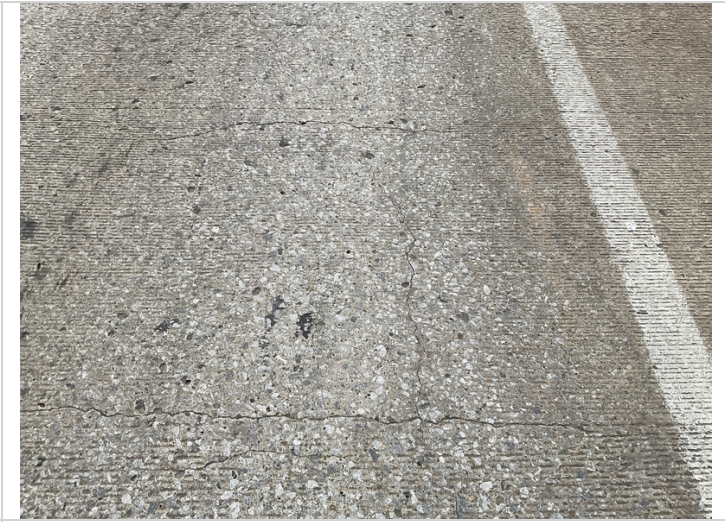
Span 5, left lane-Longitudinal and transverse cracking.
