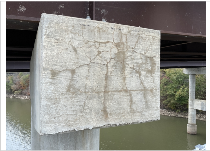
Bent 3 cap, left end-@Mapcracking.
