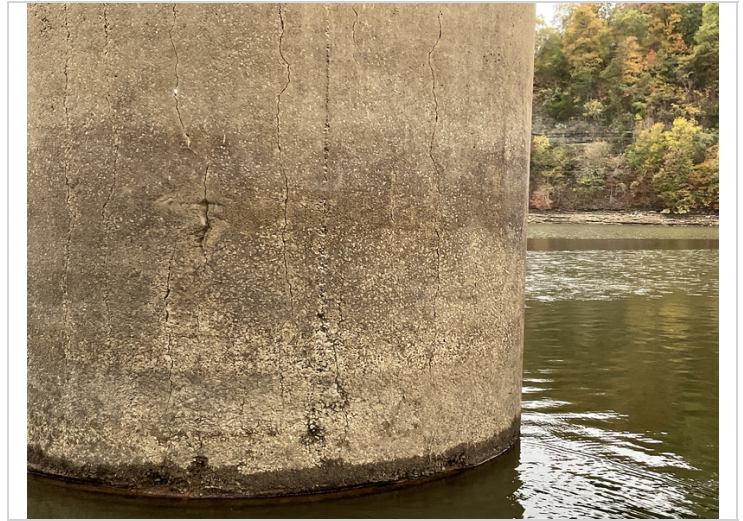
Bent 5, column 1-Vertical cracking.
