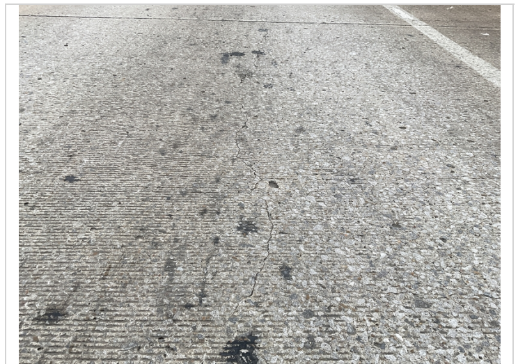
Span 5, left lane-Longitudinal cracking.
