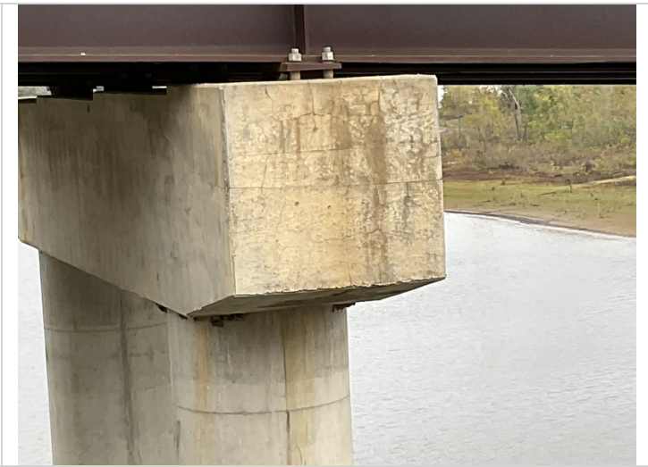
Bent 3, right end of cap has mapcracking.
