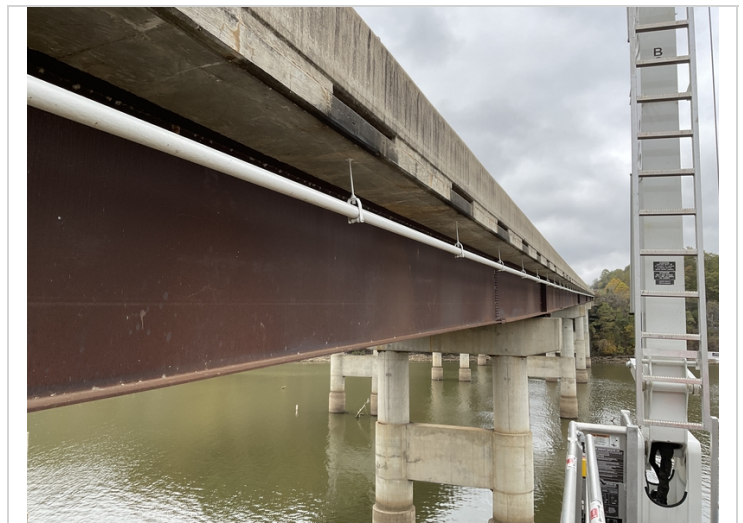
Utility attached to left side of deck.
