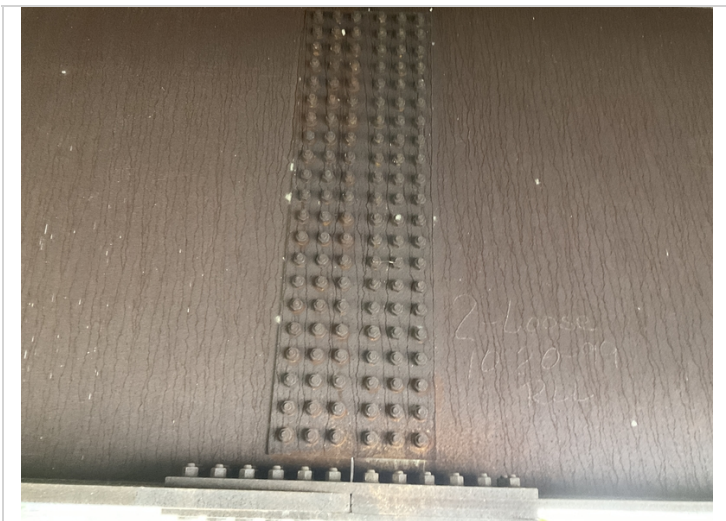
Typical of span 2 splice connections.
