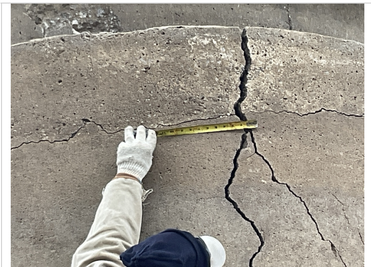
Bent 4, column 1-Wide vertical cracking with delaminated areas.
