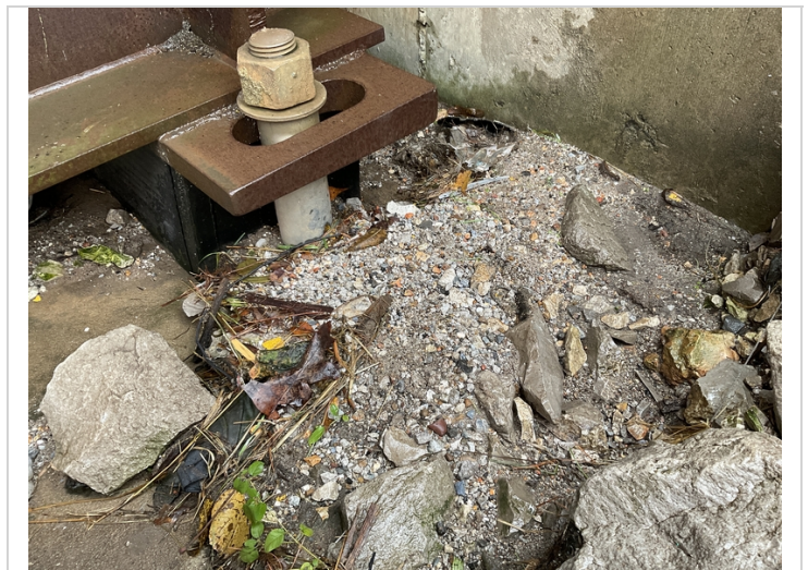
Abutment # 1 has dirt and debris accumulated against exterior bearings.
