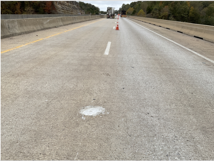
Plowable pavement markers removed.
