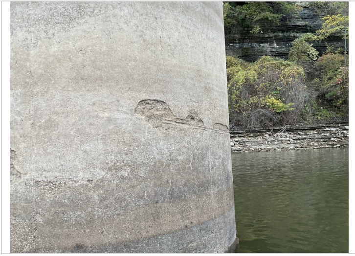
Bent 2, column 2-scaling
