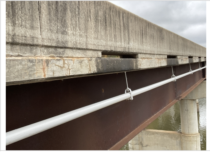
The exterior edges of the deck have mapcracking.
