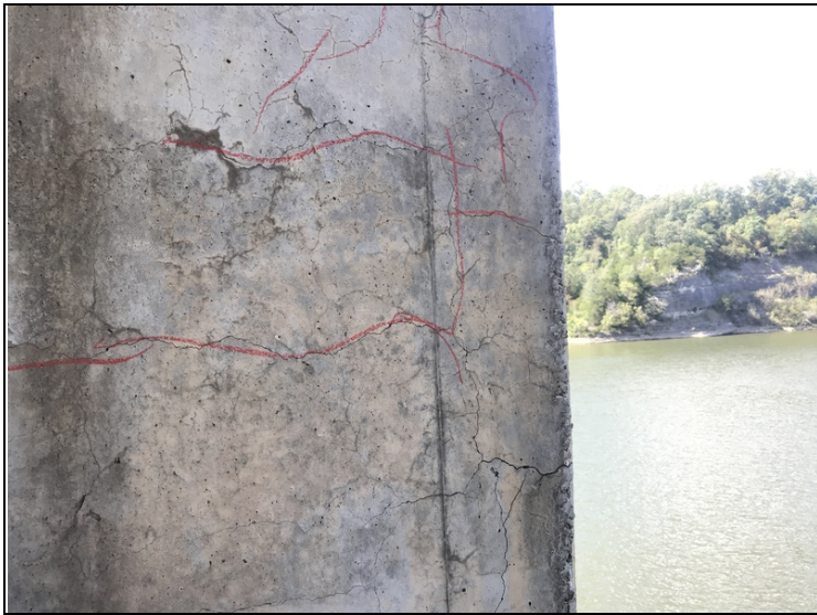
Bent # 4 cap, left side map cracking.
