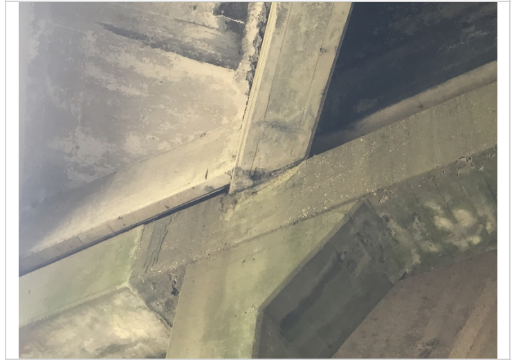
Span #2, girder #2 spalling in the bearing area of the girder.
