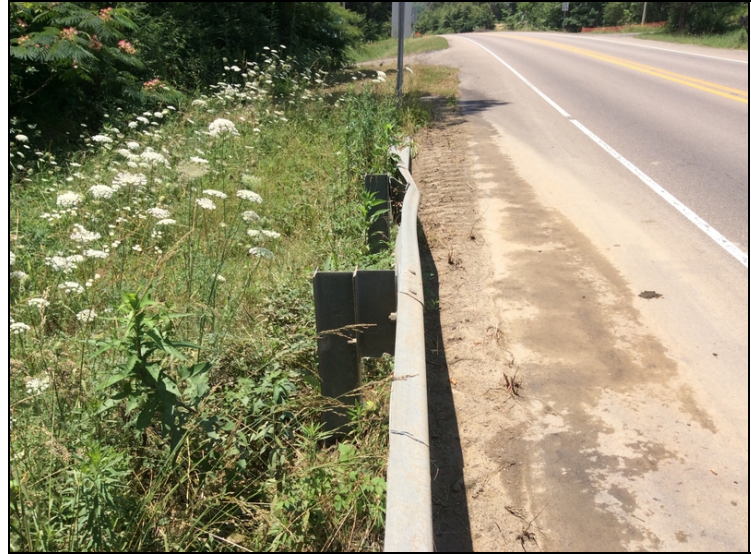
The Southeast approach guardrail has minor collision damage.
