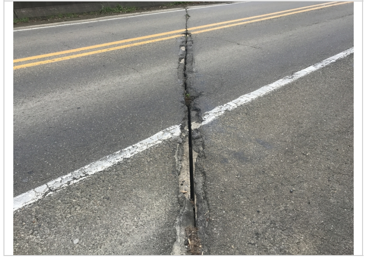
Bent #2 asphalt breaking apart over the deck joint.
