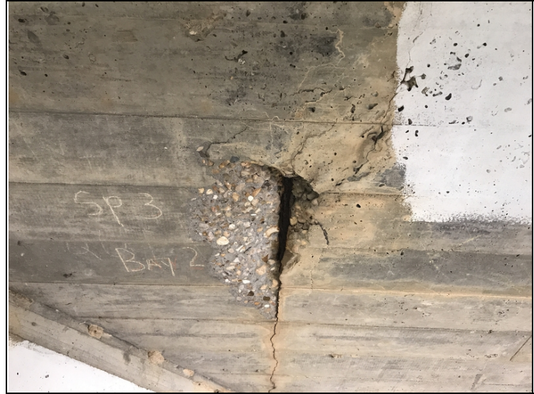
Span # 3, bay # 2-Spalling with exposed reinforcing steel in undersurface of deck at abutment # 2.
