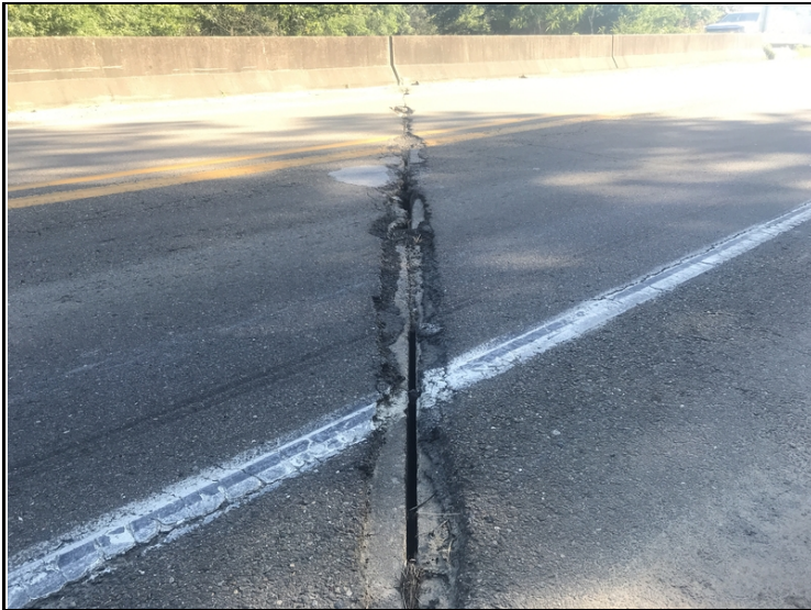
Bent # 3 expansion joint-Asphalt breaking up over expansion joints with potholes forming in driving surface.
