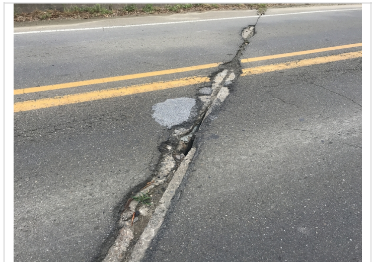
Span #2, Bent #3 with spalling adjacent to the deck joint in the top flange.
