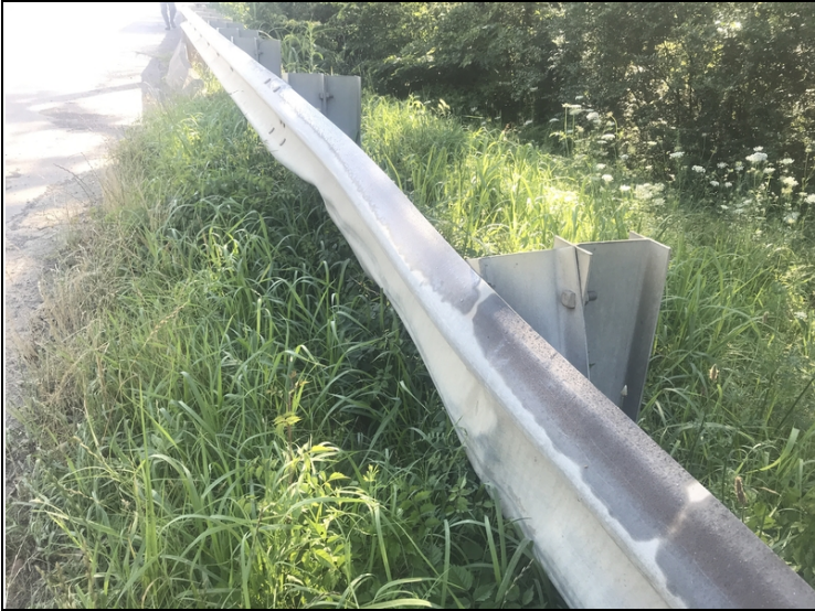
Southeast approach railing-Collision damage.
