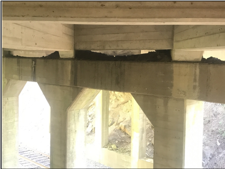
Bent # 2 cap-Dirt and debris accumulation.
