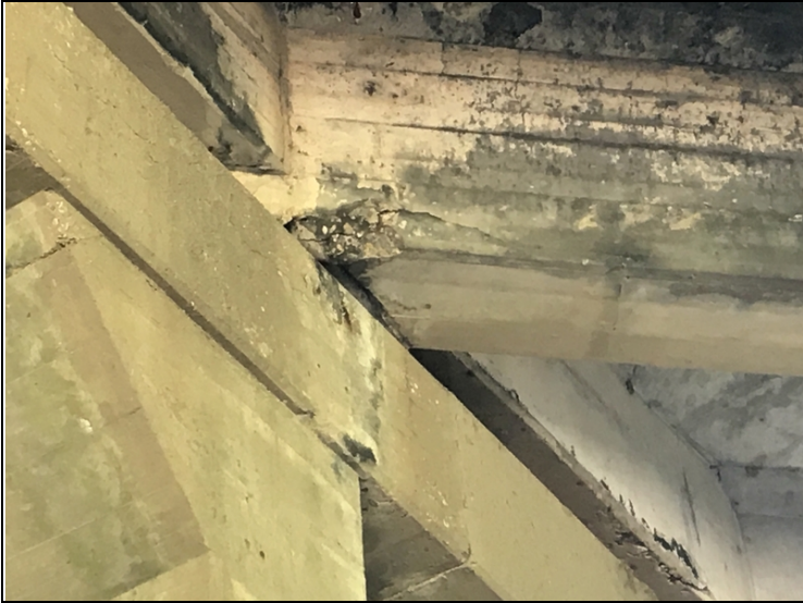
Span # 2, girder # 4 at bent # 3-Spalling with diagonal cracking.
