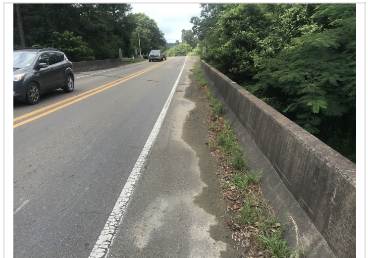
Span #2, the Lt gutter with potholes and delaminated asphalt.
