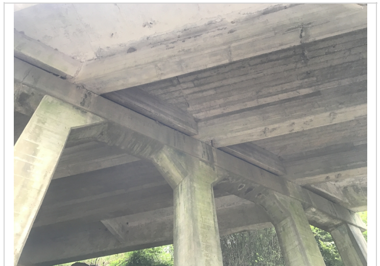
Span #2, bent #2 girders # 2, 3 & 4 has shallow spalling adjacent to bent #2.
