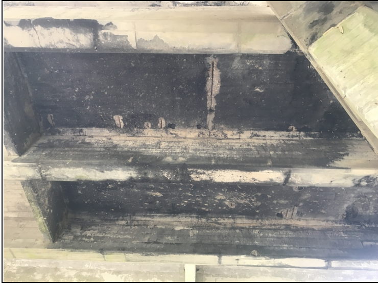
Span #2, bays # 2 & 3 spalling with exposed reinforcing steel on the undersurface of the top flange.
