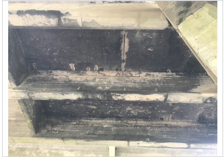
Span #2, bays # 2 & 3 spalling with exposed reinforcing steel on the undersurface of the top flange.
