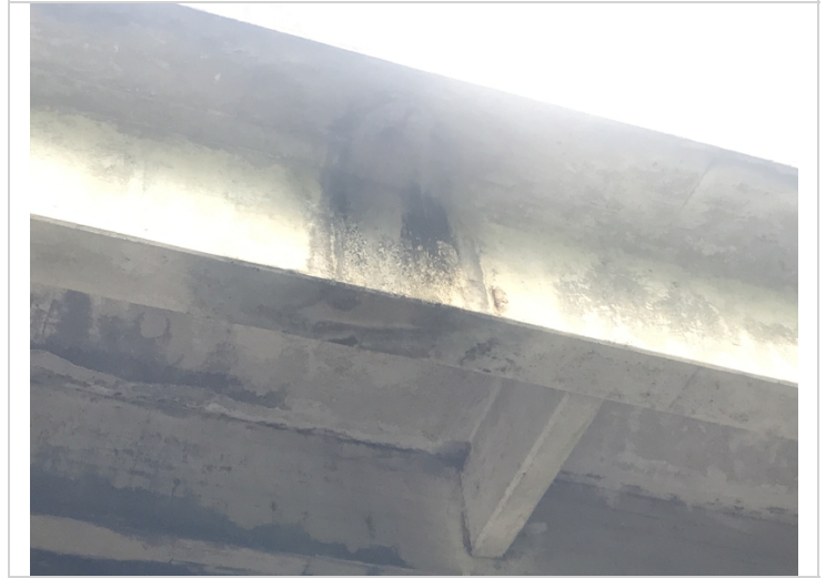
Span #2 girder #1 exterior spalling with exposed reinforcing steel below the deck drain.
