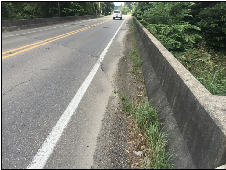
Dirt and vegetation in the gutters.
