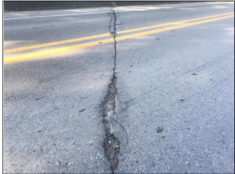
Bent # 2-Asphalt breaking up over expansion joint.
