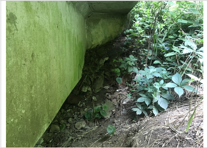
Abutment #1, beam #1 dirt accumulation.
