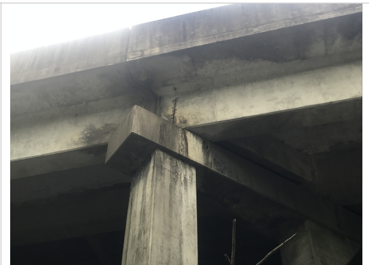
Span #2, girder #5 exterior face spalling with exposed reinforcing steel.
