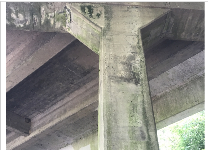
Span #2, bent #3 column #3 vertical cracking.
