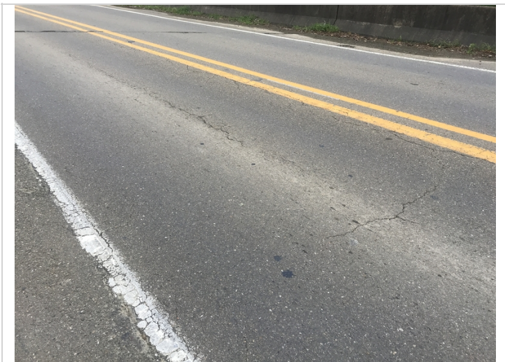
Typical cracking in the asphalt wearing surface of the deck.
