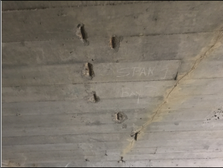
Span # 1, bay # 3-Shallow spalling with exposed reinforcing steel near abutment # 1.
