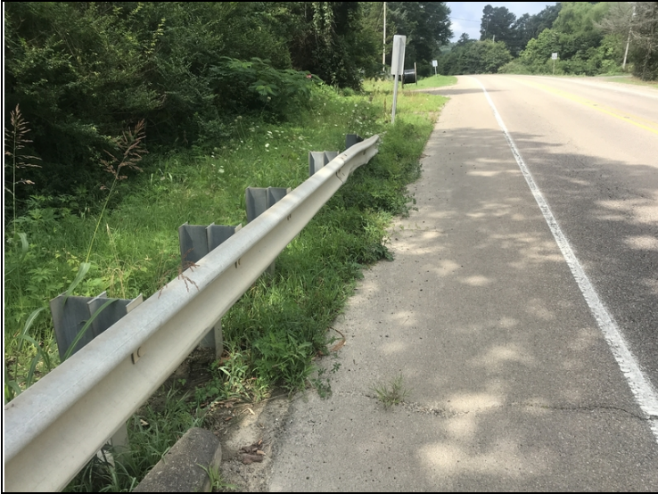
Approach guardrail with minor collision damage at the southeast approach.
