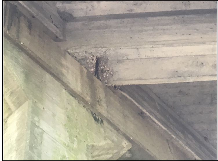
Span # 2, girder # 3 adjacent to bent # 2-Spalling with exposed reinforcing steel in undersurface.
