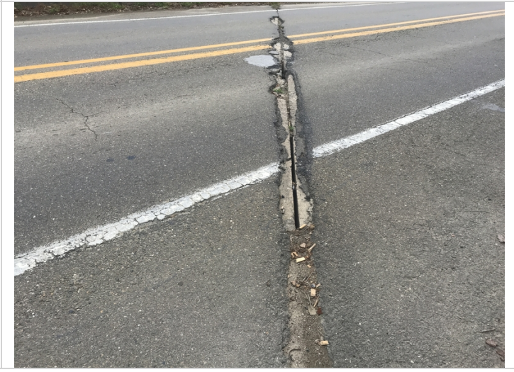
Bent #3 asphalt breaking apart over the deck joint.
