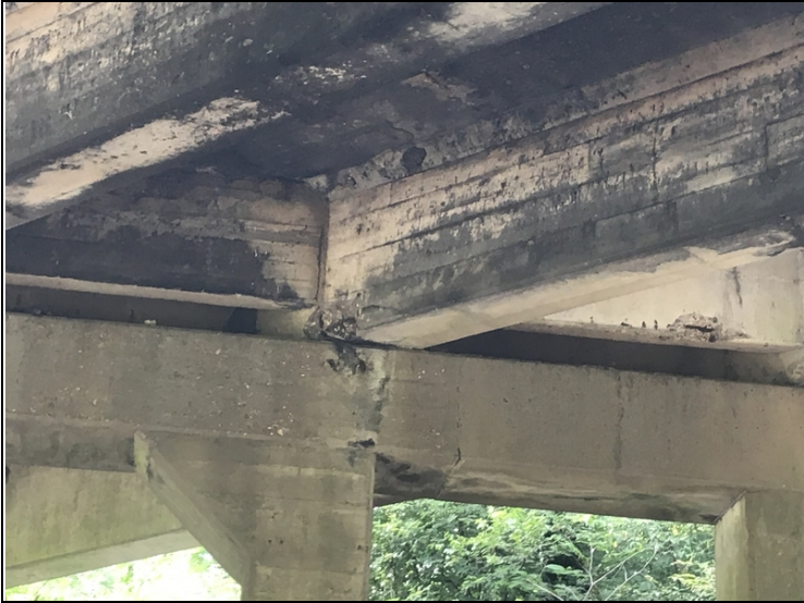
Span #2, girder # 4 spalling with exposed reinforcing steel adjacent to bent #4.
