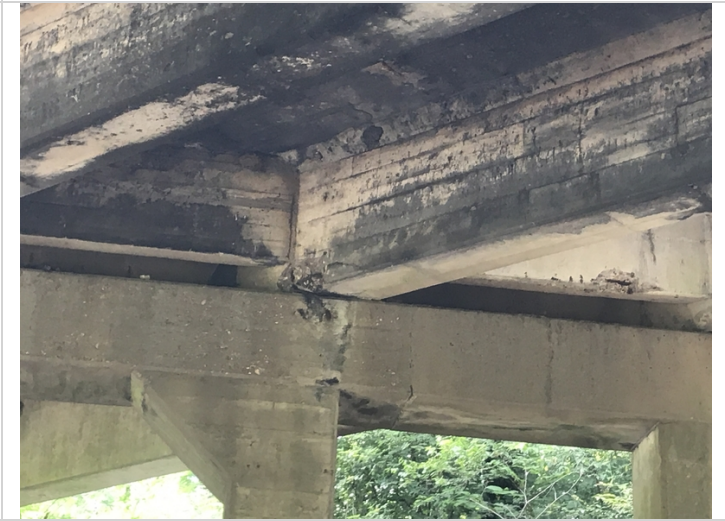
Span #2, girder # 4 spalling with exposed reinforcing steel adjacent to bent #4.
