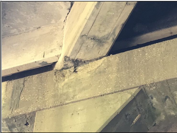
Bent # 3 cap-Spalling with exposed reinforcing steel under girder # 2.
