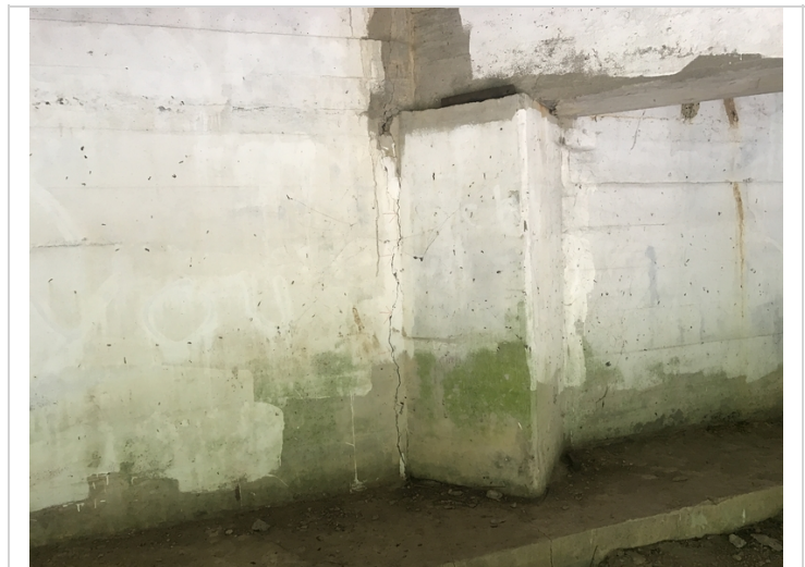
Abutment #2 with 1/8" wide cracking adjacent to girder #3.
