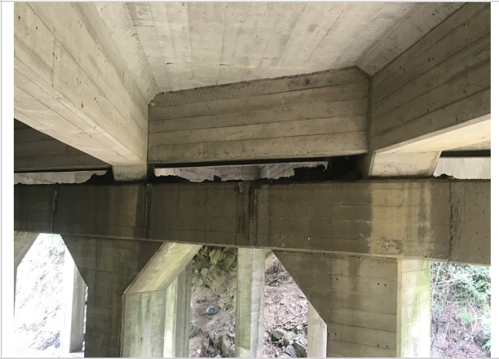
Span #1, girders # 3 & 4 cracking and delaminated areas in the bearing areas.
