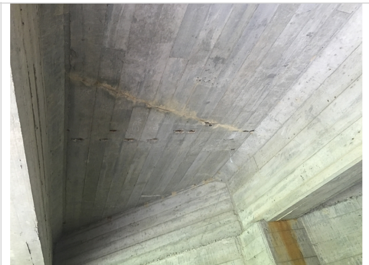
Span #1 bay #3 adjacent to abutment #1 spalling with exposed reinforcing steel.
