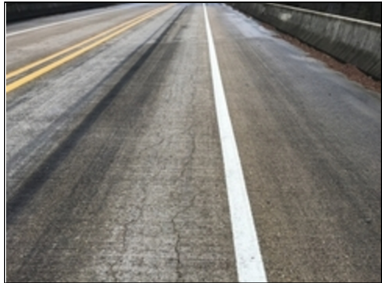
The driving surface of the deck has a few random short duration sealable cracks.
