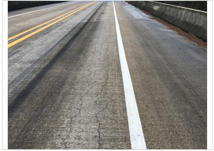
Sealable deck cracking.
