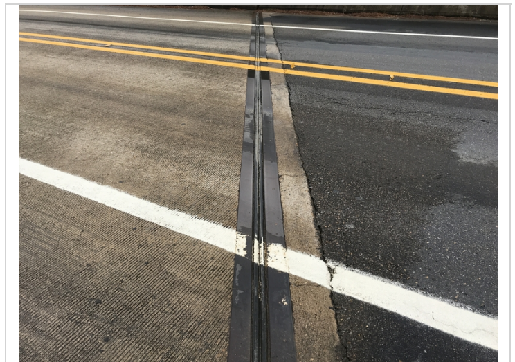
Bent # 1 compression joint seal.
