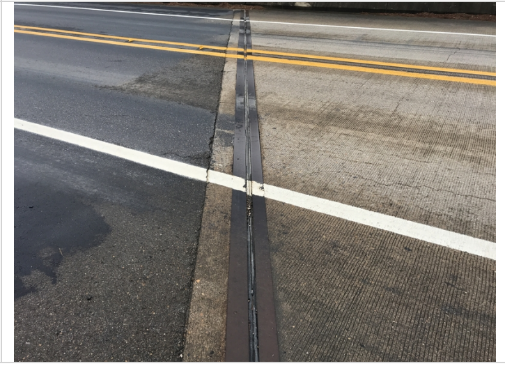
Bent # 2 compression joint seal.
