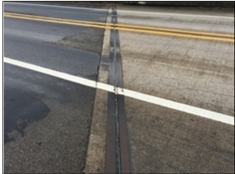
Compression joint seal at the North bridge end is losing its adhesion and is leaking through to the substructure.
