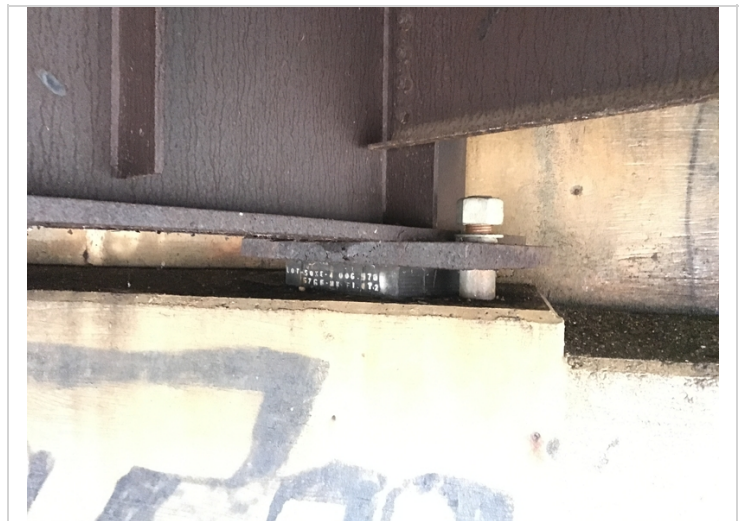
Bent 2 Bearing 4 active corrosion with layers of flaking rust.
