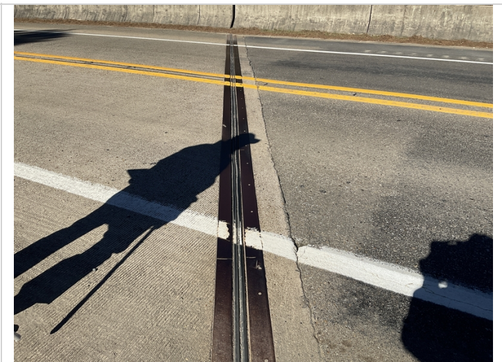
Expansion joint seal over Bent # 1.
