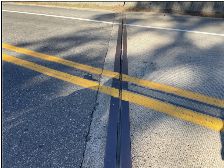
Expansion joint seal over Bent # 2.
