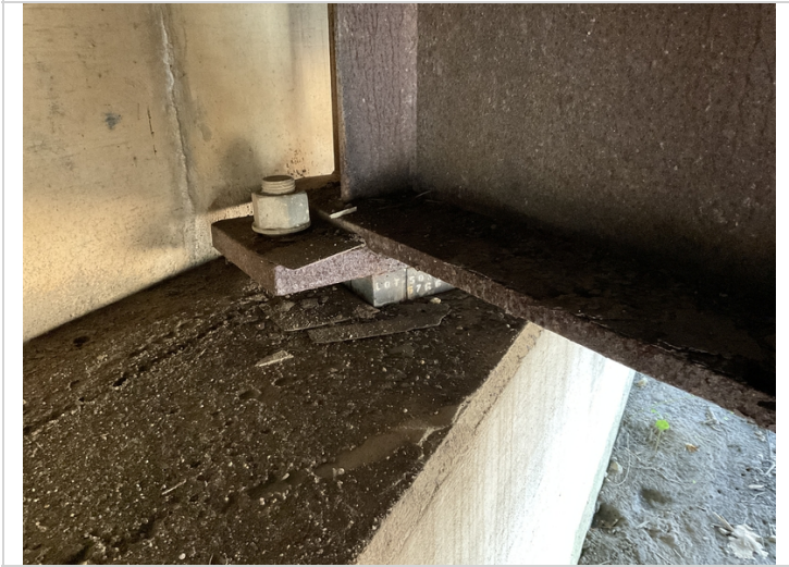
Active corrosion with flaking rust. External loading plate of Bent # 2. Girder # 4 bearing.
