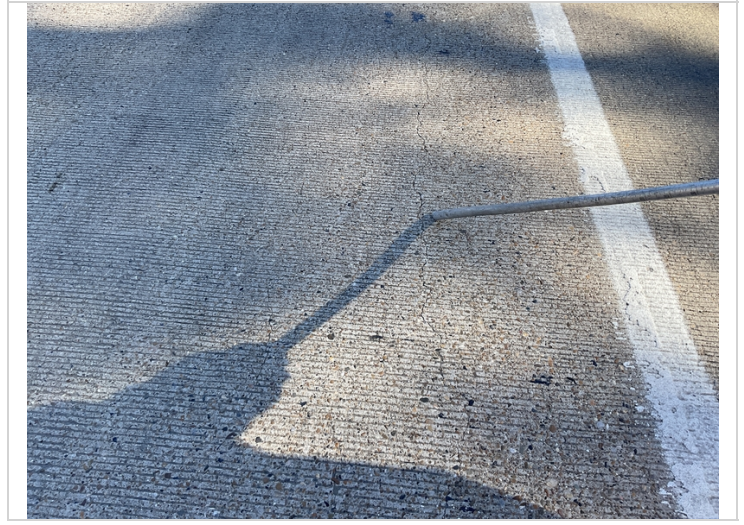
Sealable Longitudinal cracking in the deck.
