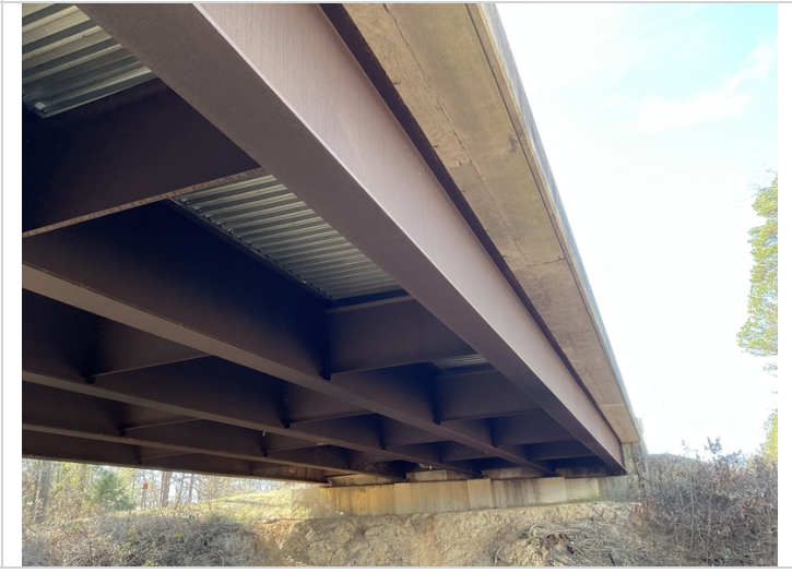
Deck soffit. Right overhang. Typical.
