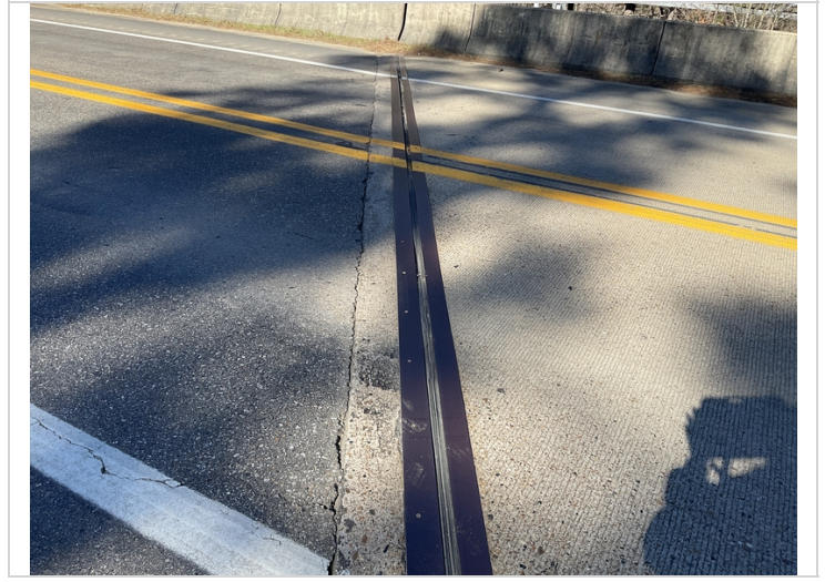
Expansion joint seal over Bent # 2.
