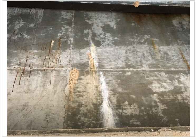
Bent # 1 backwall vertical cracking with efflorescence buildup.
