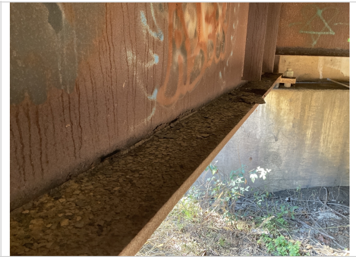
Photo of Girder # 1. Active corrosion.
