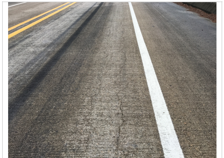
Sealable deck cracking.
