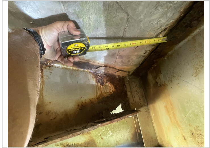
Span 3, Bent 4. Beam 5 - Top flange of Beam has knife edge section loss and reduced in width by 1".
