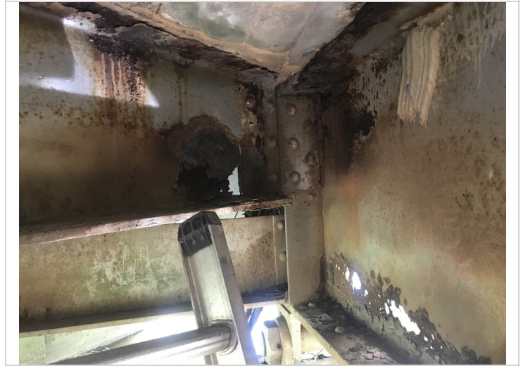
Bent # 5 bay # 4 hole in the diaphragm.
