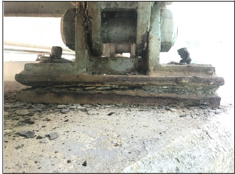
Pack rust in bearing device restricting movement.
