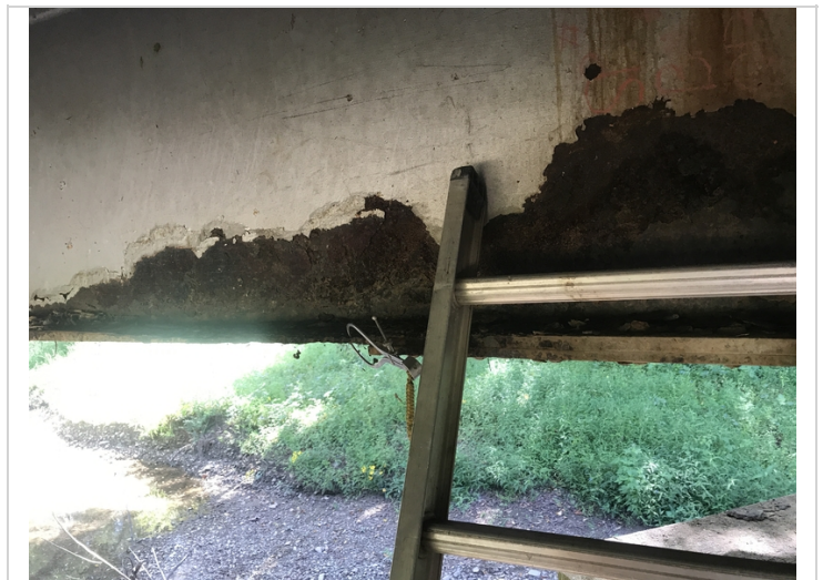
Span # 4, Bent #4 beam #5 with up to 1/2" section loss to the bottom flange.
