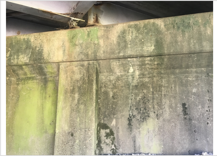
Bent # 3 cap cracking near the centerline.
