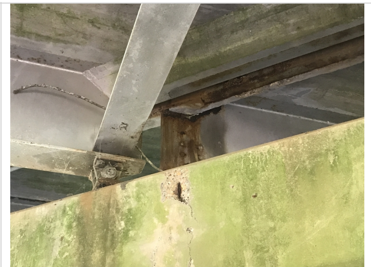
Span #6, Bent #6 beam #2 active corrosion with large hole in the web around the expansion dam.
