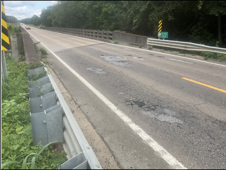
South approach roadway. Patched pot holes.
