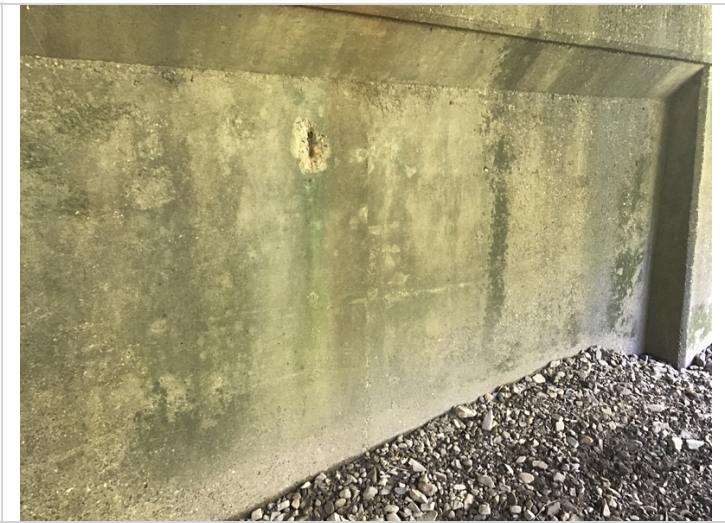
Span # 2 Bent # 2 vertical crack and spalling with exposed reinforcing steel.
