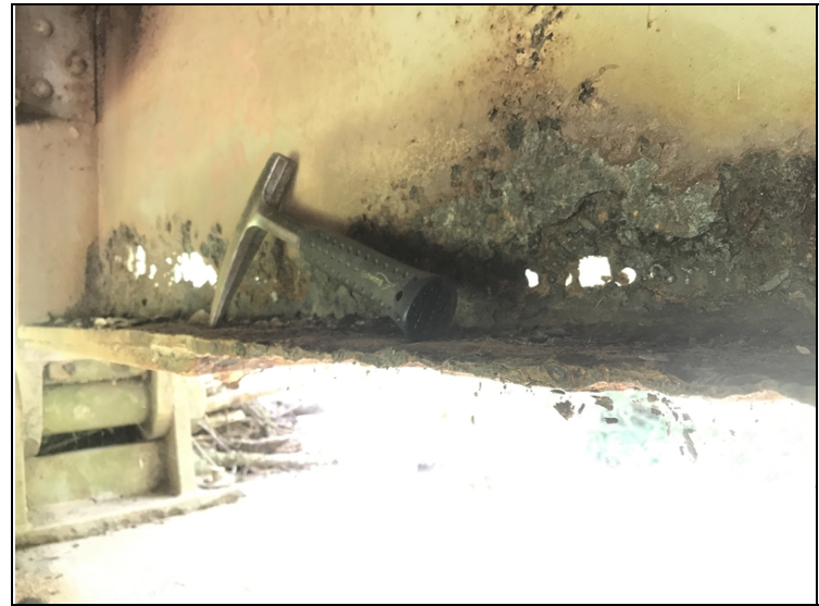
Sp #4, beam #5 at bent #5- Holes rusted through web and section loss to bottom flange.
