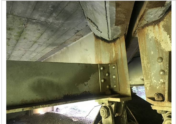
Span # 2, Bent # 2 beam # 1 with a 4" long x 1/2" wide hole through the web at the expansion dam.
