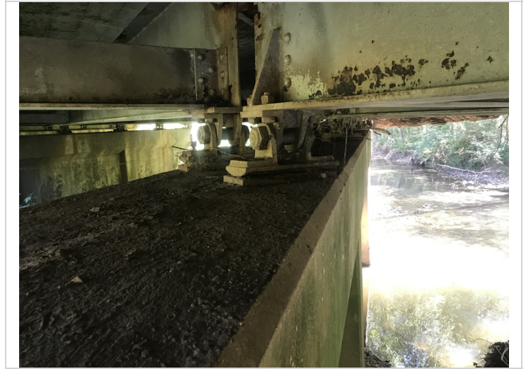
Bent # 6 with missing anchor bolts.
