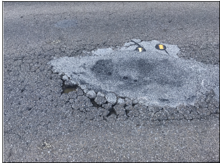
South approach roadway - Pothole forming.
