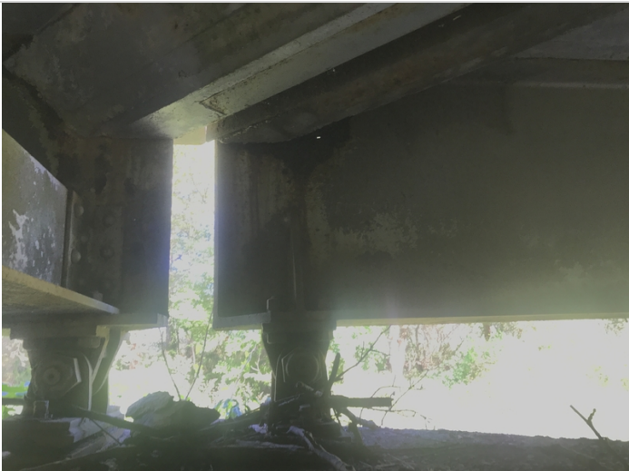
Span # 2, Bent # 2 beam # 1 with a 1/2" hole through the web.
