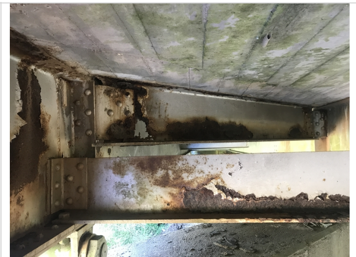
Span # 4, bay # 1 active corrosion and a hole through the web of the diaphragm adjacent to beam # 1.
