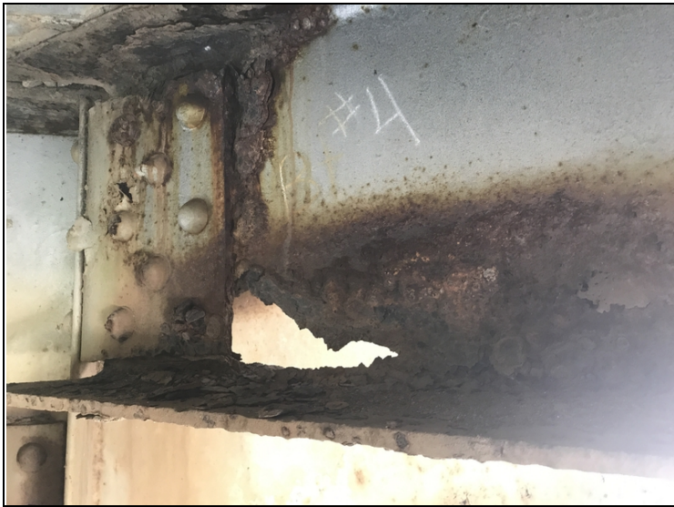
Section loss to beam web.
