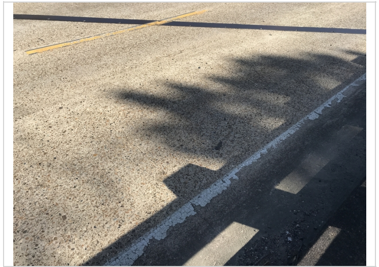
Moderate width sealable deck cracking.
