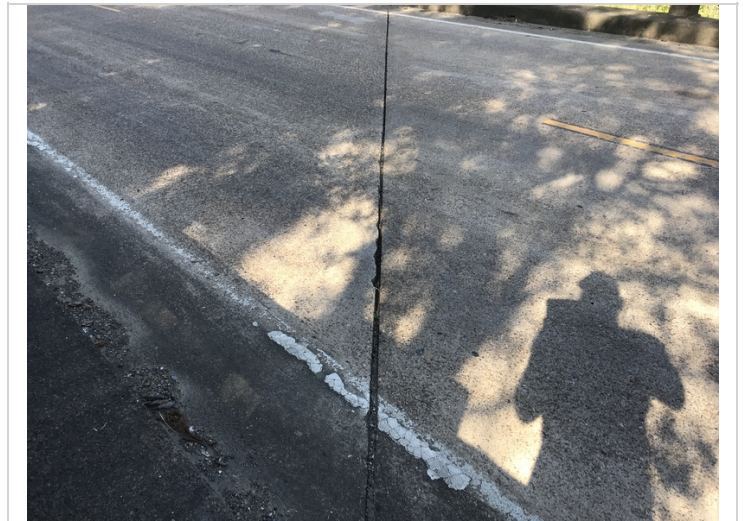
Bent # 4 missing joint sealant.
