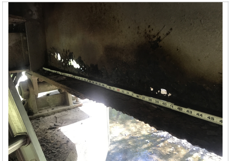
Span # 4, Bent # 5, beam #5 active corrosion with layers of flaking rust and large holes in the base of the web.
