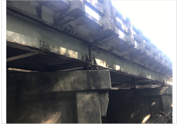
Spans # 2 & 3 Rt spalling with exposed reinforcing steel.
