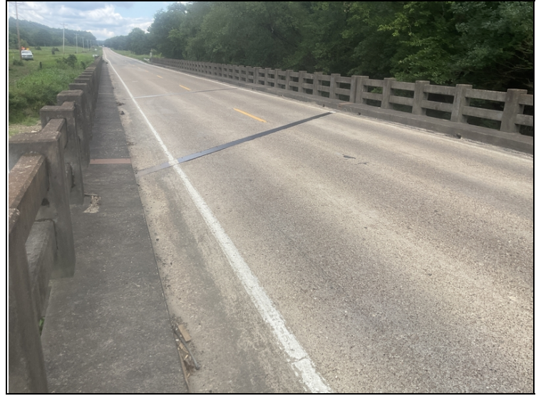
Sliding plate. Typical.
