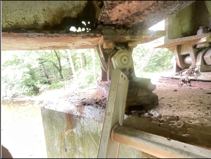
Bearing - Span 6, Bent 6. Beam 5. Active corrosion with pack rust.
