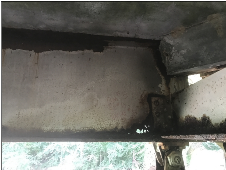
Bent #6, Span #6 Beam #5 with holes through the web. No visible cracks.
