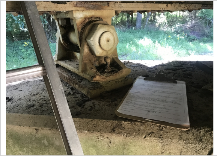
Bearings have active corrosion and layers of flaking rust.
