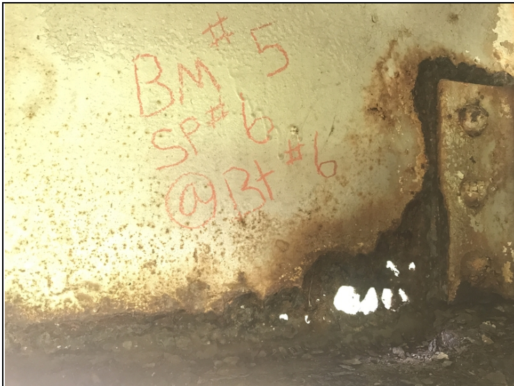
Sp #6, Beam #5 at bent #6-Hole rusted through web.
