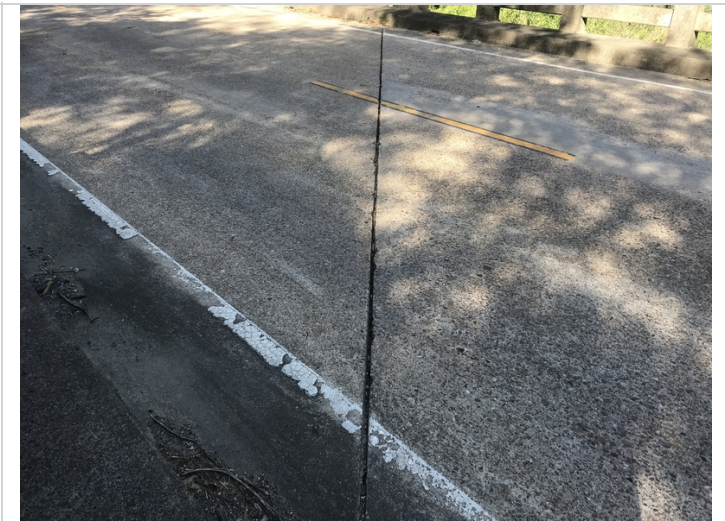
Bent # 5 missing joint sealant.
