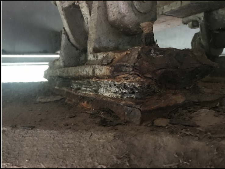
Pack rust in bearing device restricting movement.
