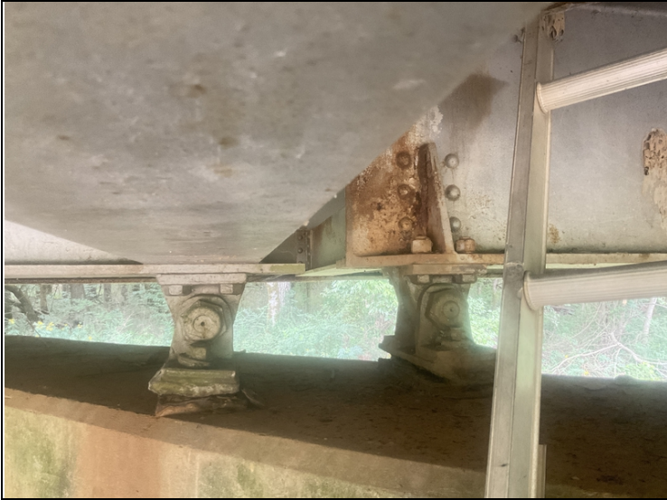
Bent 3, Beam 4 bearing corrosion.
