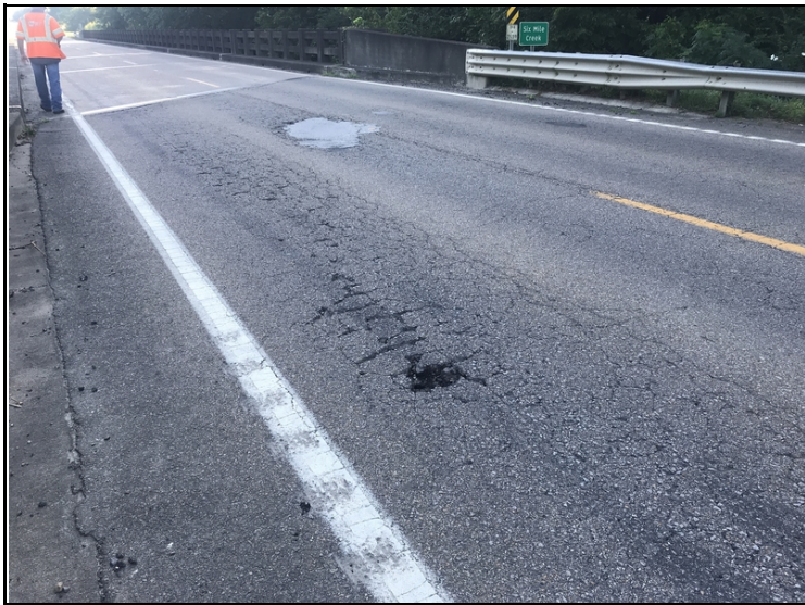
South approach roadway - Pothole forming.
