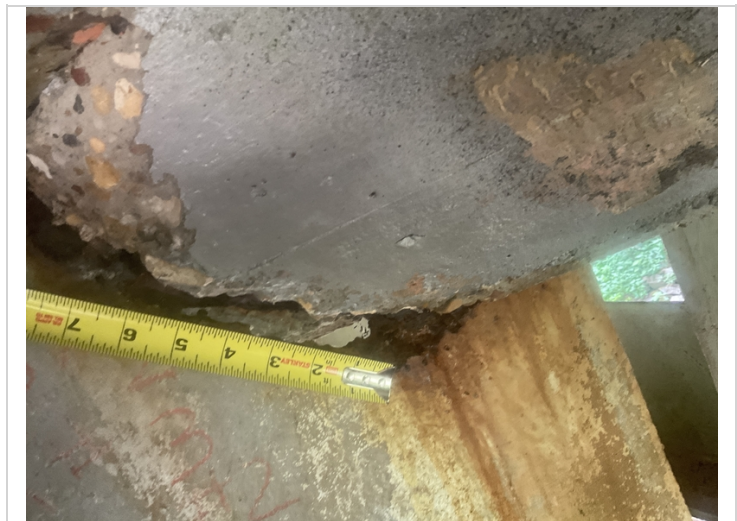
Span 2 over Bent 2. A 5" long hole in the web of beam at the expansion dam juncture.
