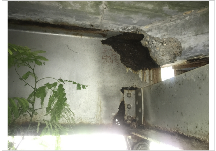
Span # 2, Bent # 3 beam # 1 with a 2" area of holes through the base of the web at the diaphragm connection.
