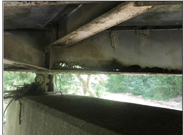
Bent #5, Span #4 Beam #5 with a 4' long section with holes in the base of the webs.
