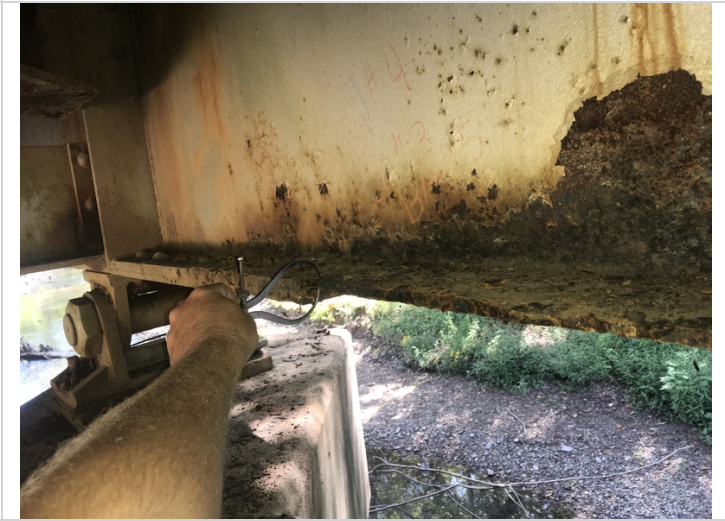
Span #3, Bent # 4 Beam #5 active corrosion with layers of flaking rust and up to 3/8" section loss adjacent to the splice plate.
