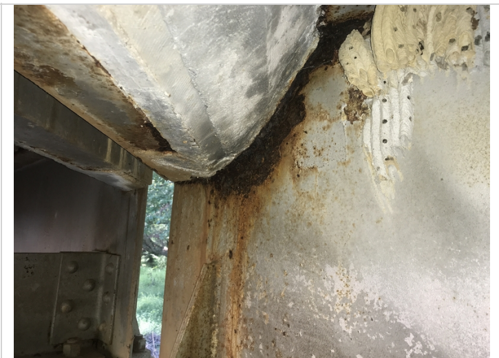
Span # 2, Bent # 3 beam # 5 with up to 7/16" section loss to the web at the expansion dam.
