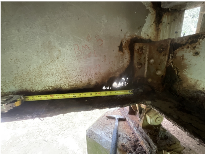
Span 6, Bent 6. Beam 5. Active corrosion with holes rusted through the base of web adjacent to the diaphragm.
