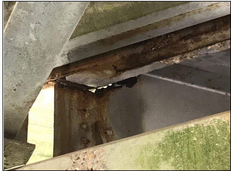
Holes rusted through upper portion of web adjacent to the deck haunch.
