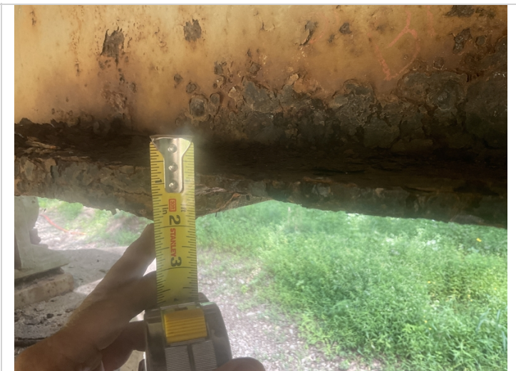
Span 3, Bent 4. Beam 5 - Bottom flange is reduced to 5/16" adjacent to the lower cover plate.
