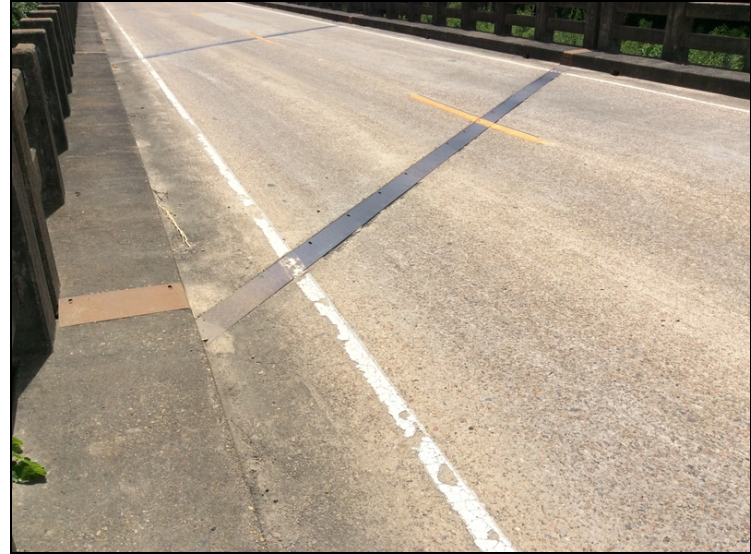
Expansion joint over Bent 7
