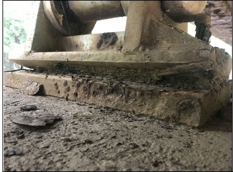
Pack rust in bearing device restricting movement.
