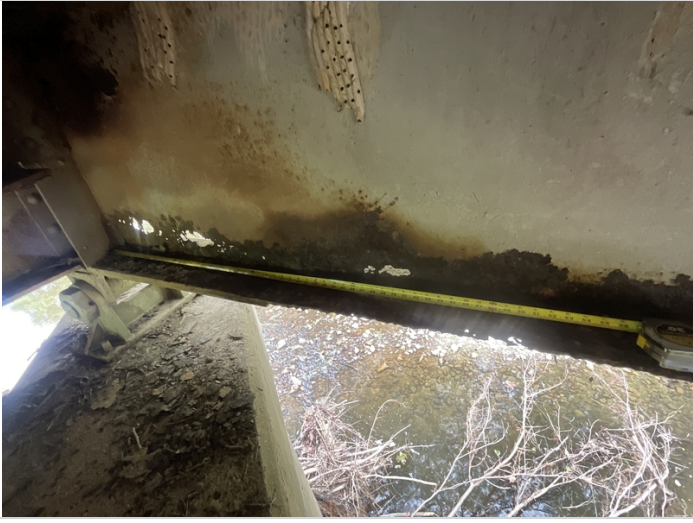
Span 4. Bent 5. Beam 5. Holes rusted through the base of web and bottom flange.
