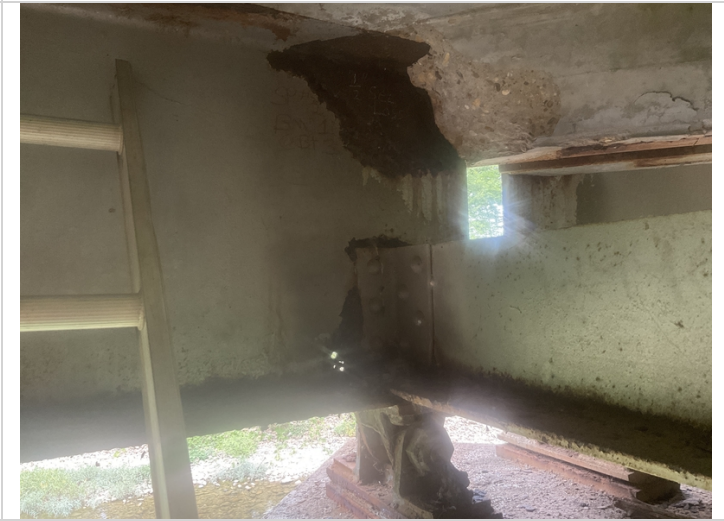
Span 2, Bent 3. Beam 1. Holes in the base of the web.
