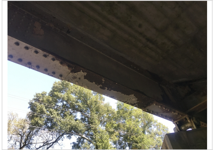
Span # 4, Beam # 1 adjacent to bent # 5 with active corrosion and up to 5/16" section loss.
