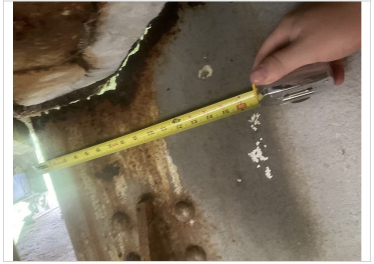
Span 6, Bent 6, Beam 2 - A 13" long X 1/2" tall area rusted through the web of the beam adjacent to the expansion dam.
