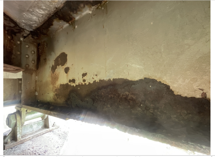
Superstructure has active corrosion with numerous areas of section loss to the webs and flanges of the beams and diaphragms. Section loss ranges from initial up to numerous holes and perforations in the web and bottom flanges.
