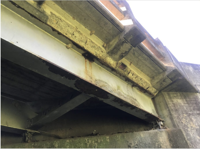
Span # 1 Lt spalling with exposed reinforcing steel on the deck undersurface in the overhang.
