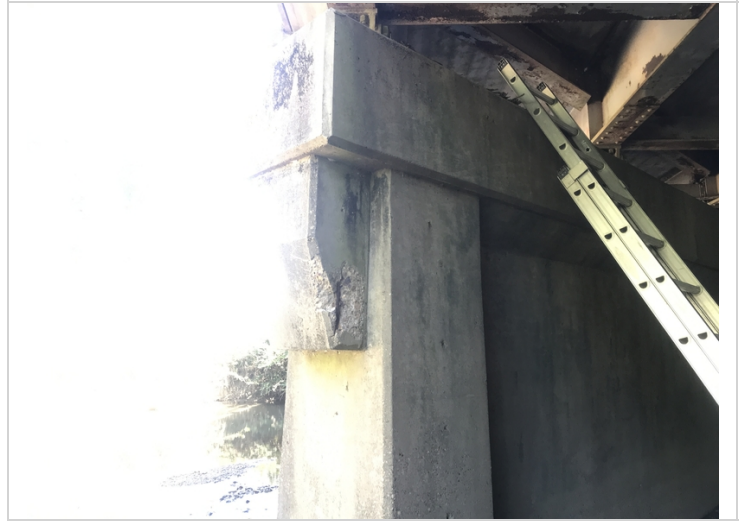
Bent # 4 cap haunch spalling with exposed reinforcing steel.
