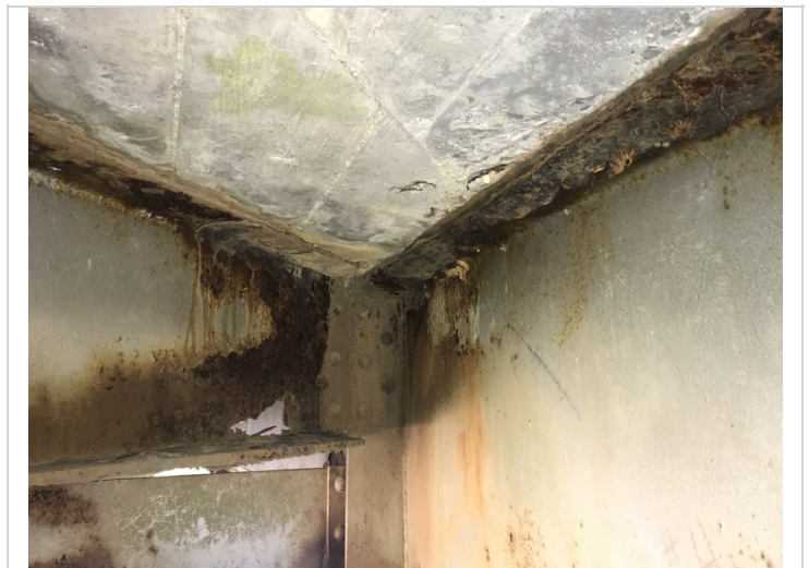
Span #3, Bent # 4 Beam #5 active corrosion with layers of flaking rust, knife edge section loss with a 3/4" reduction in flange width and a hole through the diaphragm.
