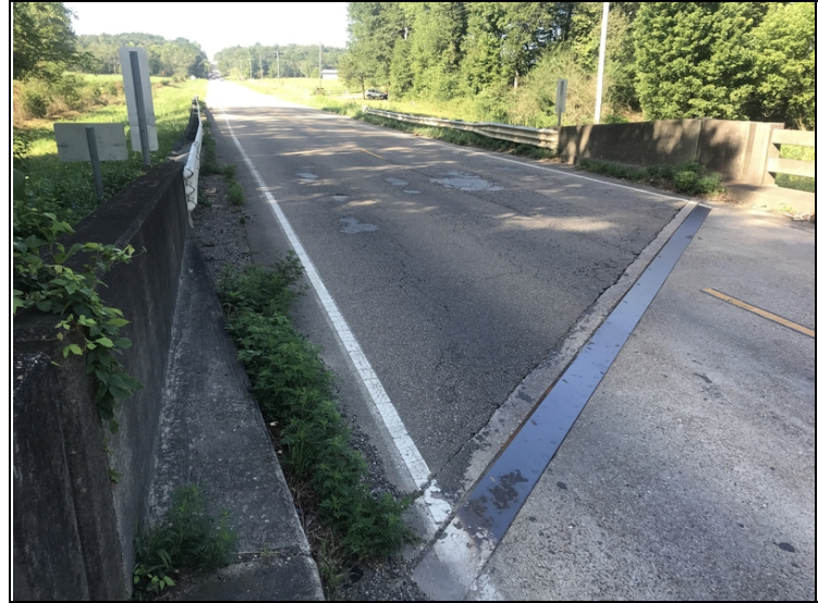
South approach roadway deterioration with potholes.
