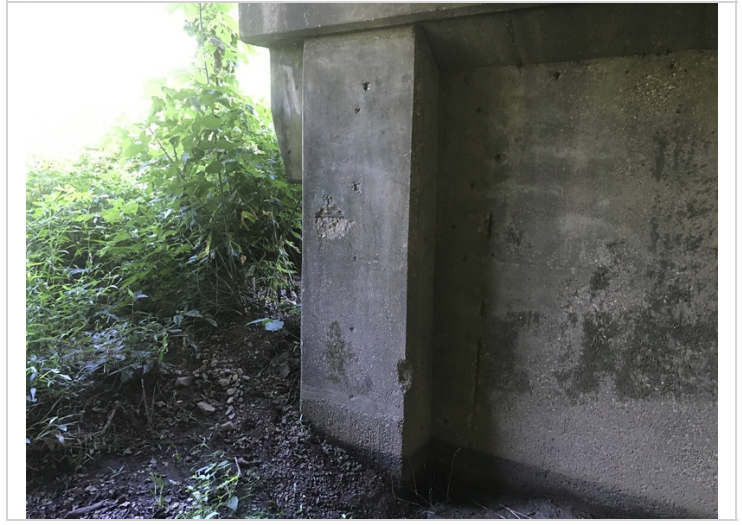
Bent # 2 Column # 1 spalling with exposed reinforcing steel.
