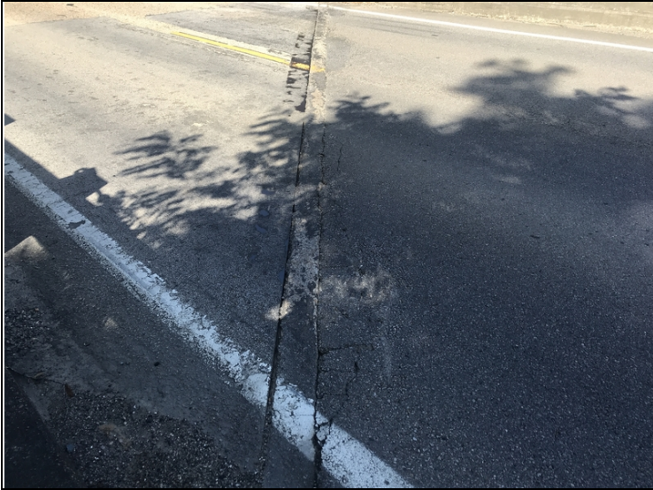
North approach roadway breaking apart at the abutment.
