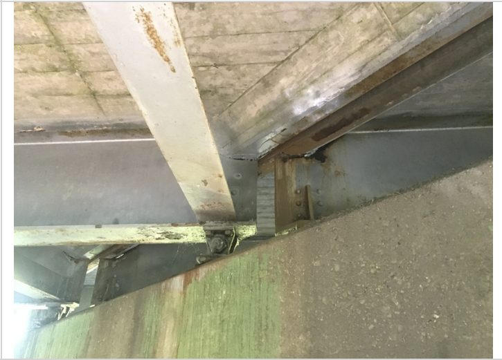
Span # 2, Bent # 2 beam # 2 & 3 with a 4" long hole through the web at the expansion dam.
